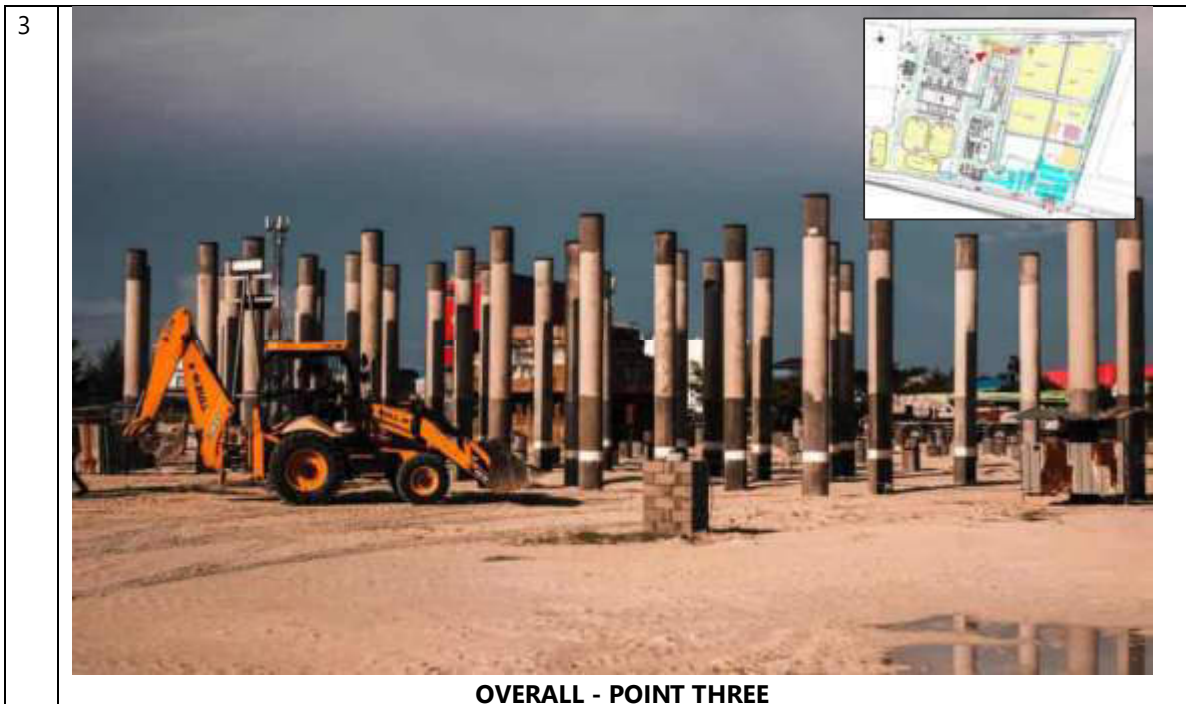
OVERALL - POINT THREE
