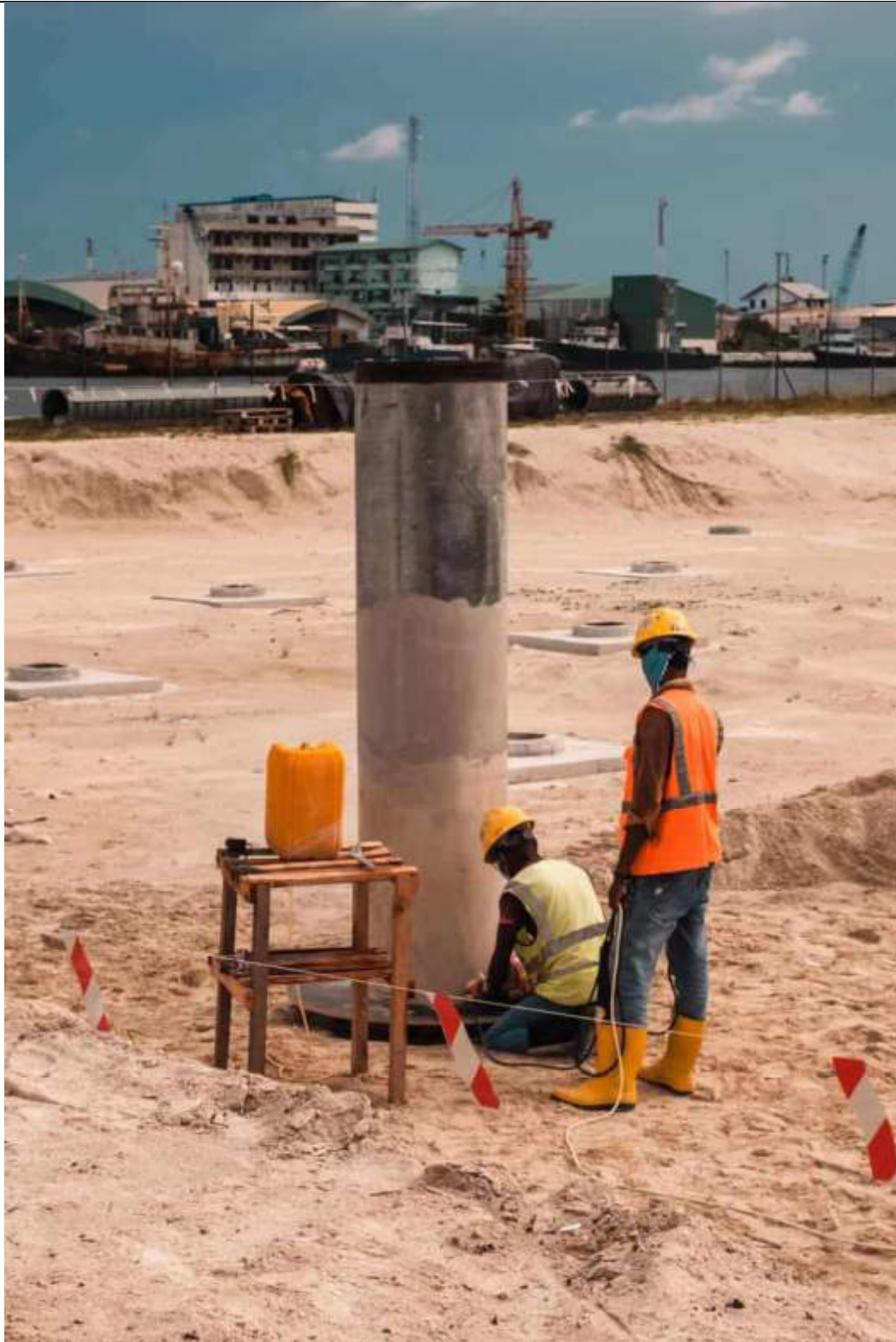
SPUN PILE CUTTING
