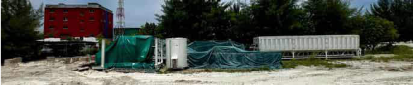
Photo 22 12/10/23 11:34hrs. Batching plant parts and equipment on site.
