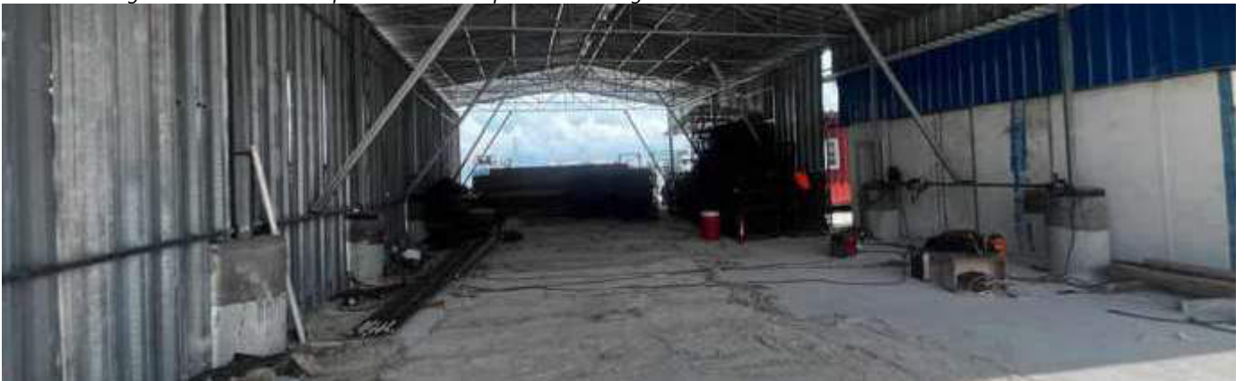
Photo 05 06/11/23 10:59hrs. Reinforcement and formwork assembly work continues.
