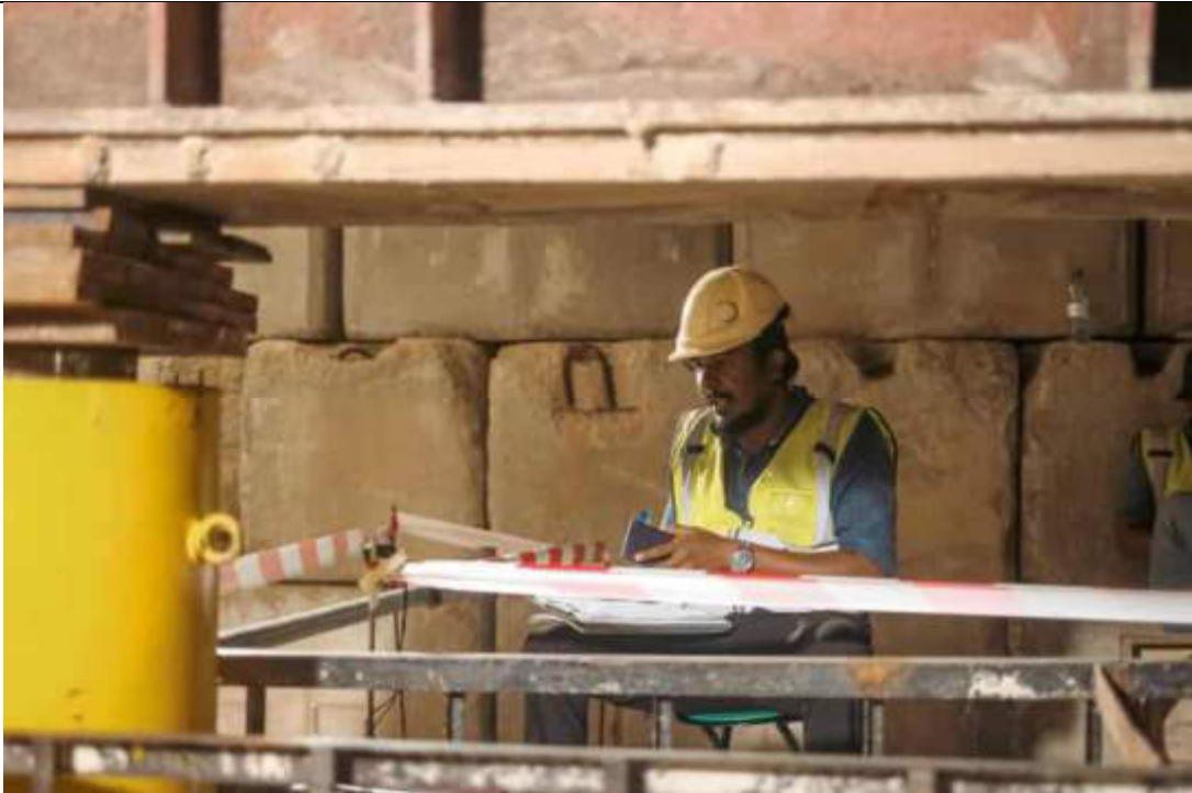
STATIC LOAD TEST FOR SP184
