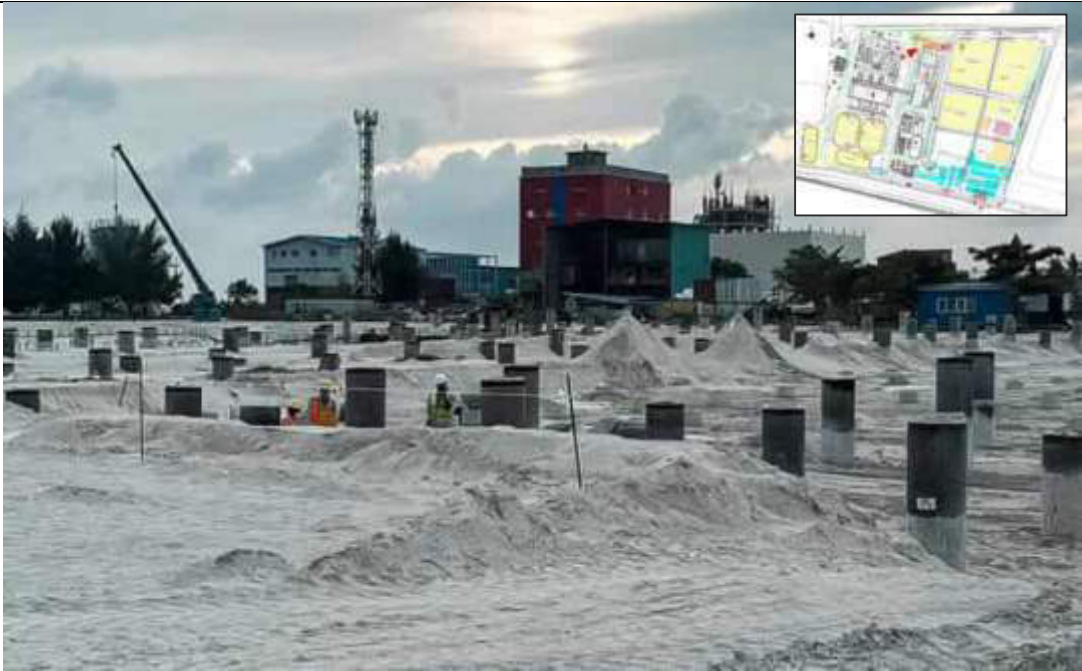
OVERALL - POINT THREE
