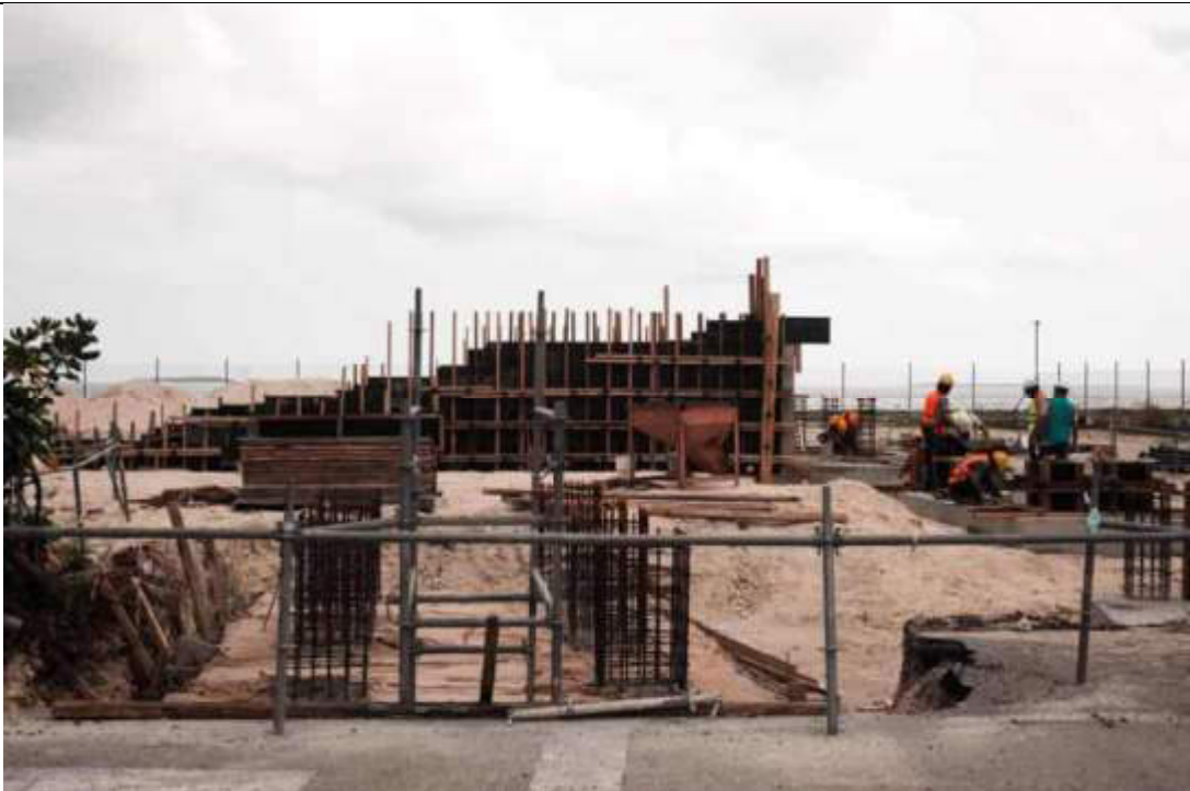
CONSTRUCTION OF TEMPORARY BATCHING PLANT
