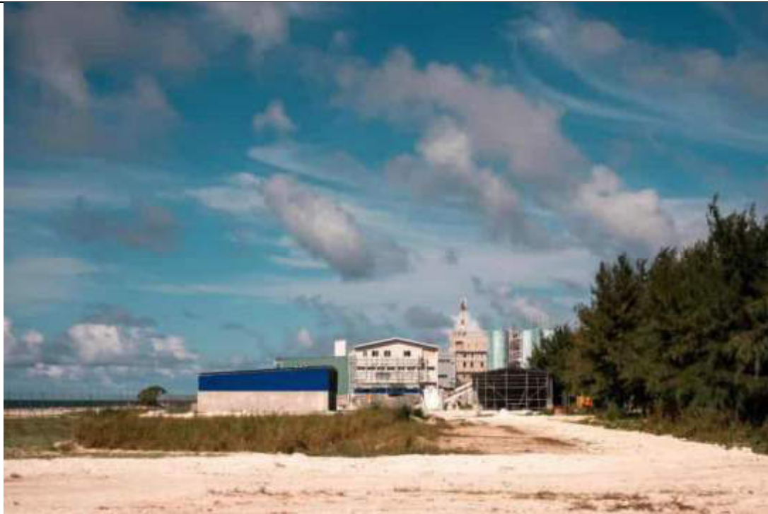
TEMPORARY CONCRETE BATCHING PLANT SETUP
