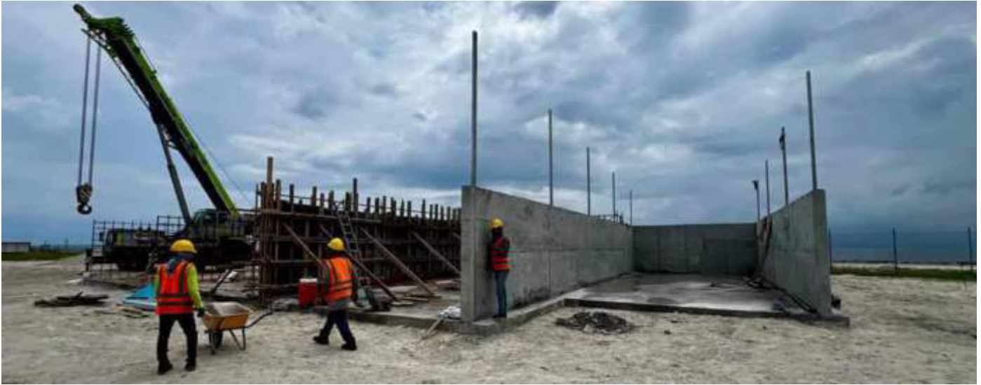
Photo 27 24/10/23 11:19hrs. Concrete works related to the batching plant is ongoing.
