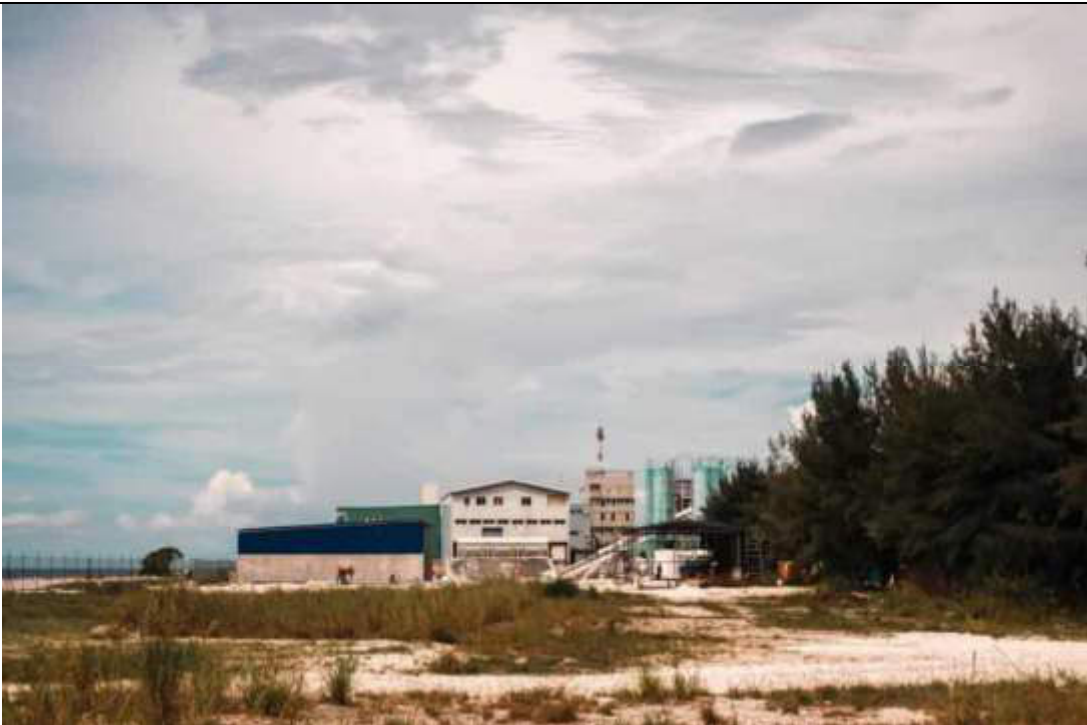
TEMPORARY CONCRETE BATCHING PLANT SETUP
