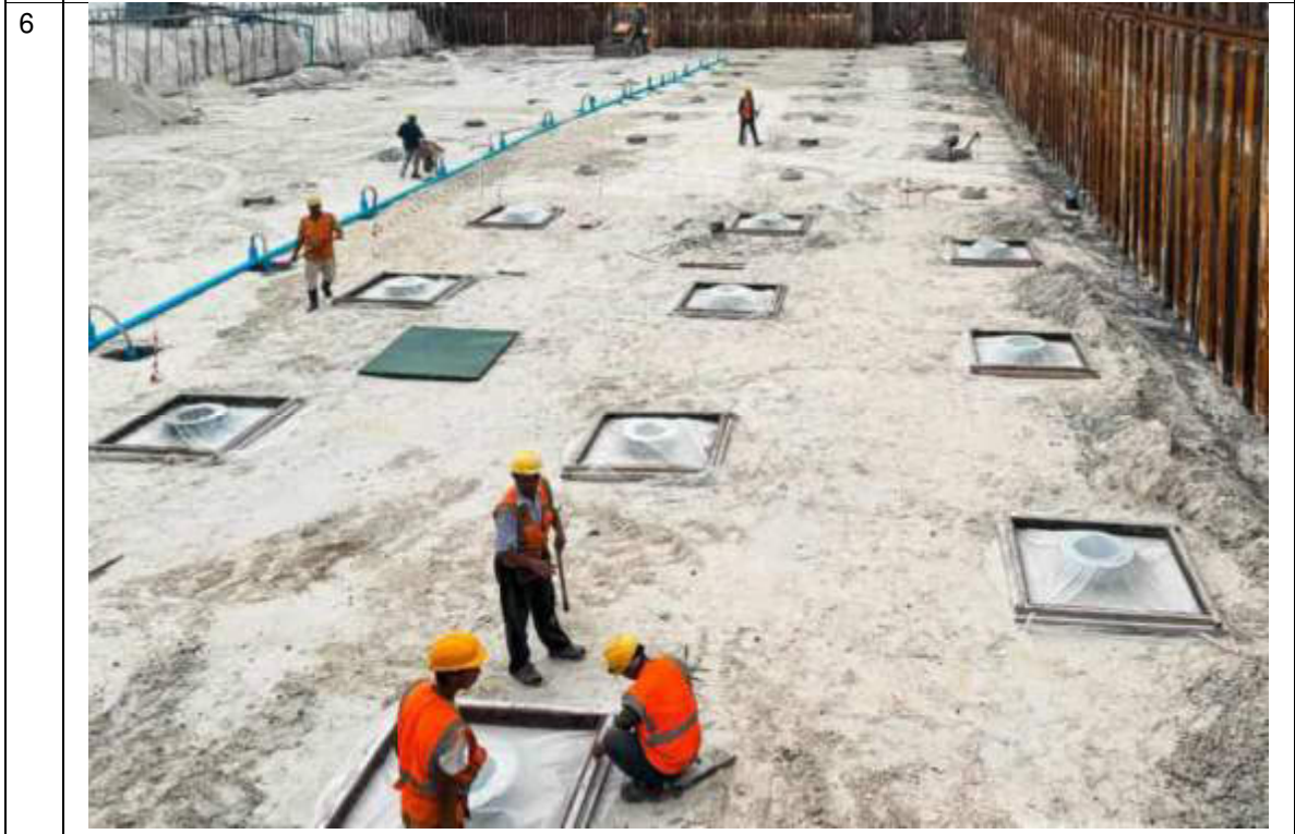
BUNKER DRAINAGE LAYER INSTALLATION IN PROGRESS. LEAN CONCRETE PREPARATION IN PROGRESS.
