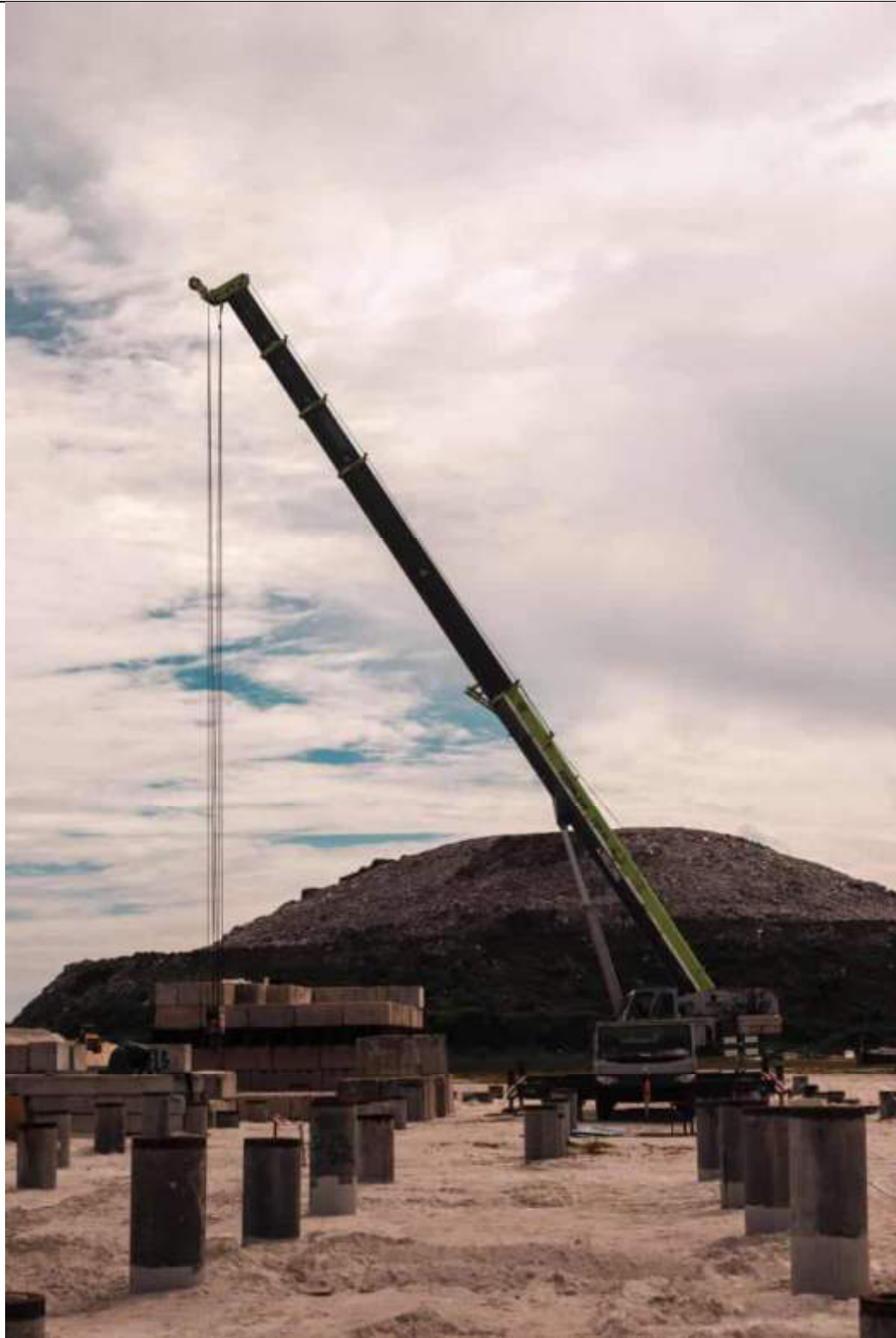
SLT SETUP PREPARATION FOR TURBINE AREA
