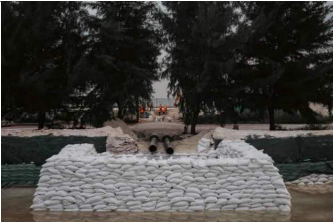
INSTALLATION OF DEWATERING PIPE (DISCHARGE OVERFLOW)
