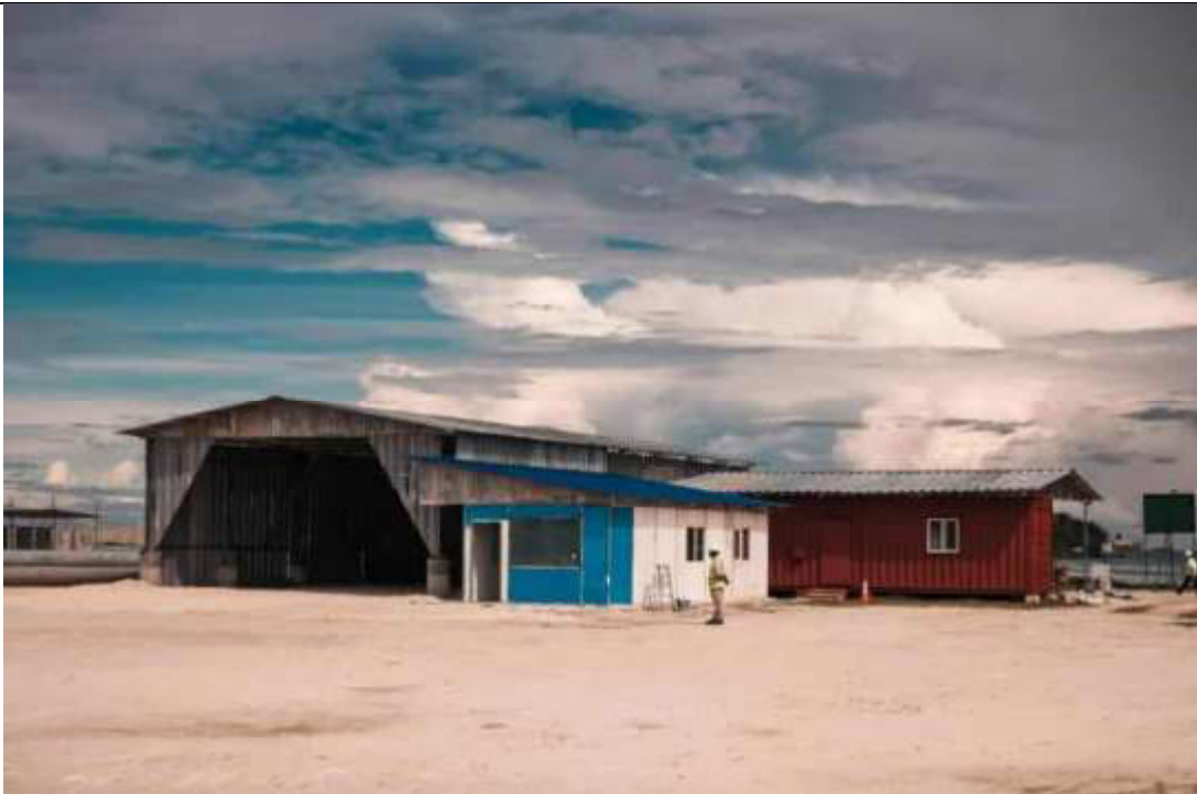
TEMPORARY REINFORCEMENT BAR BENDING & CUTTING YARD
