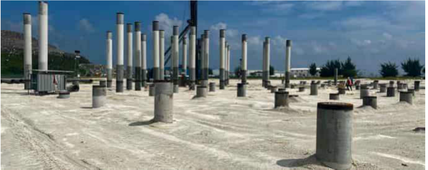
Photo 45 12/10/23 12:07hrs. Process building area, piling works ongoing.
