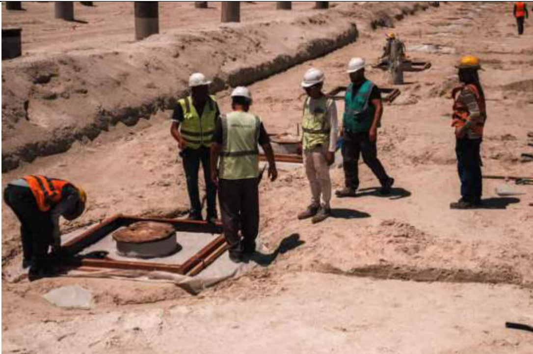
LEAN CONCRETE AT MAIN PROCESS BUILDING
