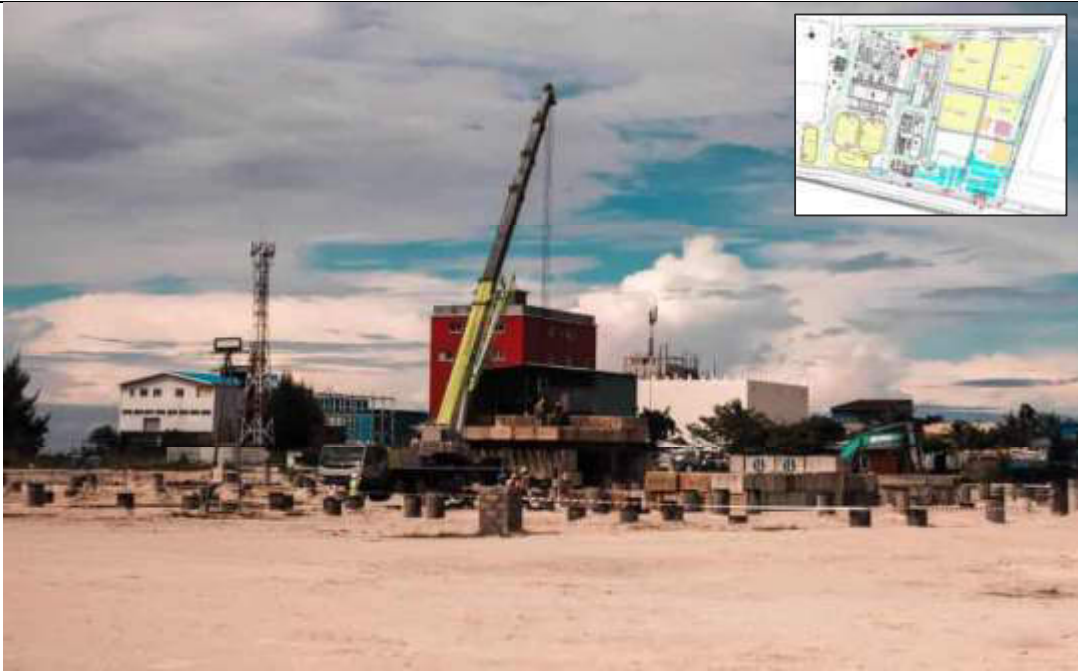
OVERALL - POINT THREE
