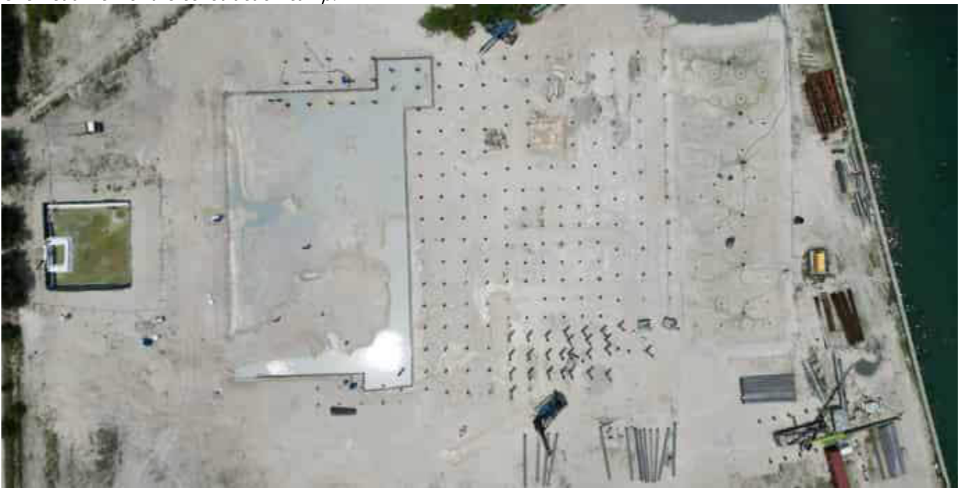
Photo 06 12/10/23 10:55hrs. Overhead view showing the current onsite works.
