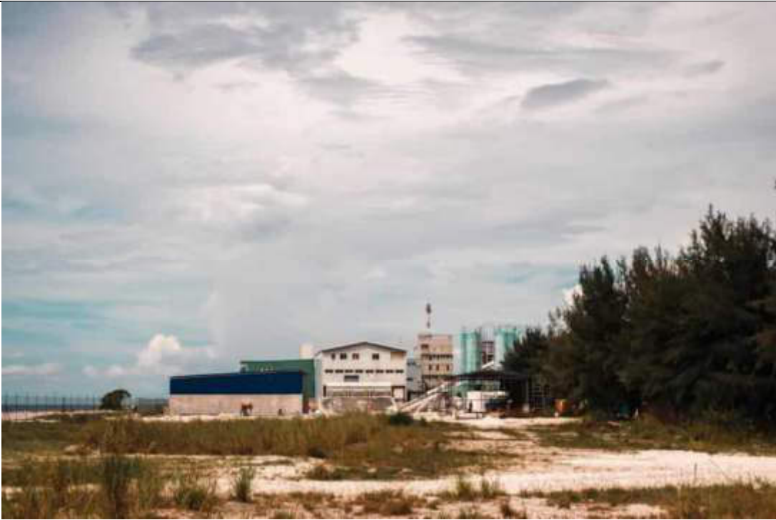
TEMPORARY CONCRETE BATCHING PLANT SETUP
