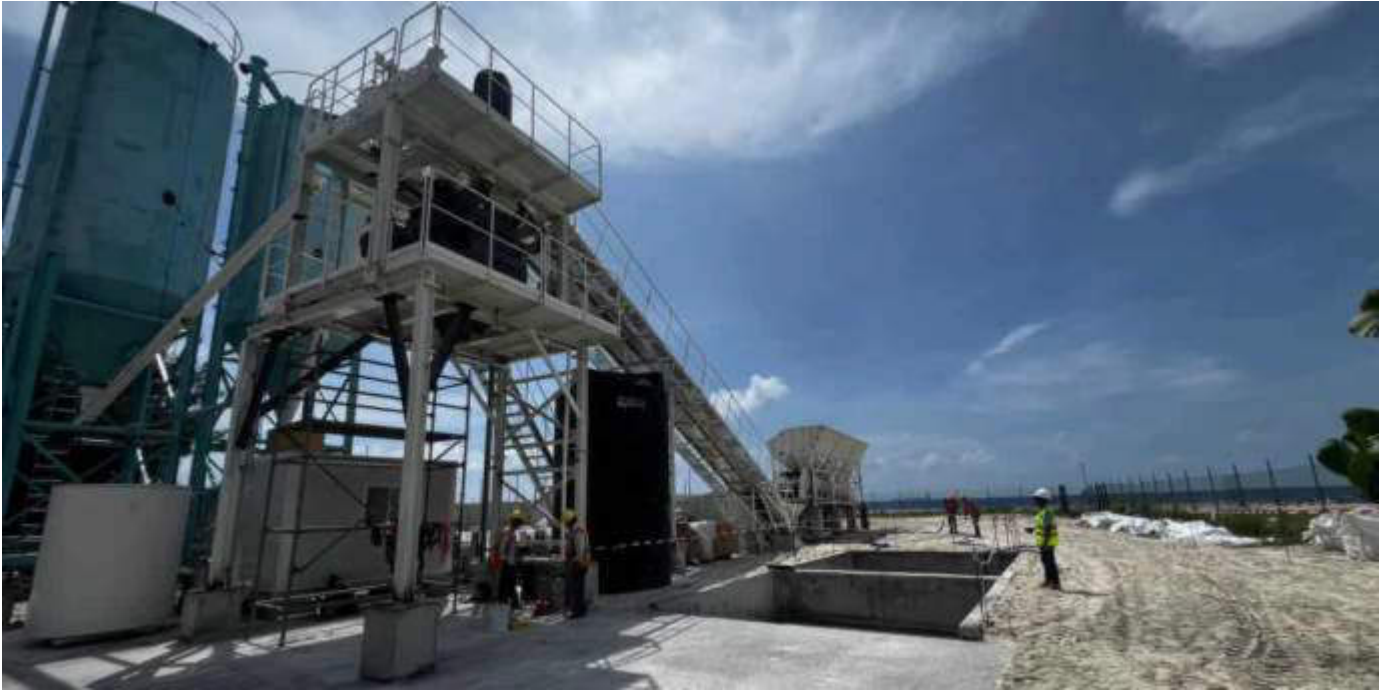
Photo 01 06/11/23 10:36hrs. Installation work on the concrete batching plant is on going.
