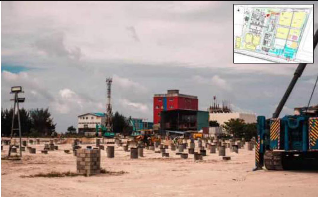
OVERALL - POINT THREE
