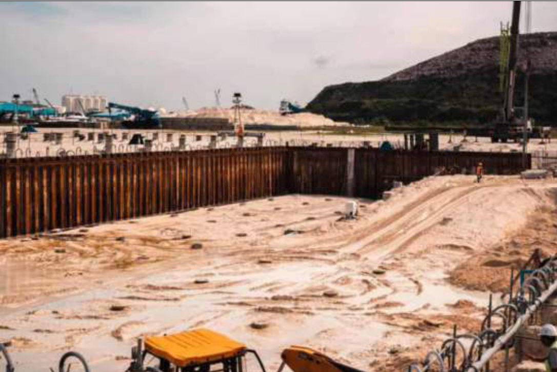
BUNKER EXCAVATION CONTINUE FROM WEST SIDE
