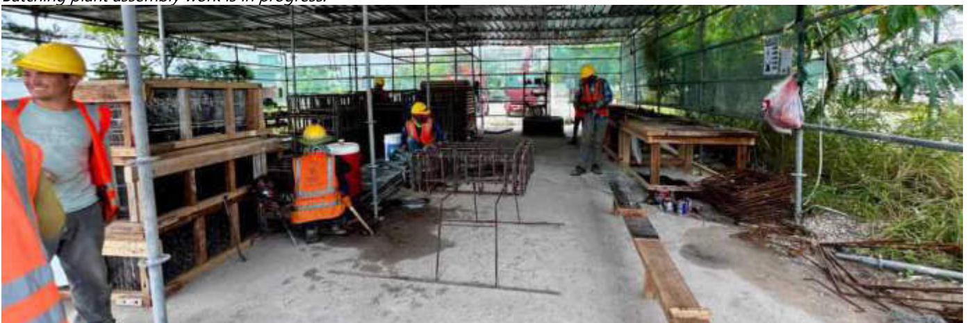
Photo 29 24/10/23 11:19hrs. Barbending work for the batching plant area is in progress.
