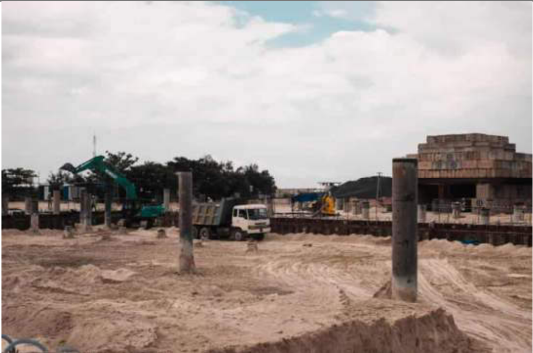
EXCAVATION OF BUNKER AREA
