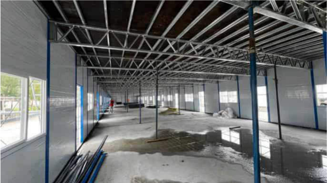
Photo 03 12/10/23 10:40hrs. Inside the new accommodation building for workers.
