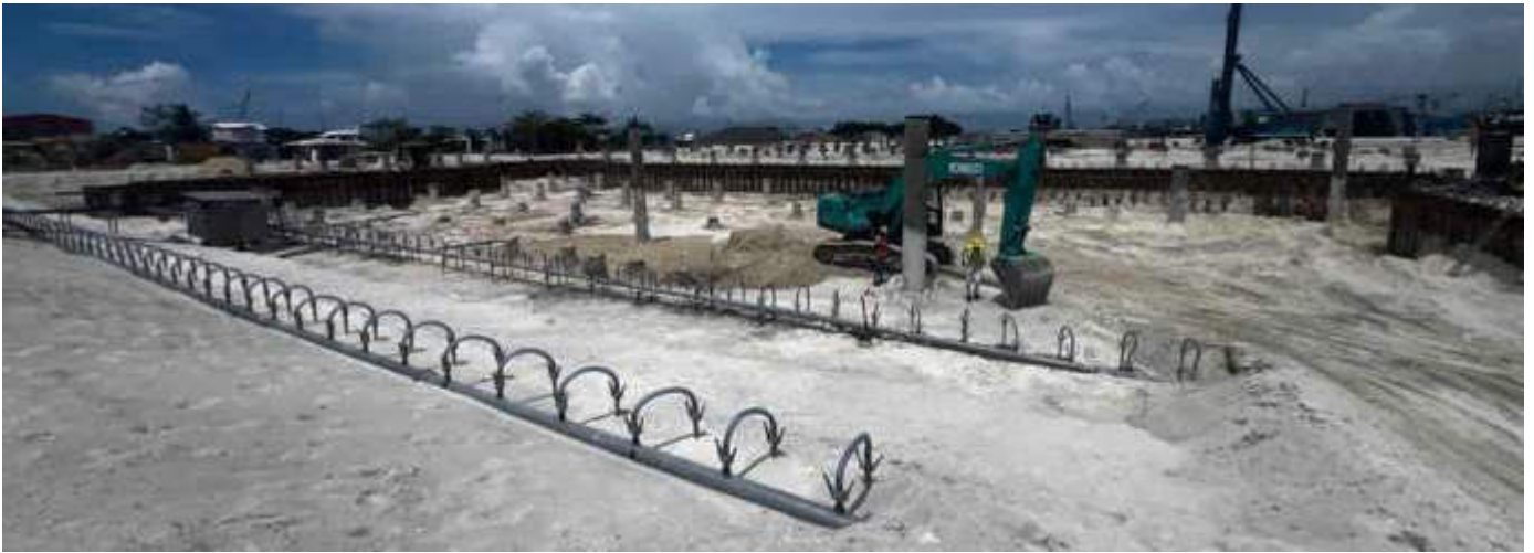
Photo 01 06/11/23 10:36hrs. Excavation work and continuous dewatering of the bunker area continues.
