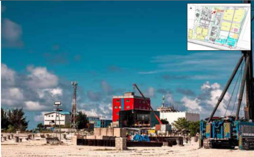
OVERALL - POINT THREE
