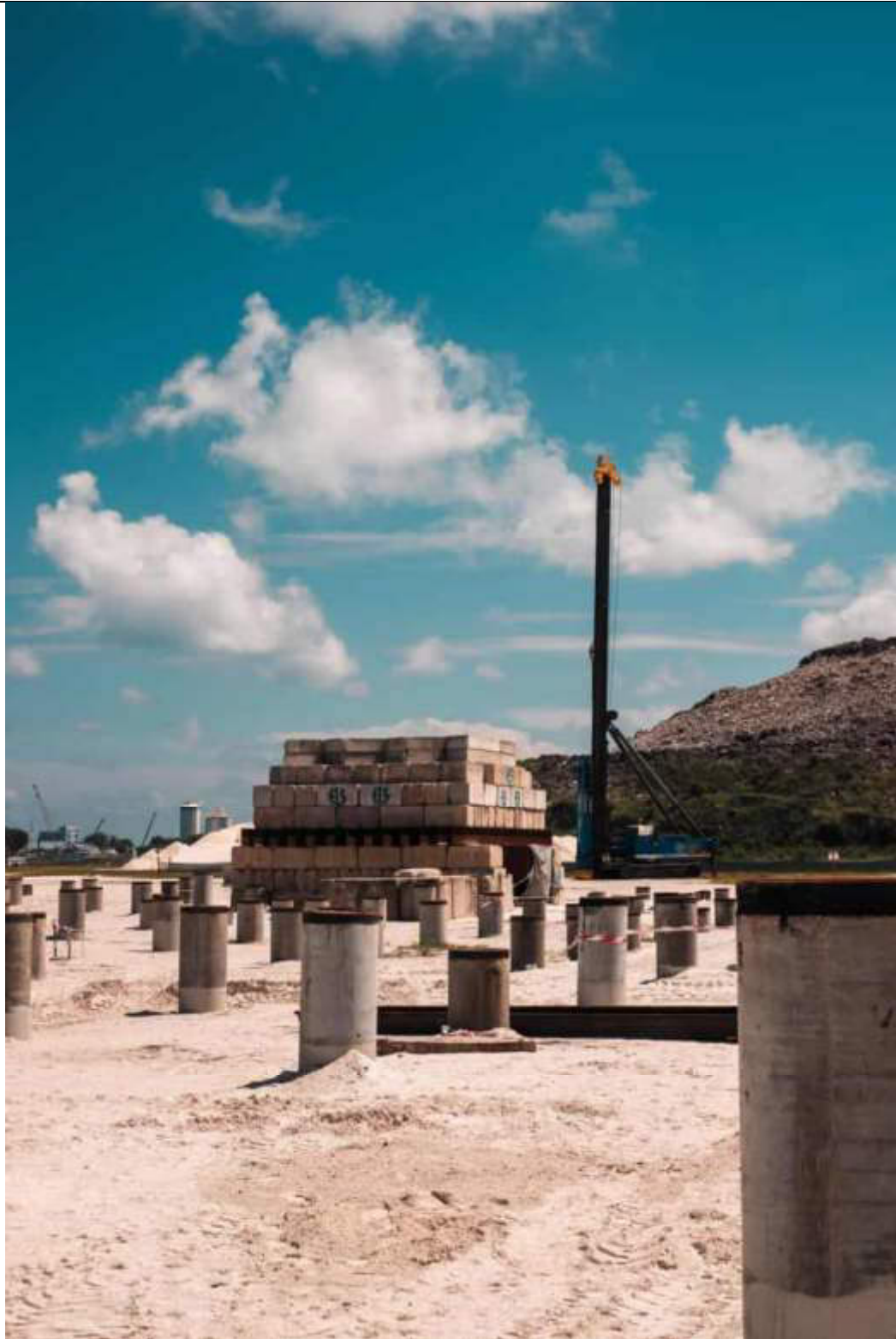
SLT SETUP PREPARATION FOR TURBINE AREA
