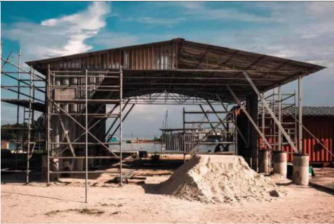
TEMPORARY REINFORCEMENT BAR BENDING YARD
