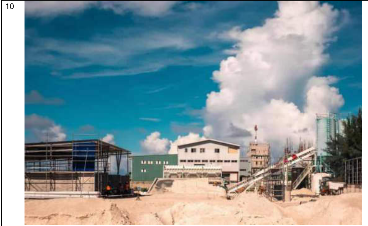
TEMPORARY CONCRETE BATCHING PLANT SETUP
