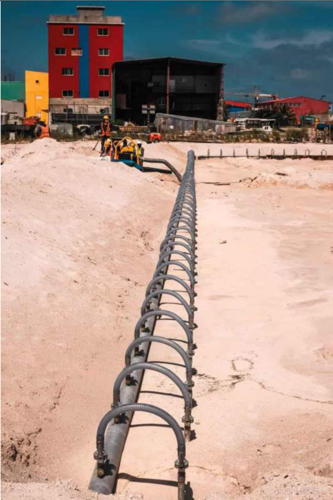
INSTALLATION OF DEWATERING PIPE AT BUNKER AREA (Line 3 of 3)
