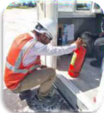
Fire Extinguisher Inspection
