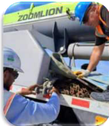
Lifting slings Inspection
