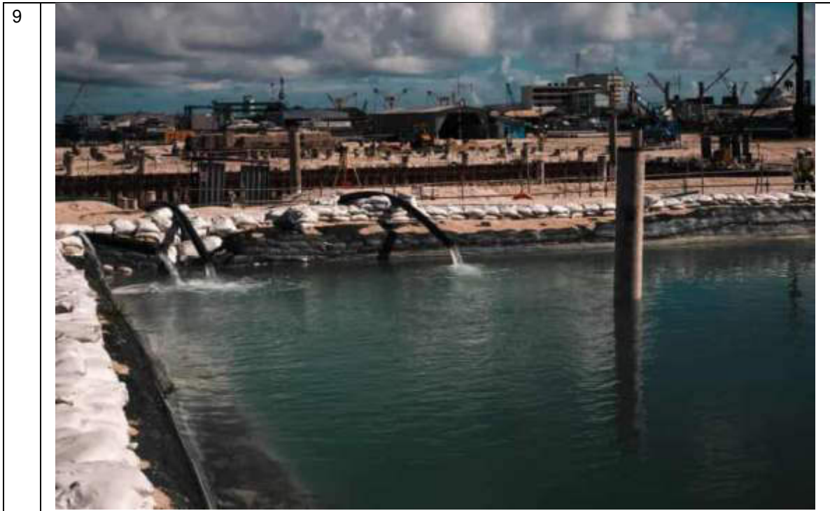
BUNKER AREA DEWATERING CONTINUE
