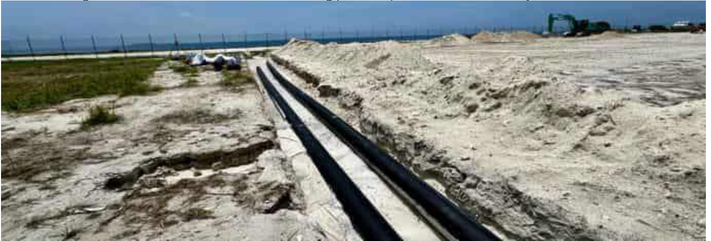
Photo 15 12/10/23 11:25hrs. Dewatering pipeline laying work ongoing.
