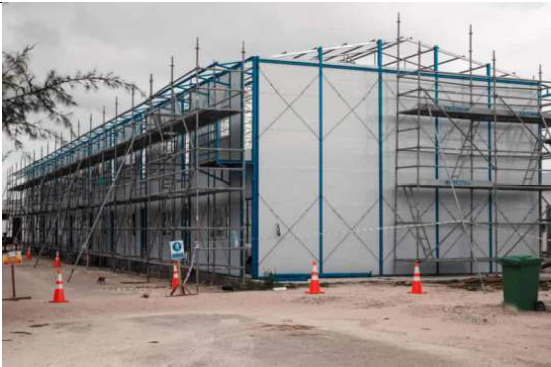
ERECTION OF WORKER'S ACCOMMODATION
