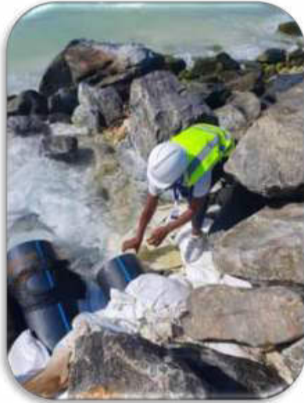
Dewatering Discharge
