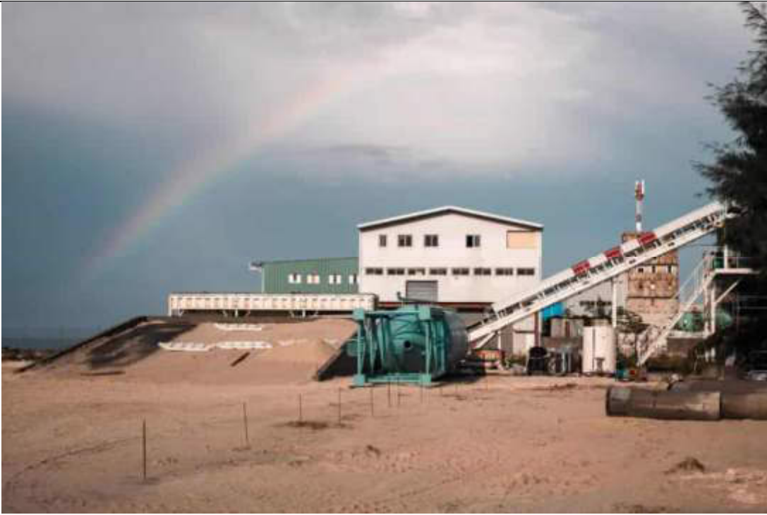
TEMPORARY CONCRETE BATCHING PLANT SETUP
