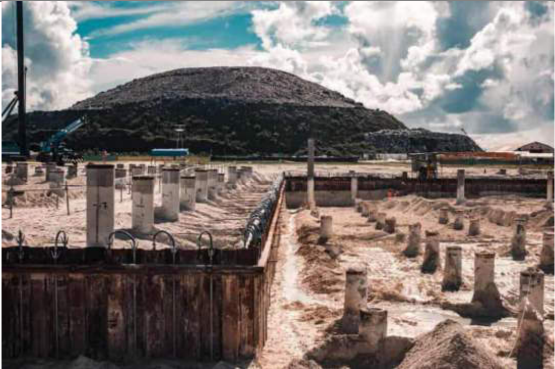
IMPROVEMENT OF SHEETPILE ANCHORAGE SYSTEM
