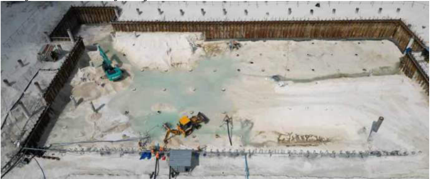
Photo 16 13/12/23 13:25hrs. Excavation work in the bunker area is ongoing.
