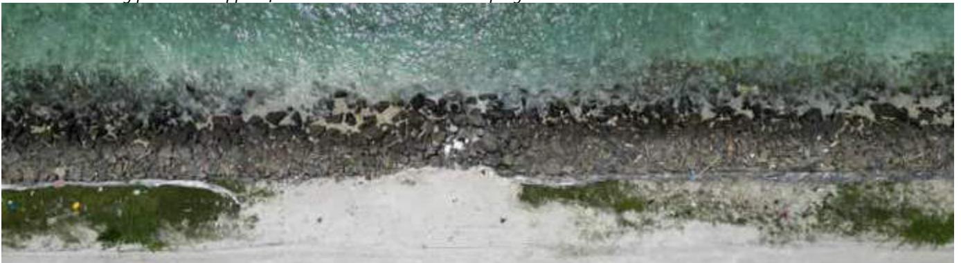
Photo 13 06/11/23 11:19hrs. Dewatering outfall to sea, no visible change seen to the surrounding.
