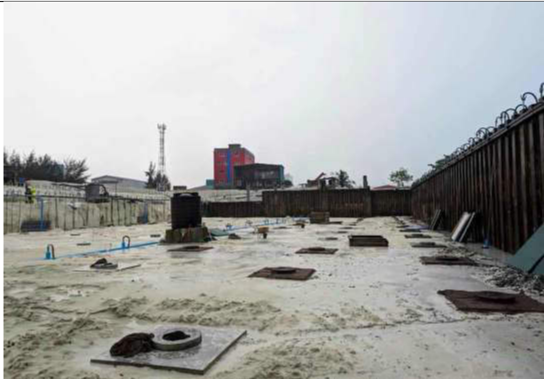
BUNKER DRAINAGE LAYER COMPLETED. 24 NOS LEAN CONCRETE COMPLETED.
