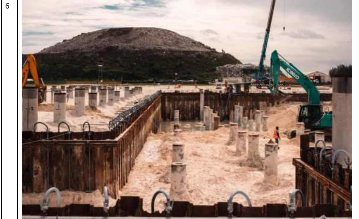
BUNKER EXCAVATION CONTINUE FROM WEST SIDE
