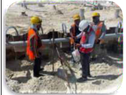
Hand tools Inspection
