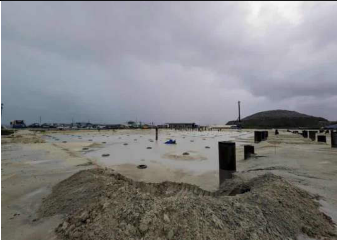
MAIN PROCESS BUILDING & TURBINE (SECOND PHASE) EXCAVATION.
