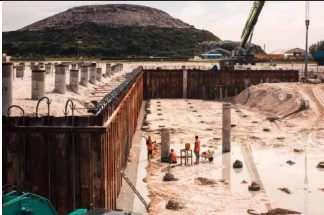
DRAINAGE LAYER BUNKER AREA
