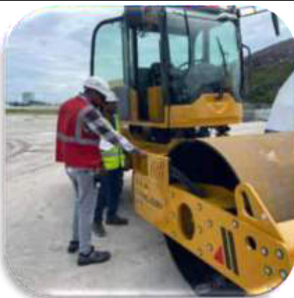
Plant and Equipment Inspection
