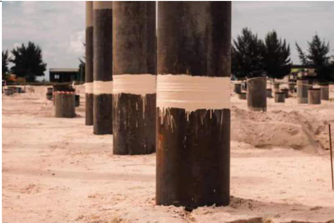
SPUN PILE WELDING COATING
