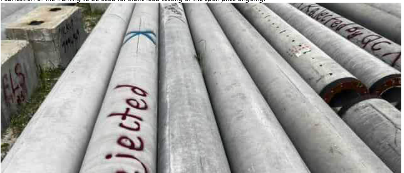
Photo 47 12/10/23 12:09hrs. Rejected spunpiles clearly marked and put aside.
