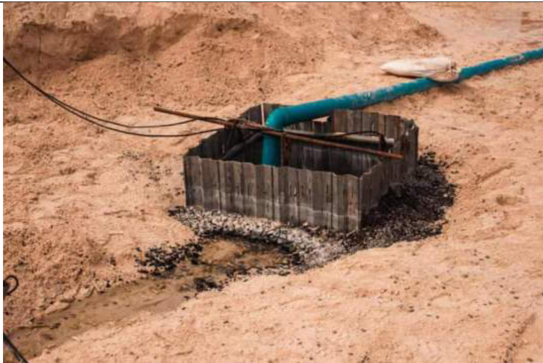
DRAINAGE LAYER BUNKER AREA
