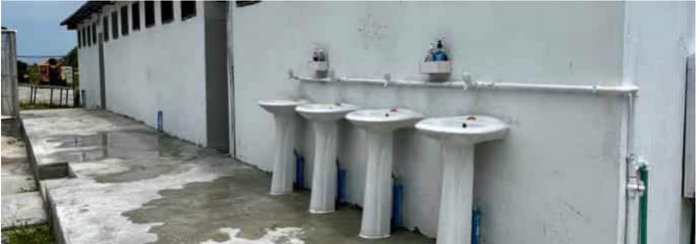
Photo 31 12/10/23 11:47hrs. Handwash area at the workers mess hall kept clean.
