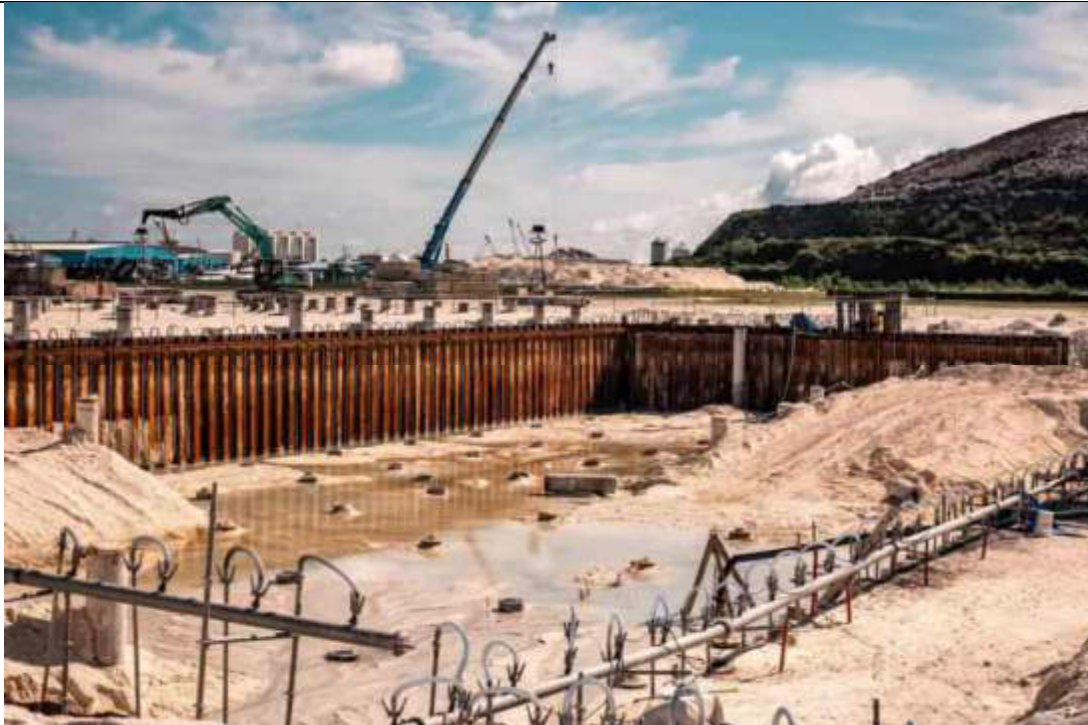
BUNKER EXCAVATION CONTINUE FROM WEST SIDE
