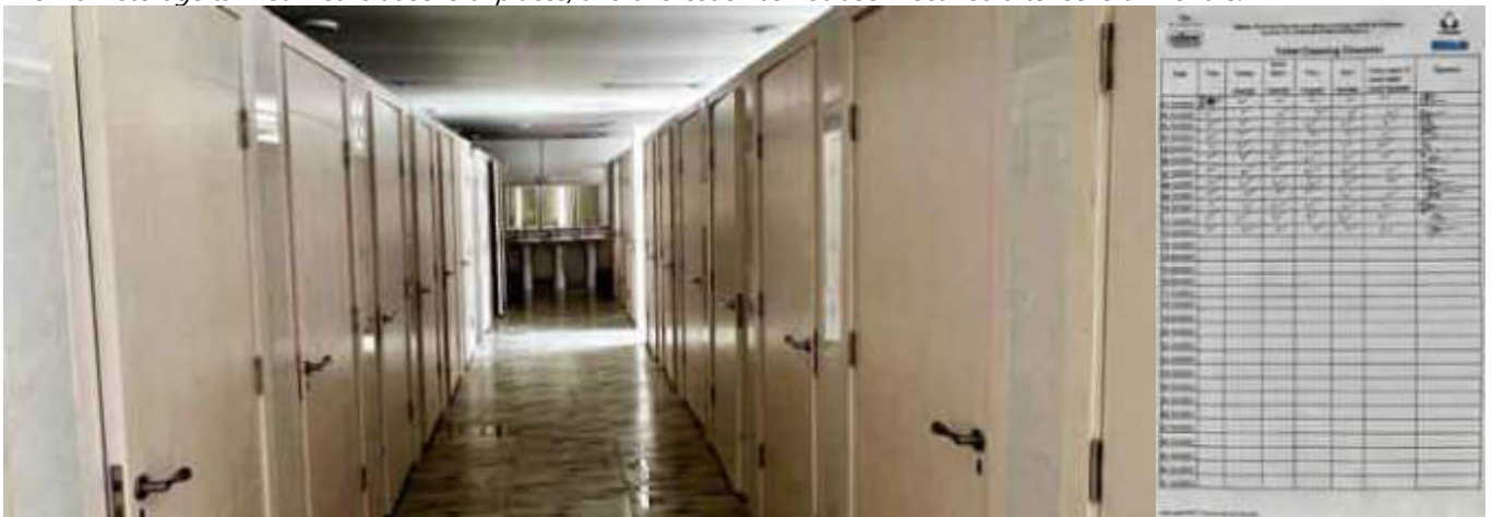
Photo 30 12/10/23 11:45hrs. The main toilet block has been completed and is in use, kept clean and cleaning log maintained.
