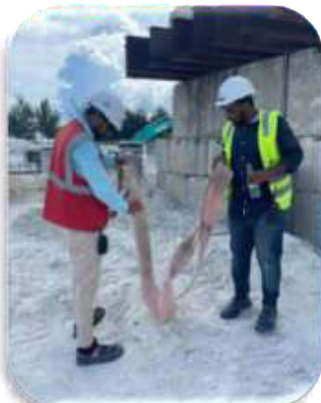
Lifting slings Inspection
