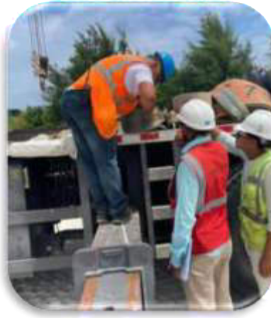
Lifting slings Inspection
