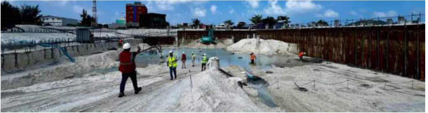
Photo 05 13/12/23 10:52hrs. Reinforcement and formwork assembly work continues.
