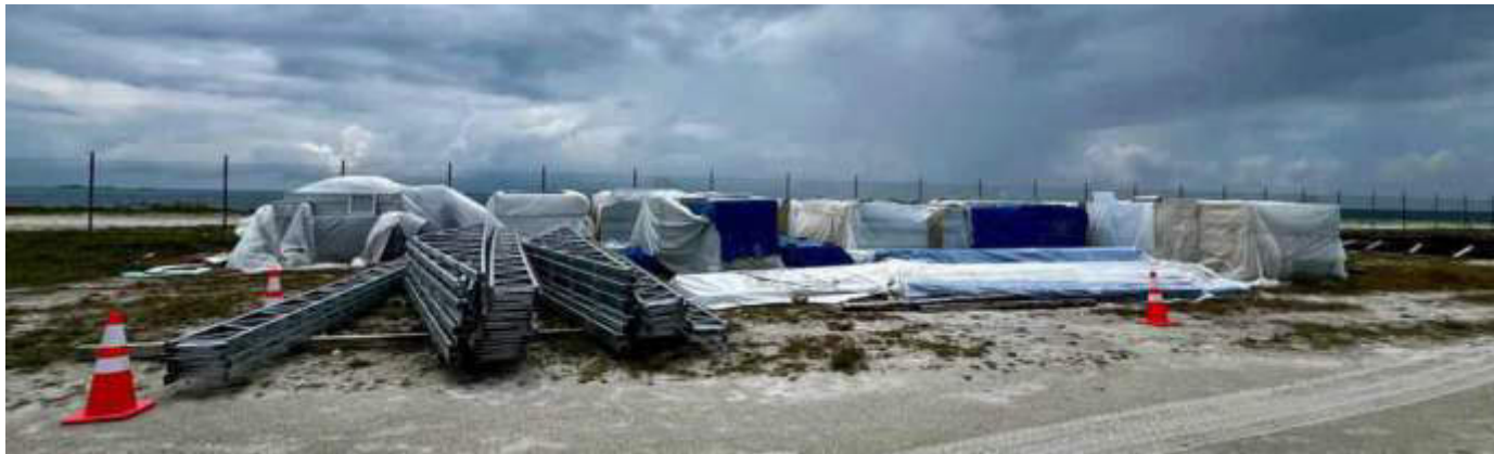
Photo 24 24/10/23 11:19hrs. Materials for new workers accommodation on site.
