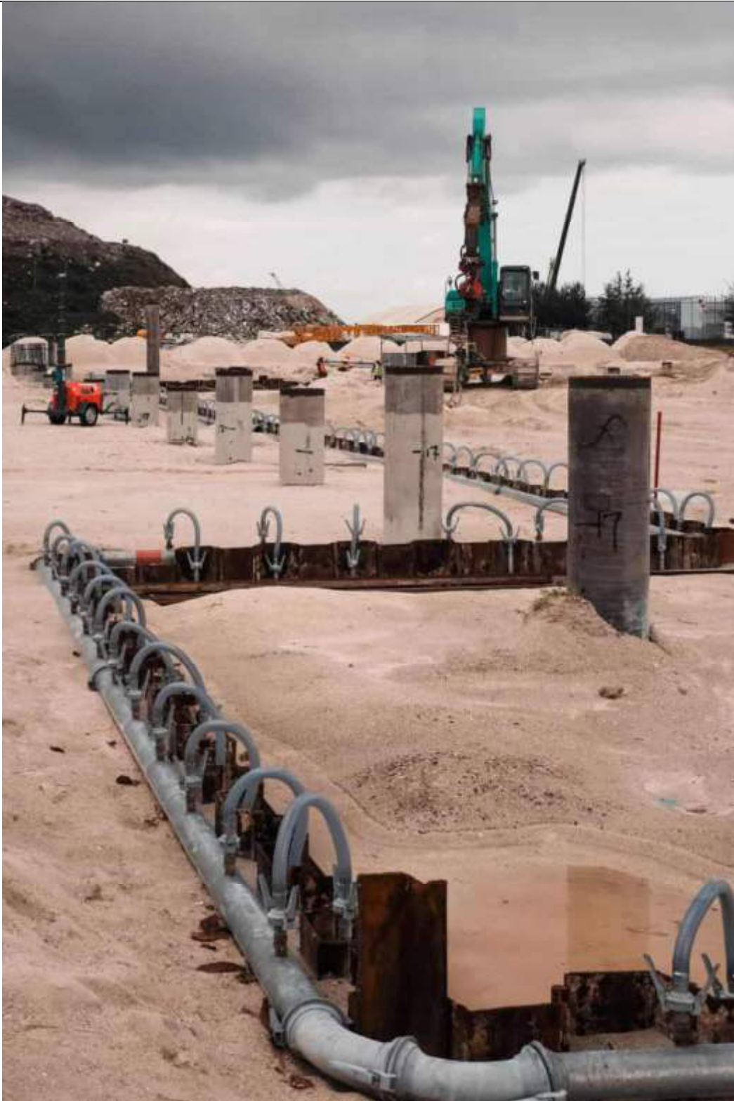
INSTALLATION OF DEWATERING PIPE AT BUNKER AREA (Line 1 of 3)
