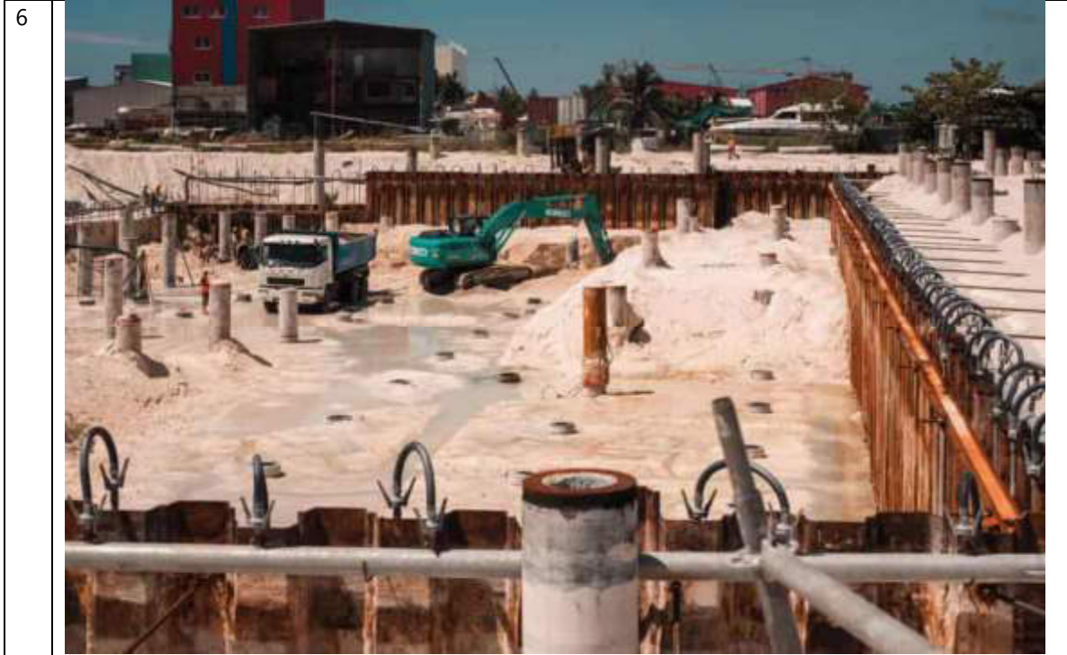
BUNKER EXCAVATION CONTINUE FROM WEST SIDE
