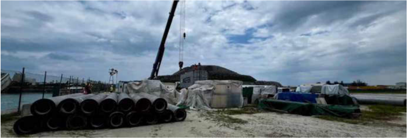
Photo 10 24/10/23 14:02hrs. Laydown area close to the sea side entrance gate.
