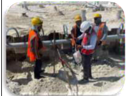
Hand tools Inspection
