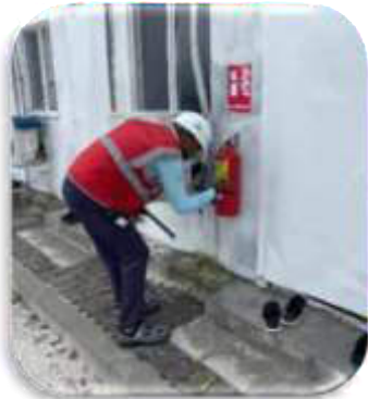
Fire Extinguisher Inspection
