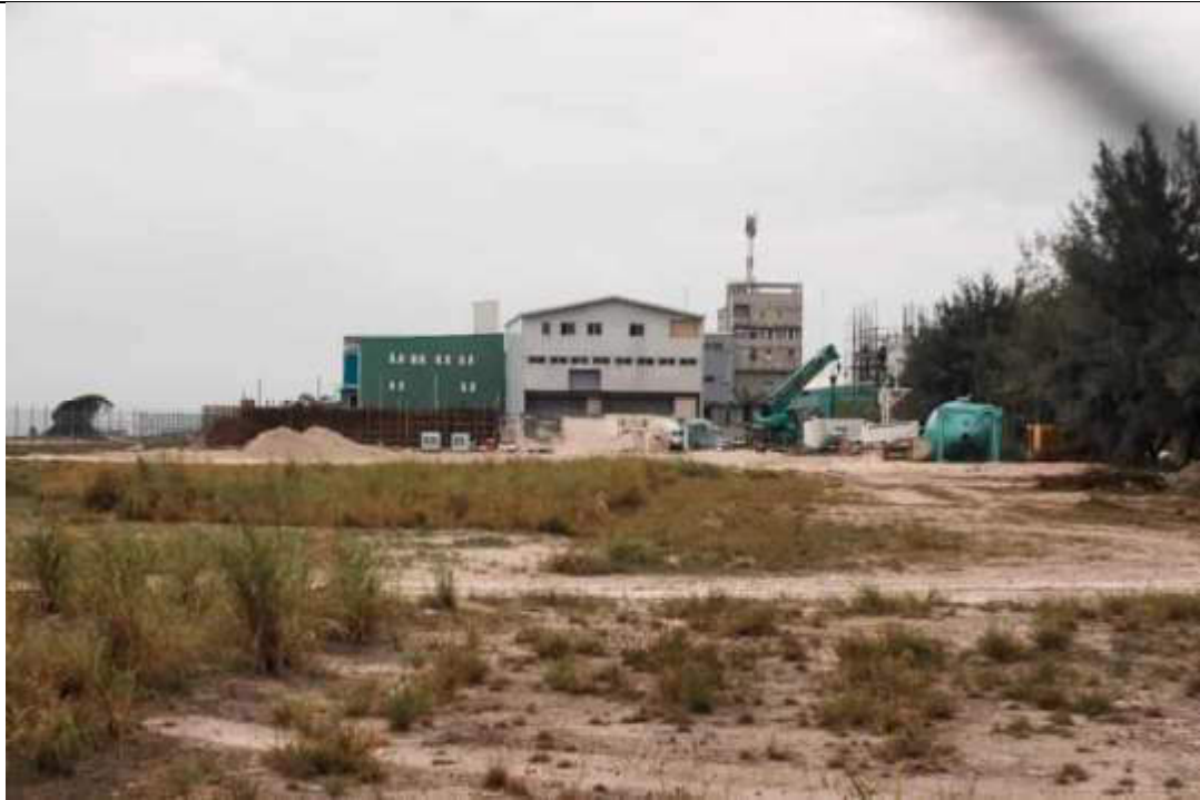
SETTING UP TEMPORARY BATCHING PLANT
