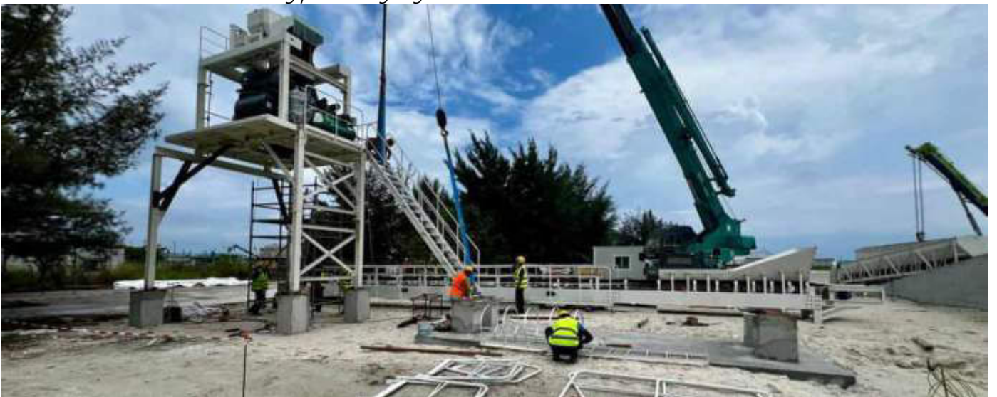
Photo 28 24/10/23 11:19hrs. Batching plant assembly work is in progress.
