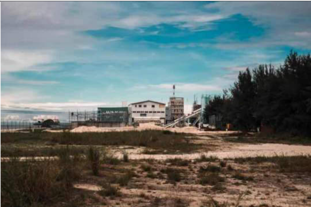
TEMPORARY CONCRETE BATCHING PLANT SETUP
