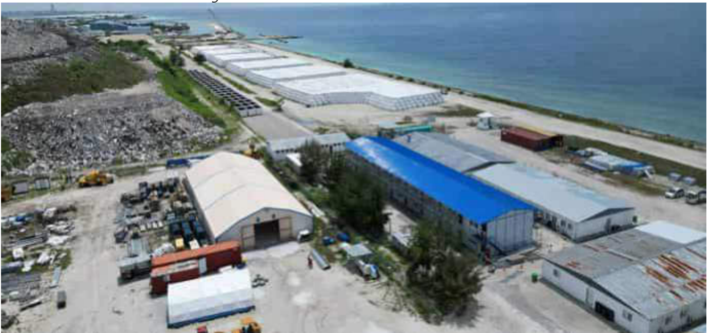
Photo 04 12/10/23 10:45hrs. Storage area, Construction camp view and the WAMCO landfill area and the Bale stacking area. The landfill corner is very close to the site boundary fence, and is currently being used. The bales are now placed about 26m from the site boundary fence.
