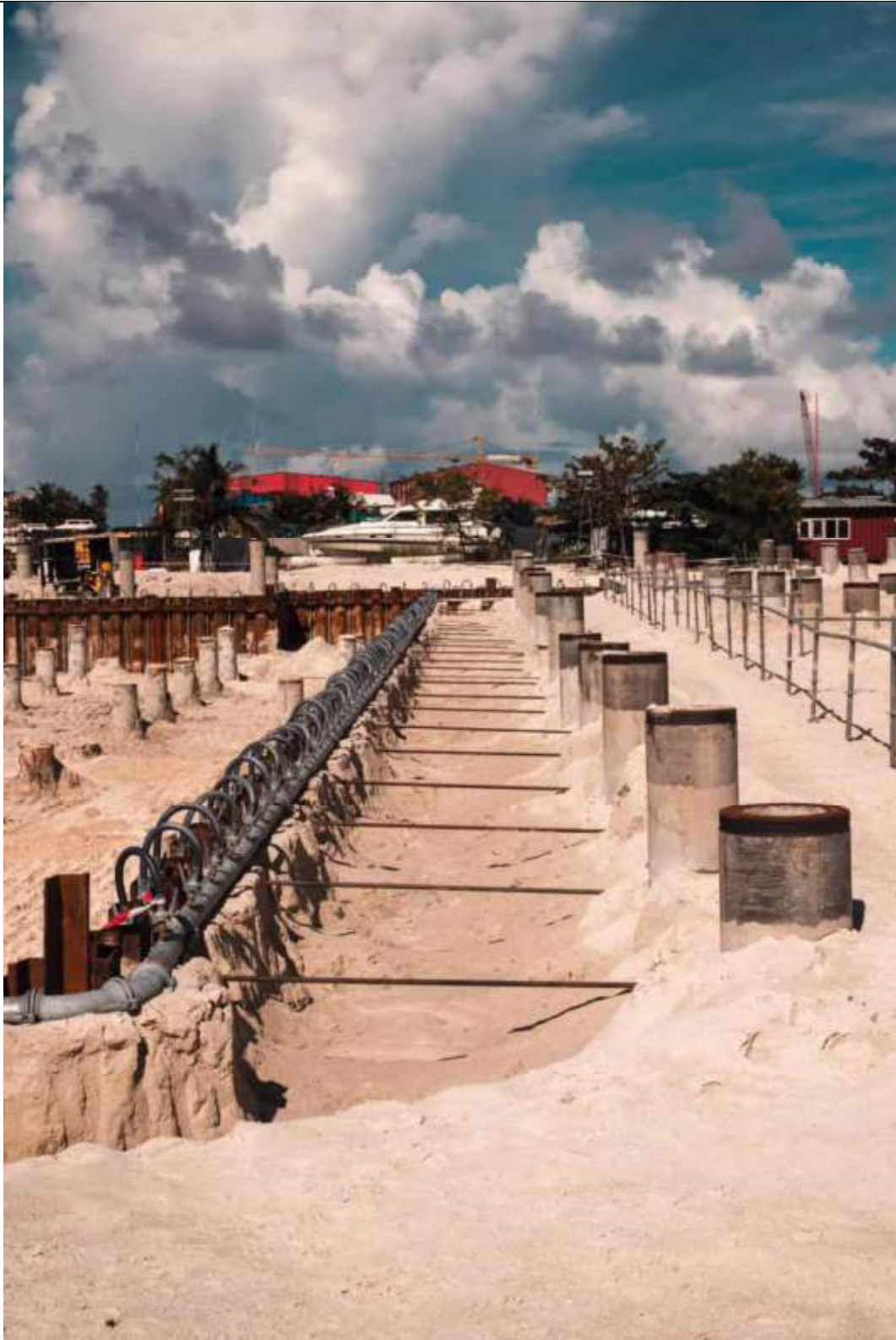
IMPROVEMENT OF SHEETPILE ANCHORAGE SYSTEM
