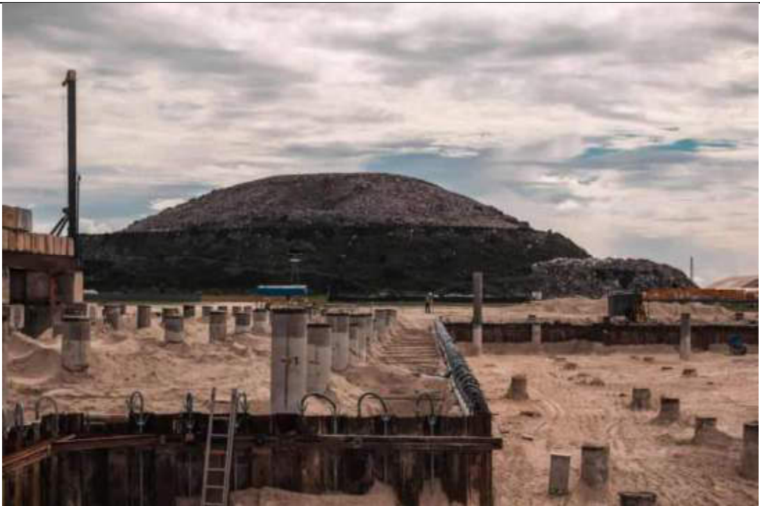
EXCAVATION OF BUNKER AREA
