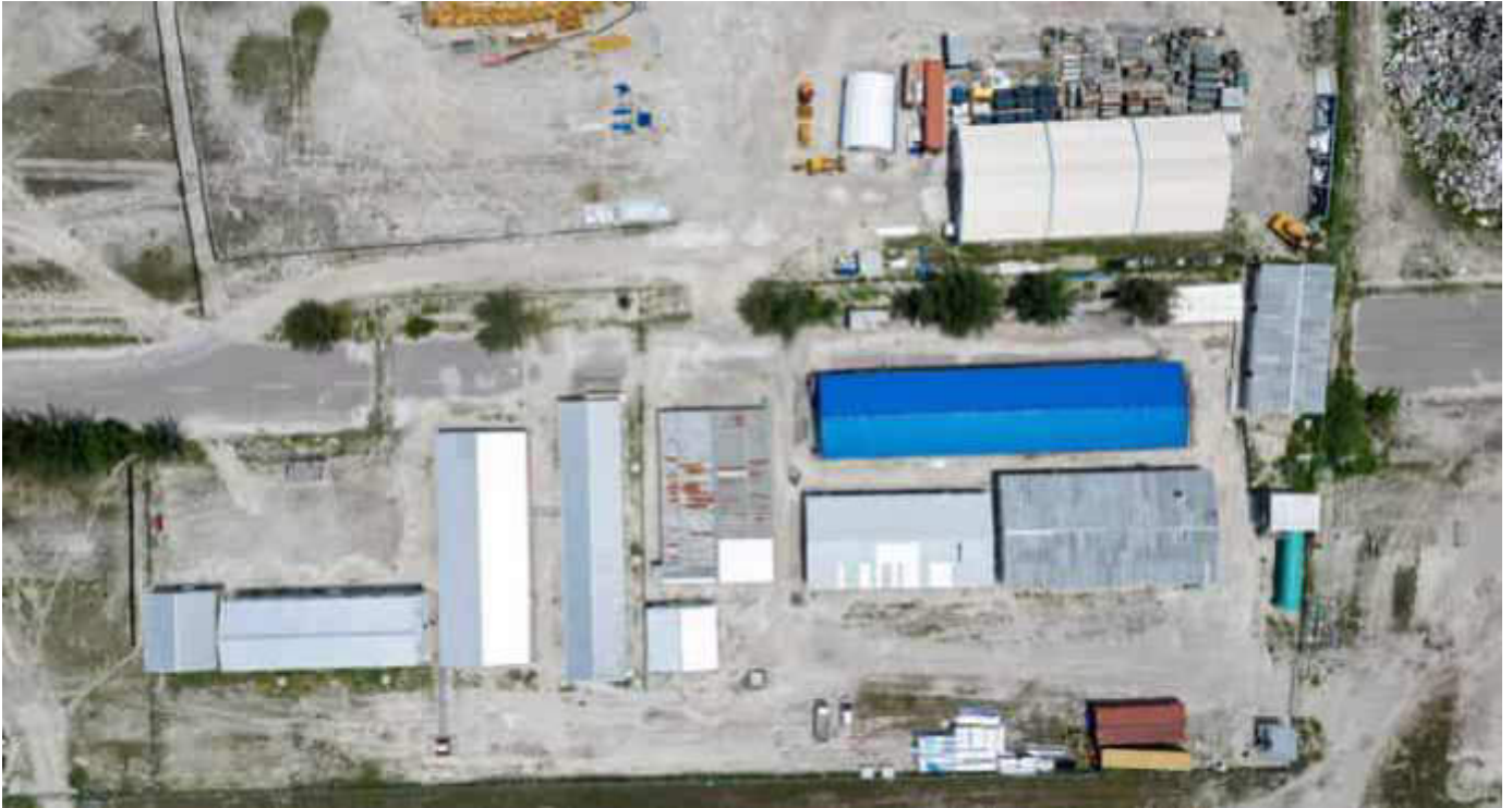
Photo 05 12/10/23 10:50hrs. Overhead view of the construction camp.
