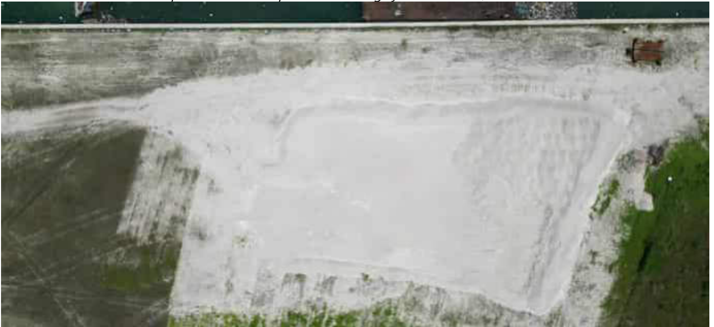
Photo 08 12/10/23 11:08hrs. Overhead view of the excavated soil stored in the laydown area, within the site boundary.
