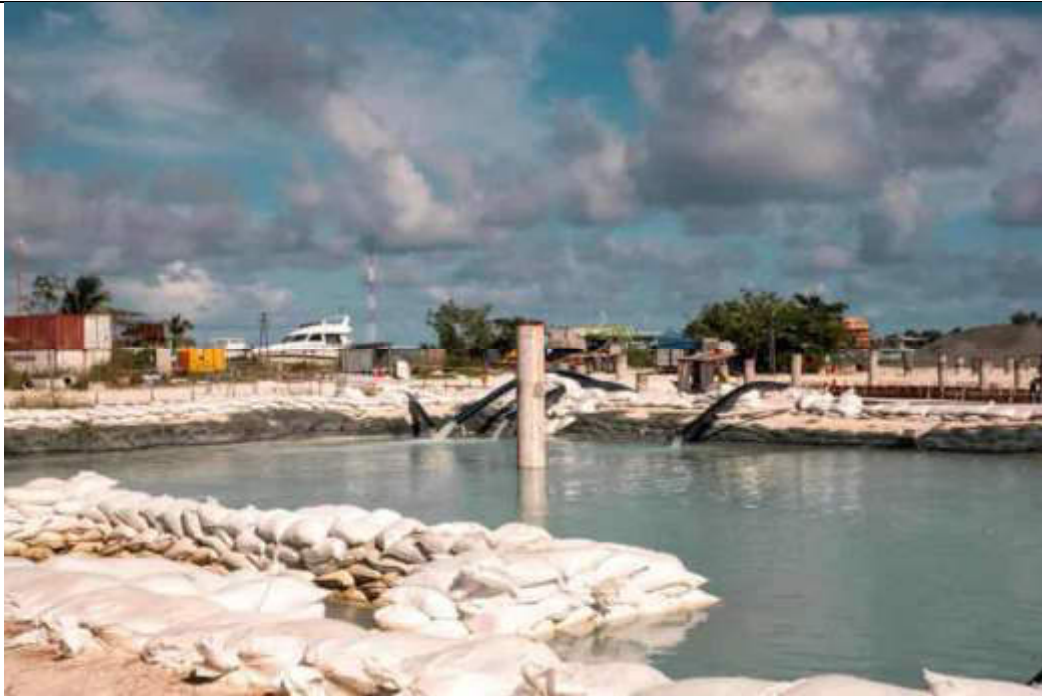
DEWATERING BUNKER AREA
