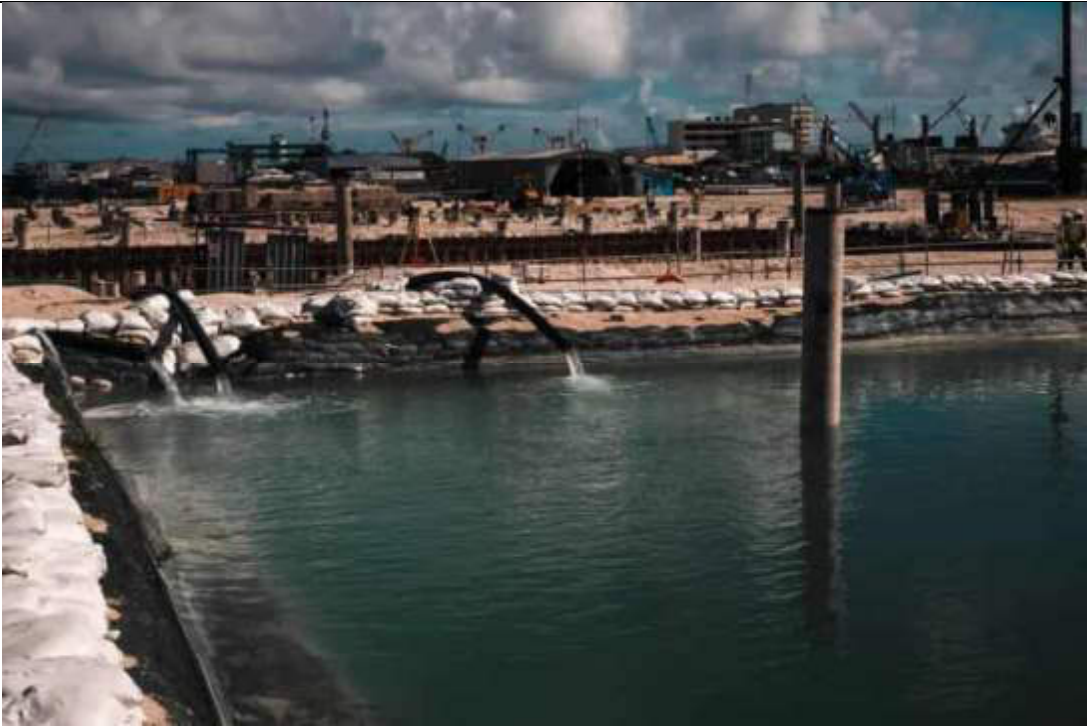
BUNKER AREA DEWATERING CONTINUE
