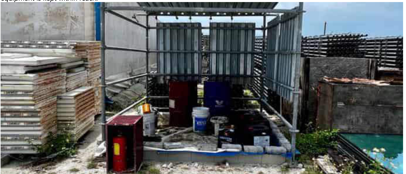
Photo 24 12/10/23 11:37hrs. Waste oil storage area.
