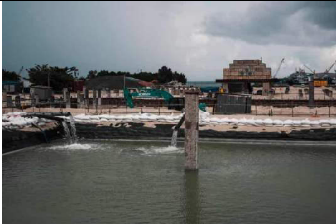
BUNKER AREA DEWATERING CONTINUE
