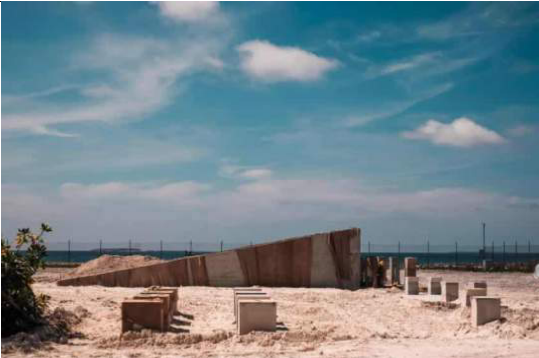
CONSTRUCTION OF TEMPORARY BATCHING PLANT
