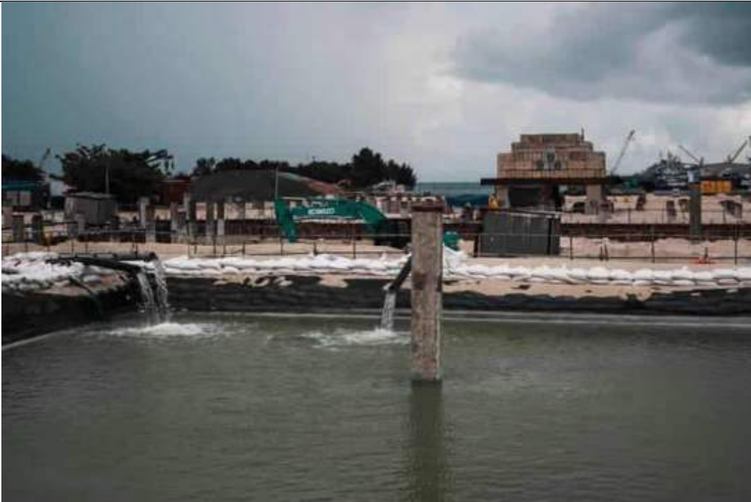
BUNKER AREA DEWATERING CONTINUE
