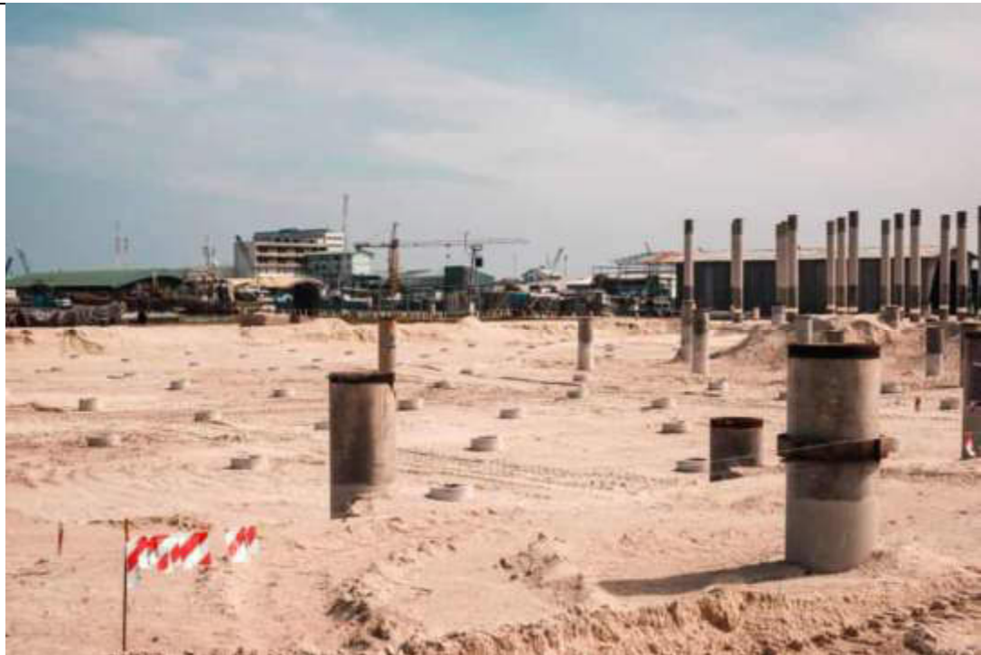
MAIN PROCESS BUILDING EXCAVATION
