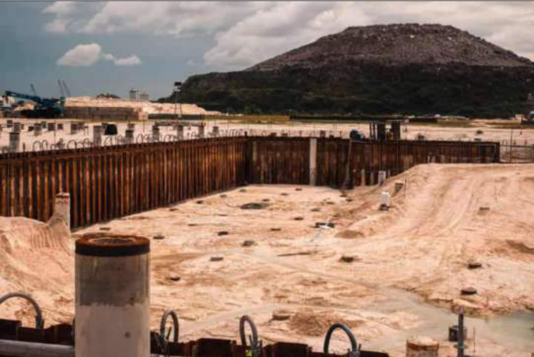
BUNKER EXCAVATION CONTINUE FROM WEST SIDE
