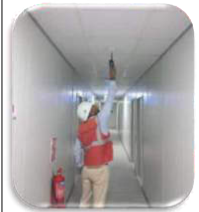
Smoke Detector Inspection
