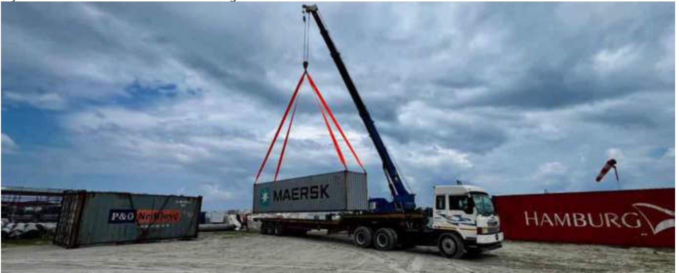
Photo 11 24/10/23 11:19hrs. Loading/Unloading work ongoing from the sea side gate area.
