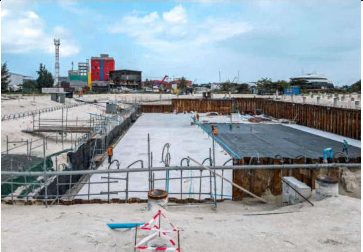
BUNKER AREA - WATERPROOFING MEMBRANE AT AREA 1 & LEACHATE AREA.
