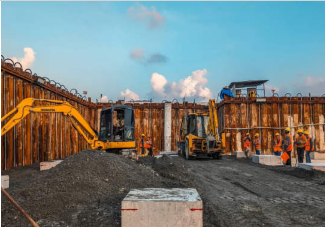
BUNKER FIRST LAYER BACKFILLING & COMPACTION.
