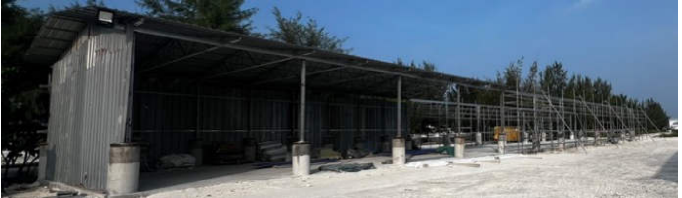
Photo 17 15/01/24 – Construction work for the batching plant support facilities ongoing.
