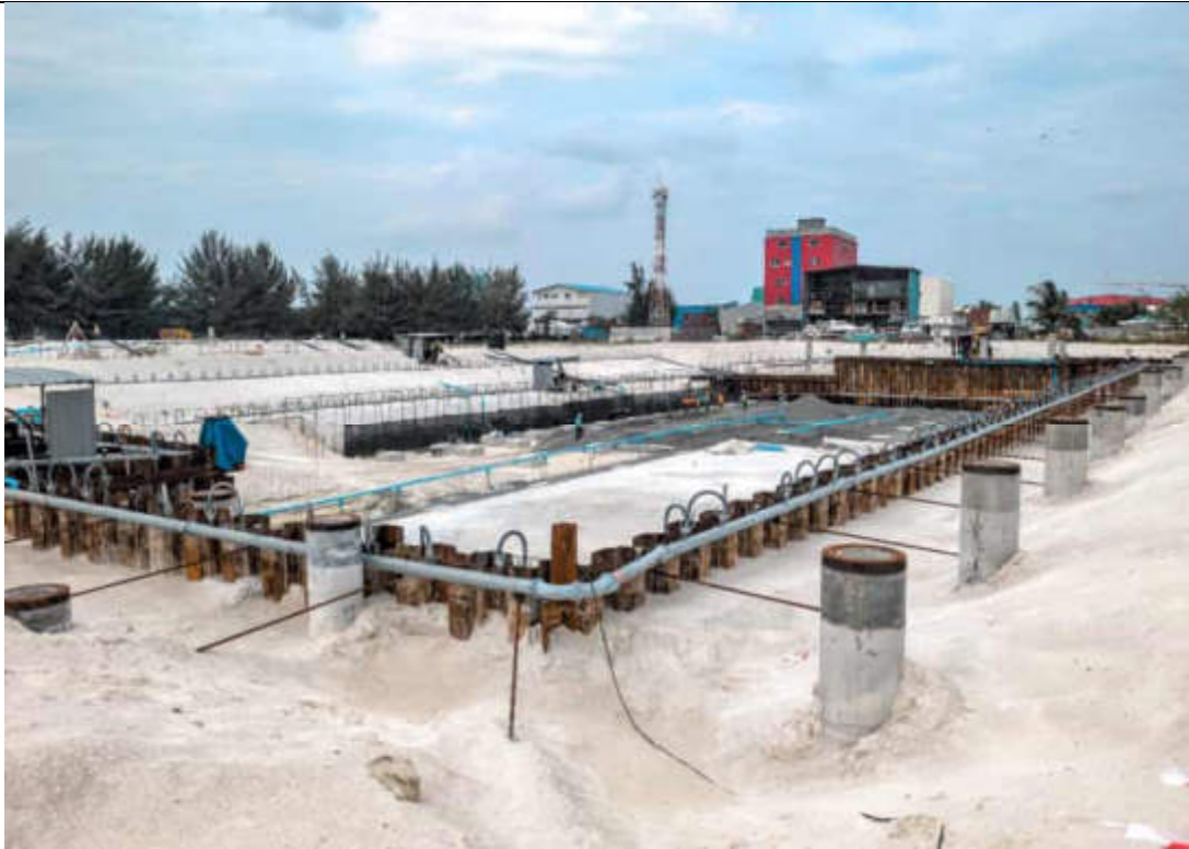
BUNKER AREA 1 COMPLETED LEAN CONCRETE
