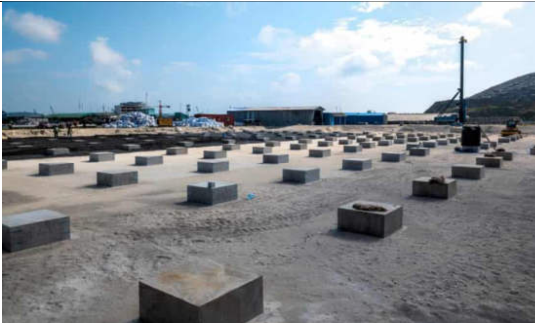
COMPLETED 17 NOS. PILECAPS AT BUNKER & 14 NOS. AT PROCESS BUILDING
