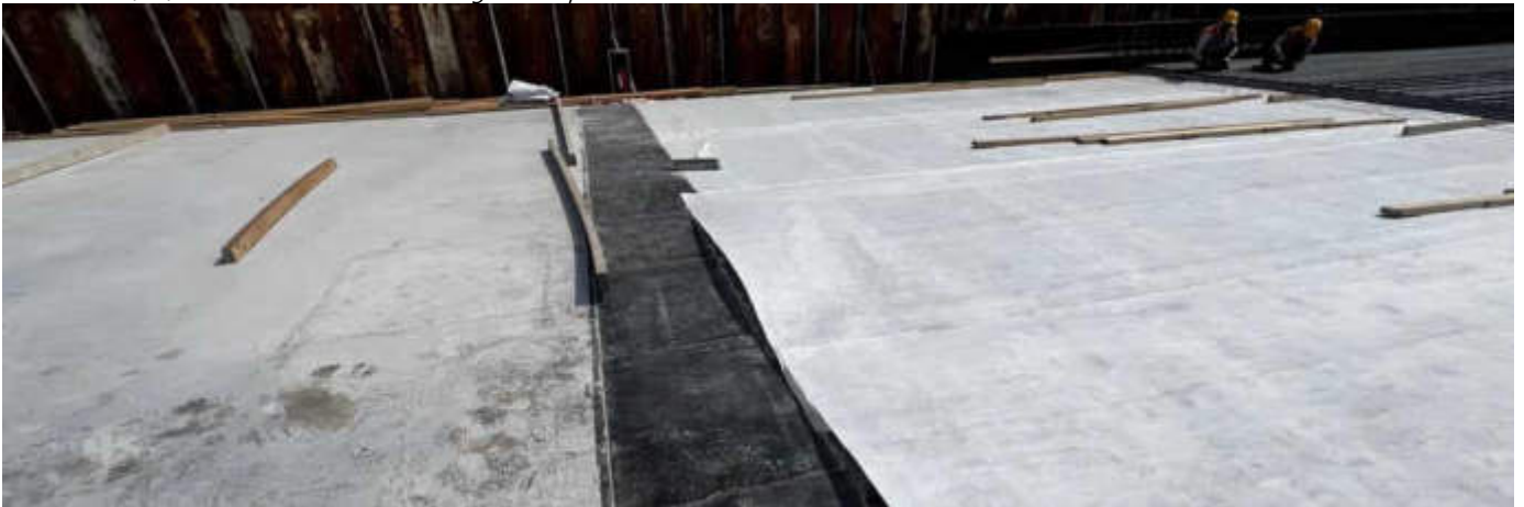
Photo 06 06/03/24 – Bunker Area 4 geomembrane installation work is in progress.
