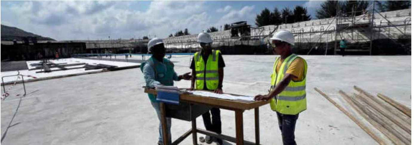
Photo 05 06/03/24 – Ramboll staff conducting HSE inspection on site.
