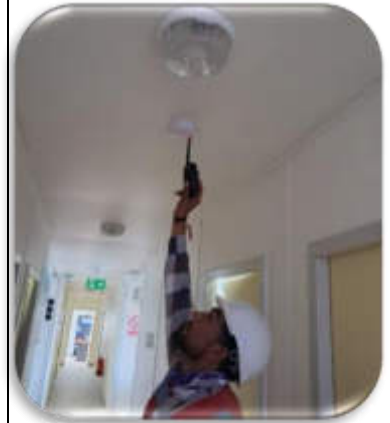
Smoke Detector Inspection
