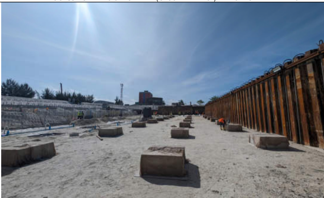
COMPLETED 24 NOS. PILECAPS AT BUNKER
