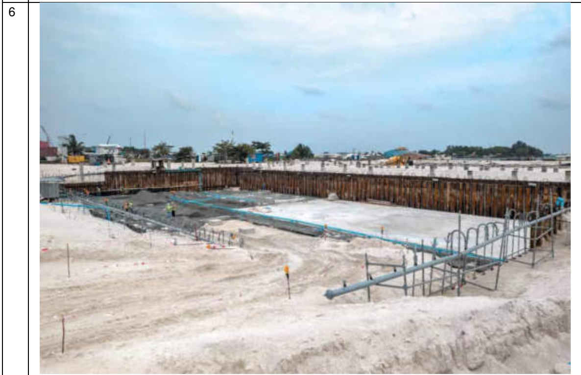
BUNKER AREA 2 & AREA 3 FIRST LAYER BACKFILLING.
