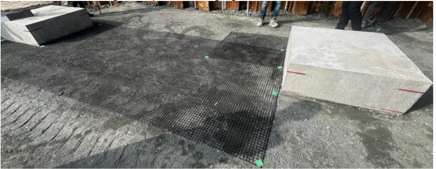
Photo 11 15/01/24 – Geomesh layer placed after first layer of soil is compacted.
