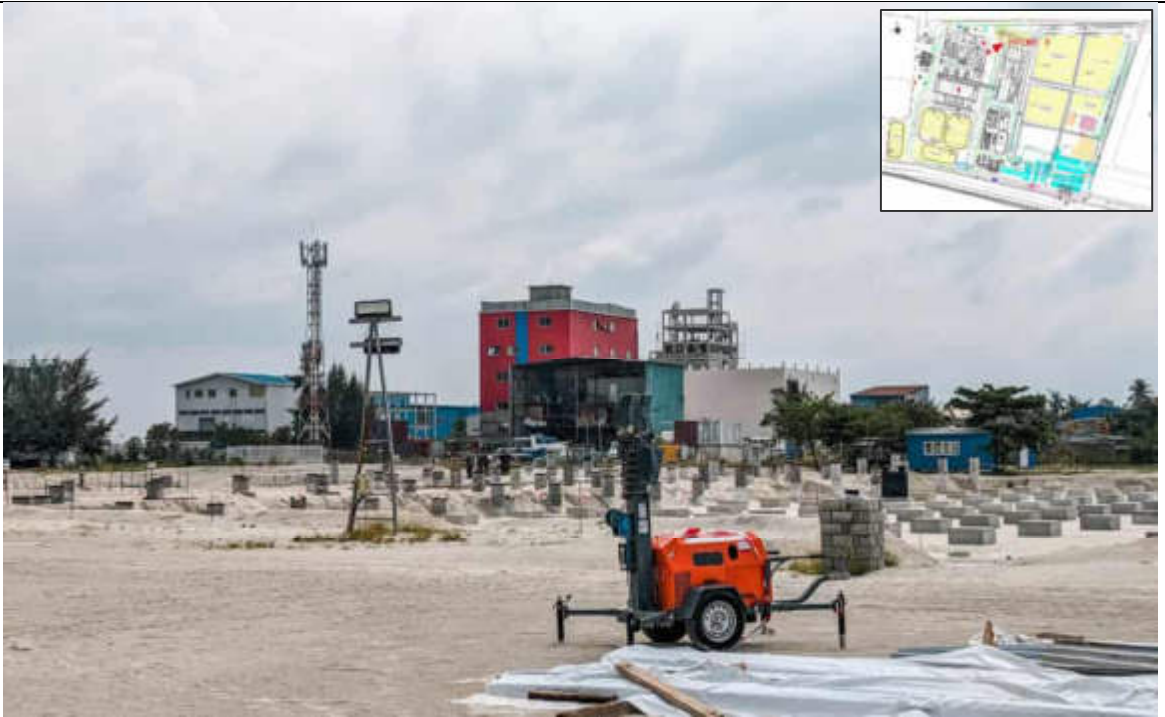
OVERALL - POINT THREE
