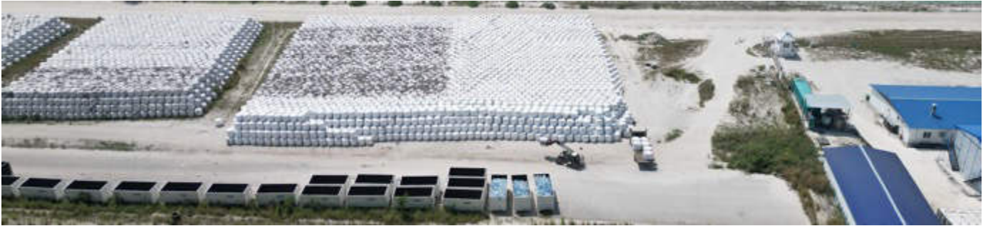
Photo 56 25/01/24 – WAMCO waste bales kept close to the site boundary, risk of fire is there.
