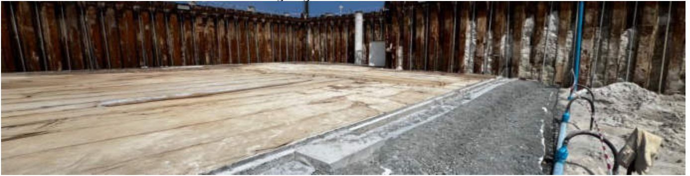
Photo 45 30/01/24 – Lean concrete work is on going in the bunker area.
