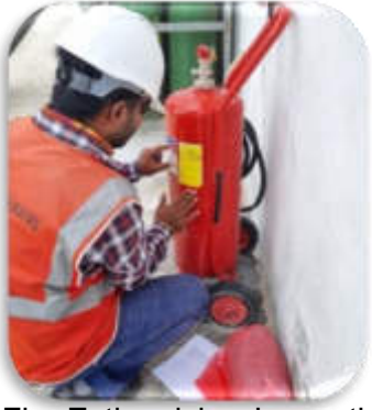
Fire Extinguisher Inspection
