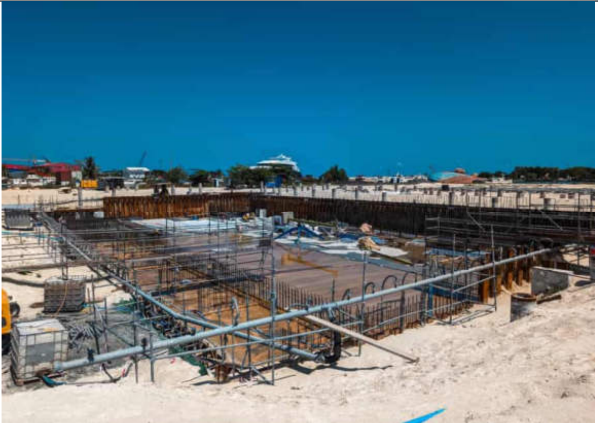
FORMWORK & REINFORCEMENT BAR IN PROGRESS AT AREA 2
