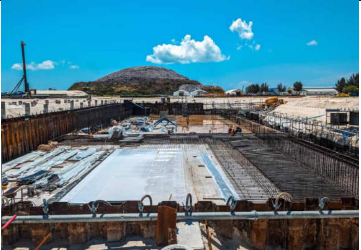
BUNKER AREA - AREA 4 FOUNDATION SLAB COMPLETED.
