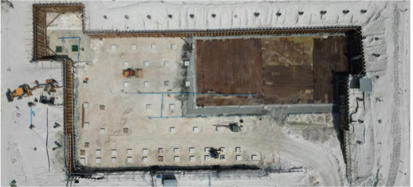
Photo 53 25/01/24 – Lean concrete works completed in part of the bunker
