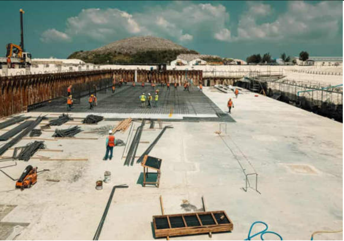
BUNKER AREA - REINFORCEMENT BAR & FORMWORK AT AREA 1 IN PROGRESS.
