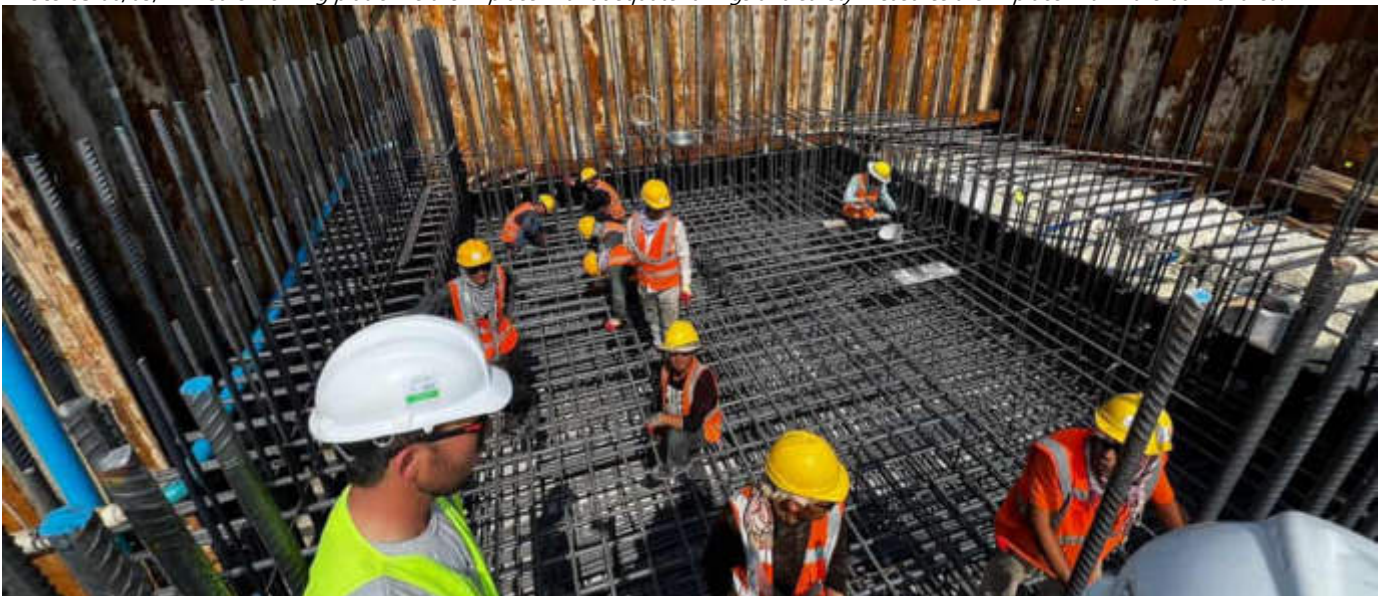
Photo 04 06/03/24 – Leachate pit area (Area 1) reinforcement installation work is in progress.
