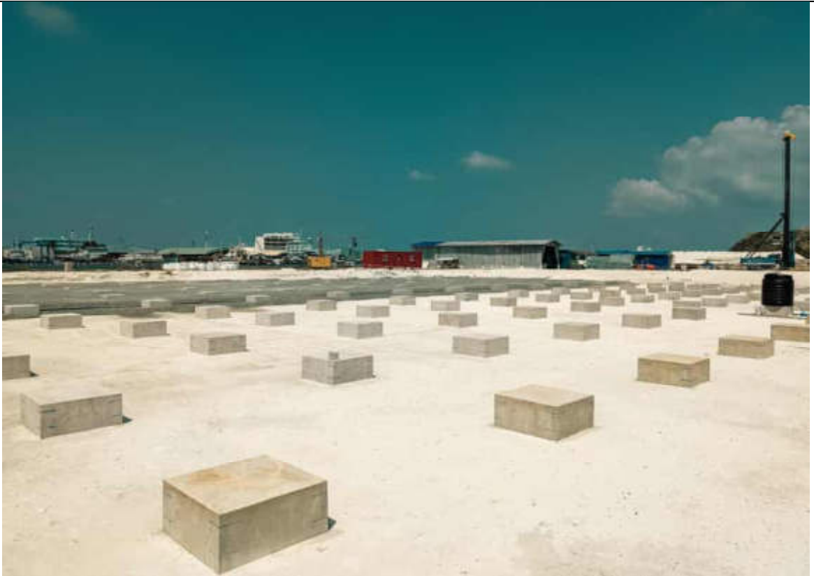
BACKFILLING SECOND LAYER AT PROCESS AREA M1-M10 COMPLETED.
