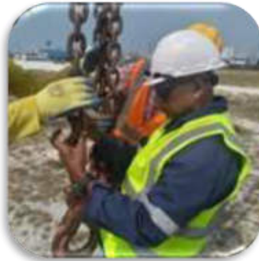
Lifting slings Inspection
