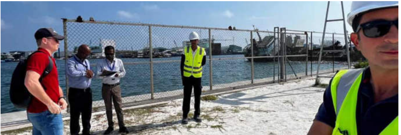
Photo 01 06/03/24 – Site visit conducted by PMU – Project Director – Mr. Murthaza and Project Manager – Mr. Zameel
