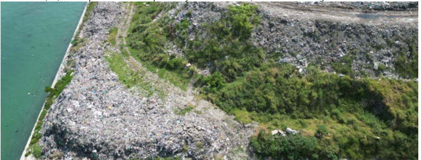
Photo 55 25/01/24 – WAMCO landfill very close to quaywall and risk of spill over into the lagoon is there.
