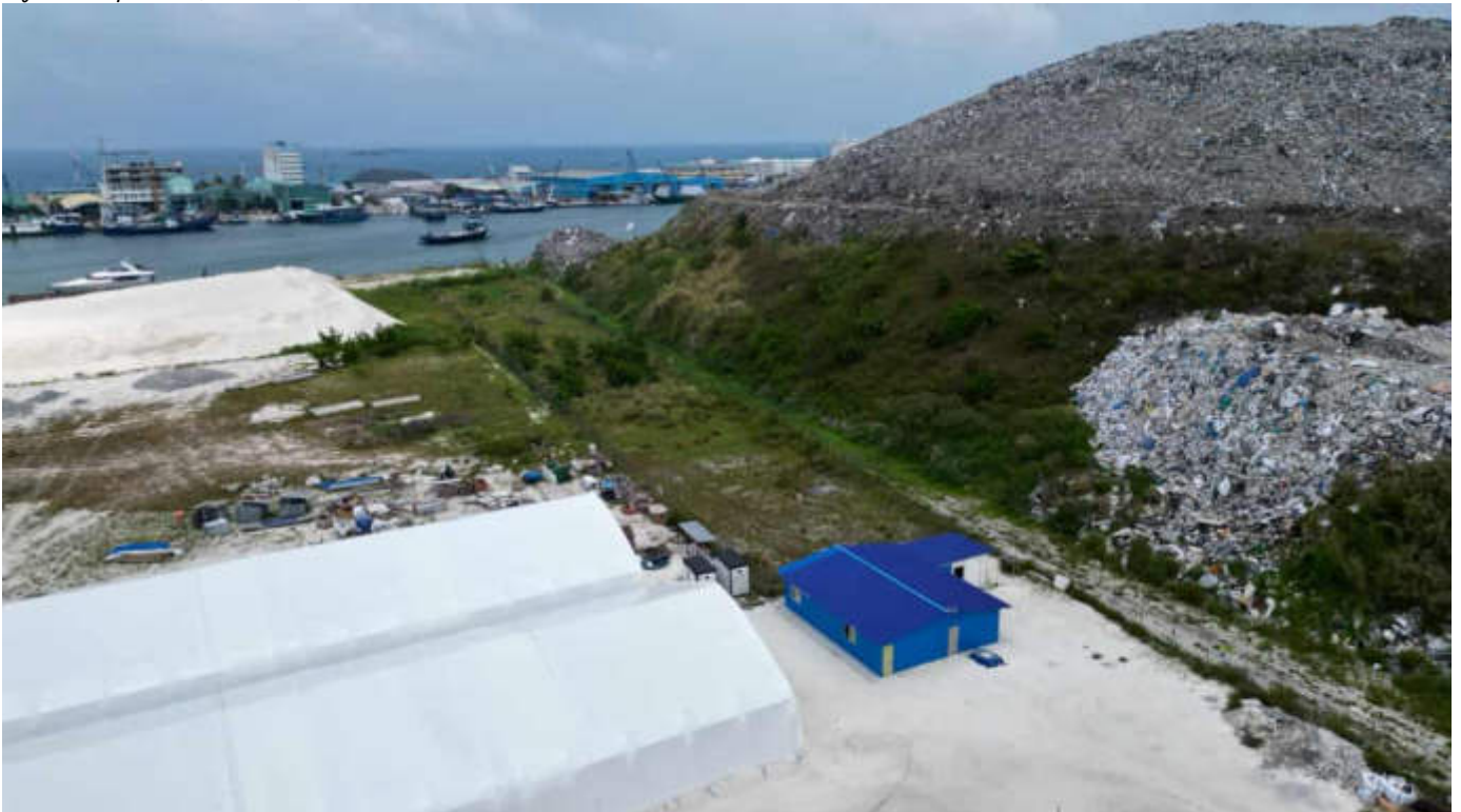
Photo 18 27/02/24 – WAMCO landfill (right side) adjacent to the site, with 20m buffer zone for safety incase of falling objects.
