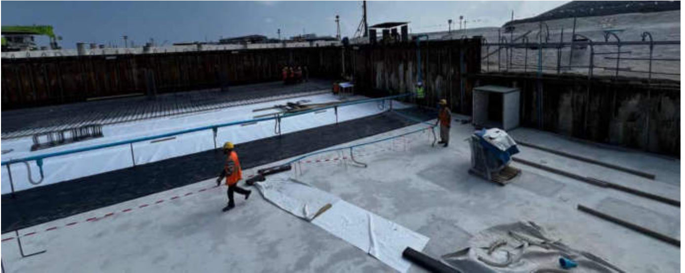
Photo 02 06/03/24 – Bunker Area 1 reinforcement installation work for the bunker bottom slab continues
