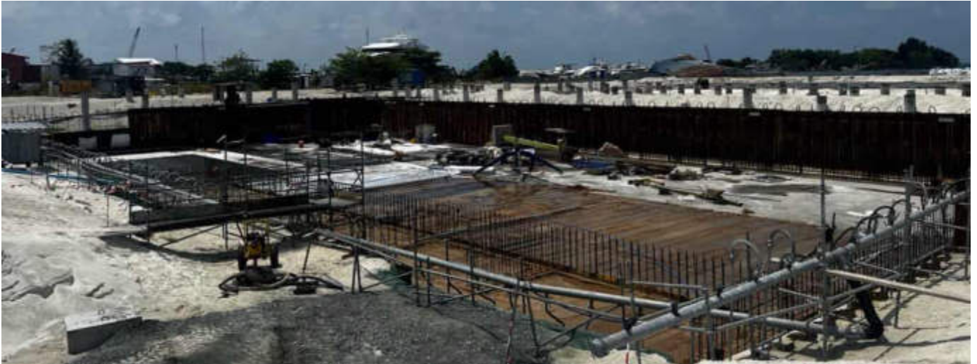
Photo 17 27/03/24 – Overall bunker construction area. Reinforcement installation works continues.
