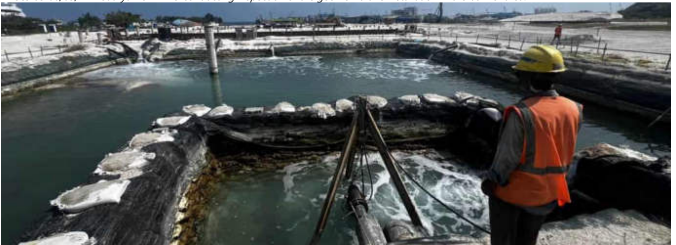
Photo 10 06/03/24 – Dewatering works continues and the sedimentation pit is clean and water quality tests are carried out at the outfall monthly.
