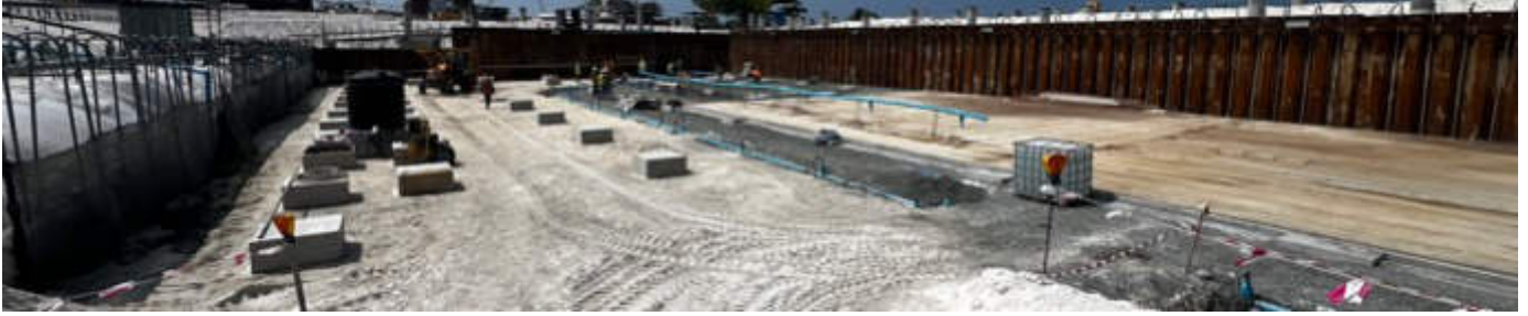
Photo 44 30/01/24 – Lean concrete work is on going in the bunker area.
