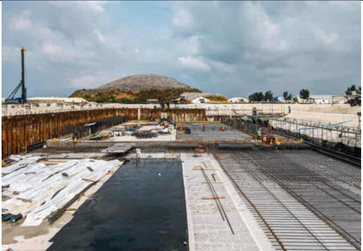
BUNKER AREA - AREA 1 FOUNDATION SLAB COMPLETED.
