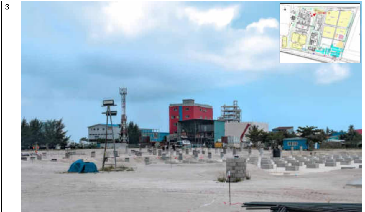
OVERALL - POINT THREE
