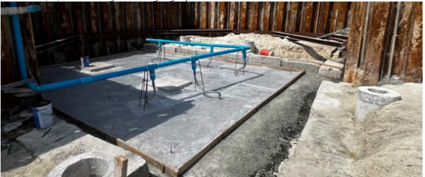
Photo 46 30/01/24 – Leachate pit area, lean concrete and backfilling works in progress.
