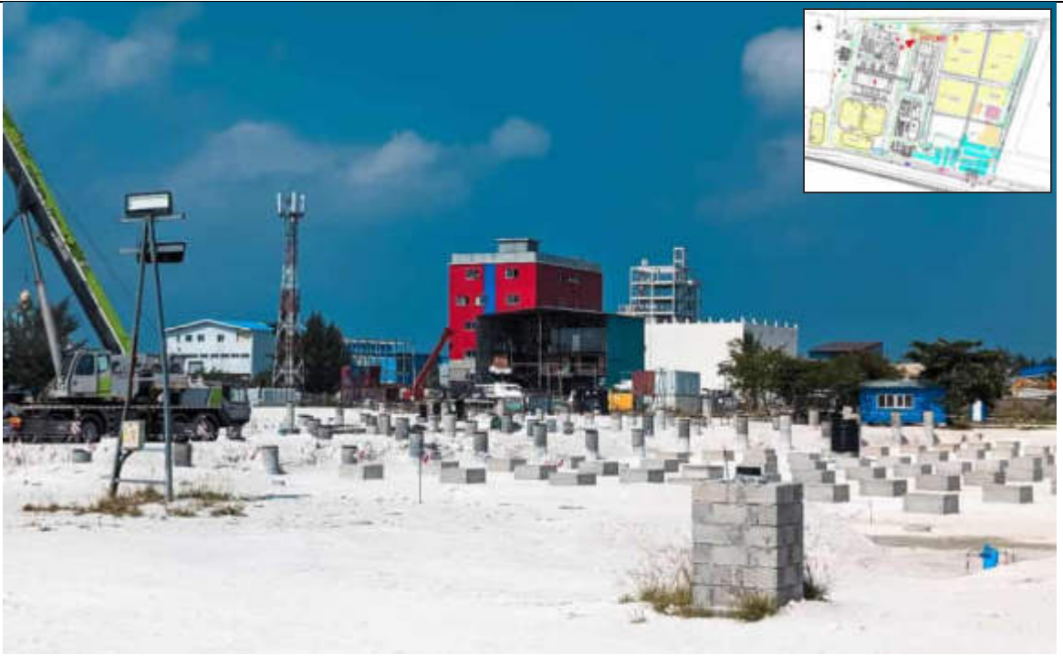
OVERALL - POINT THREE
