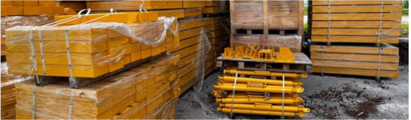
Photo 06 03/01/24 – Scaffolding materials delivered to site.
