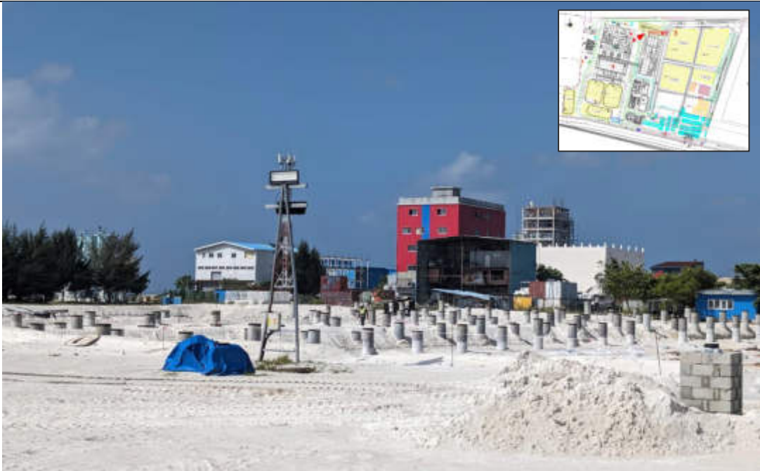
OVERALL - POINT THREE
