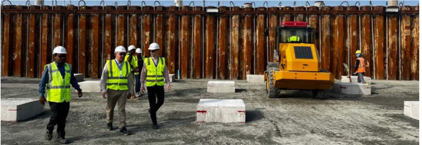
Photo 13 15/01/24 – Members of the ER with Mr. Latheef inside the bunker area.
