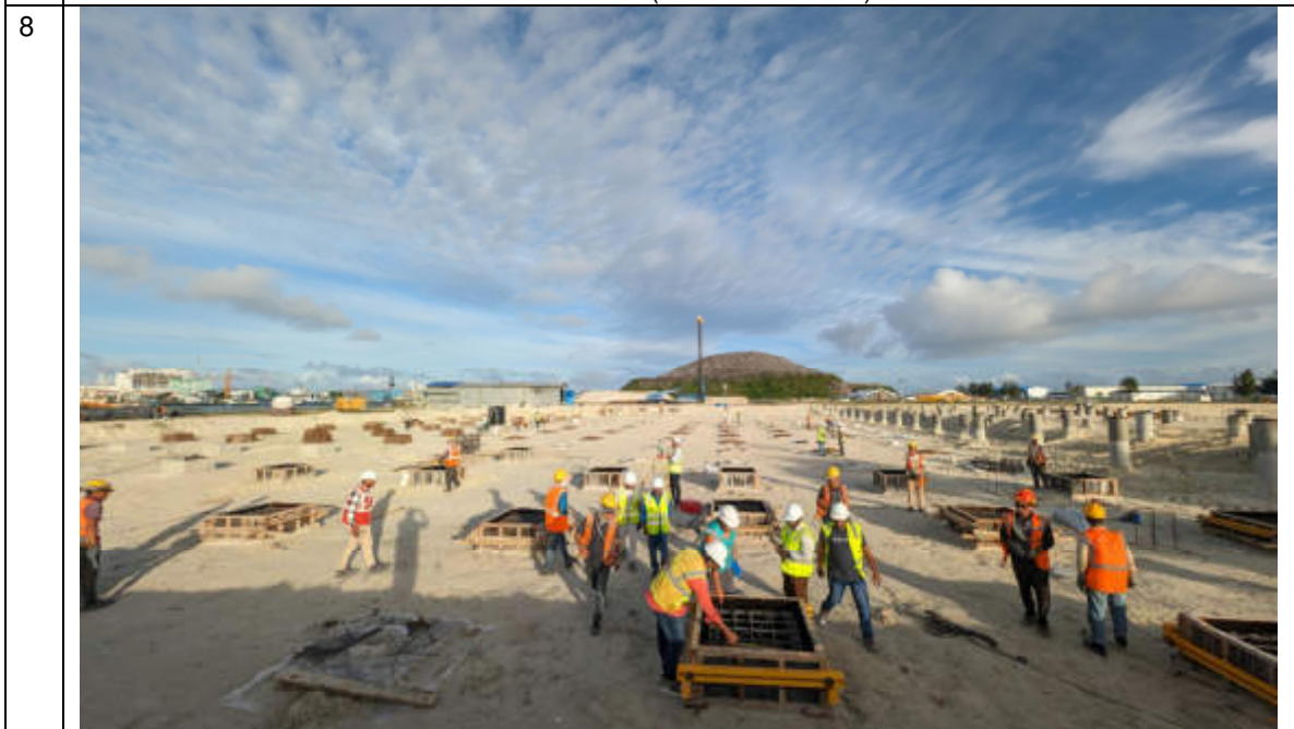
COMPLETED 18 NOS. PILECAPS AT BUNKER & 46 NOS. AT PROCESS BUILDING
