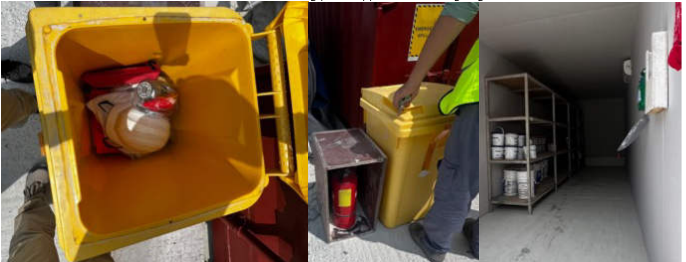
Photo 18 15/01/24 – Spill control kit kept near the chemical storage container.
