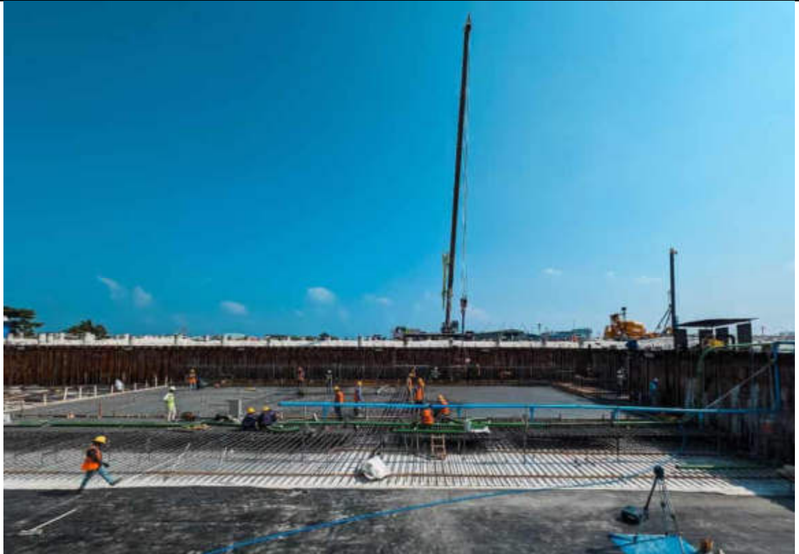
BUNKER AREA - CONCRETING WORK AT AREA 1 IN PROGRESS.
