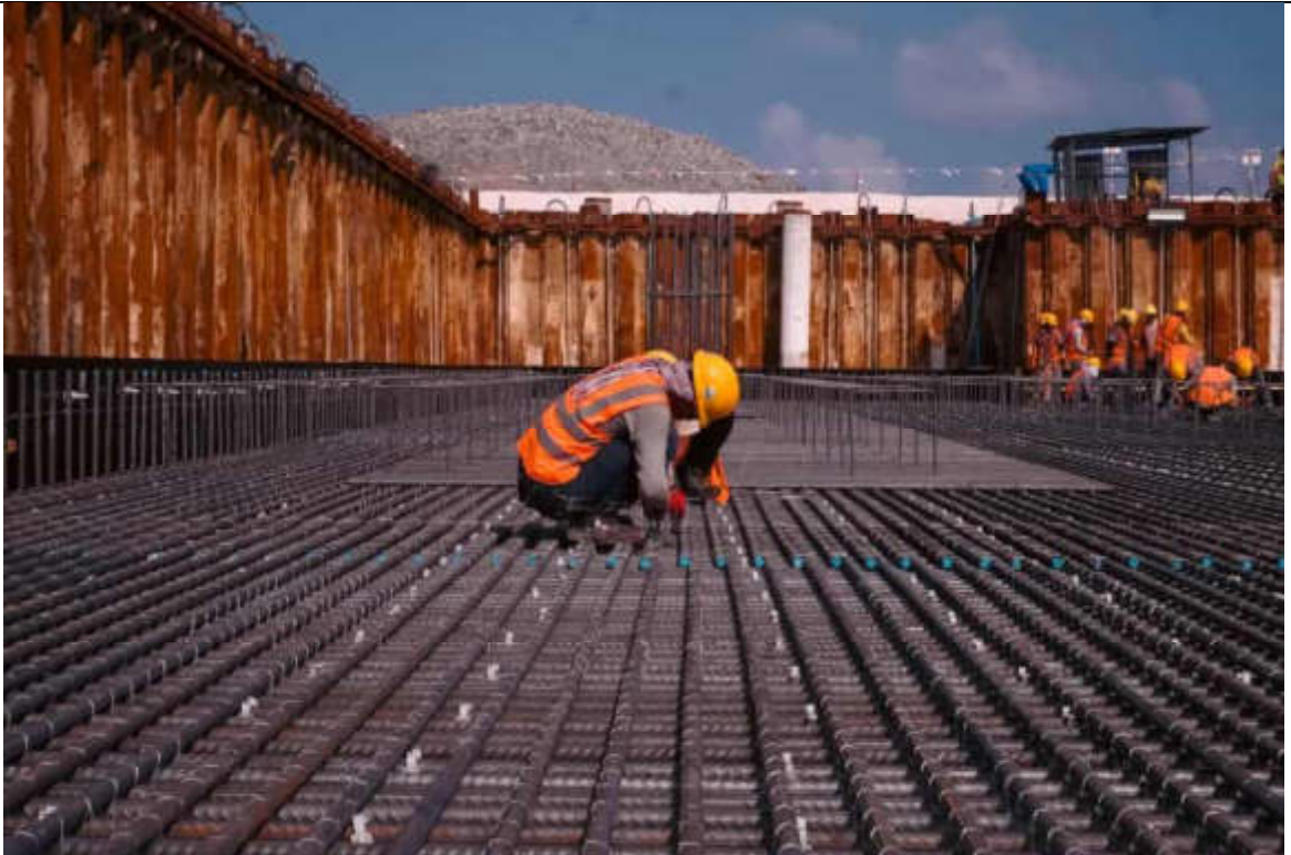
REINFORCEMENT BAR & FORM WORK AT AREA 1 INSTALLATION.
