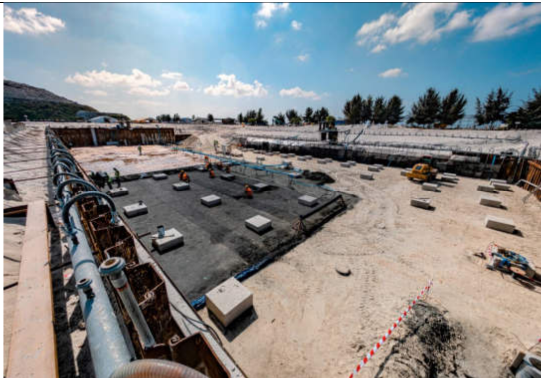
BUNKER AREA 2 FIRST LAYER BACKFILLING.
