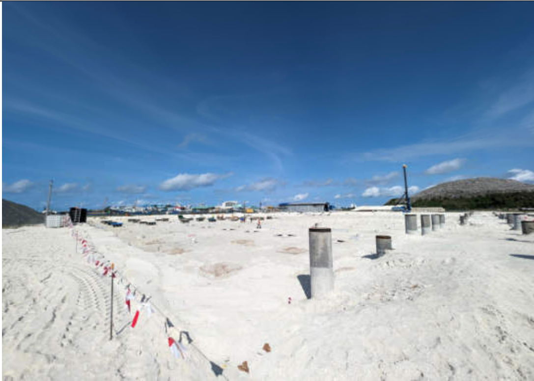
MAIN PROCESS BUILDING & TURBINE (SECOND PHASE) PILECAPS PREPARATION.
