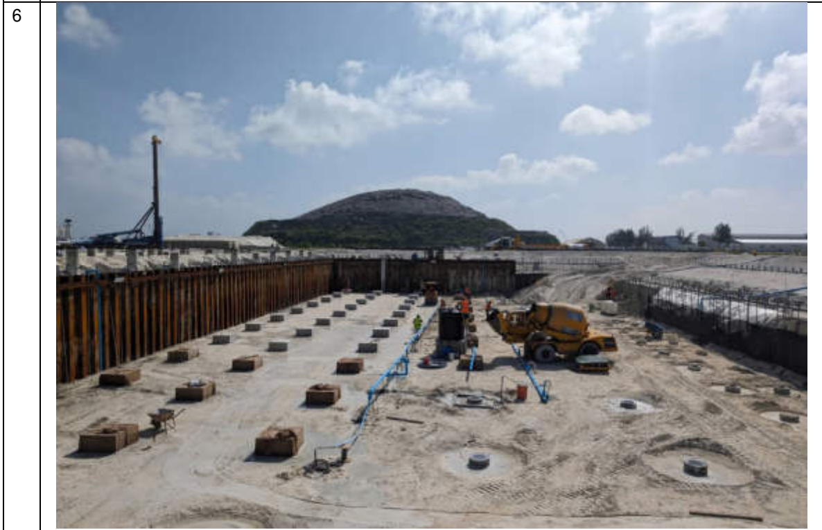
BUNKER PILECAPS CONCRETING WORK.
