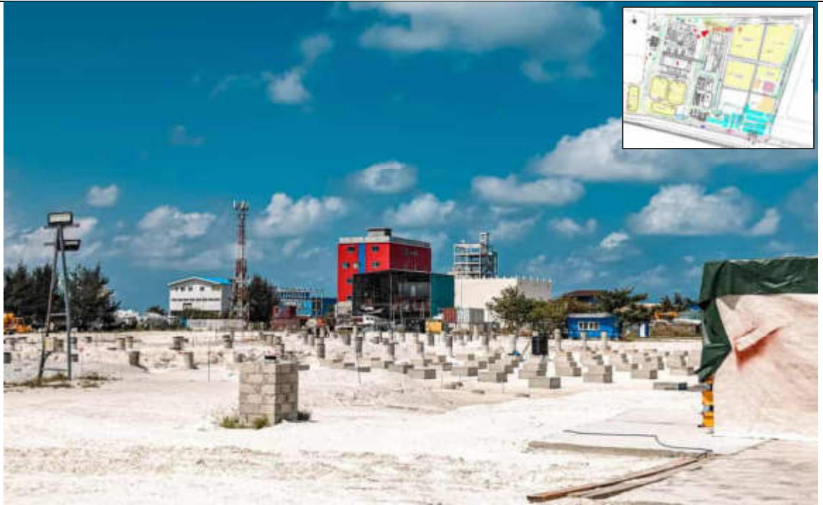
OVERALL - POINT THREE
