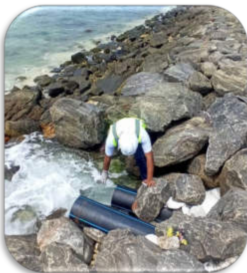
Dewatering Effluent Sampling
