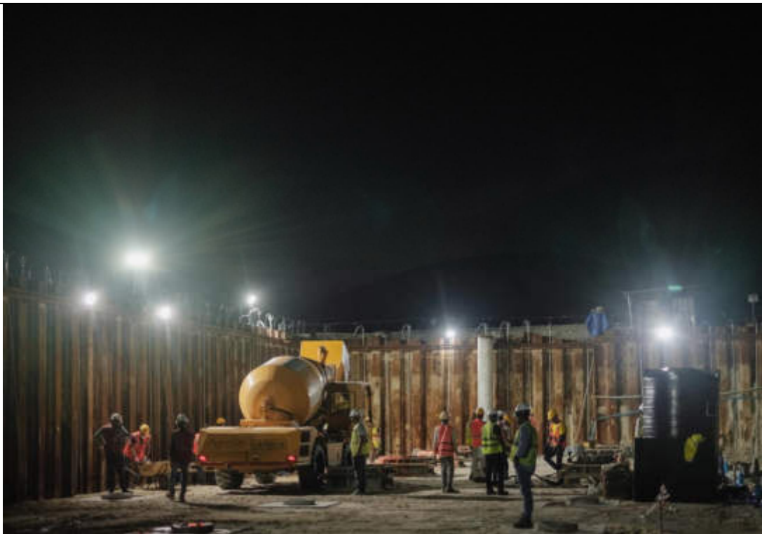
BUNKER PILECAPS CONCRETING WORK.
