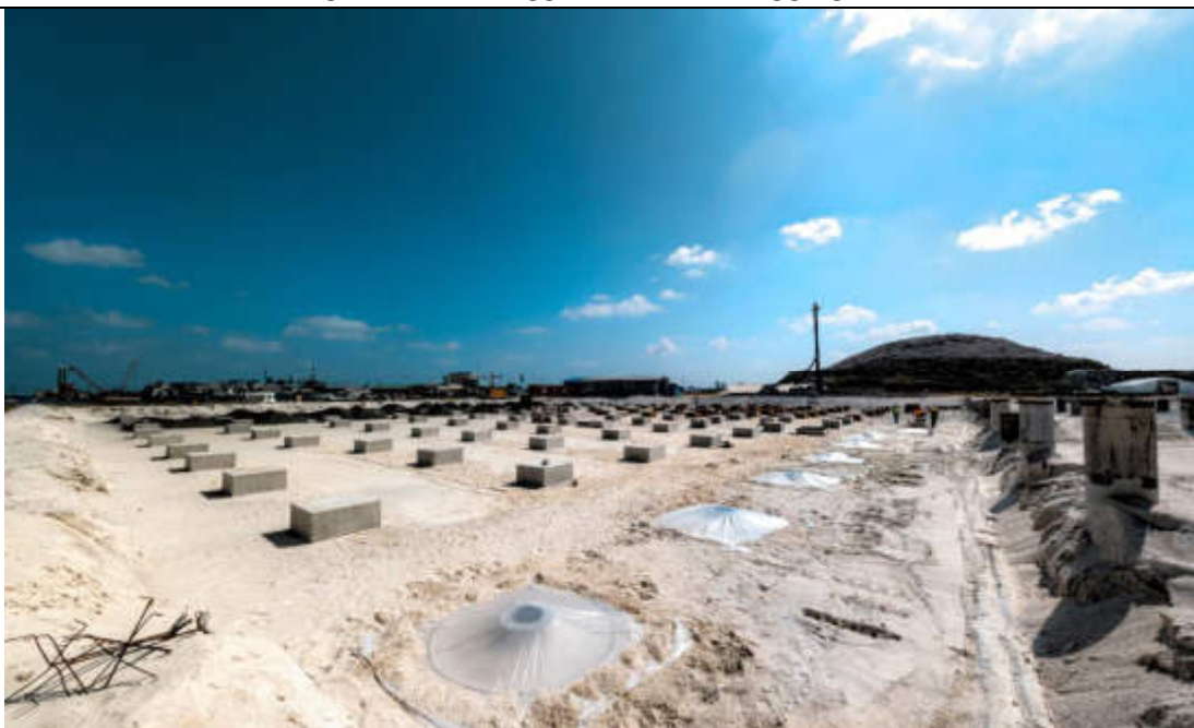
COMPLETED 8 NOS. PILECAPS AT BUNKER & 46 NOS. AT PROCESS BUILDING
