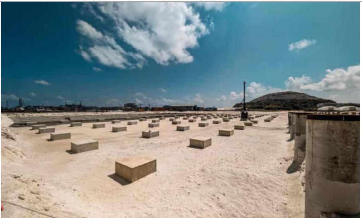
BACKFILLING SECOND LAYER PROCESS AREA AT M1-M10
