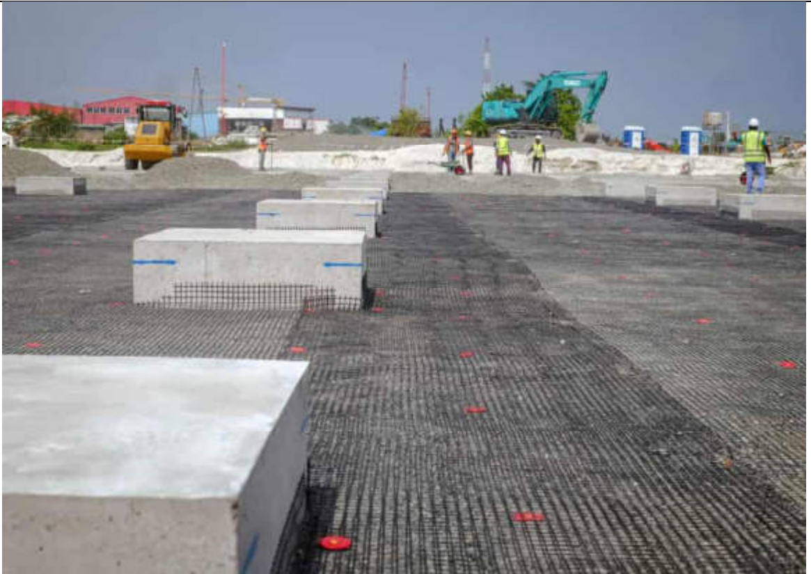
GEOGRID INSTALLATION AT PROCESS AREA M1-M10.
