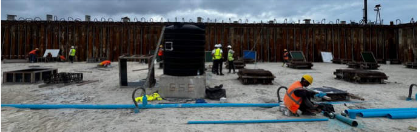
Photo 02 03/01/24 – Bunker area pile concrete works in progress.
