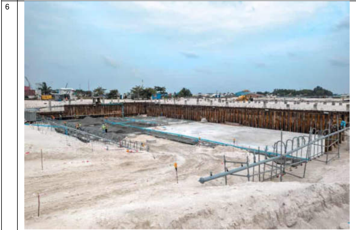
BUNKER AREA 3 SECOND LAYER BACKFILLING.
