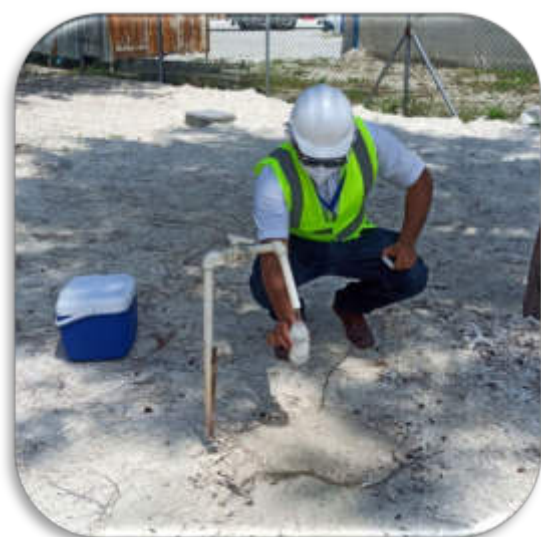
Supply Water for Camp And Construction Sampling
