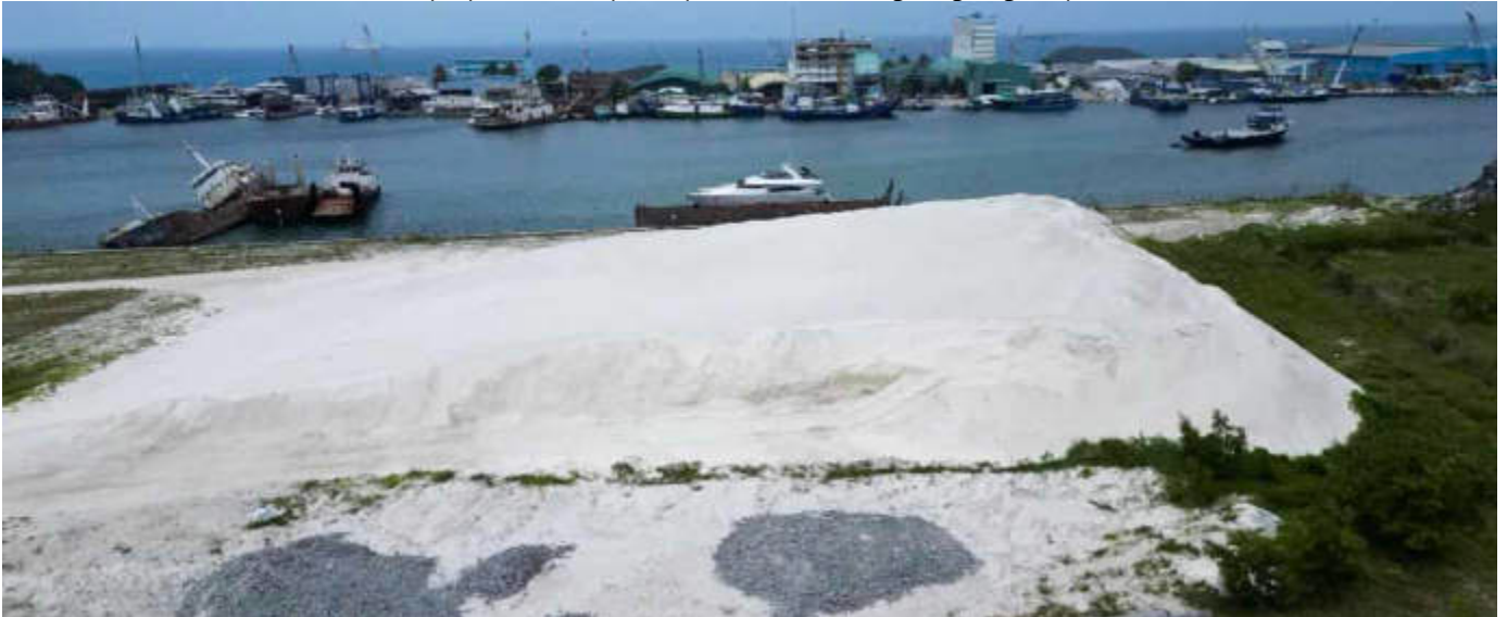
Photo 07 27/02/24 – Excavated Sand stockpile on site.
