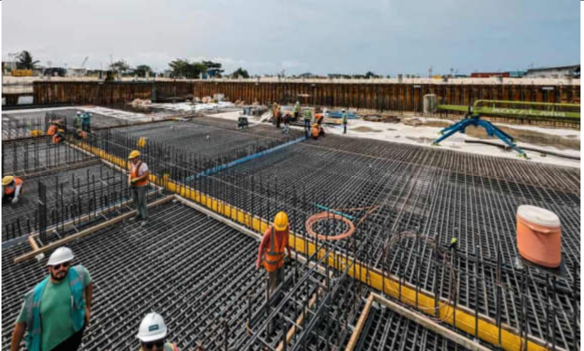
REINFORCEMENT BAR & FORMWORK WORKMANSHIP HAS BEEN IMPROVED.
