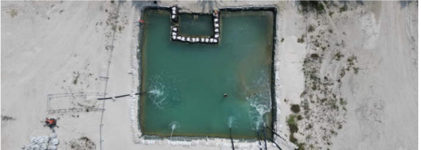
Photo 49 17/01/24 – Dewatering sedimentation pit, continuous dewatering is ongoing until foundation is complete.
