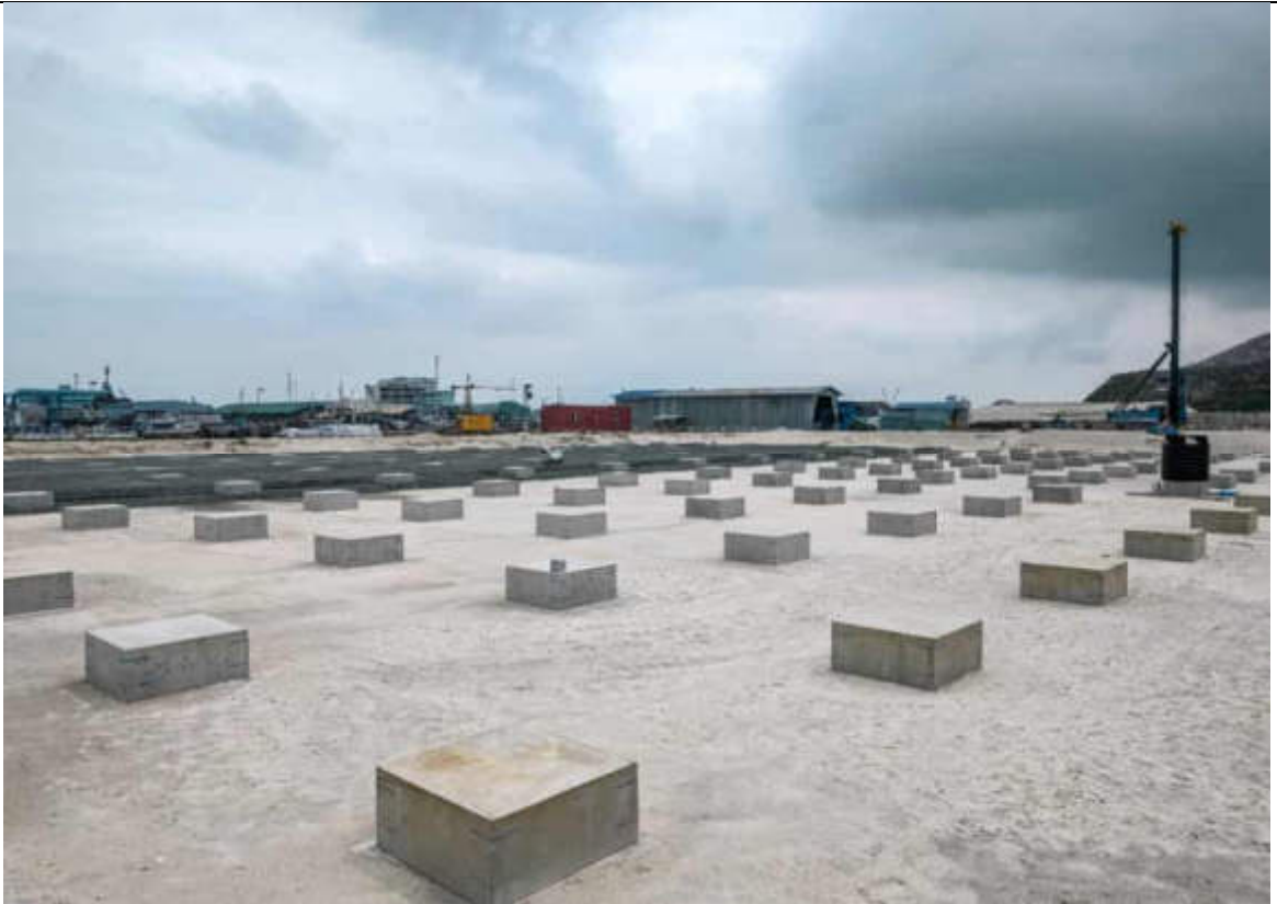
BACKFILLING SECOND LAYER AT PROCESS AREA M1-M10.
