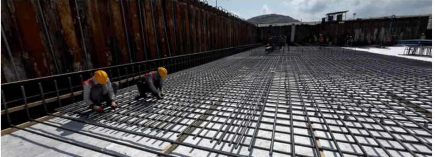
Photo 07 06/03/24 – Reinforcement installation work in the Bunker Area 1 and Area 3 continues.
