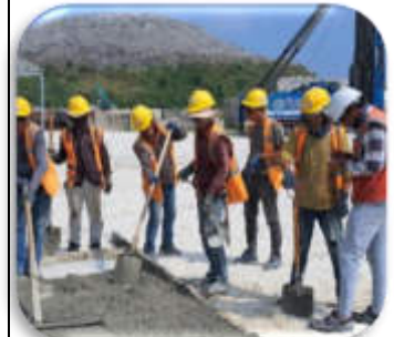
Hand tools Inspection
