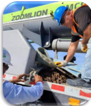
Lifting slings Inspection
