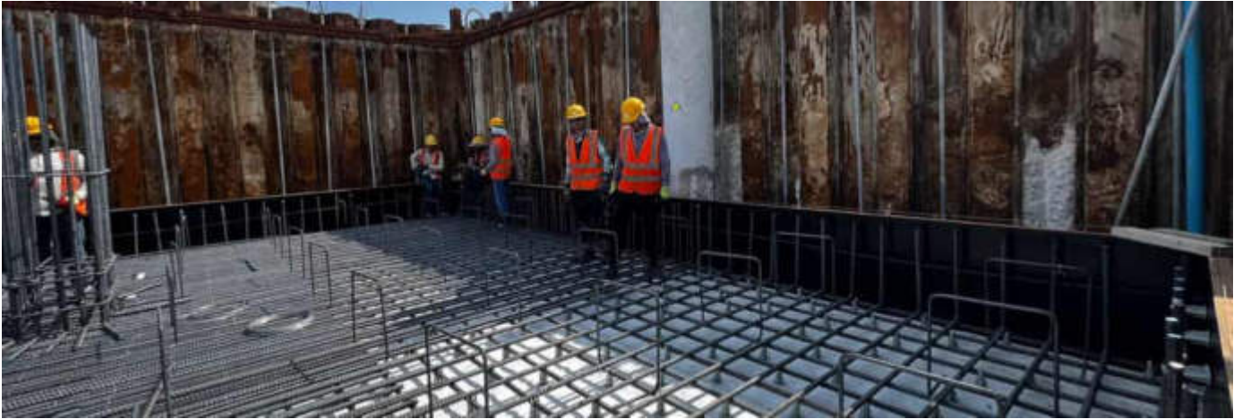
Photo 08 06/03/24 – Reinforcement installation work in the bunker leachate pit (Area 1) continues.
