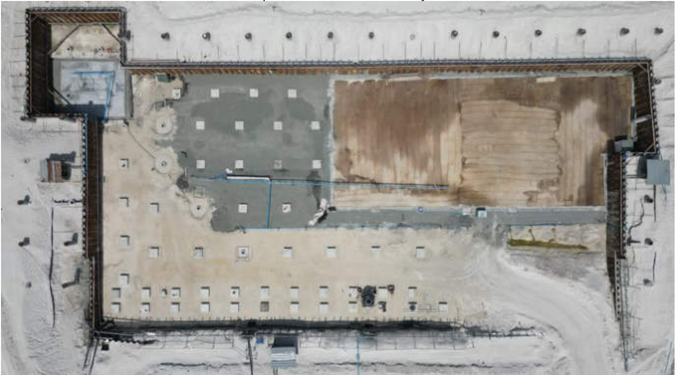
Photo 56 30/01/24 – Backfilling and lean concrete works continue in the bunker area.
