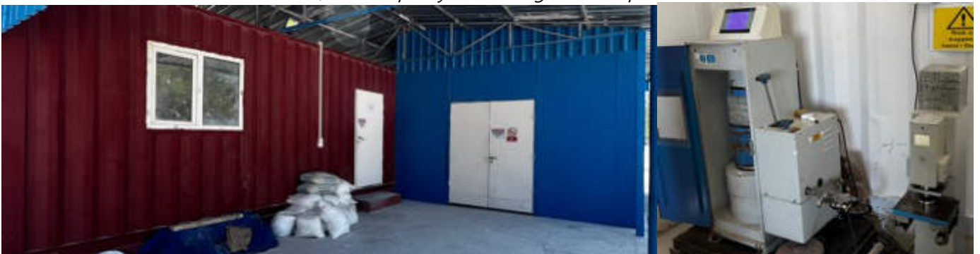
Photo 40 15/01/24 – Concrete testing lab is operational on site.
