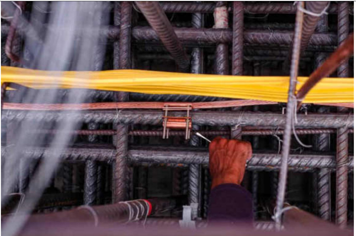
EARTHING CABLE AND WATERSTOP INSTALLATION AT LEACHATE AREA.
