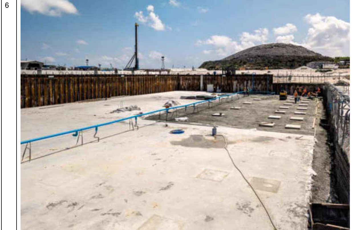
BUNKER AREA 4 LEAN SECOND LAYER BACKFILLING.
