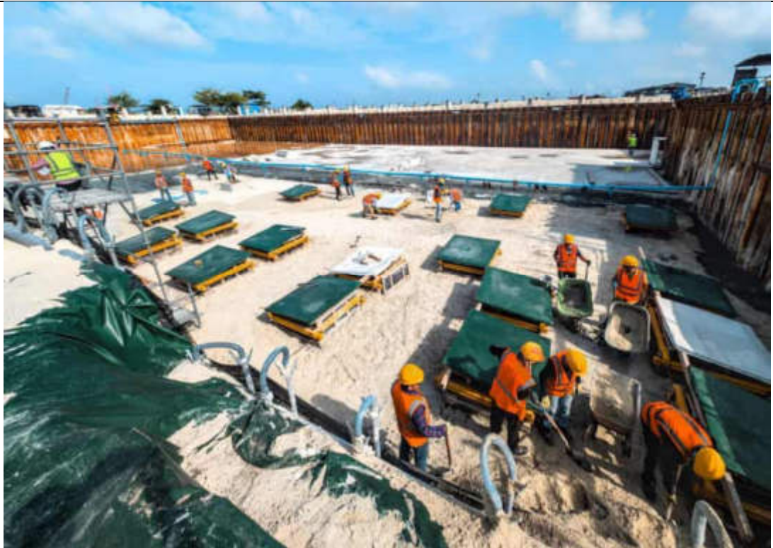
BUNKER AREA 4 COMPLETED PILECAPS.
