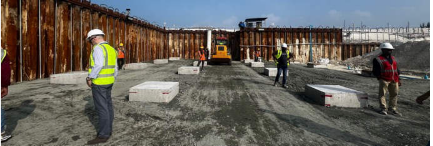
Photo 10 15/01/24 – Backfilling and compaction work on going in the bunker.
