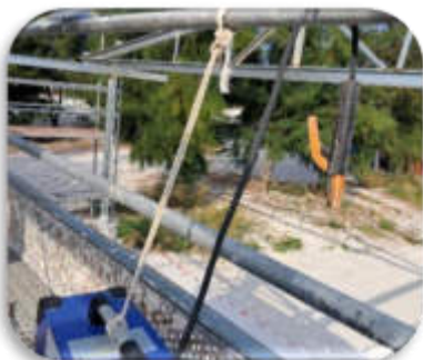
Provided tool lanyard on the Welding Machine to prevent falling objects
