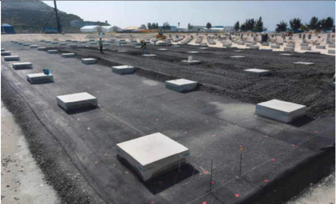
GEOGRID INSTALLATION AT PROCESS AREA.
