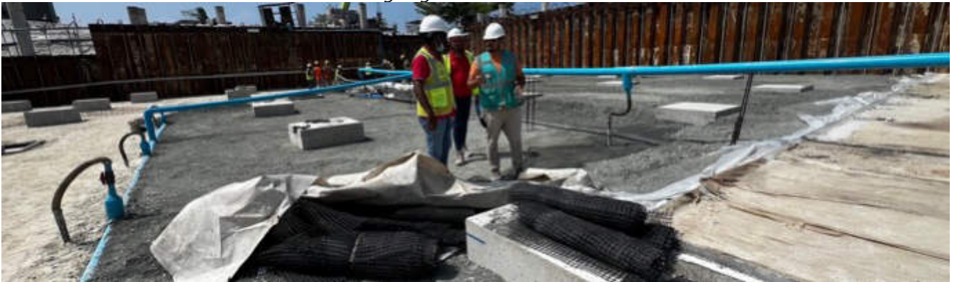
Photo 46 30/01/24 – Backfilling work is ongoing in part of the bunker area.
