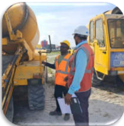
Plant and Equipment Inspection
