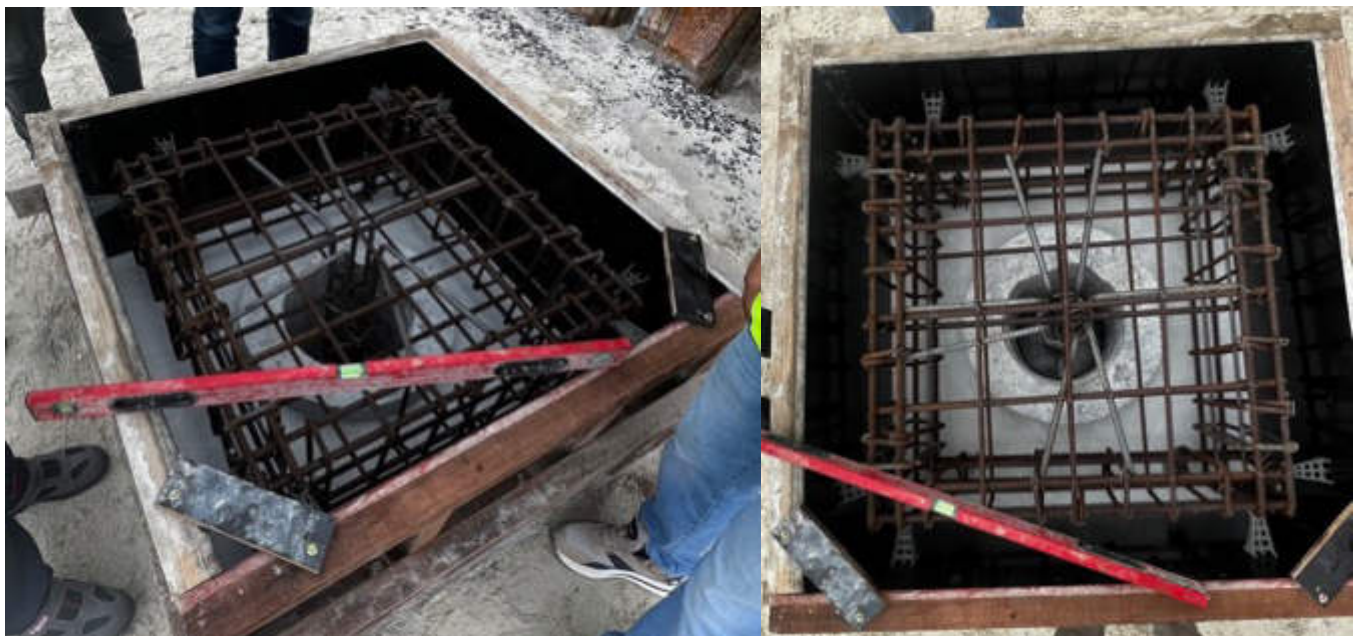
Photo 01 03/01/24 – Pile cap concrete works on going, pile cap reinforcement placed.
