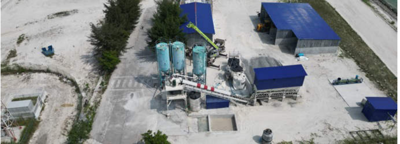
Photo 50 17/01/24 – Concrete batching plant area, batching plant is operational.
