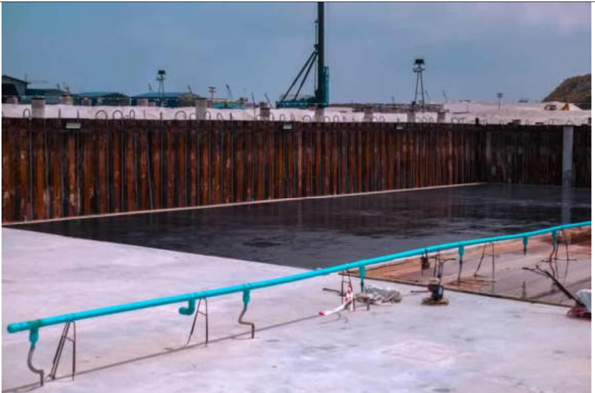
PRIMER APPLICATION BEFORE WATERPROOFING MEMBRANE
