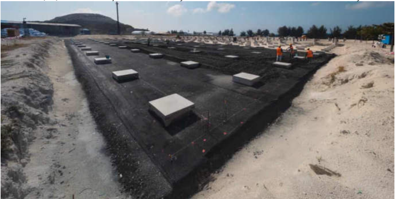
Photo 03 13/02/24 - Bunker area backfilling and geotextile installation in progress
