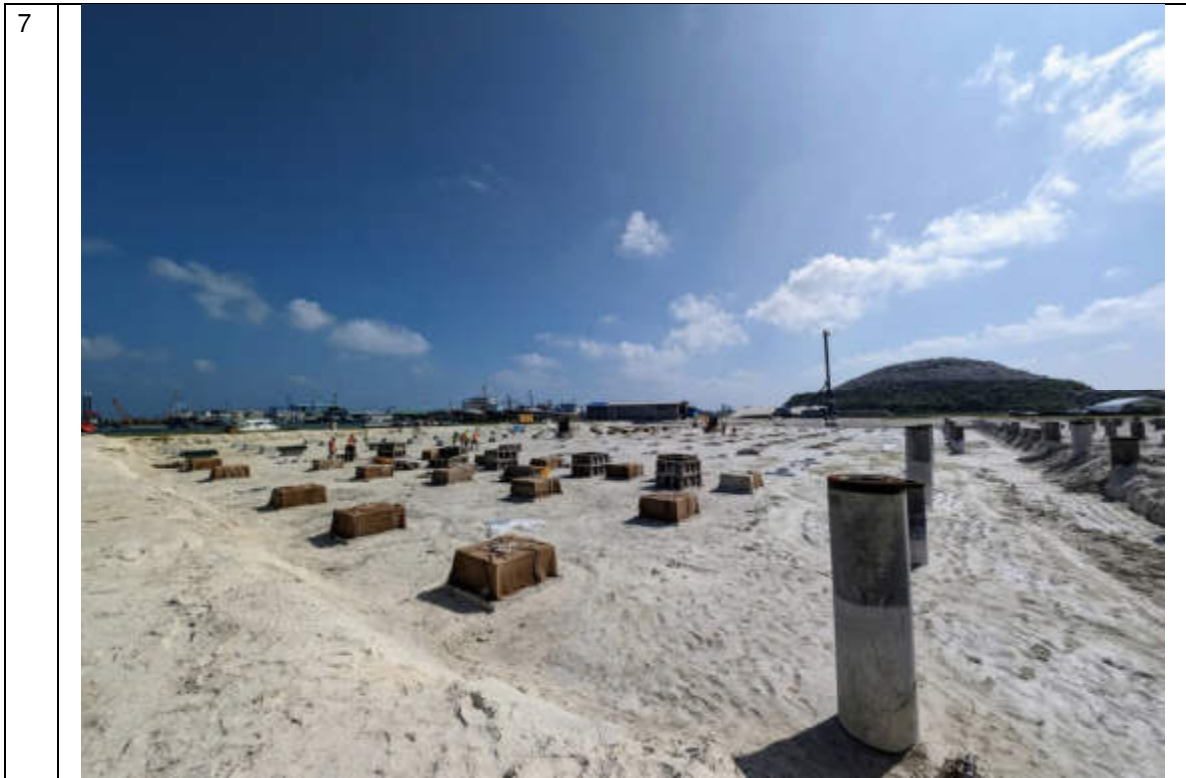
MAIN PROCESS BUILDING & TURBINE (SECOND PHASE) PILECAPS PREPARATION.
