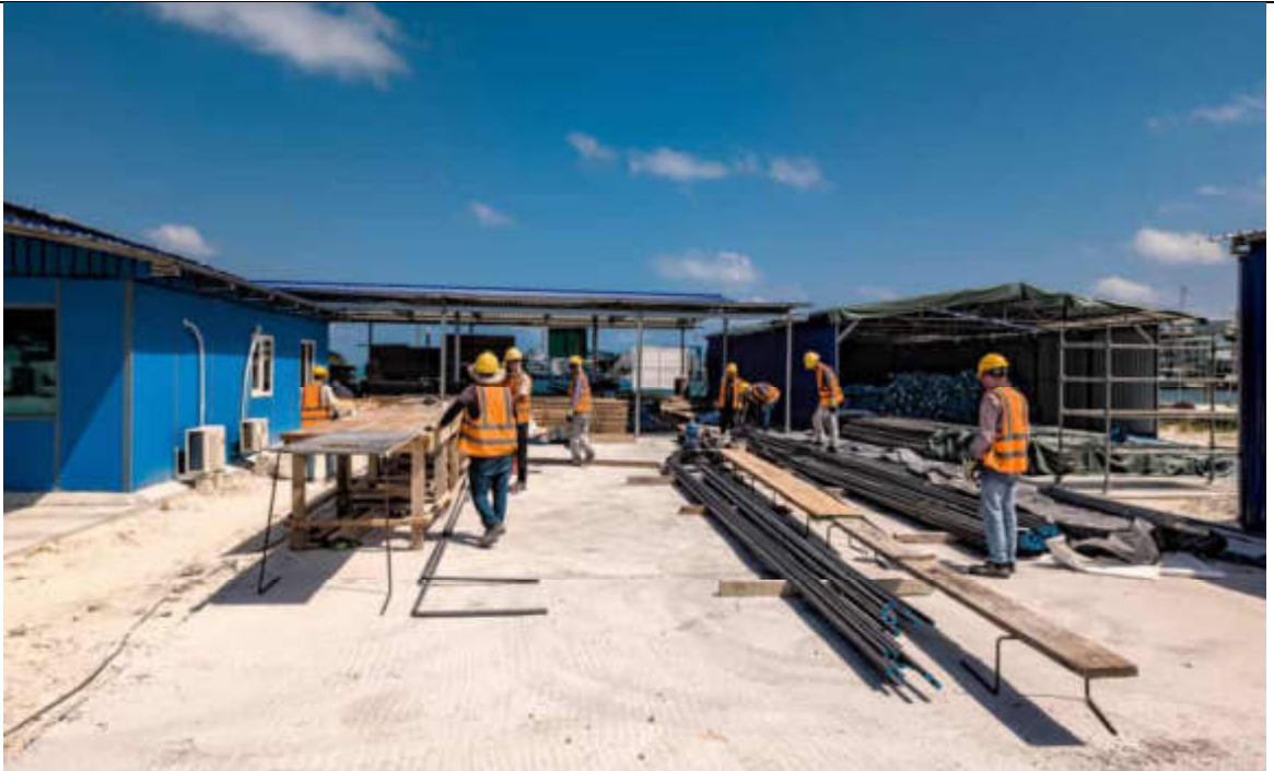
REINFORCEMENT BAR FABRICATION FOR BUNKER SLAB IN PROGRESS.
