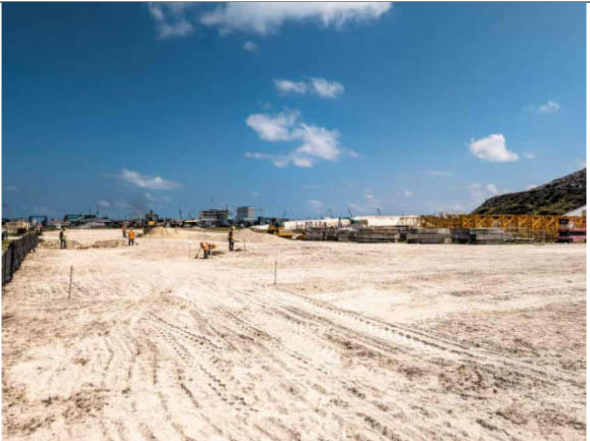
PREPARATION OF LAYDOWN AREA IN PROGRESS.
