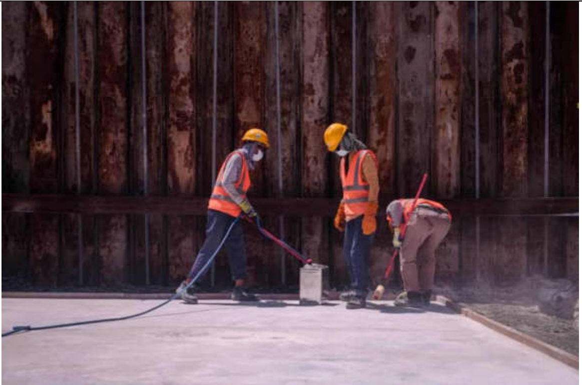
SURFACE CLEANING PRIOR TO WATERPROOFING MEMBRANE INSTALLATION.
