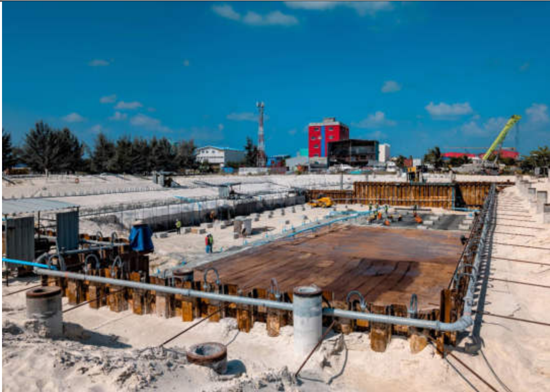
BUNKER AREA 1 COMPLETED LEAN CONCRETE
