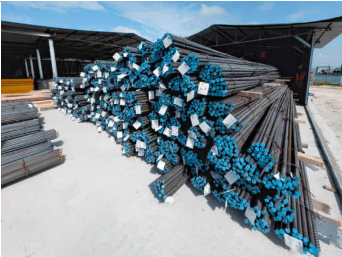
REINFORCEMENT BAR ARRIVED ON SITE
