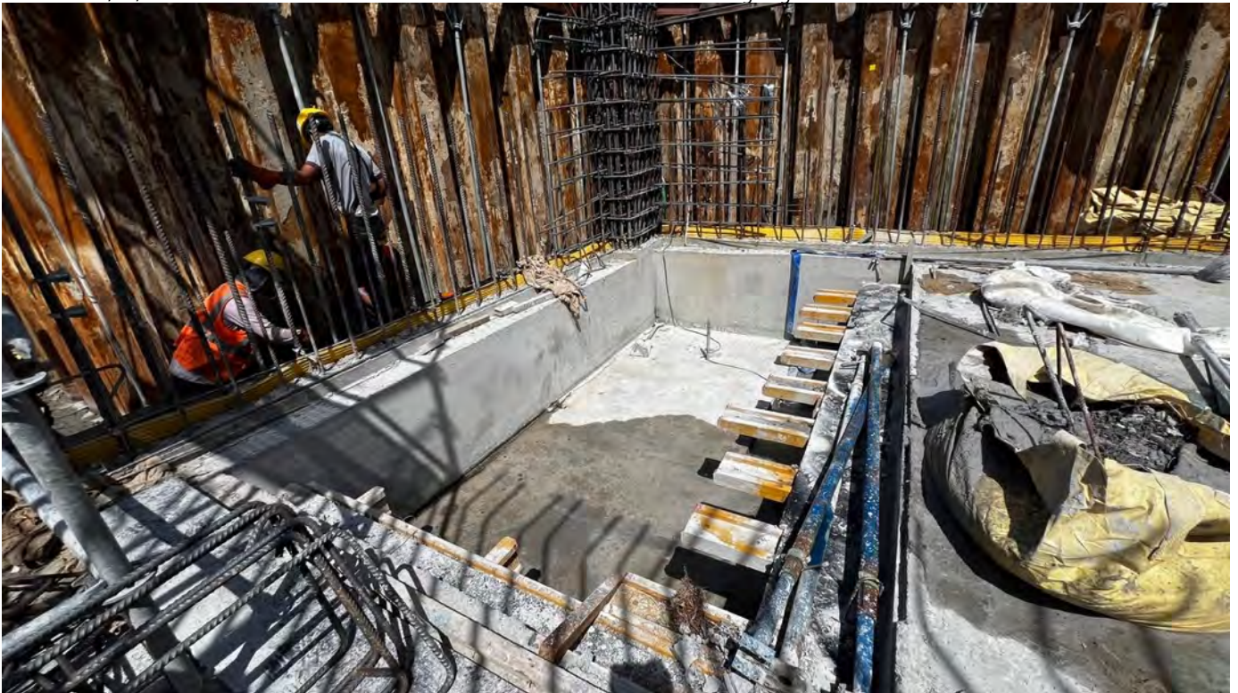
Photo 11 02/05/24 – Leachate pit area work, waterbar installation work is ongoing.
