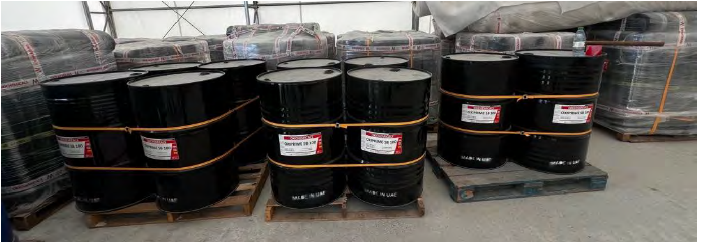
Photo 10 07/05/24 - Construction chemicals in the storage area, requires adequate measures to ensure safety, and spillage containment.
