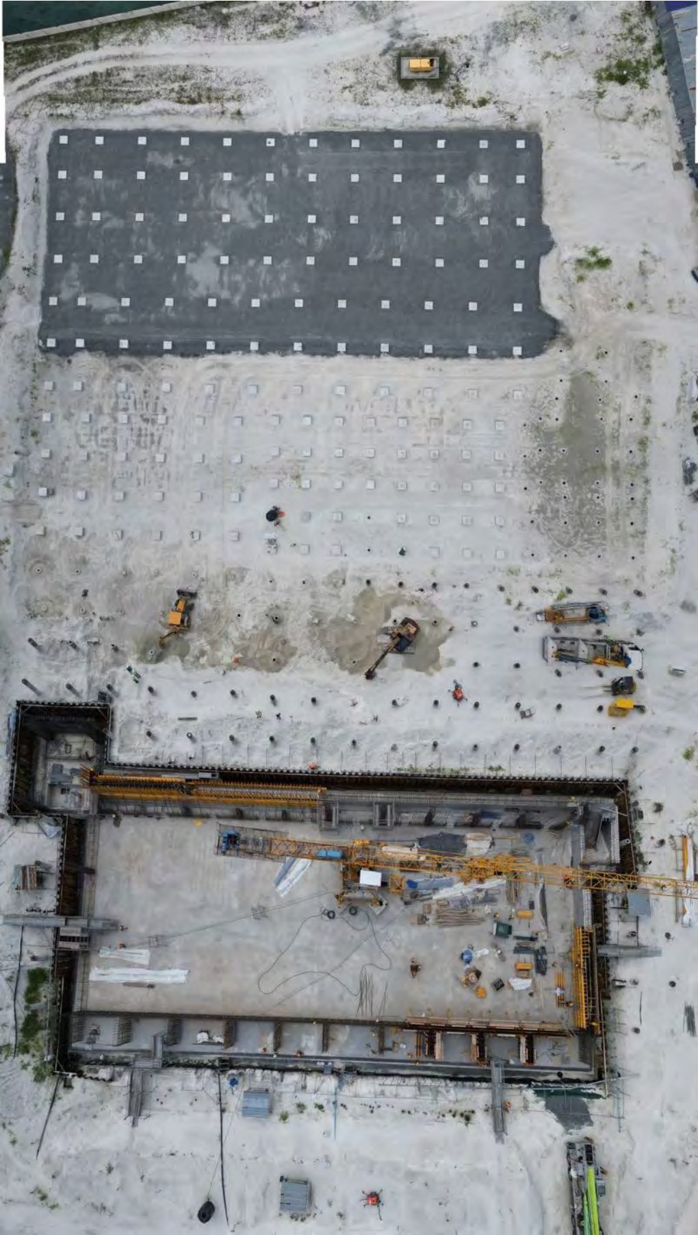
Photo 36 09/05/24 – Main process building and Bunker construction overview.
