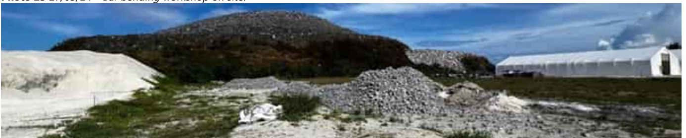
Photo 26 27/03/24 – Excavated sand, and waste concrete stockpile in the laydown area.
