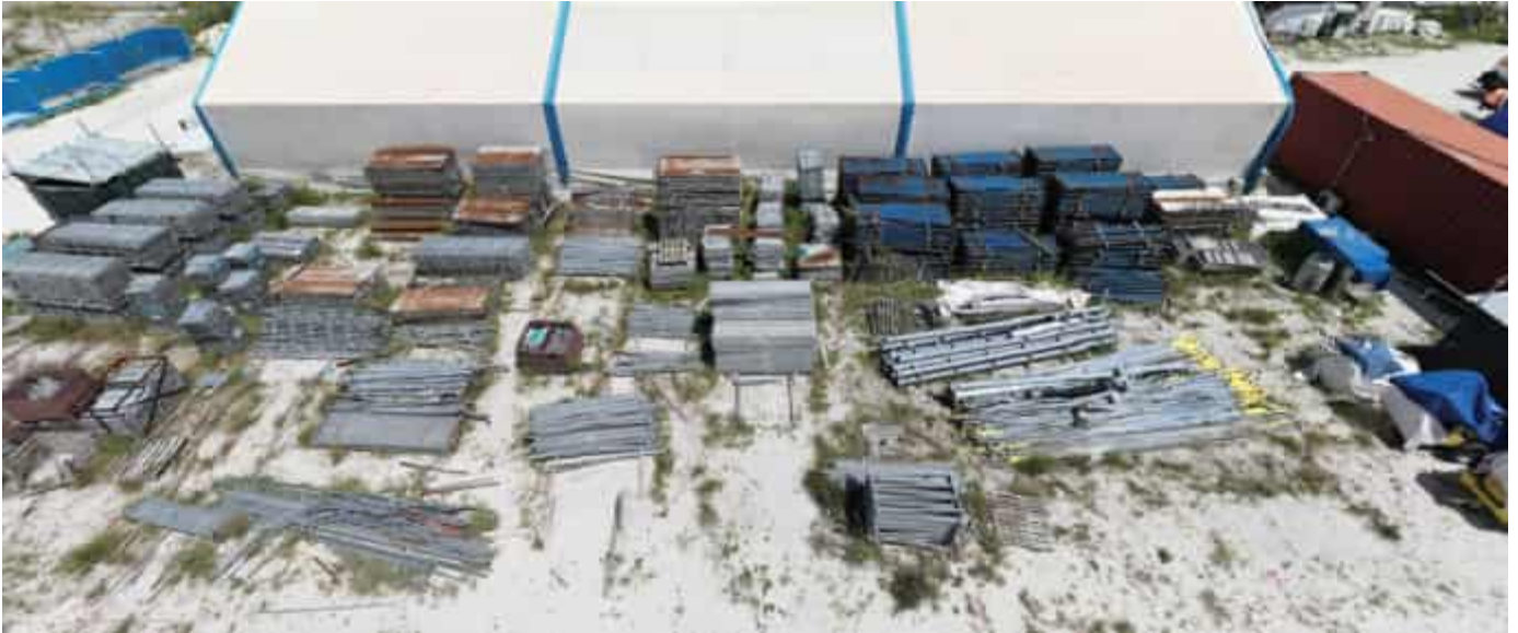
Photo 33 13/06/24 – Scaffolding material being stored close to the storage tent.
