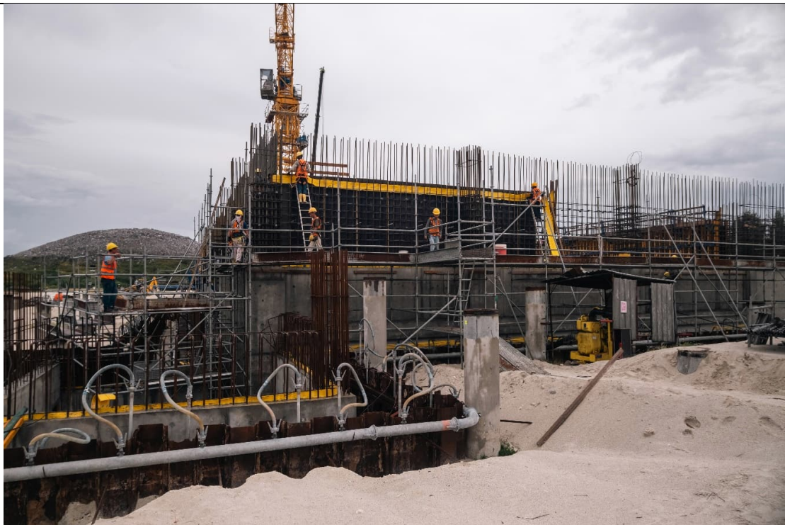
WORKING PLATFORM AND SCAFFOLDING WAS ERECTED BY COMPETENT SCAFFOLDERS
