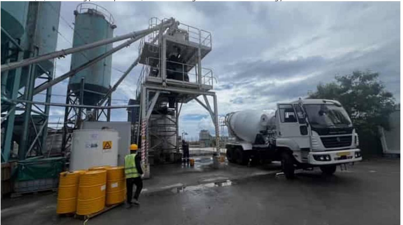
Photo 06 04/04/24 – Batching plant is operational.
