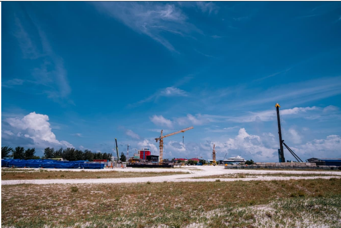
OVERALL VIEW FROM EAST SIDE
