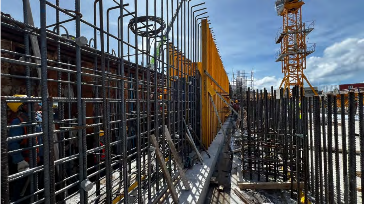
Photo 10 02/05/24 – Bunker wall reinforcement and formwork installation work is ongoing.
