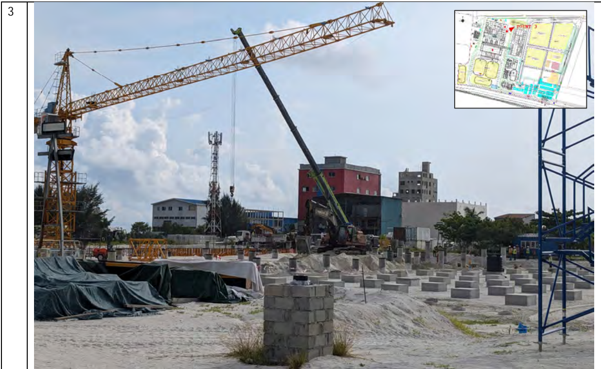
OVERALL - POINT THREE
