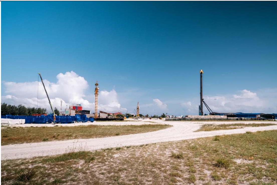
OVERALL VIEW FROM EAST SIDE
