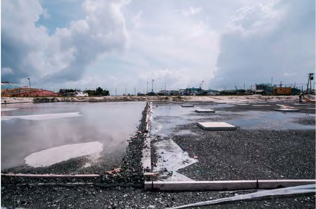
MAIN PROCESS AREA - LEAN CONCRETE PREPARATION
