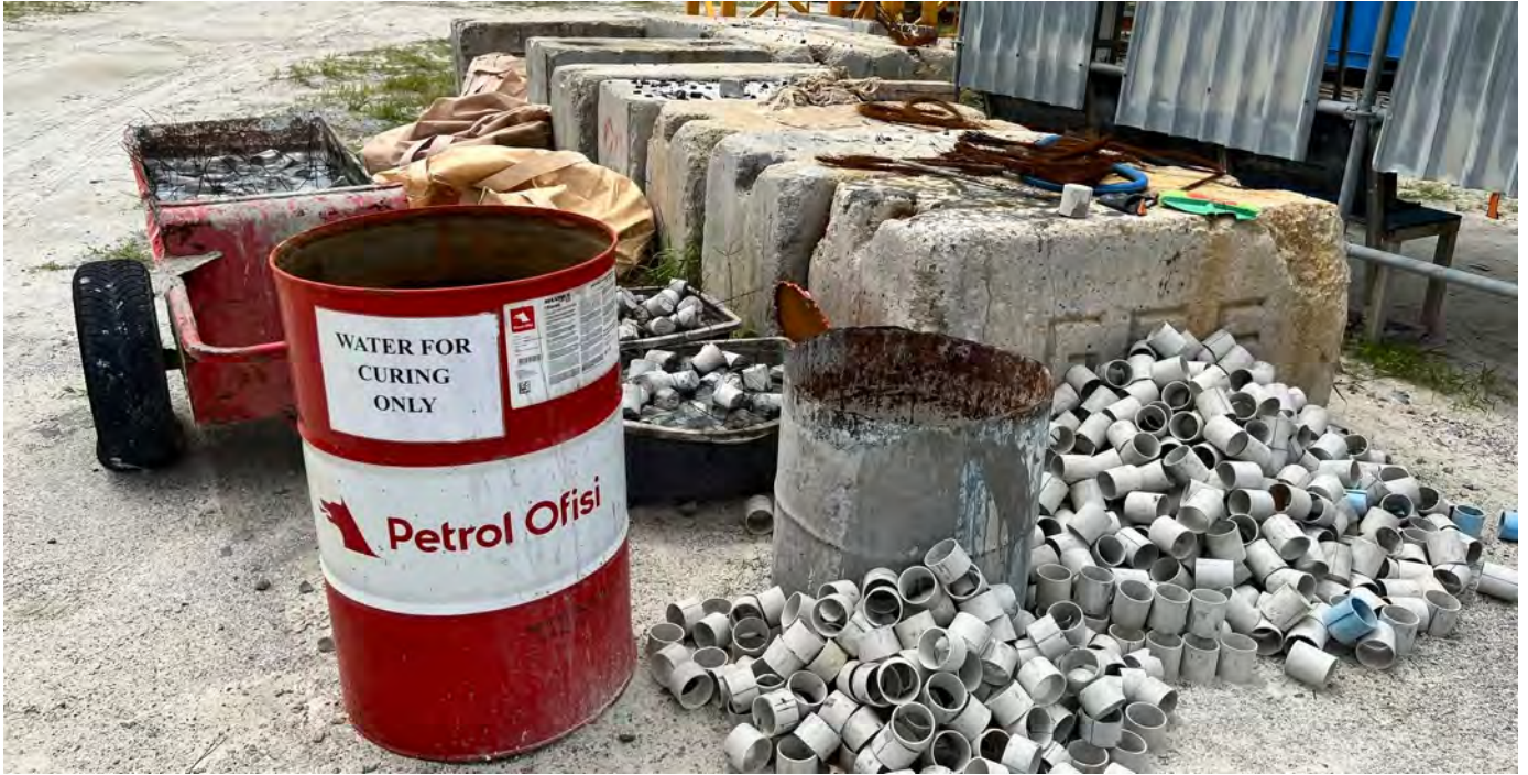
Photo 04 30/05/24 – Cover blocks preparation area, open water tank to be covered to prevent mosquito breeding.
