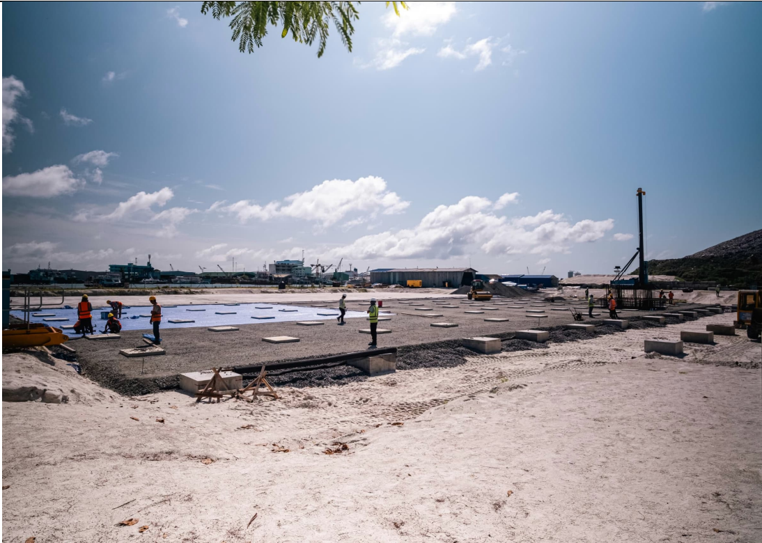
BOILER AREA - BACKFILLING 100% COMPLETED.
