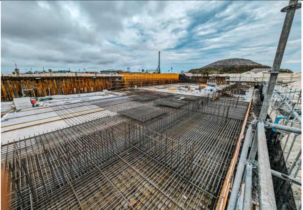
BUNKER AREA - AREA 2 IN PROGRESS.
