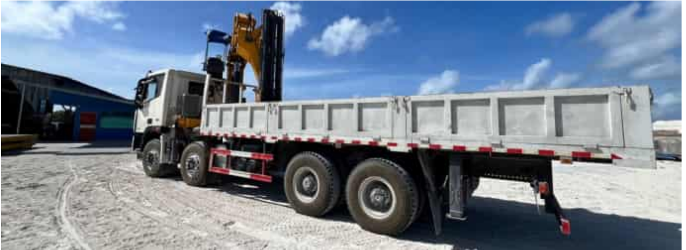
Photo 19 13/06/24 – Several heavy vehicles are being used in the site.
