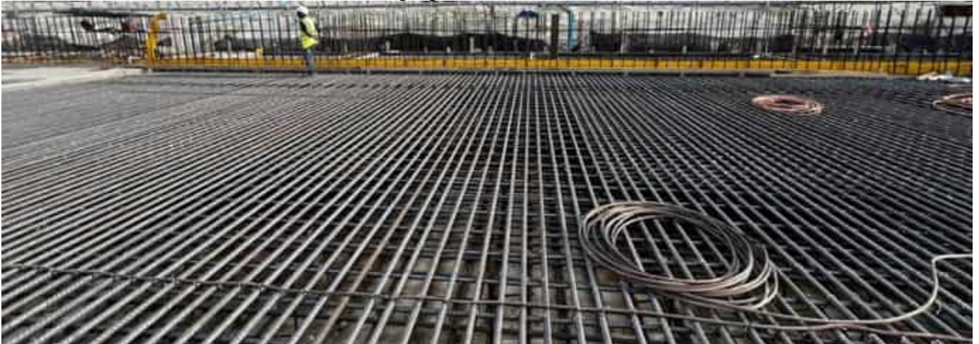
Photo 32 15/04/24 – Earthing cable installed on the reinforcement.
