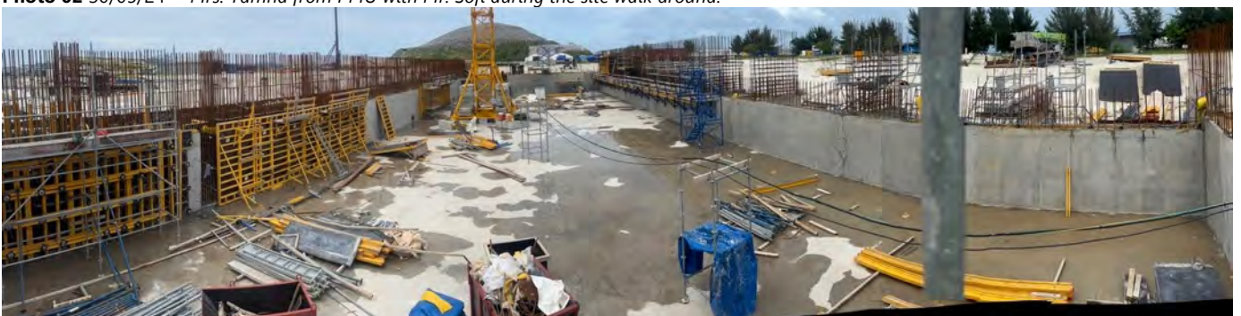
Photo 03 30/05/24 – Bunker wall reinforcement and formwork installation work is ongoing.
