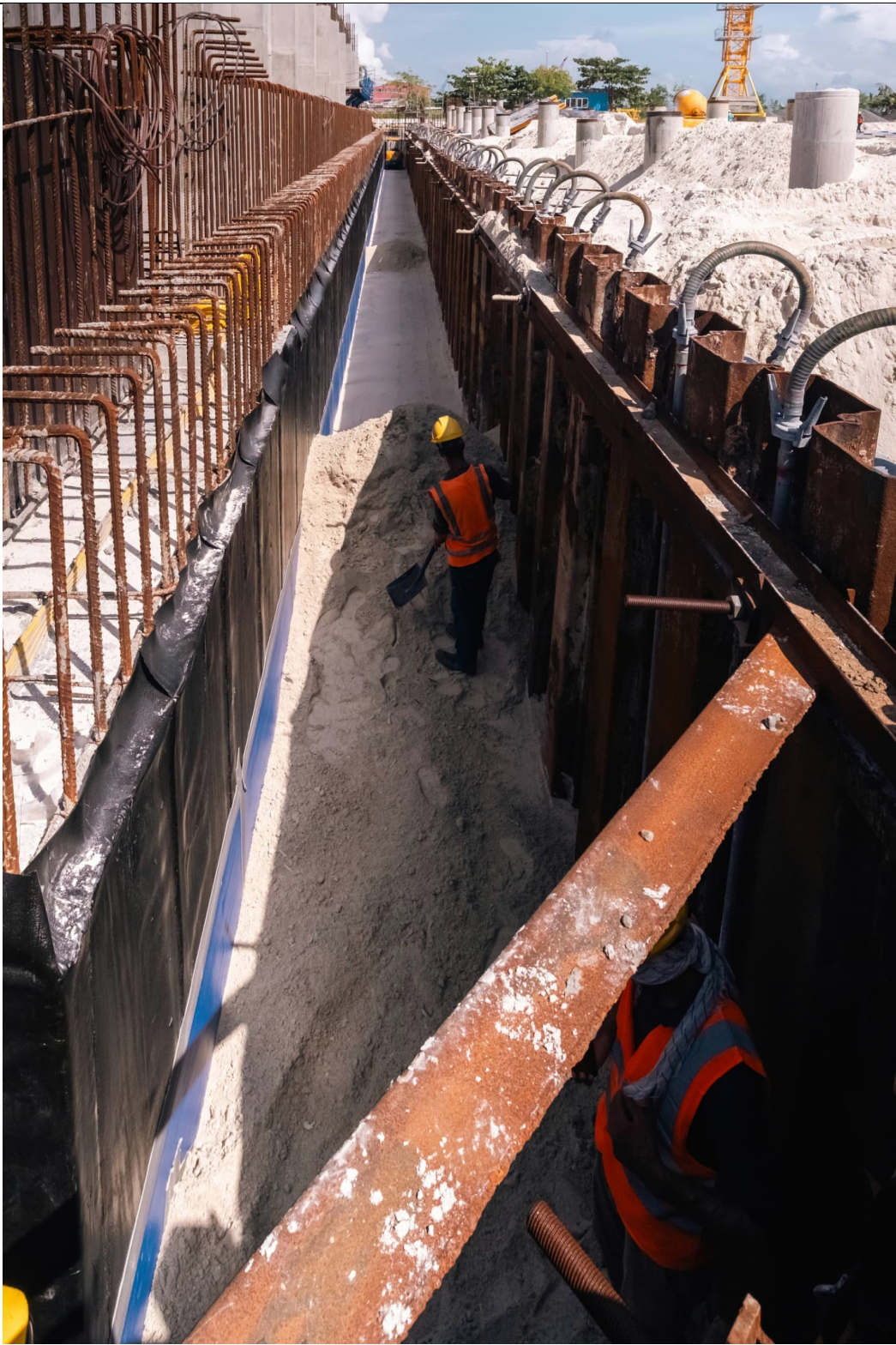
STRUCTURAL BACKFILLING BEHIND BUNKER WALL IN PROGRESS
