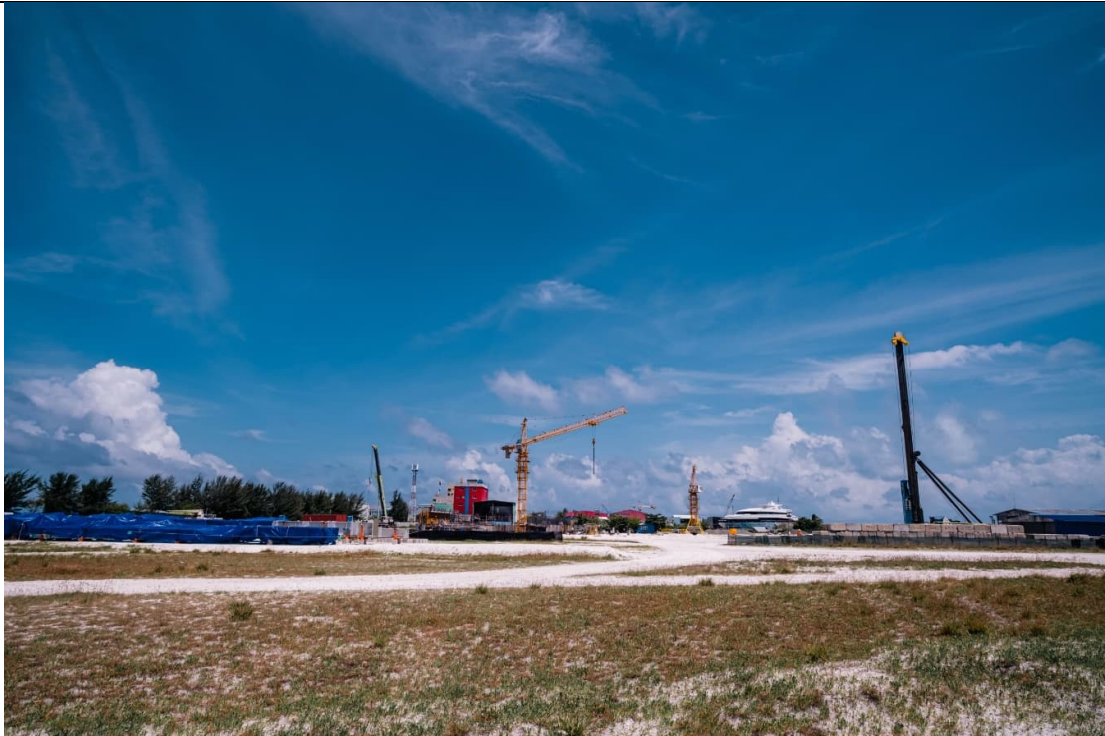
OVERALL VIEW FROM EAST SIDE
