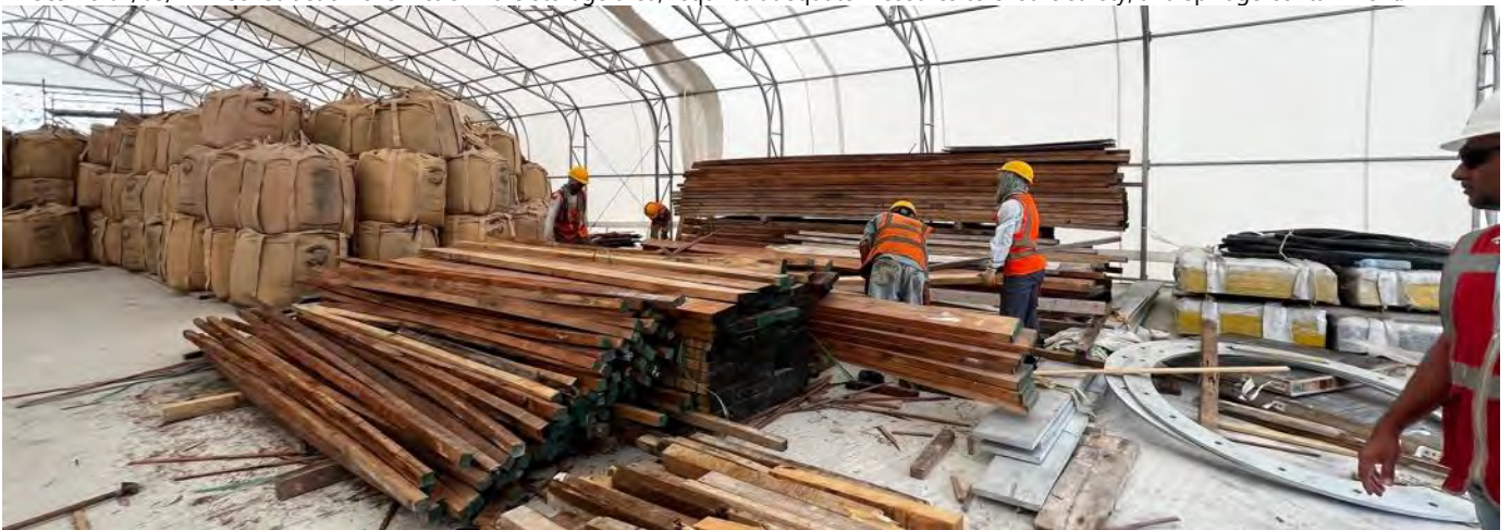
Photo 11 07/05/24 – construction material storage area.
