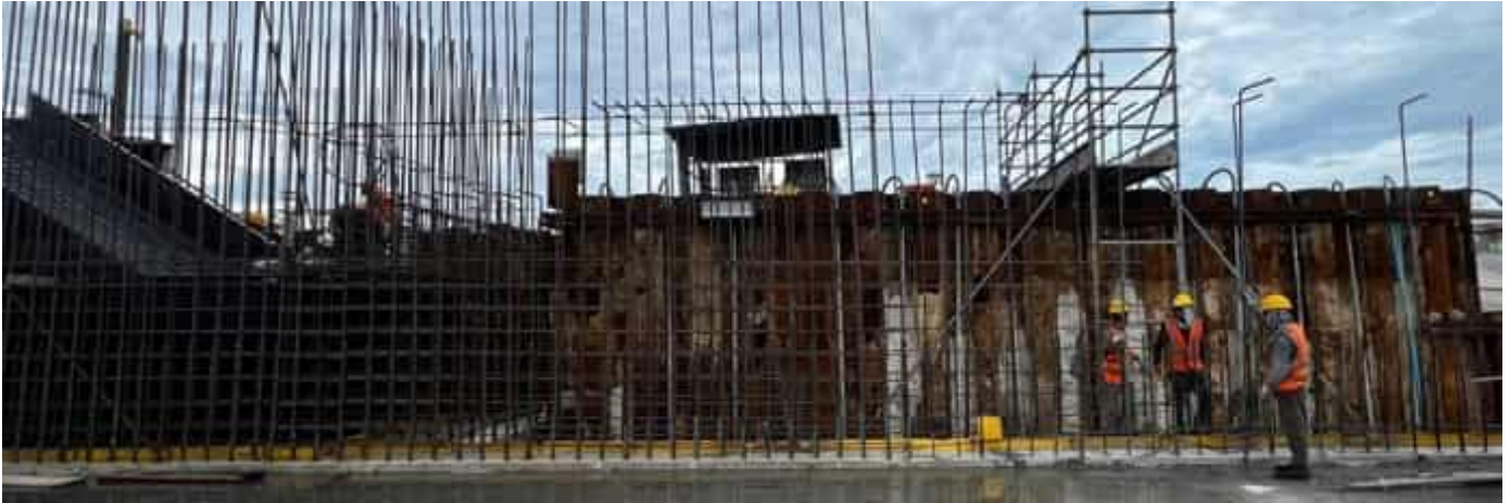
Photo 34 16/04/24 – Reinforcement installment is ongoing for the bunker walls.
