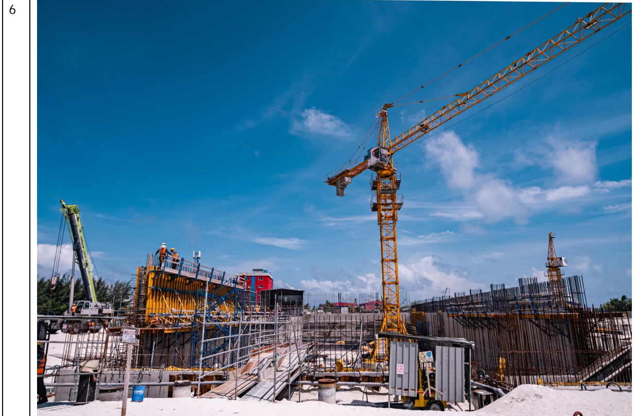
BUNKER AREA - OVERALL BUNKER WALL 2 ND LAYER COMPLETED 80%
