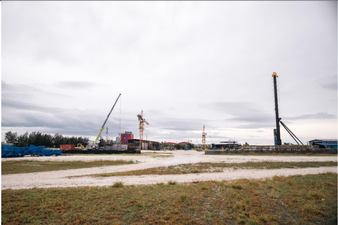
OVERALL VIEW FROM EAST SIDE
