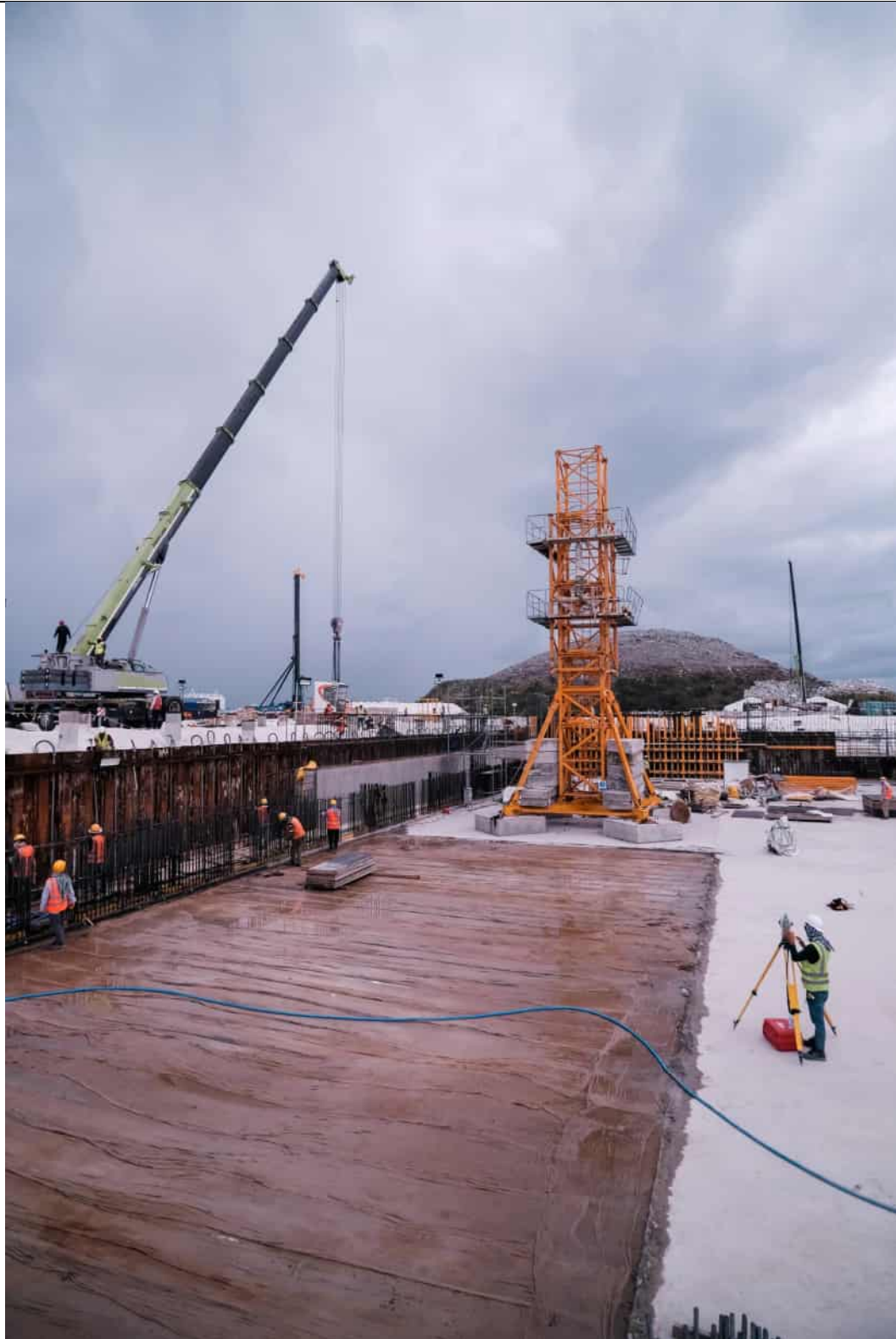
TEMPORARY TOWER CRANE INSTALLATION IN PROGRESS
