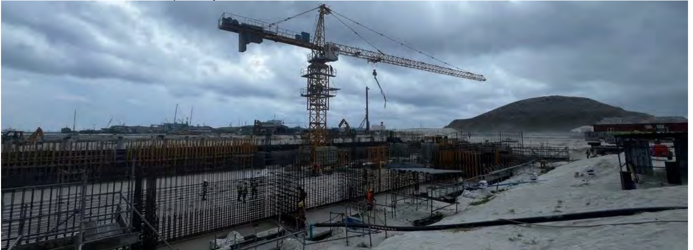
Photo 03 07/05/24 – Bunker wall reinforcement and formwork installation work is ongoing.
