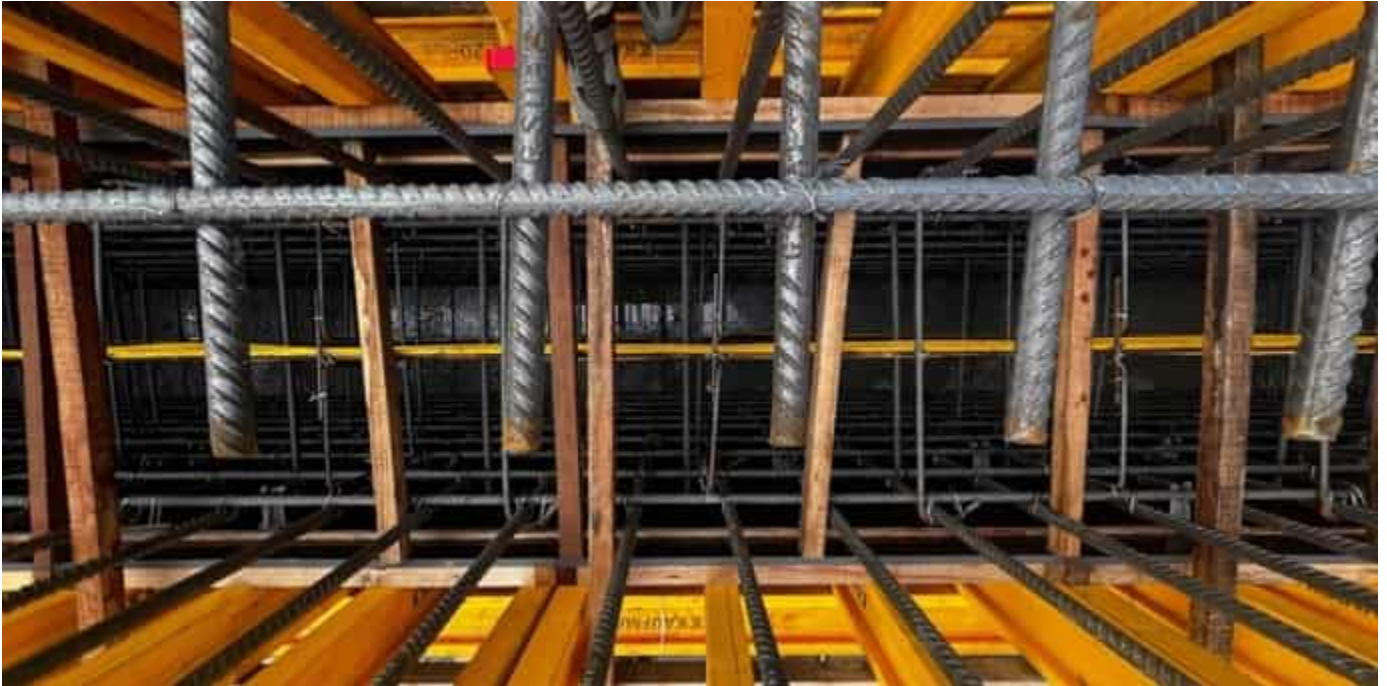
Photo 24 27/03/24 – Wall B is being made ready for concrete pouring.
