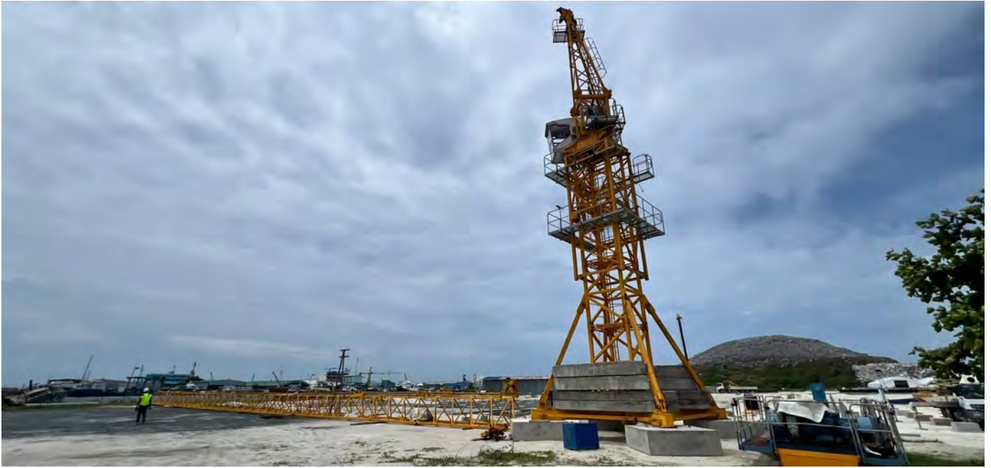
Photo 06 30/05/24 – Installation work for the tower cranes on site are ongoing.
