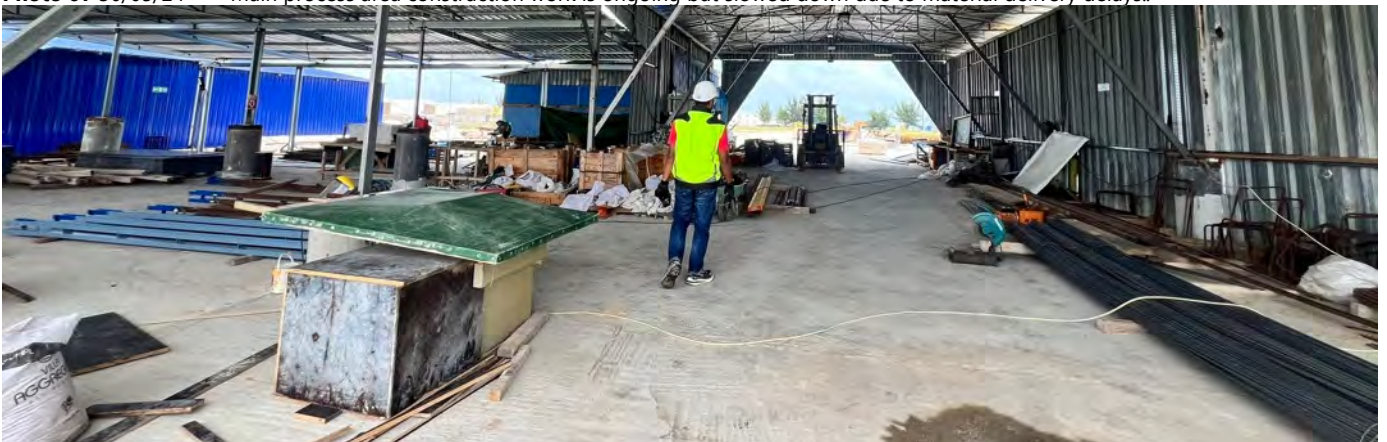
Photo 08 30/05/24 – Reinforcement fabrication workshop area..
