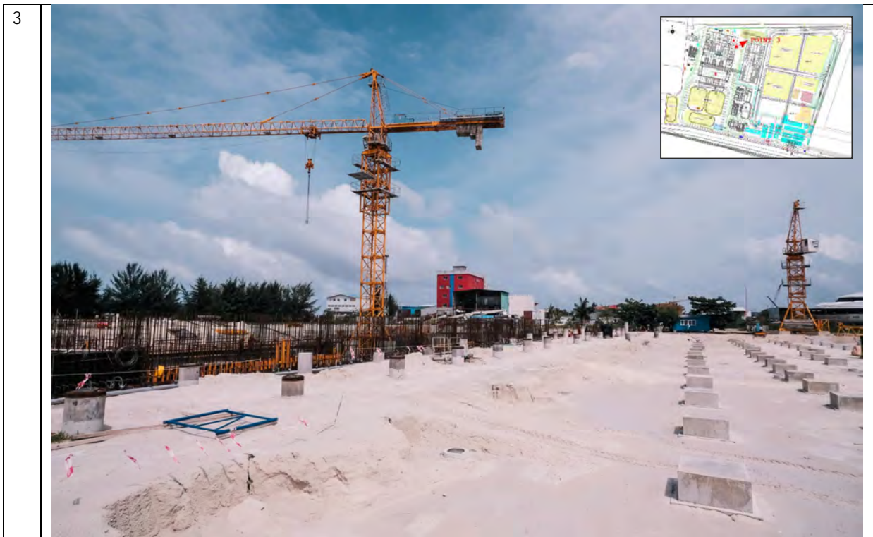
OVERALL - POINT THREE
