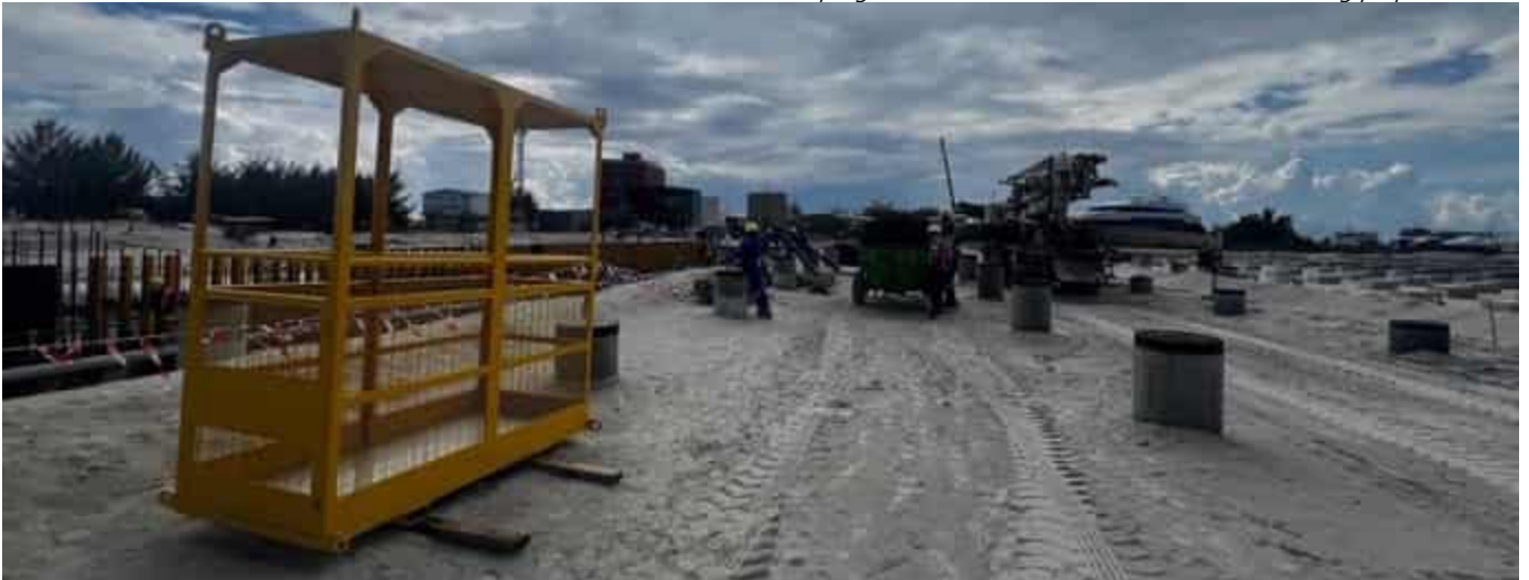
Photo 20 27/03/24 – Cage for safe removal of persons in case of an emergency has been bought and brought to site.
