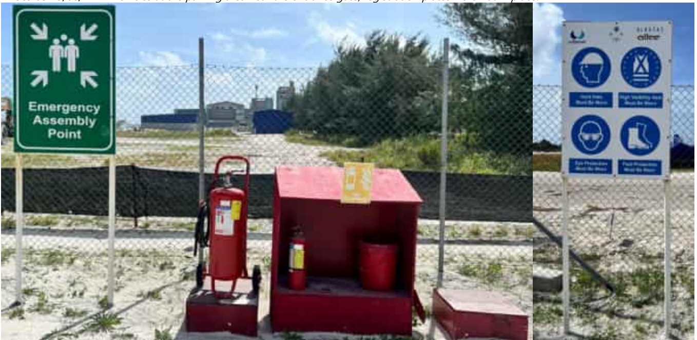
Photo 06 13/06/24 – Safety signage is placed around the site and maintained, and fire fighting stations also maintained.
