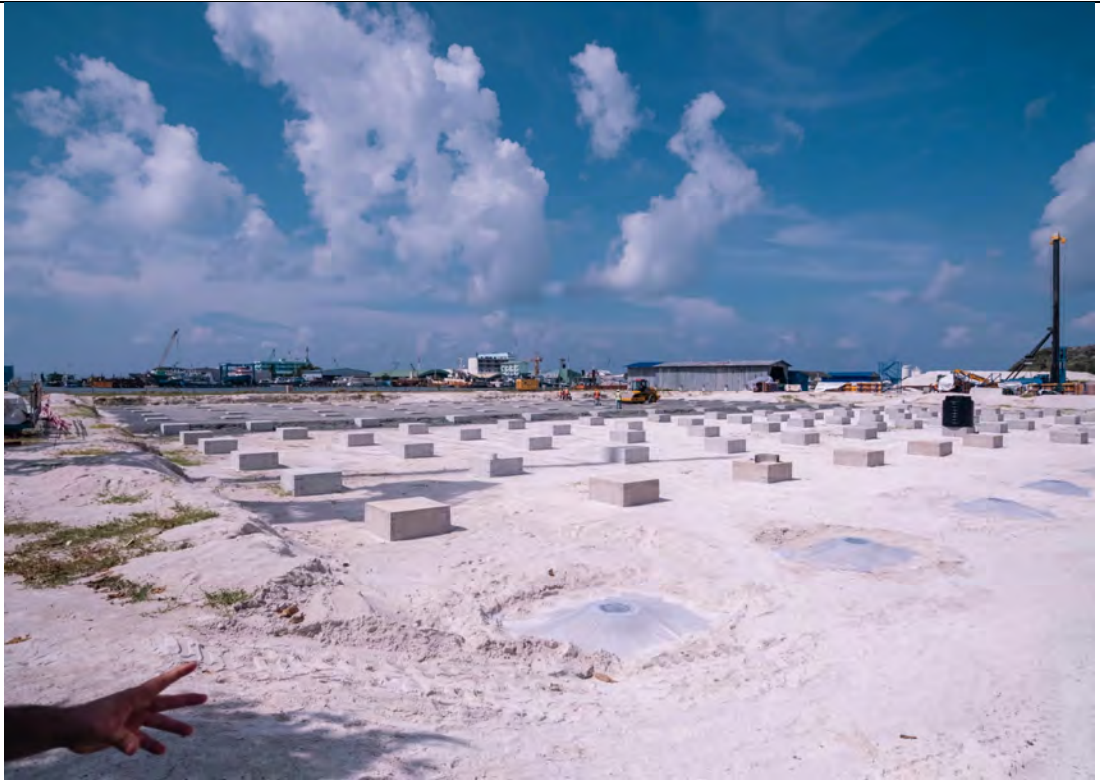
MAIN PROCESS AREA - PILE CUTTING AND COMPACTION IN PROGRESS
