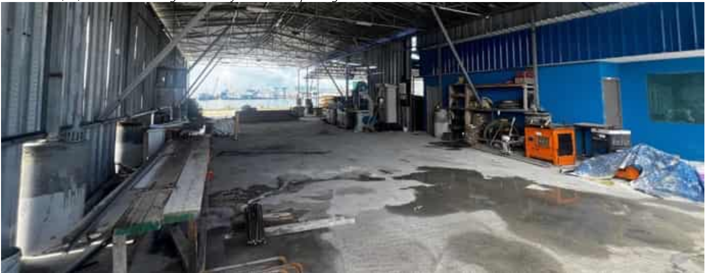
Photo 25 27/03/24 – Bar bending workshop on site.
