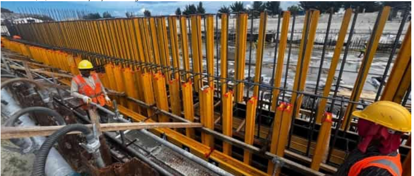
Photo 23 27/03/24 – Wall B is being made ready for concrete pouring.
