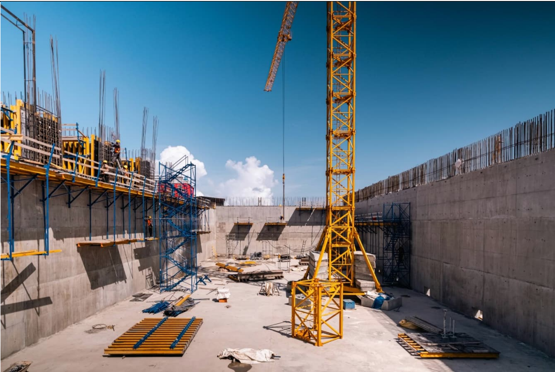
BUNKER - VIEW FROM INSIDE (EAST)
