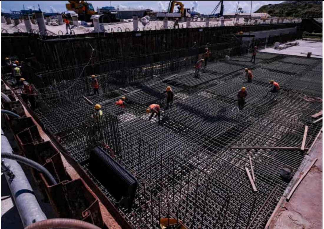
BUNKER - AREA 3 REINFORCEMENT BAR AND FORMWORK IN PROGRESS.
