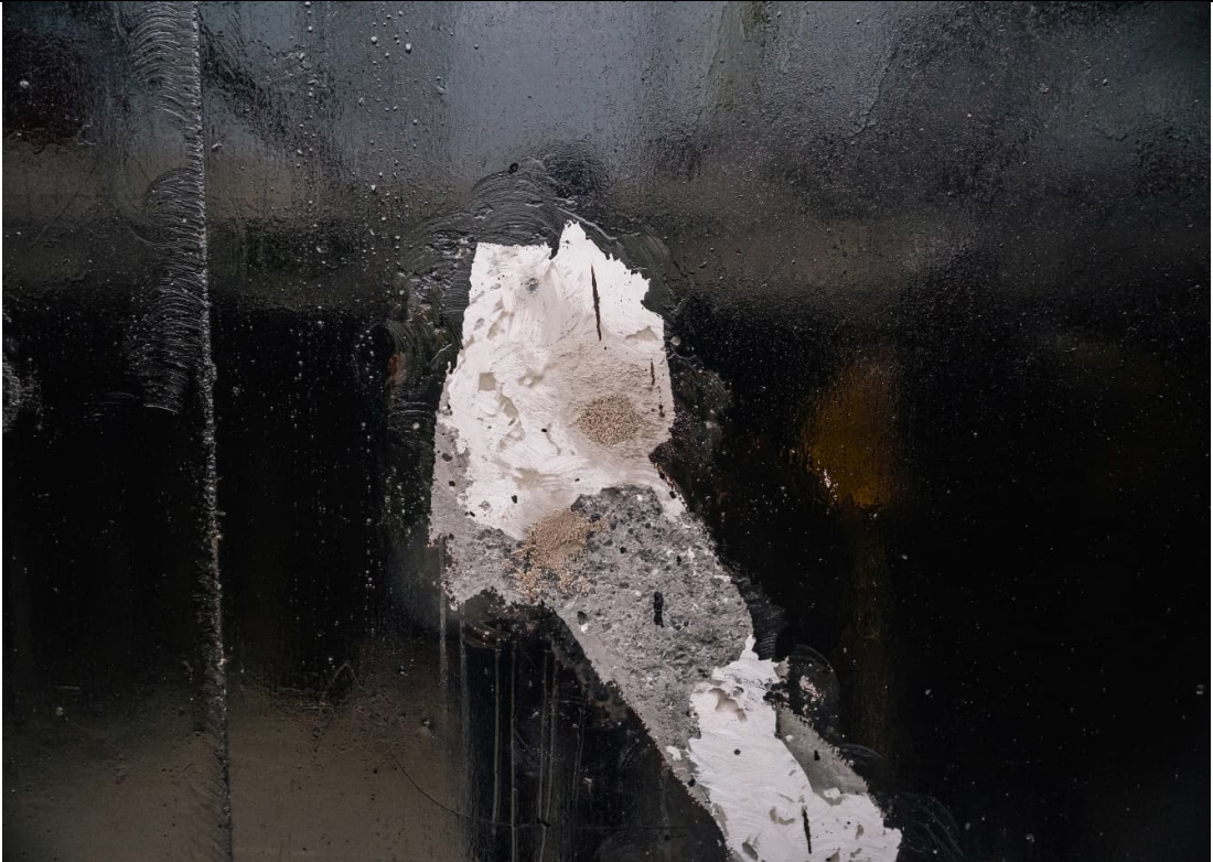
BUNKER AREA - CRACK REMEDIAL WORK IN PROGRESS
