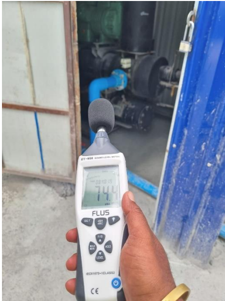
Batching Plant Chiller Plant Pump
