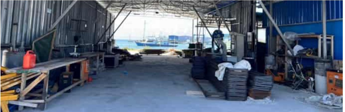
Photo 15 13/06/24 – Bar bending works are ongoing.
