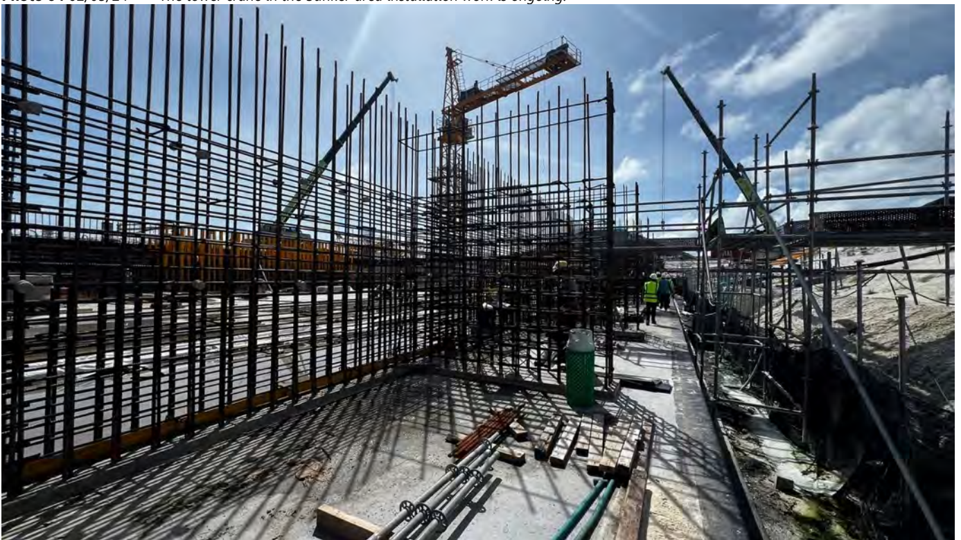
Photo 05 02/05/24 – Bunker wall reinforcement and formwork installation work is ongoing.
