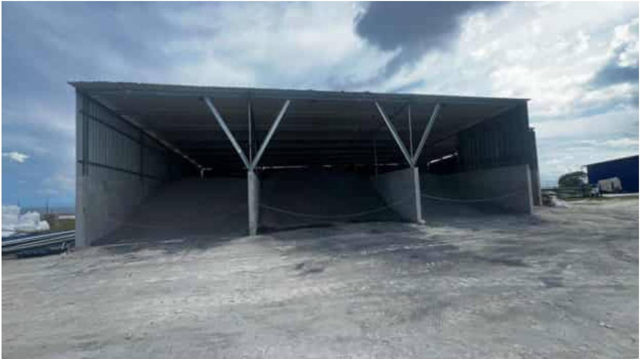
Metal sheets provided for dust suppression in storage area of construction materials in batching plant area
