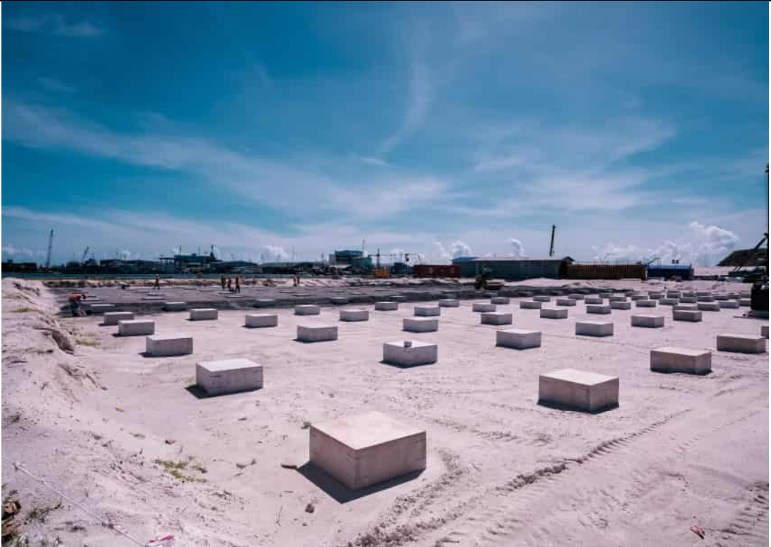
PROCESS AREA - COMPACTION WORK IN PROGRESS
