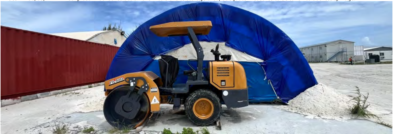
Photo 12 30/05/24 – New machinery on site.
