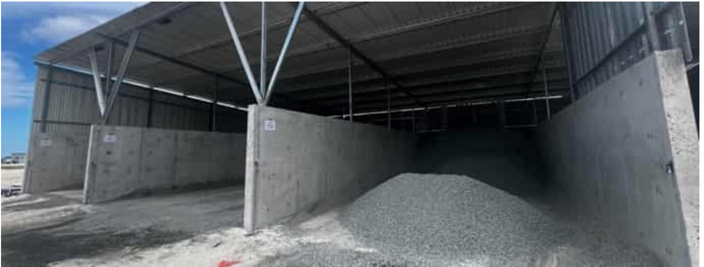
Photo 09 04/04/24 – Aggregate storage area for the concrete batching plant.
