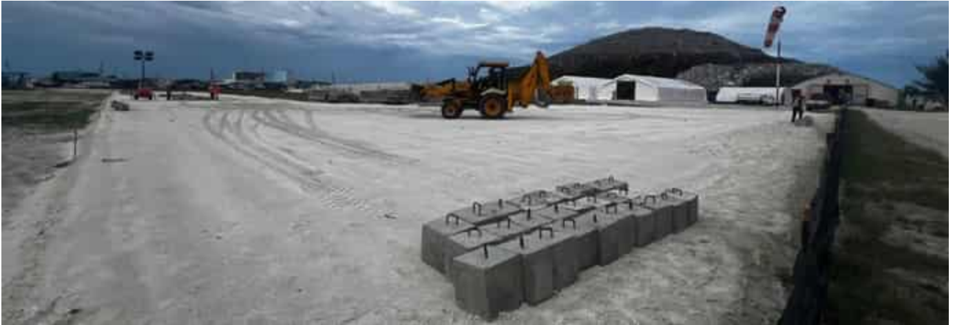
Photo 37 16/04/24 – Equipment laydown area being prepared for .
