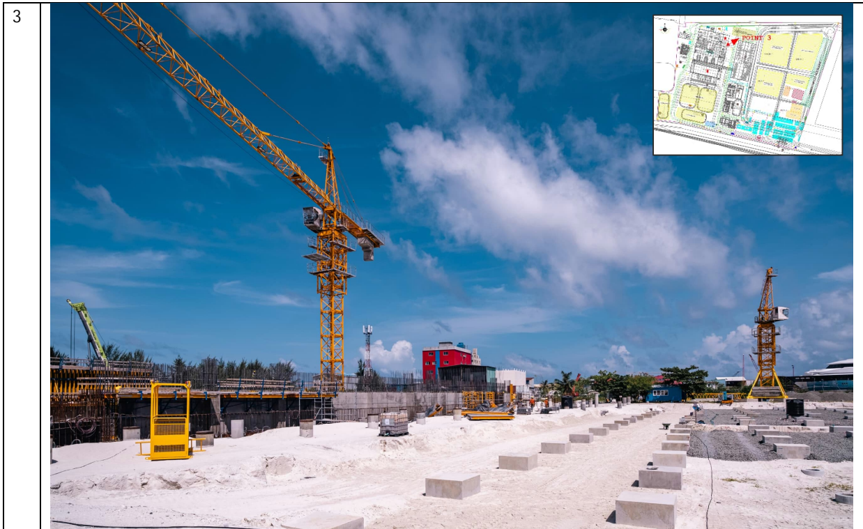
OVERALL - POINT THREE
