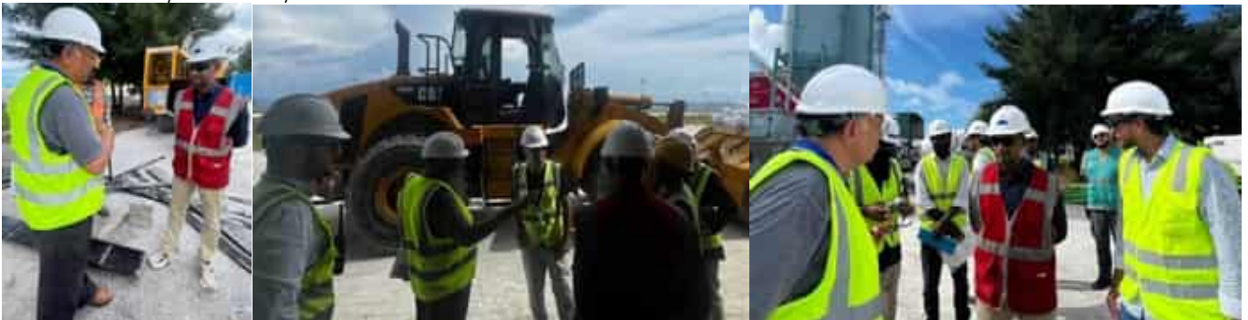
Photo 08 14/04/24 – Mr. Sunil conducting site walk about with EPC site team.
