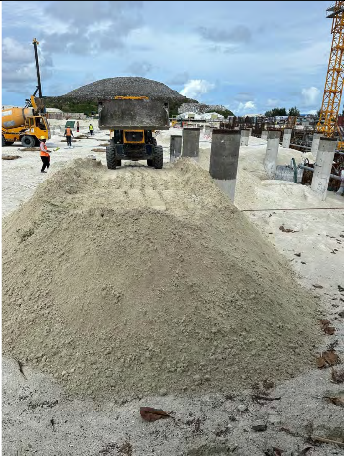
REINSTALLATION FOR SHEETPILE ANCHOR COMPLETED
