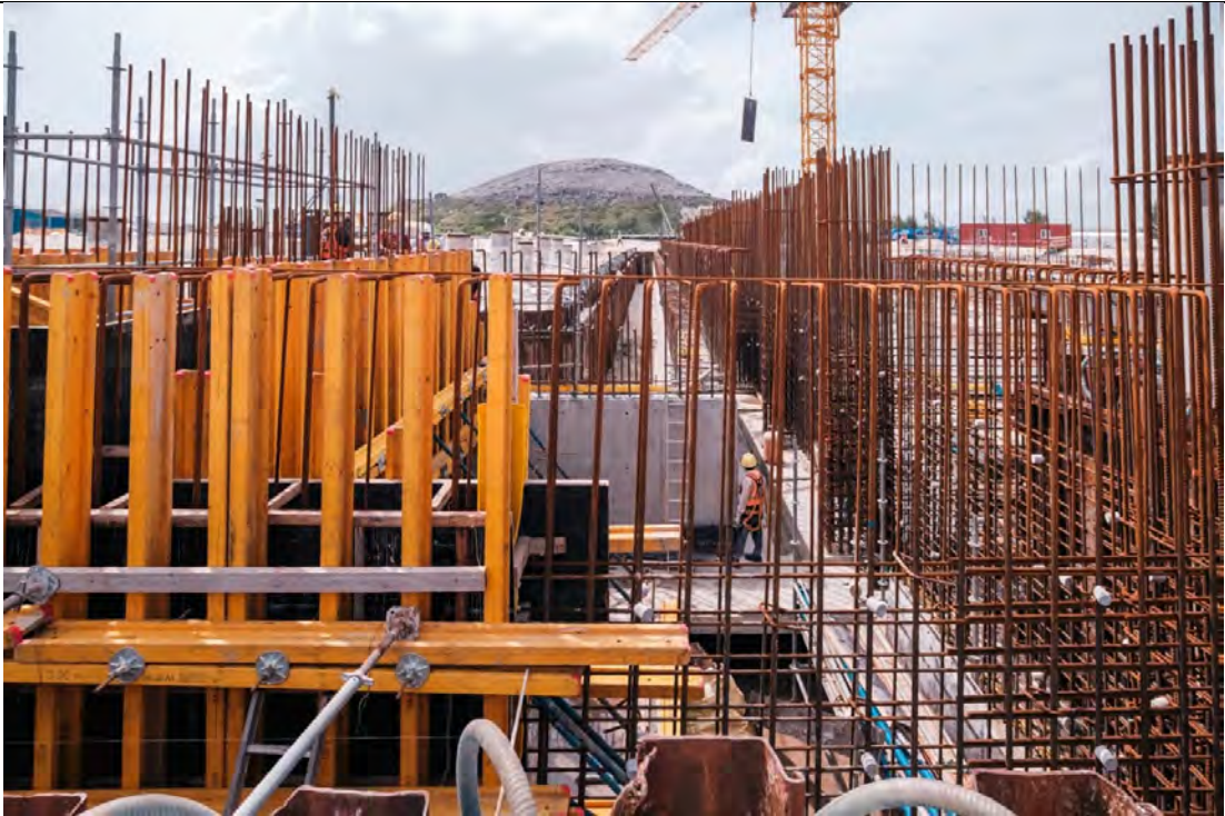
BUNKER - LEACHATE AREA WALL IN PROGRESS
