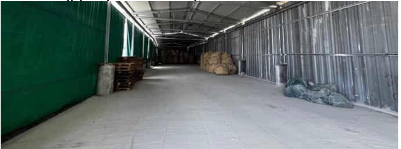
Photo 10 04/04/24 – Cement storage area for the concrete batching plant.
