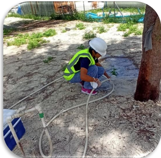
Supply Water for Camp And Construction Sampling
