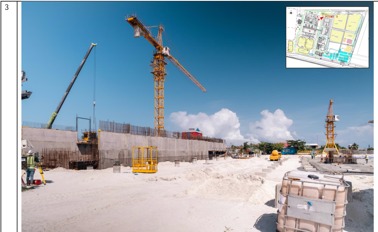
OVERALL - POINT THREE
