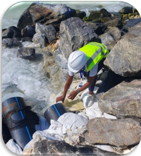
Dewatering Effluent Sampling
