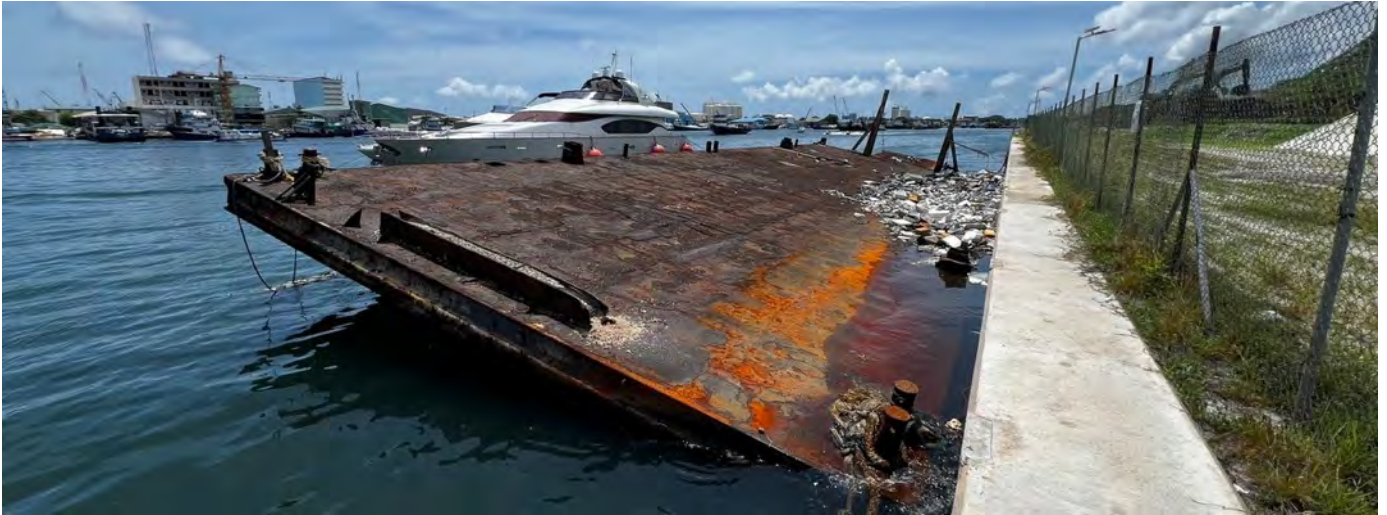
Photo 20 02/05/24 – The barge next to the quay wall has been damaged and is sinking, MOE has been informed of this issue.
