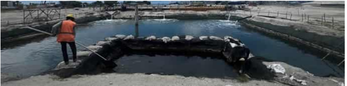
Photo 01 04/04/24 – Continuous dewatering is ongoing, dewatering pond is kept clean.
