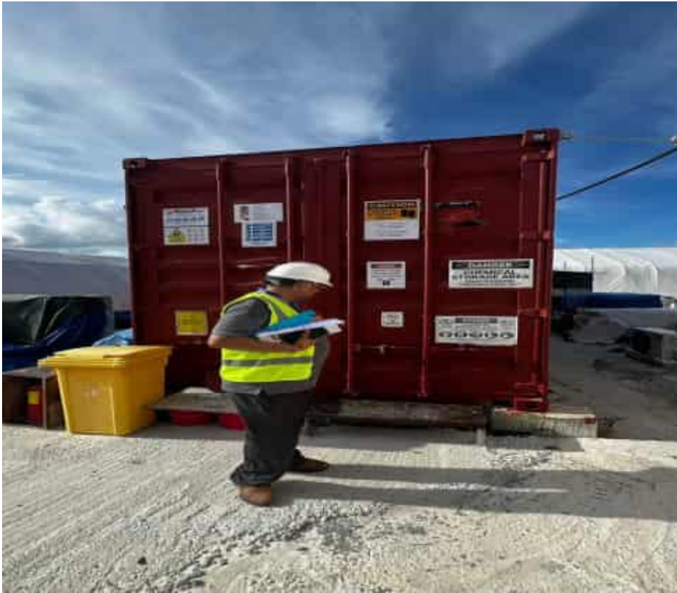
Hazardous chemical storage container and Spill Kit
