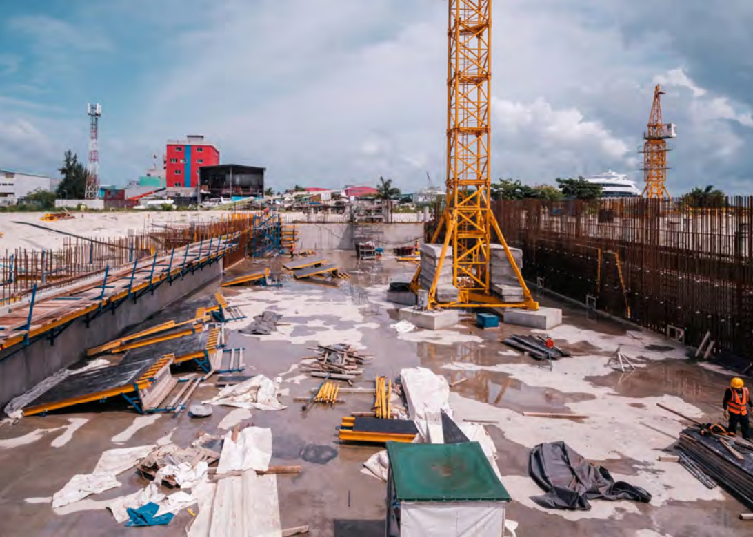
BUNKER AREA - WALL D, I & G IN PROGRESS
