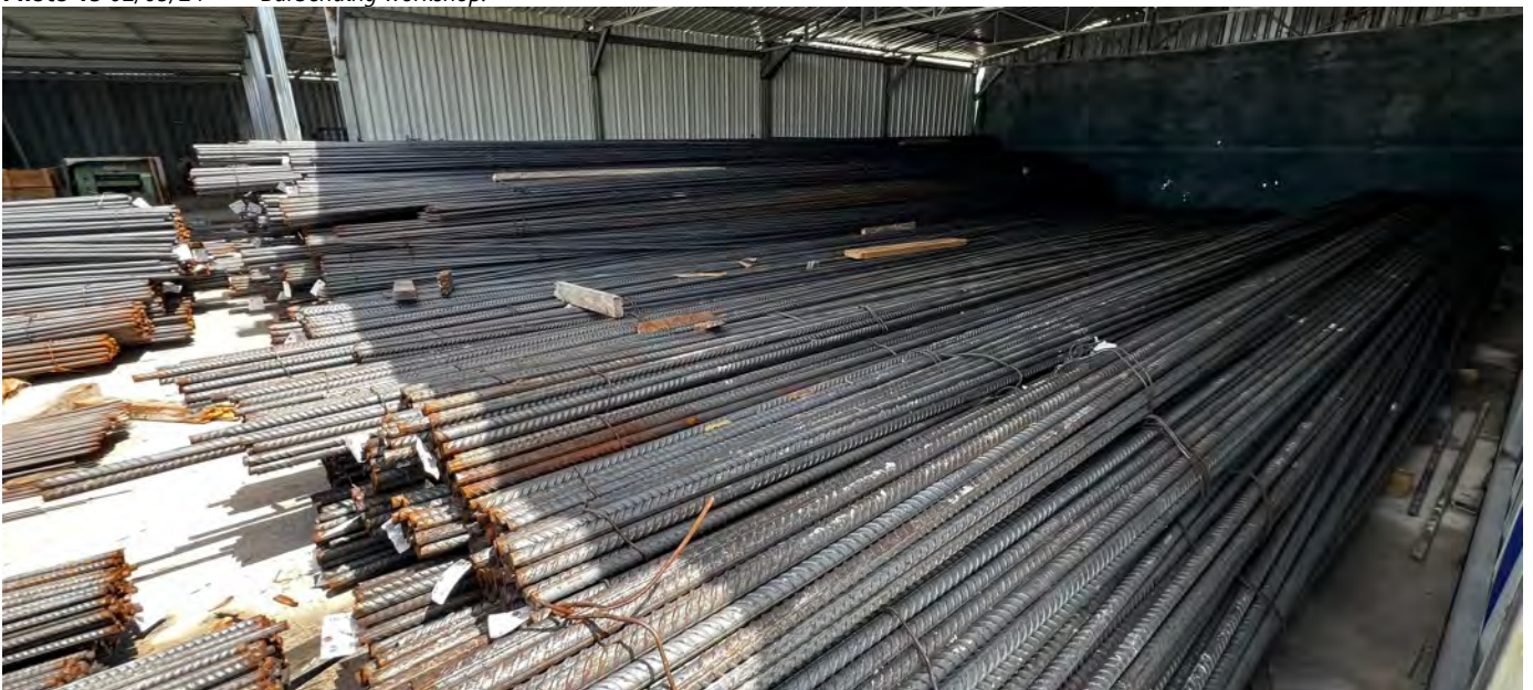
Photo 16 02/05/24 – Rebar stock on site.
