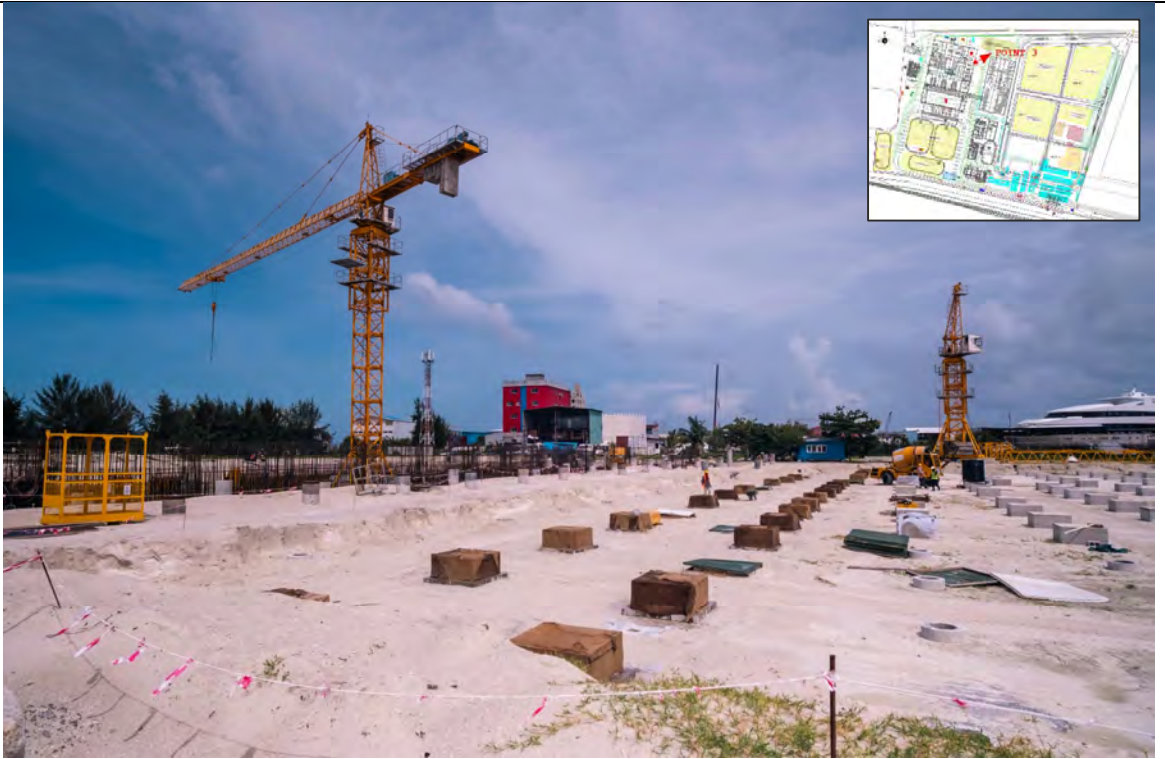
OVERALL - POINT THREE
