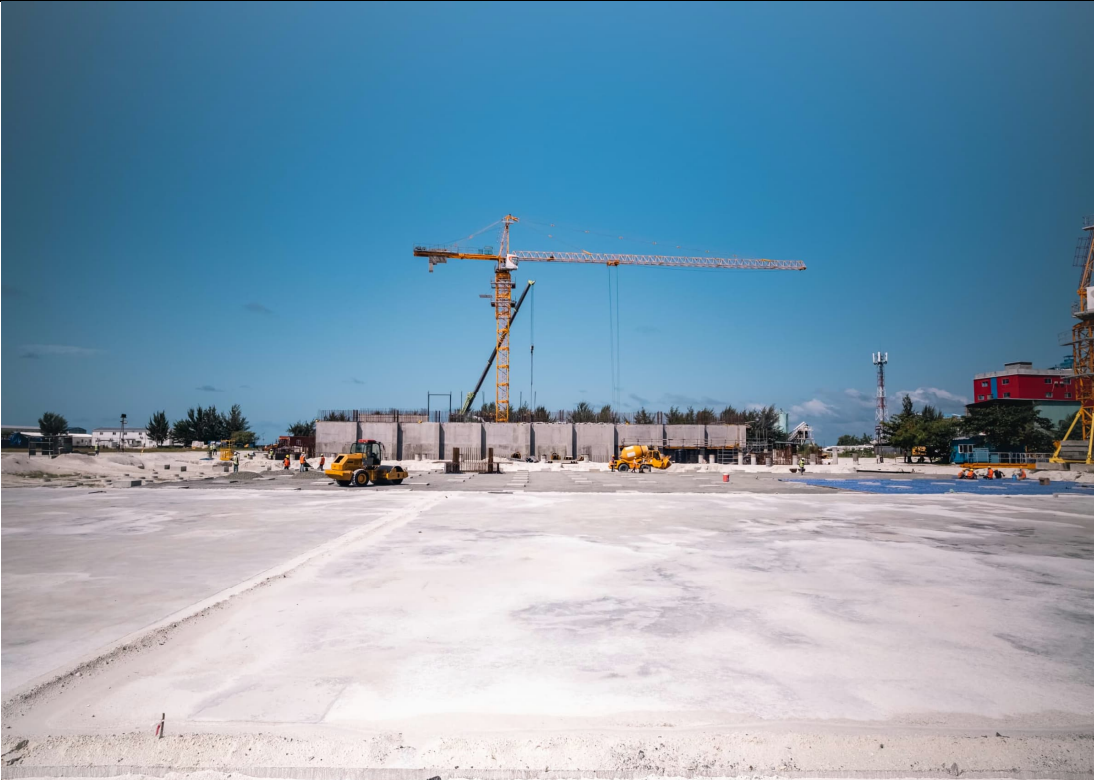
APC AREA - LEAN CONCRETE 100% COMPLETED.
