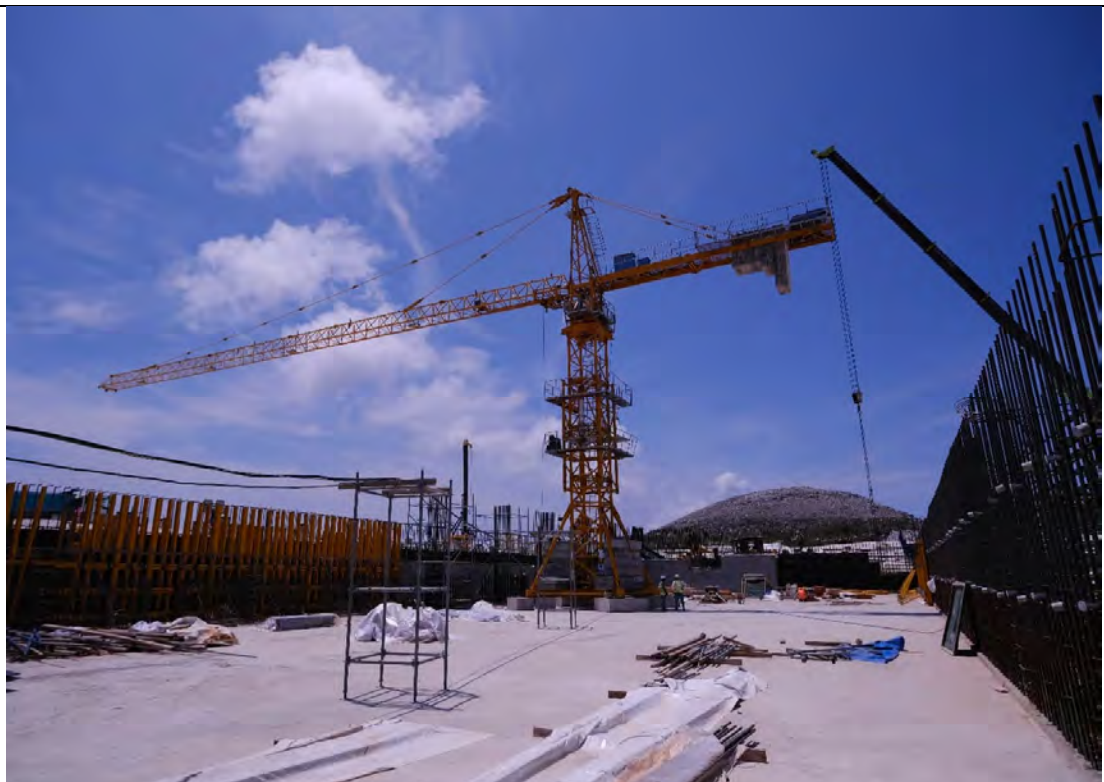
TEMPORARY TOWER CRANE INSTALLATION IN PROGRESS
