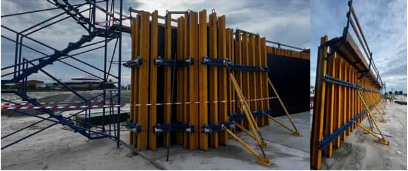
Photo 27 15/04/24 – Sample scaffolding setup for inspection.
