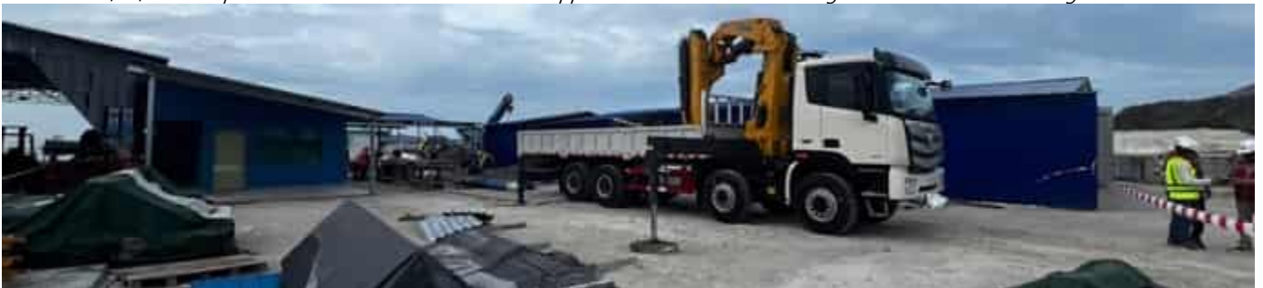
Photo 26 15/04/24 – New crane truck being used on site.
