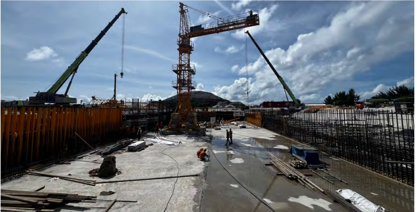
Photo 04 02/05/24 – The tower crane in the bunker area installation work is ongoing.
