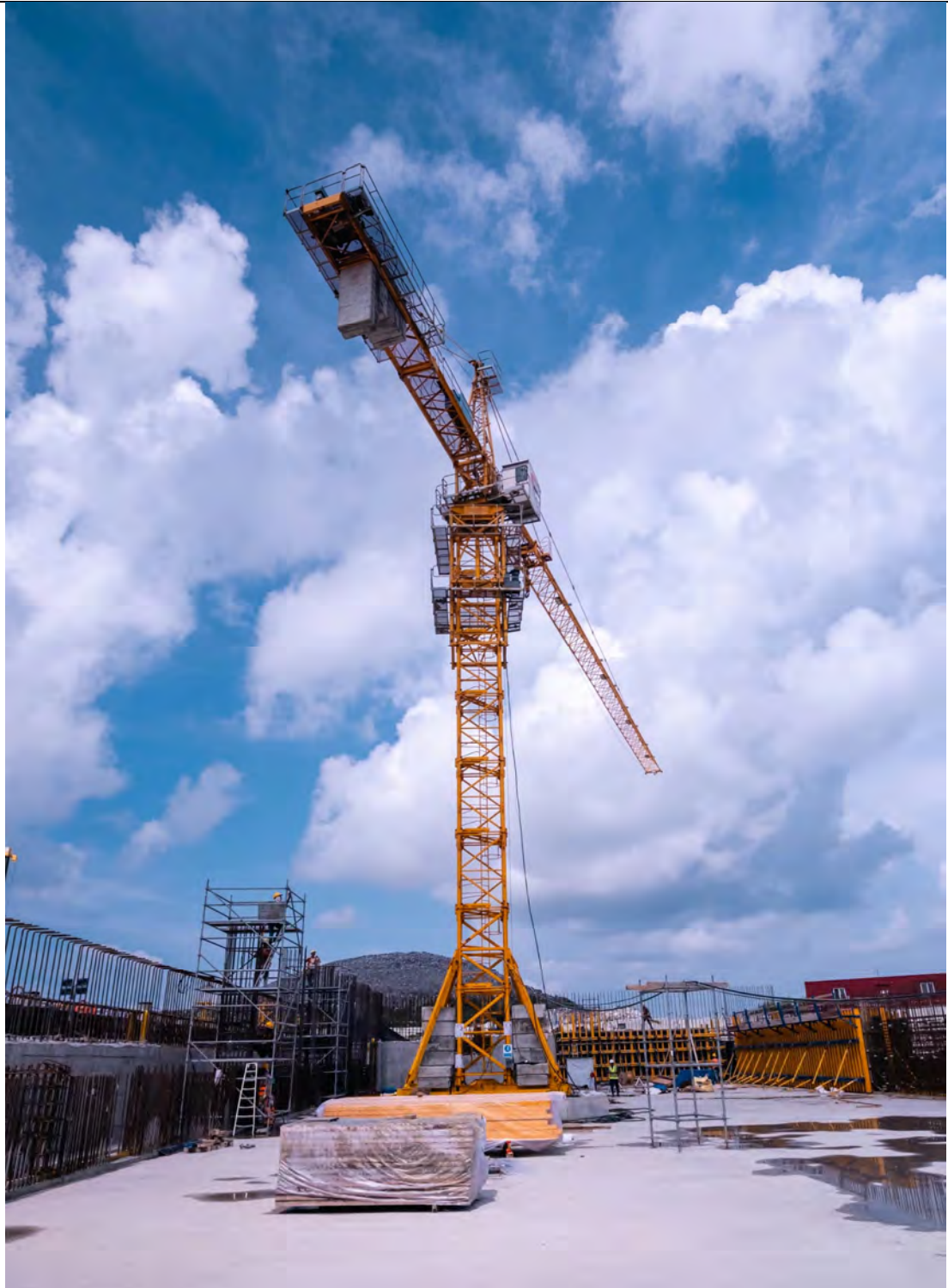
TEMPORARY TOWER CRANE INSTALLATION IN PROGRESS
