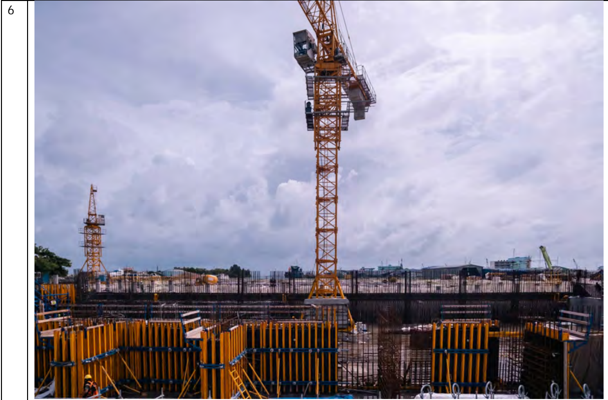
BUNKER AREA - WALL J, C, H, G & I COMPLETED (+0 LEVEL)
