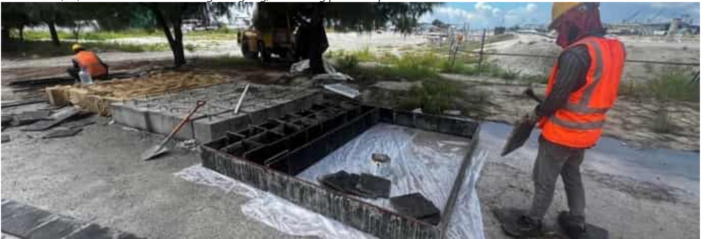
Photo 02 04/04/24 – Concrete blocks for equipment laydown area being prepared.
