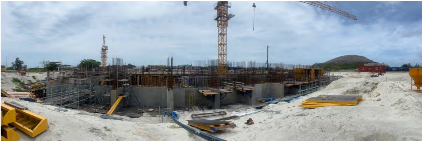
Photo 01 30/05/24 – Construction of the bunker walls ongoing.
