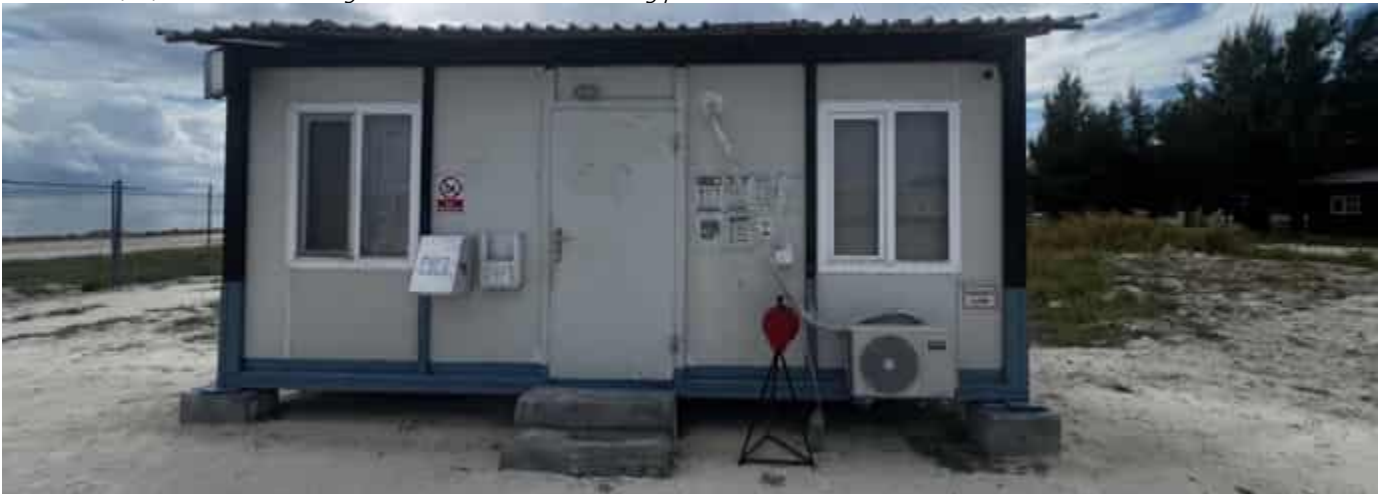
Photo 12 04/04/24 – Security office on site near the main entrance gate.
