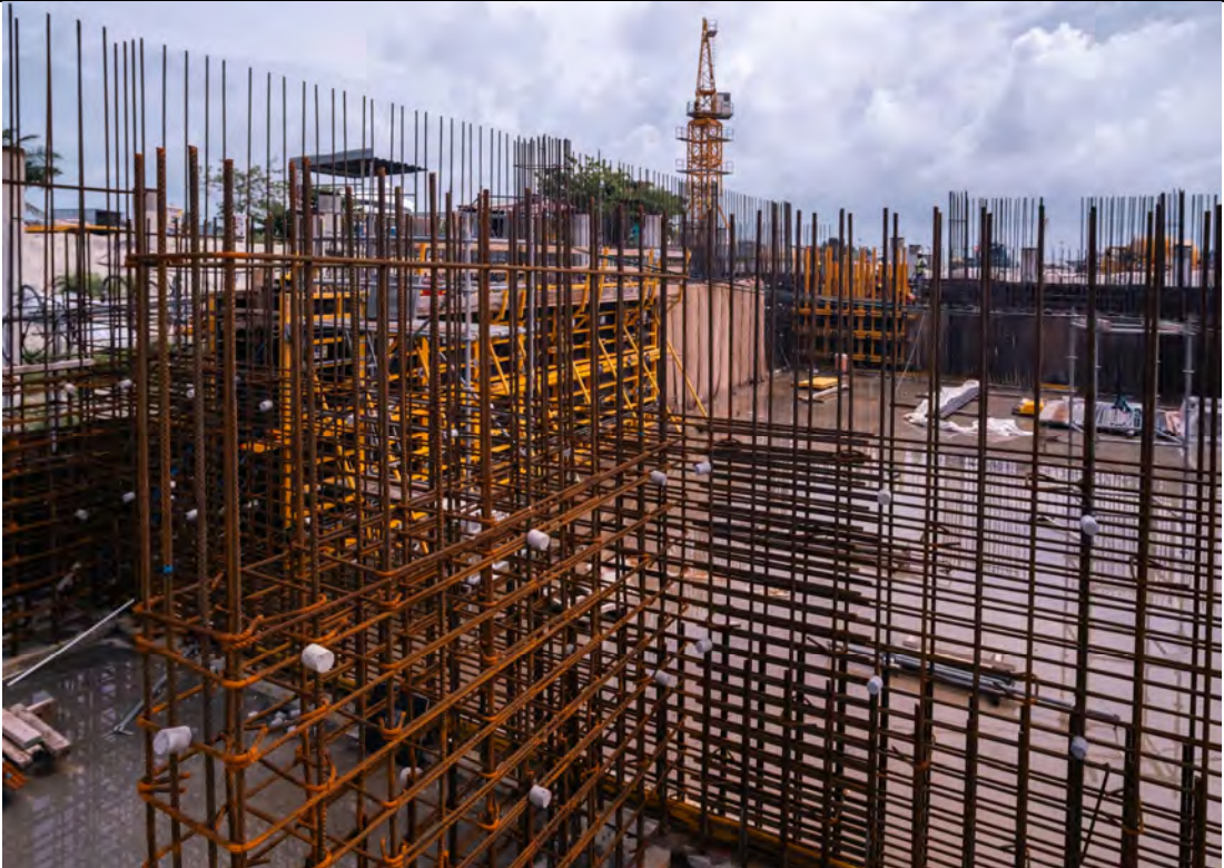
BUNKER AREA - WALL D & F IN PROGRESS
