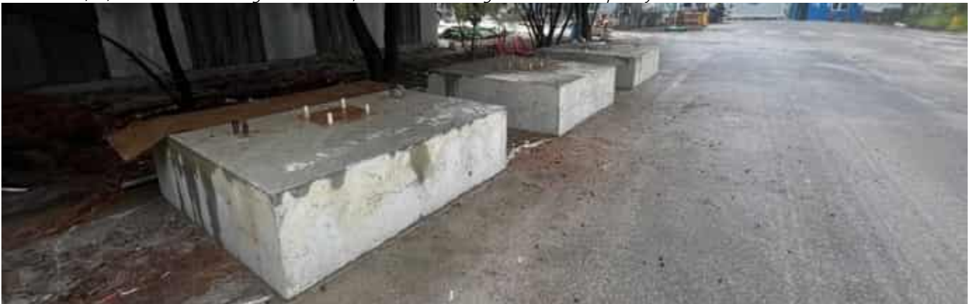
Photo 04 04/04/24 – Concrete blocks for the equipment laydown area being prepared.
