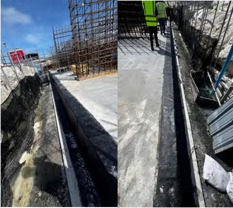
Photo 06 02/05/24 – Waterproofing membranes on the bunker slab being installed.
