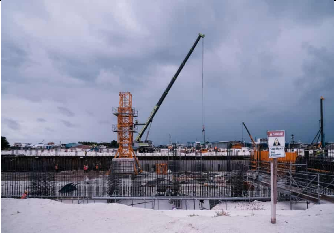
BUNKER AREA - AREA 3 & LEACHATE AREA CONCRETING COMPLETED.
