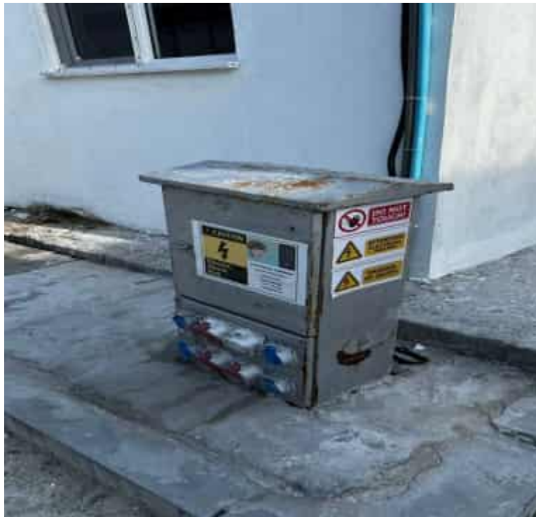
Electrical hazard- Open socket
