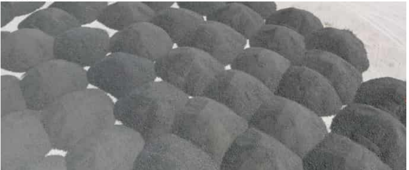
Photo 26 13/06/24 – Backfilling material for the main process building area has been delivered to site.
