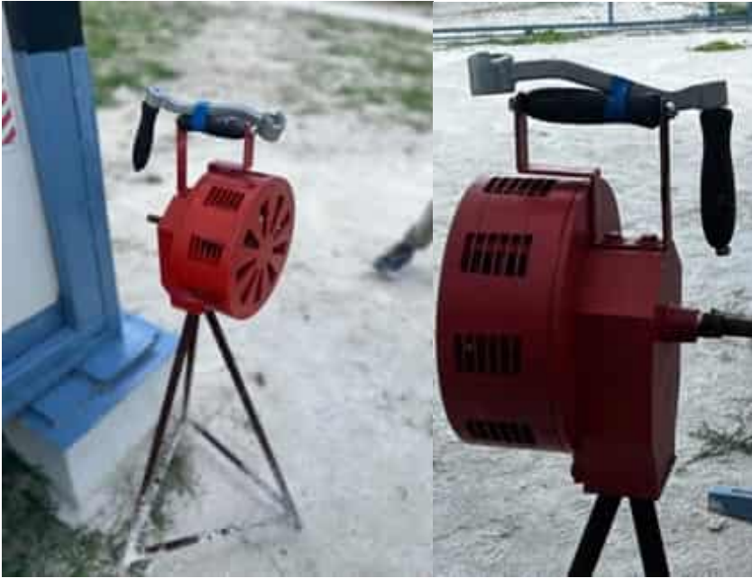
Photo 06 14/04/24 – Rust seen on the siren, should have SOP for maintenance of these in place.
