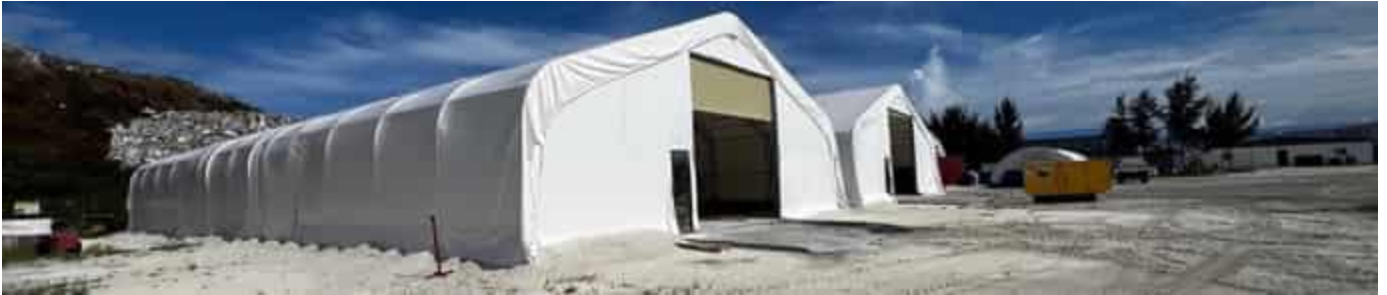
Photo 27 27/03/24 – 2 new storage tents have been completed and being used.
