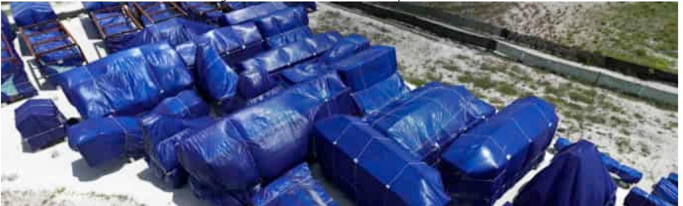
Photo 25 13/06/24 – CNTY delivered the grate parts and are stored on the site laydown area and covered with several sheets of canvas to protect from the elements.
