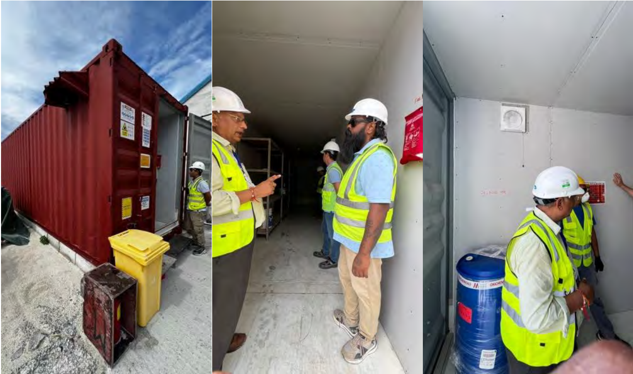
Photo 13 07/05/24 – Inspection of the hazardous chemical store. Requirement of adequate ventilation was highlighted.
