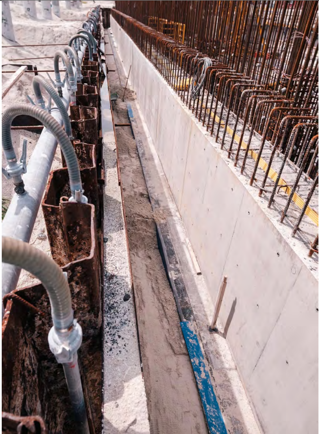
BUNKER - BACKFILLING WORK BEHIND BUNKER WALL IN PROGRESS
