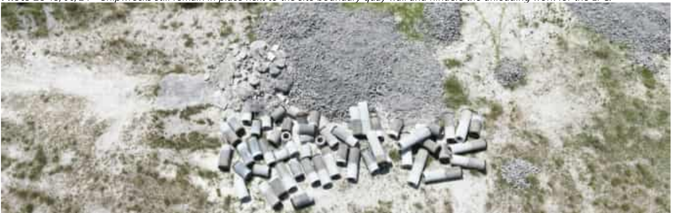
Photo 29 13/06/24 – Waste concrete and waste from piling works are stored on the laydown area.
