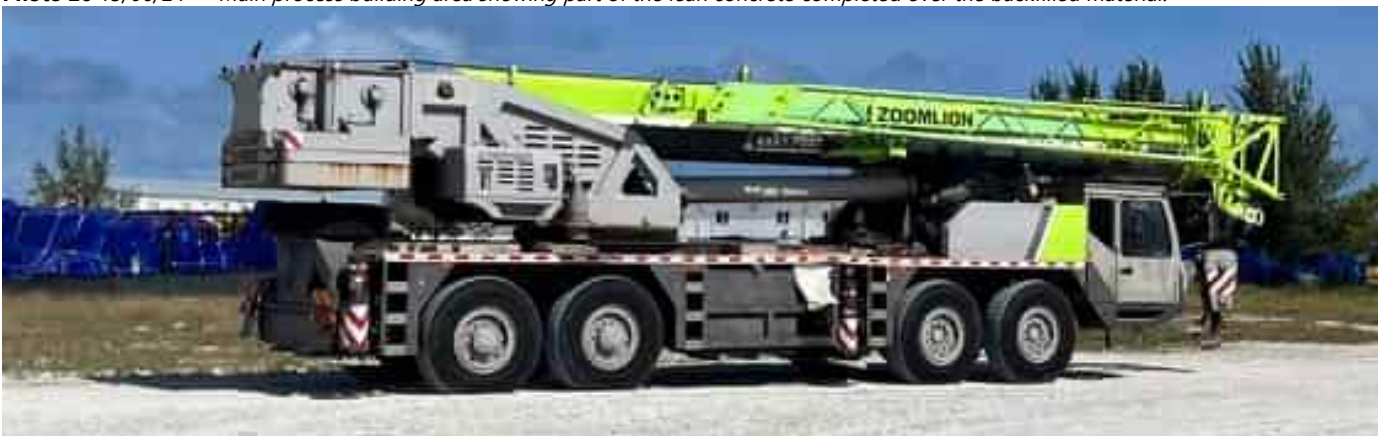
Photo 21 13/06/24 – Several heavy vehicles are being used in the site.
