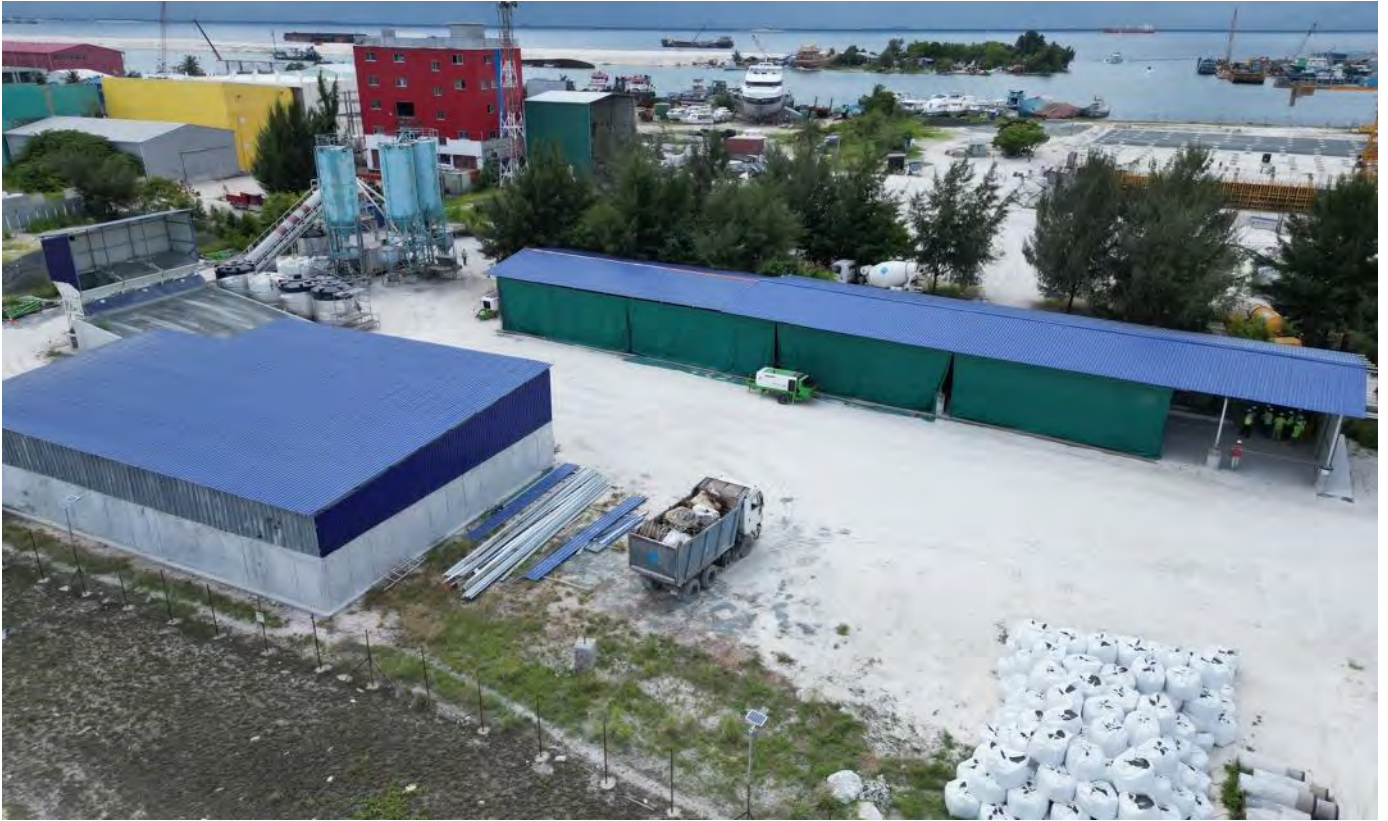
Photo 31 09/05/24 – Batching plant area and material storage area, well kept and maintained.
