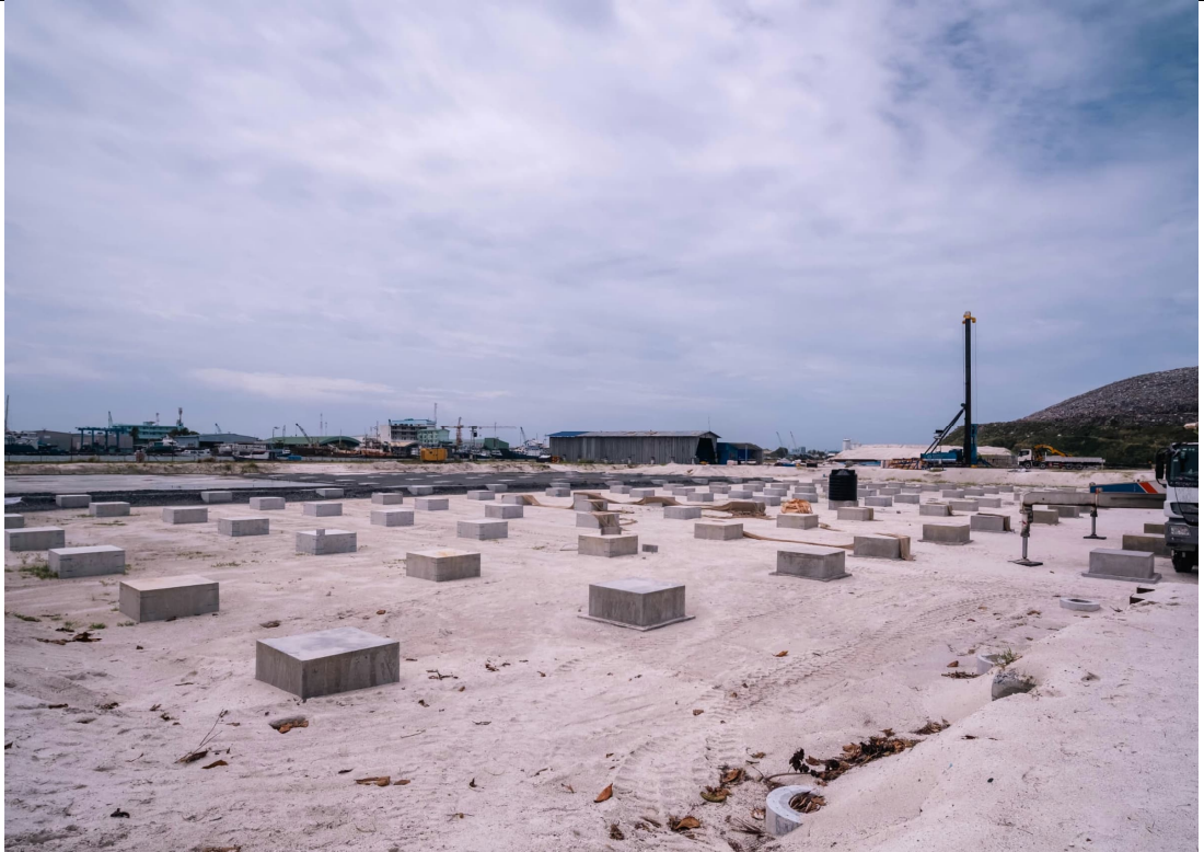
MAIN PROCESS AREA - LEAN CONCRETE AREA 3 COMPLETED
