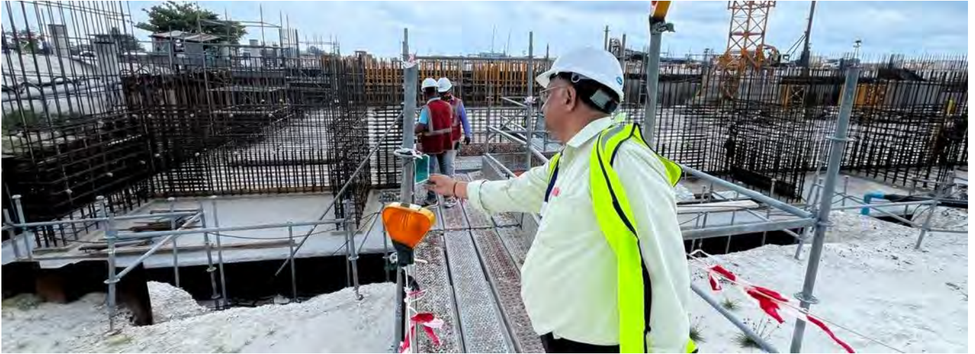
Photo 04 07/05/24 – Mr. Sunil inspecting the scaffolding at the bunker construction area.
