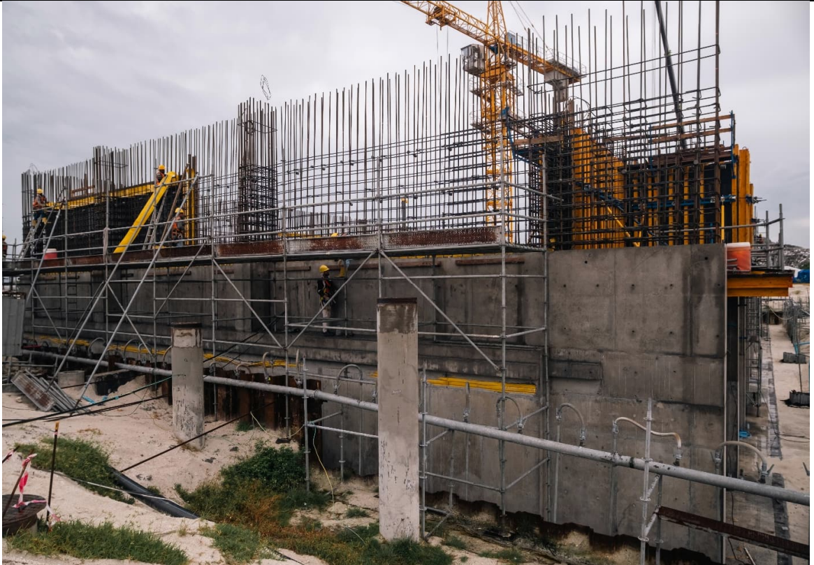
BUNKER AREA - OVERALL BUNKER WALL 3 rd LAYER COMPLETED 70%
