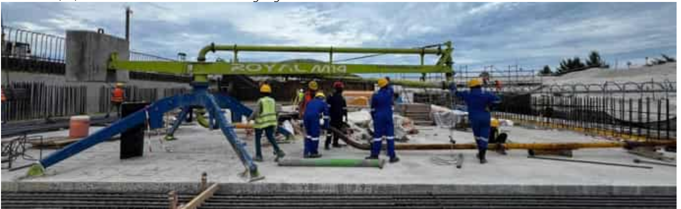
Photo 35 16/04/24 – Concrete pump boom placed in the bunker area.
