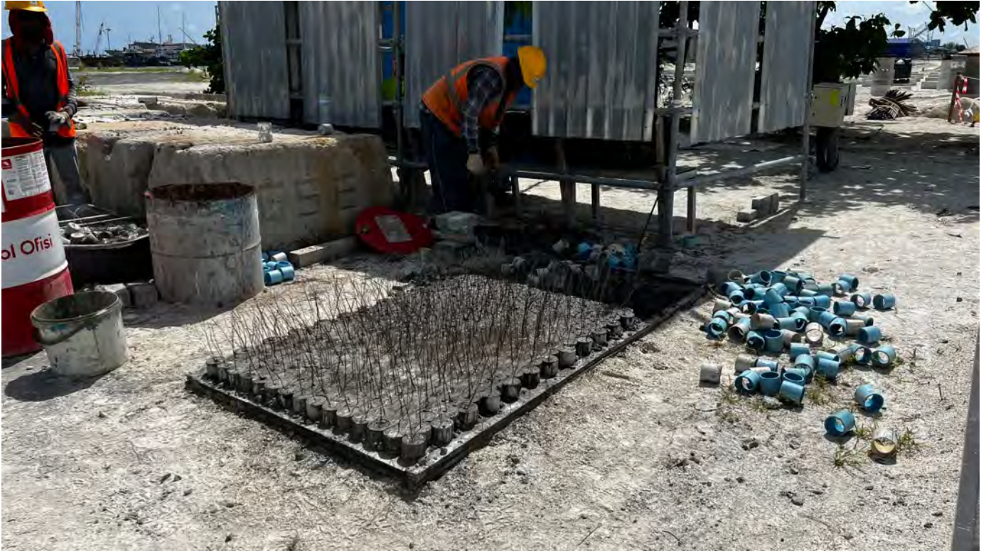
Photo 12 02/05/24 – Concrete cover blocks being made.
