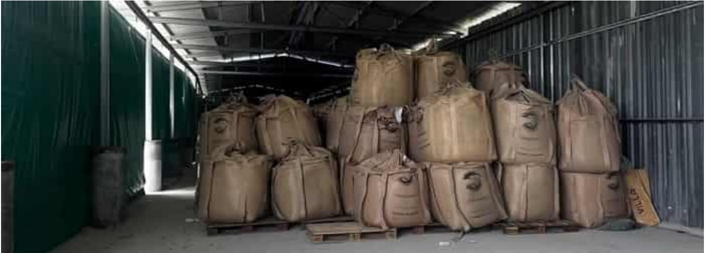
Photo 09 14/04/24 – Cement storage area for the concrete batching plant.
