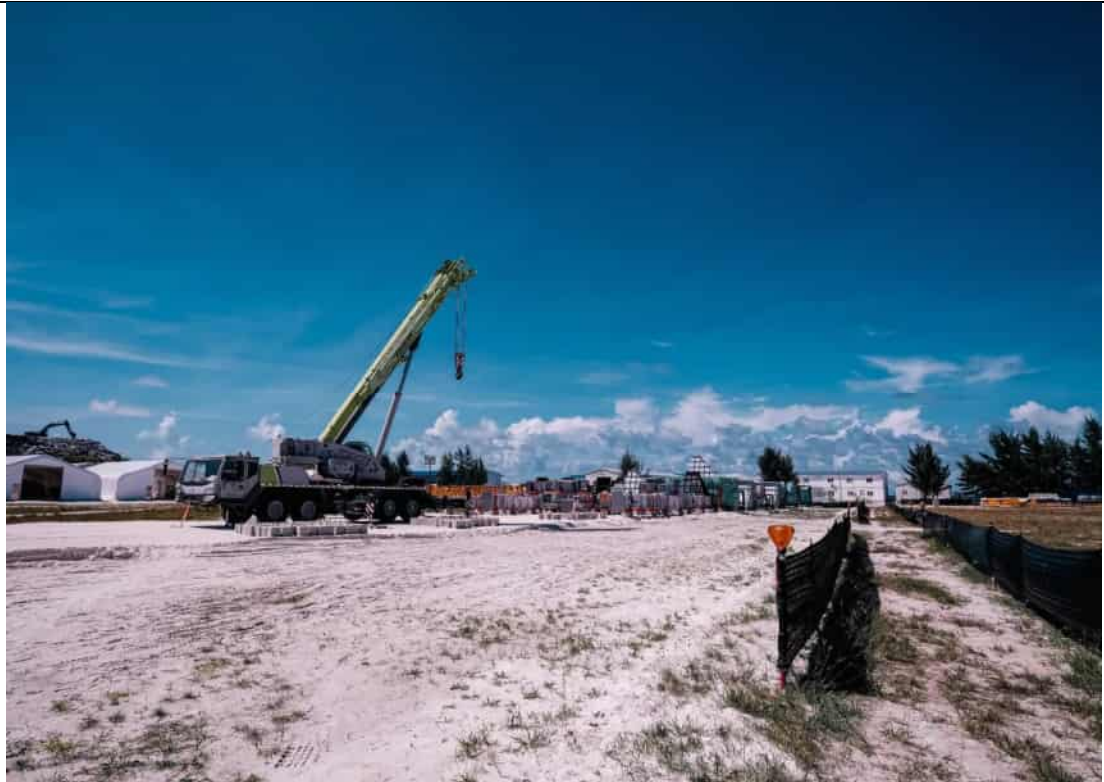
FIRST SHIPMENT - INCINERATOR & INCINERATOR STEEL STRUCTURE ON SITE
