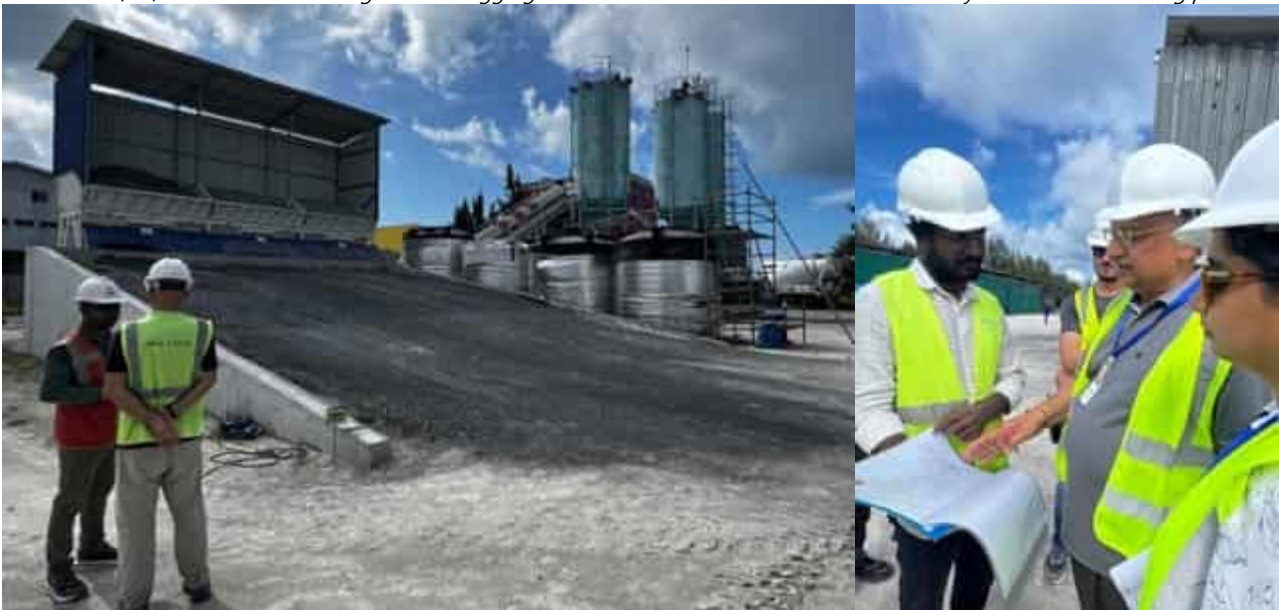
Photo 11 14/04/24 – Mr.Sunil checking with Villa staff operating the batching plant on the SOP's, logs, MSDS etc.
