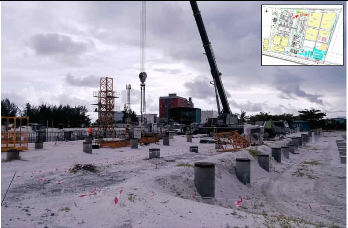
OVERALL - POINT THREE
