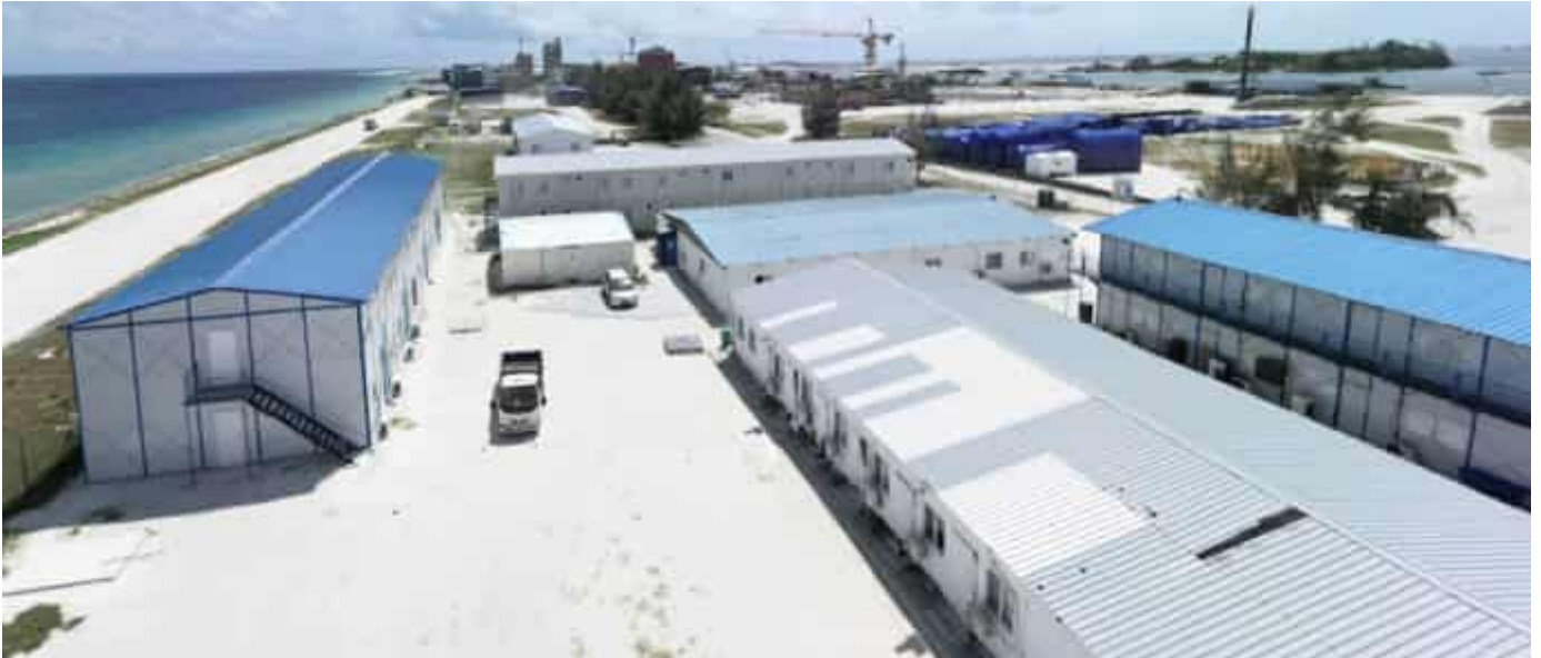
Photo 36 13/06/24 – Construction camp is kept clean and well maintained.
