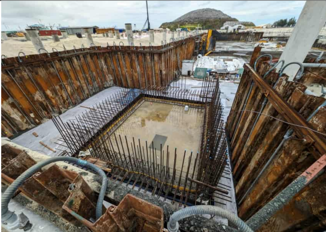
BUNKER - LEACHATE AREA STRUCTURAL BACKFILLING COMPLETED
