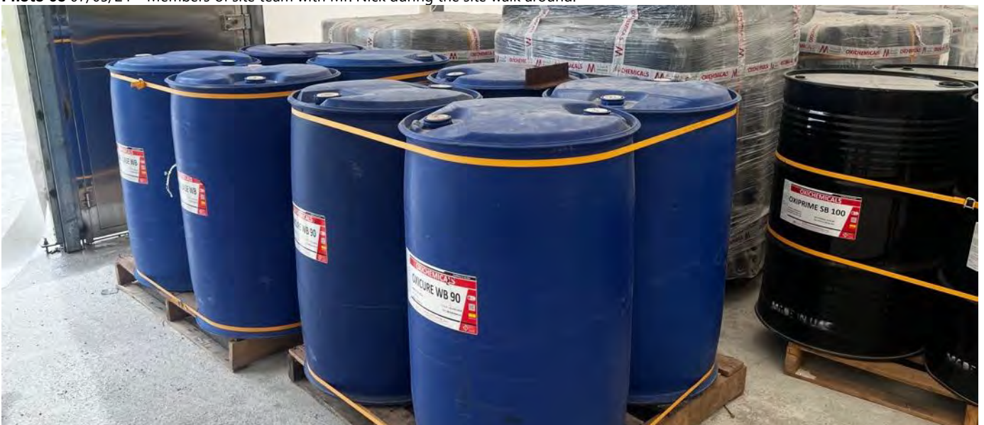
Photo 09 07/05/24 – Construction chemicals in the storage area, requires adequate measures to ensure safety, and spillage containment.
