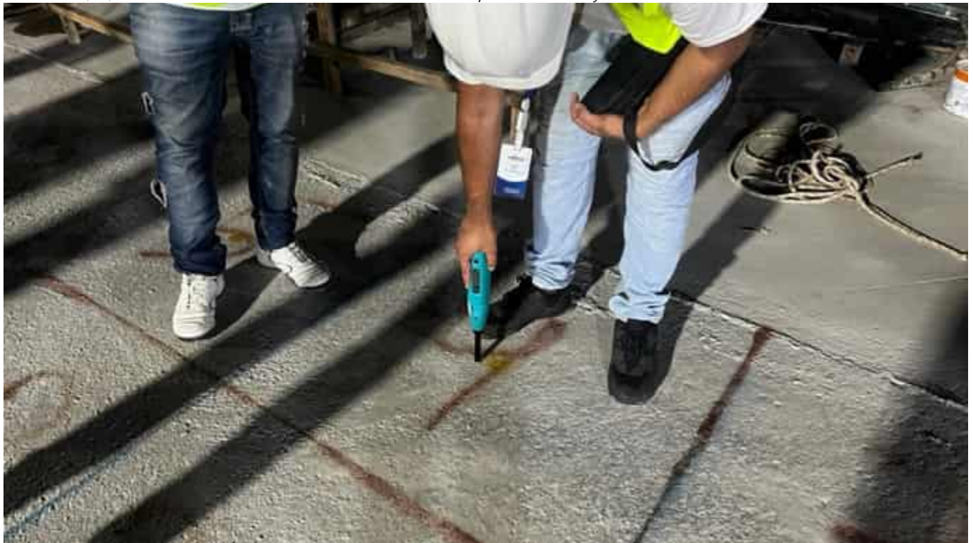
Photo 02 08/04/24 – Rebound hammer test being done on the Bunker slab in Area 1, by third party inspector Falcon Laboratories.
