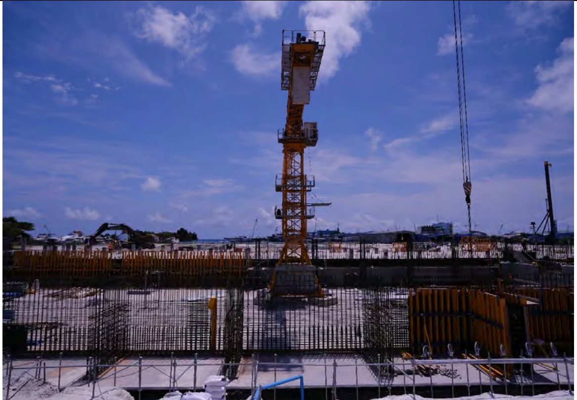
BUNKER AREA - WALL A & WALL C COMPLETED
