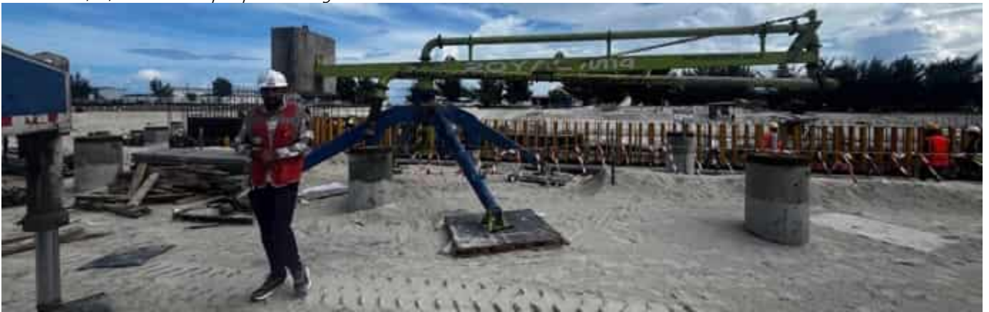
Photo 22 27/03/24 – Concrete pump truck being utilized on site.
