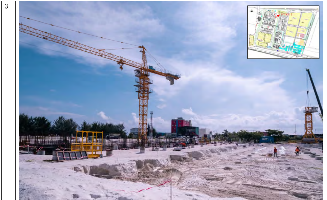
OVERALL - POINT THREE
