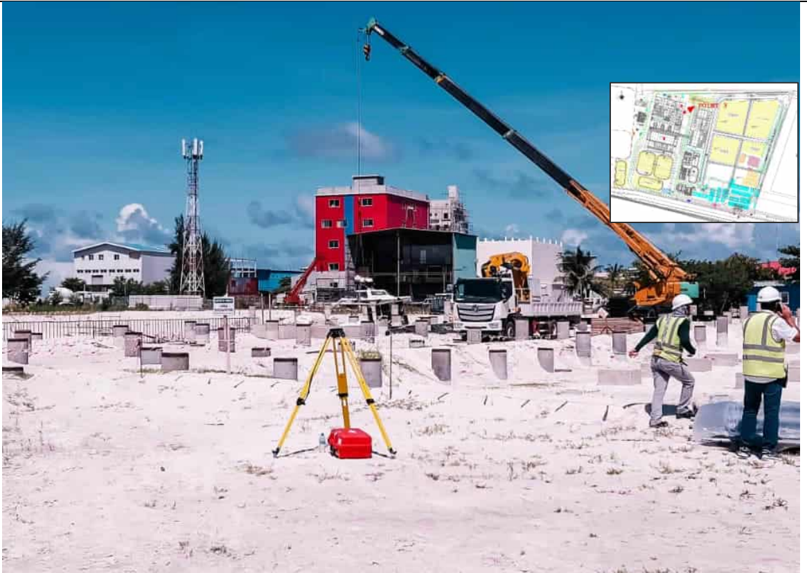
OVERALL - POINT THREE
