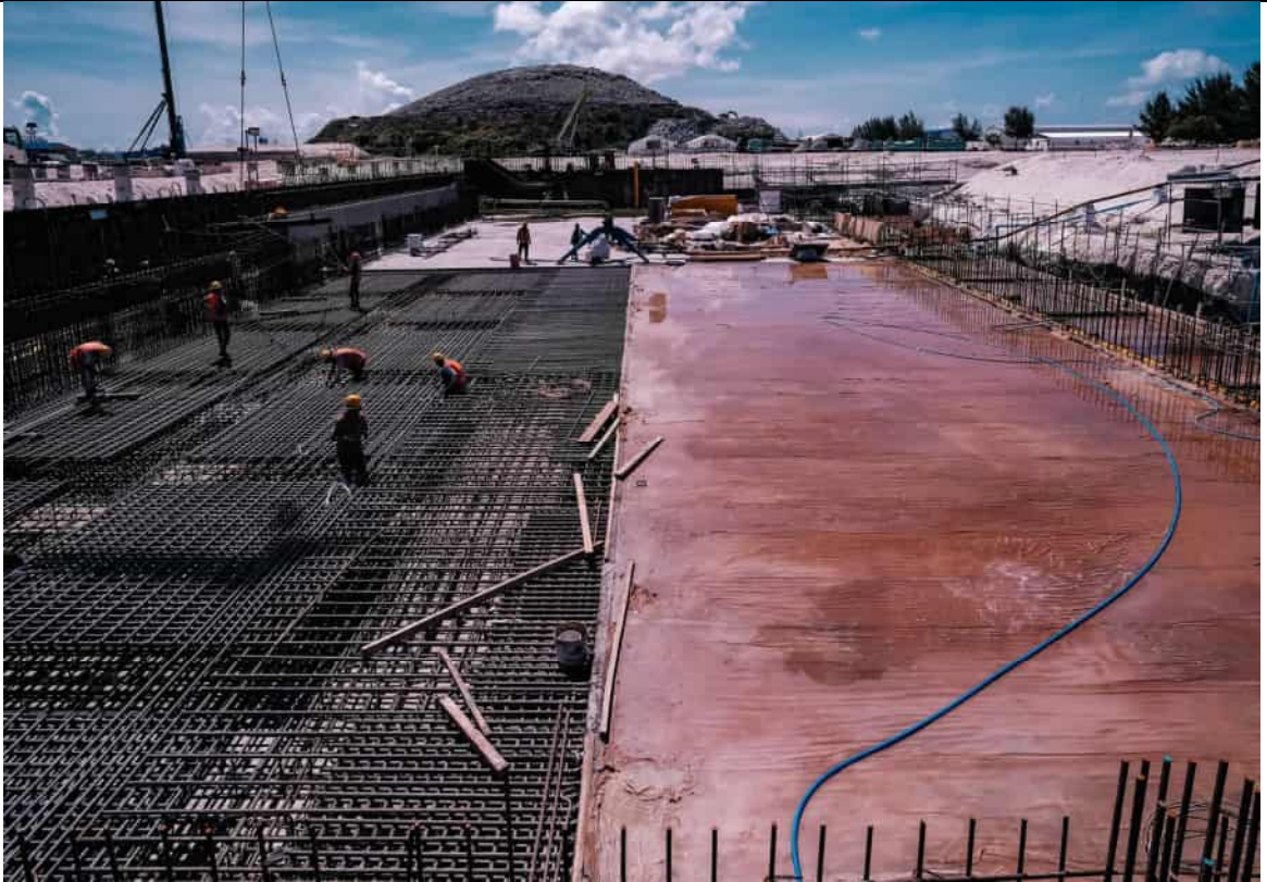
BUNKER AREA - AREA 2 CONCRETING COMPLETED.
