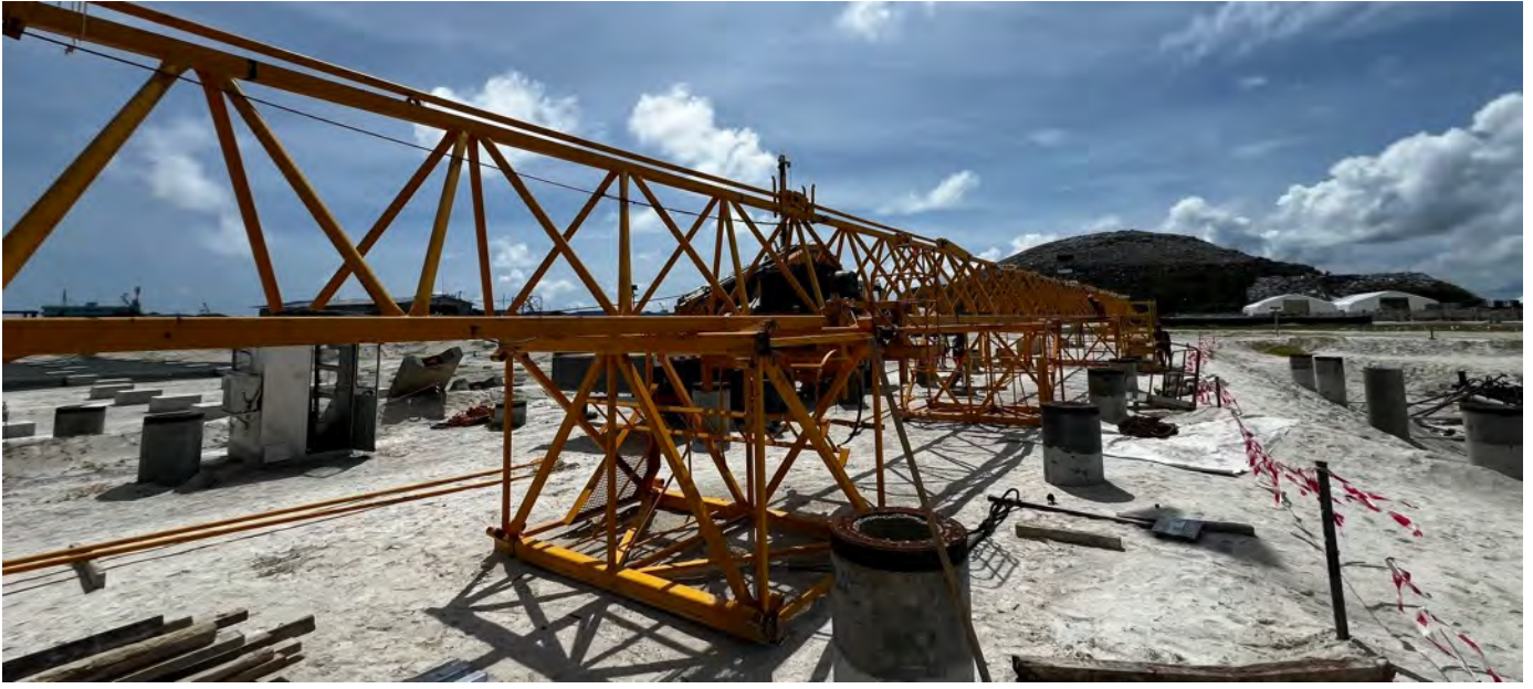
Photo 14 02/05/24 – Tower crane assembly work is ongoing.
