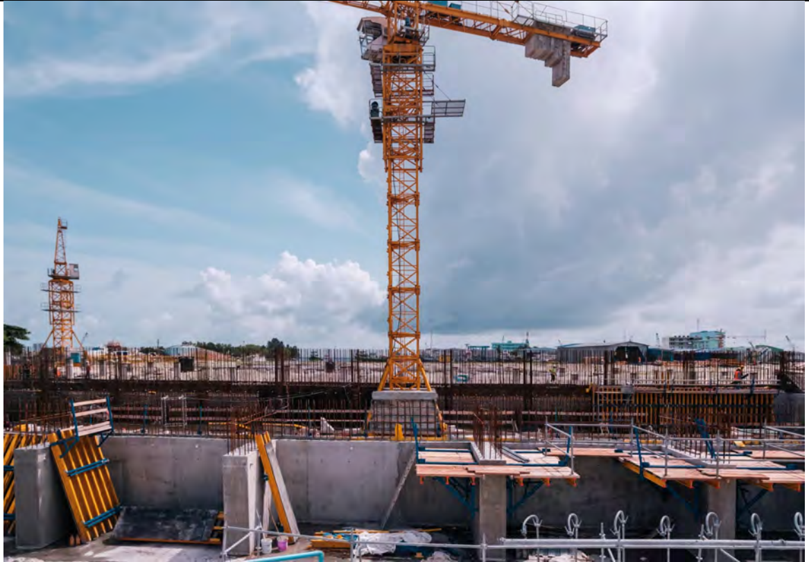
BUNKER AREA - WALL F, E, I & J COMPLETED (+0 LEVEL)
