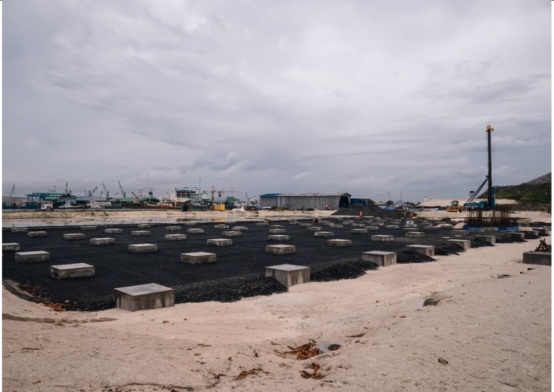
MAIN PROCESS AREA - STRUCTURAL BACKFILLING IN PROGRESS
