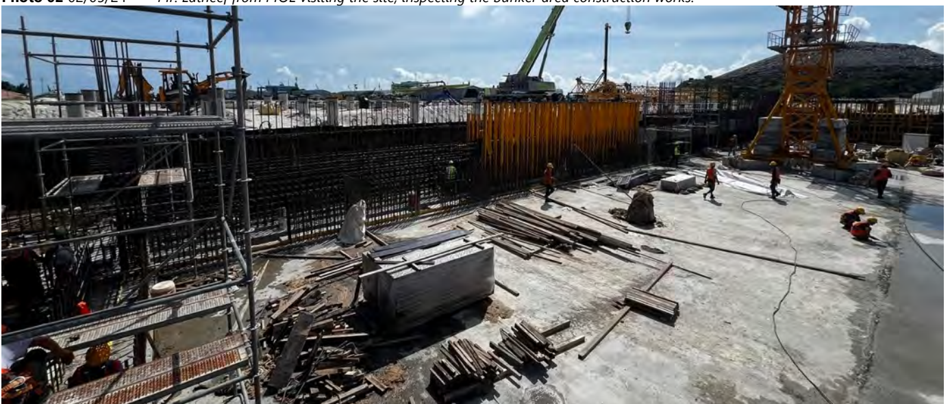
Photo 03 02/05/24 – Bunker wall reinforcement and formwork installation work is ongoing.
