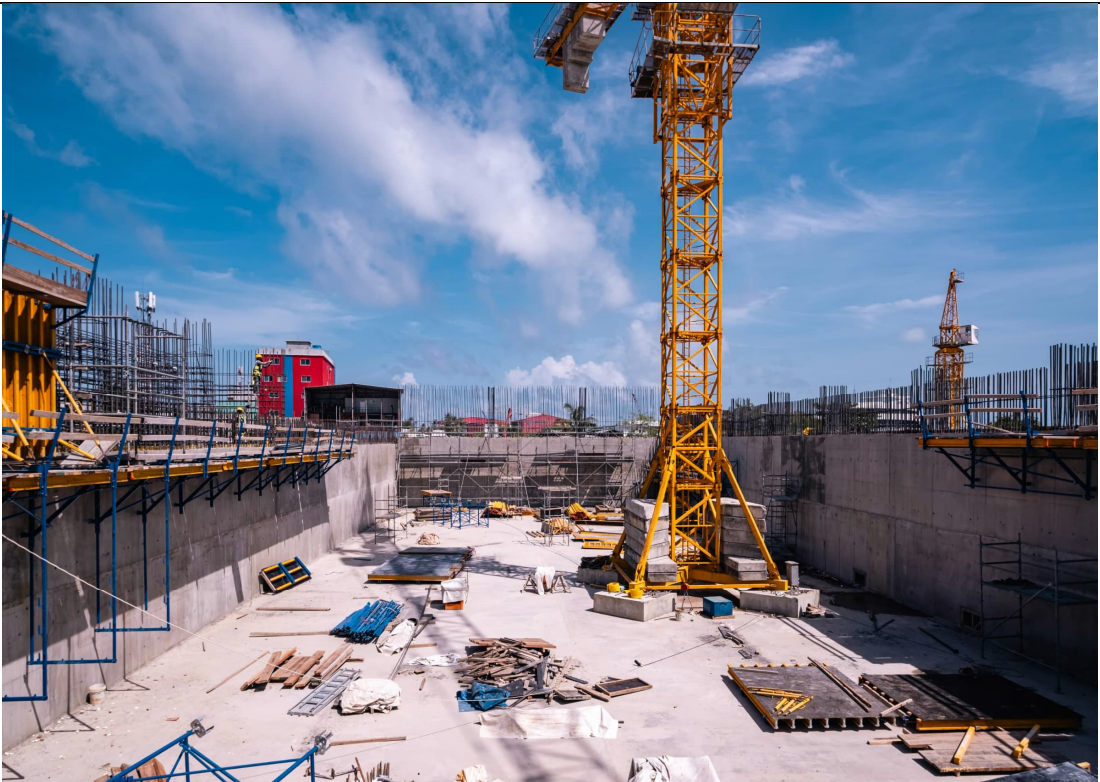
BUNKER AREA - OVERALL BUNKER 1 ST LAYER COMPLETED 100%
