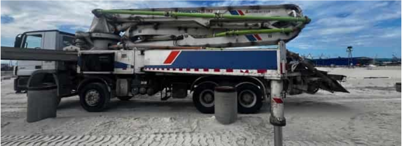
Photo 21 27/03/24 – Concrete pump truck being utilized on site.
