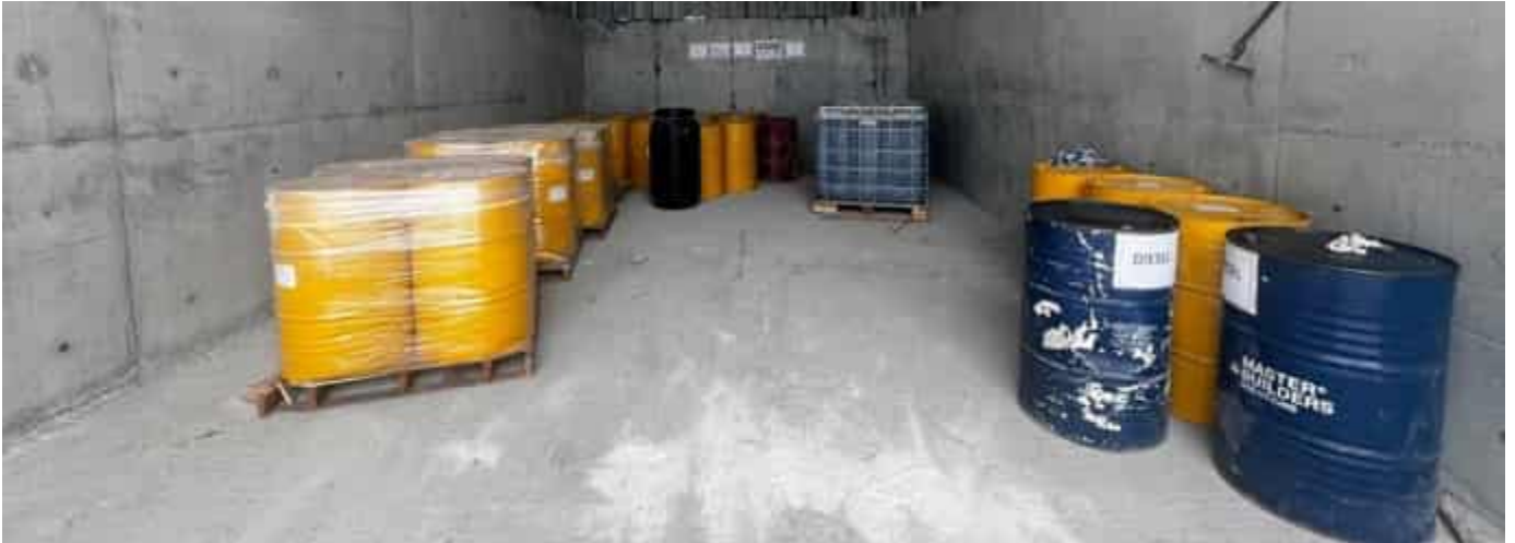
Photo 08 04/04/24 – Chemical admixtures storage area for the concrete batching plant.
