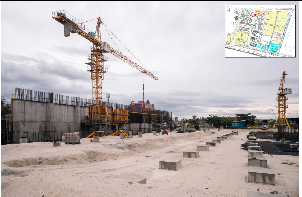
OVERALL - POINT THREE
