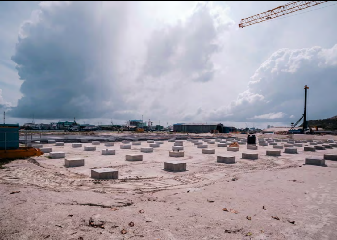
MAIN PROCESS AREA - CONCRETE CASTING FOR PILECAPS IN PROGRESS
