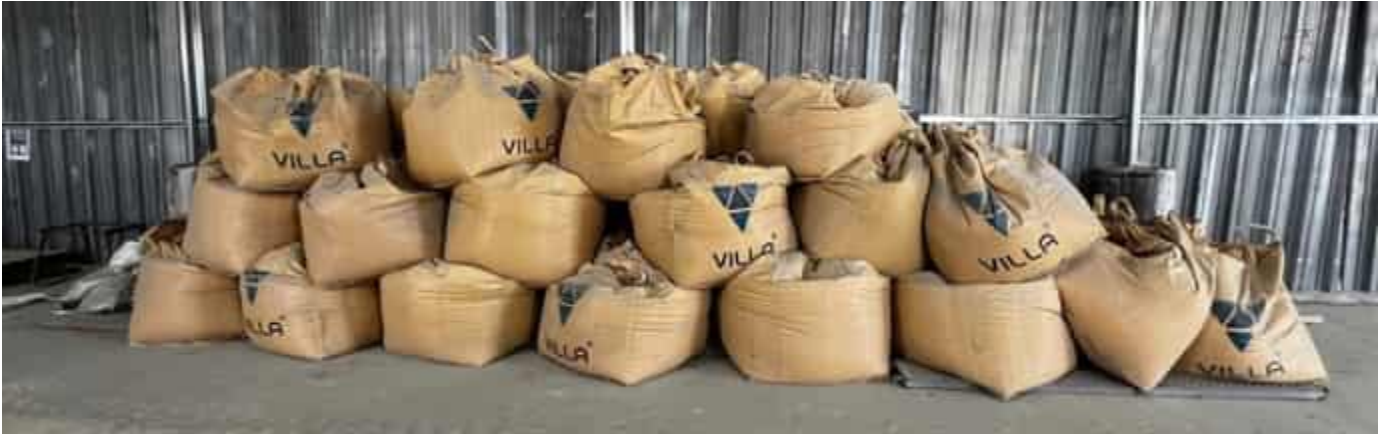
Photo 11 04/04/24 – Cement storage area for the concrete batching plant.
