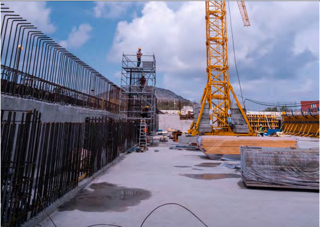
BUNKER AREA - WALL J, C & H IN PROGRESS
