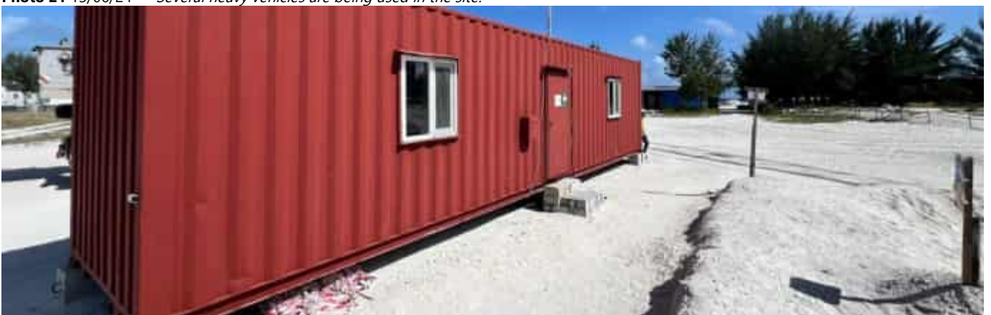
Photo 22 13/06/24 – Construction site office established near the construction area.
