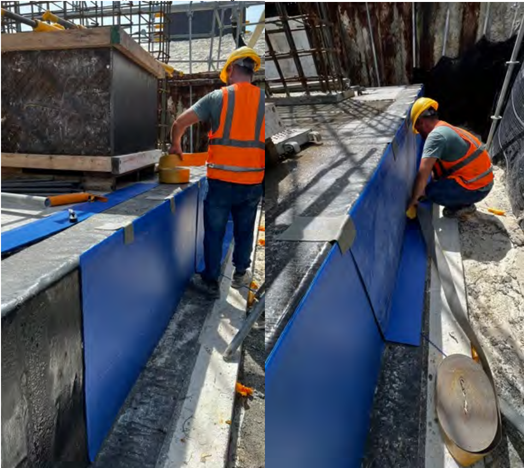
Photo 09 02/05/24 – Waterproofing membrane being installed on the bunker slab edge.
