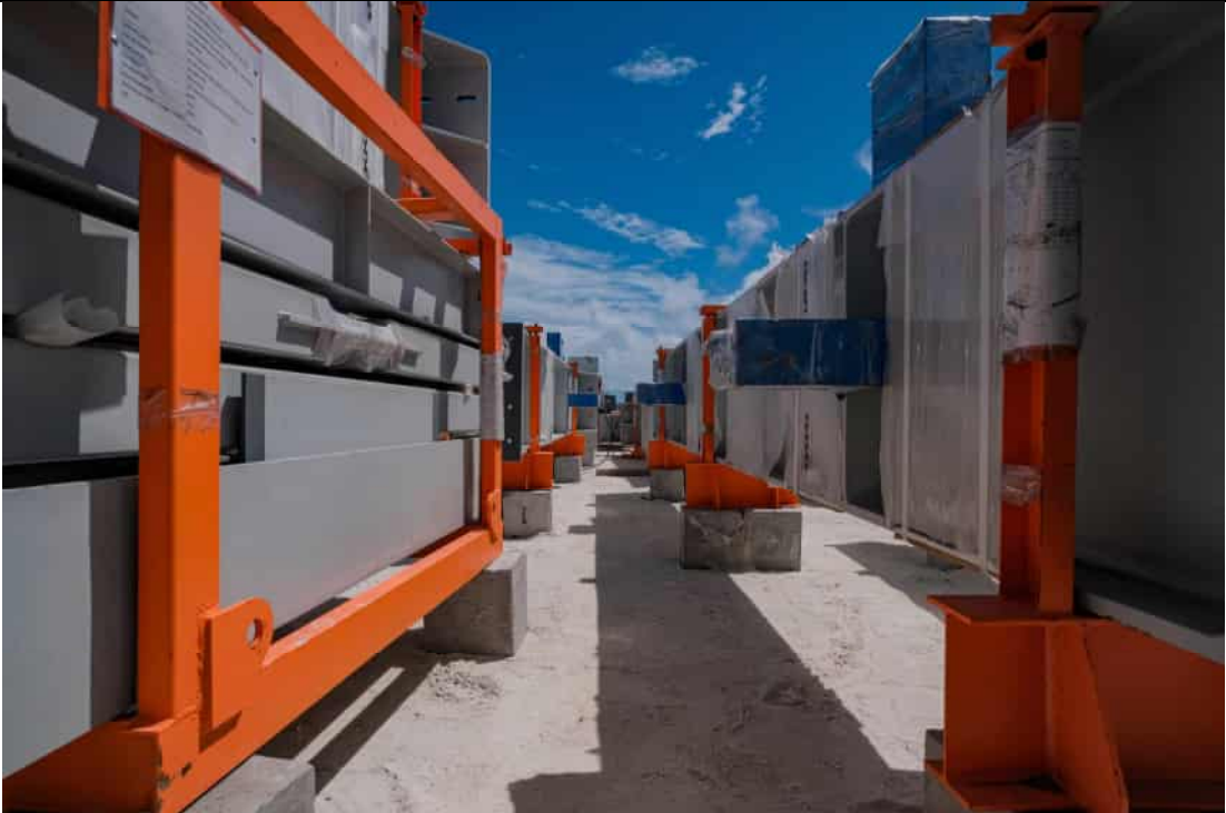
FIRST SHIPMENT - INCINERATOR STEEL STRUCTURE
