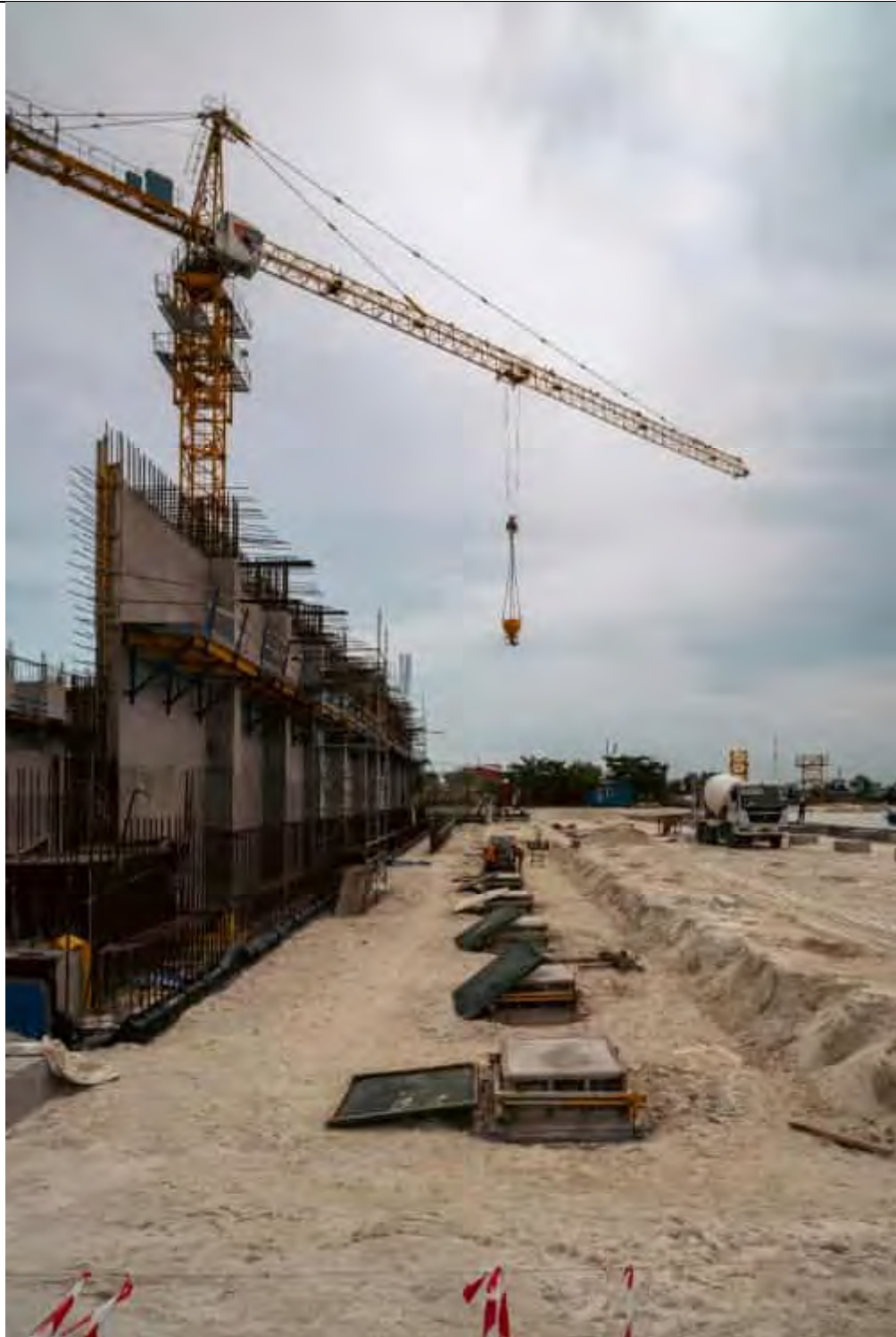
INCINERATOR AREA - 12 PILECAPS CONCRETED.
