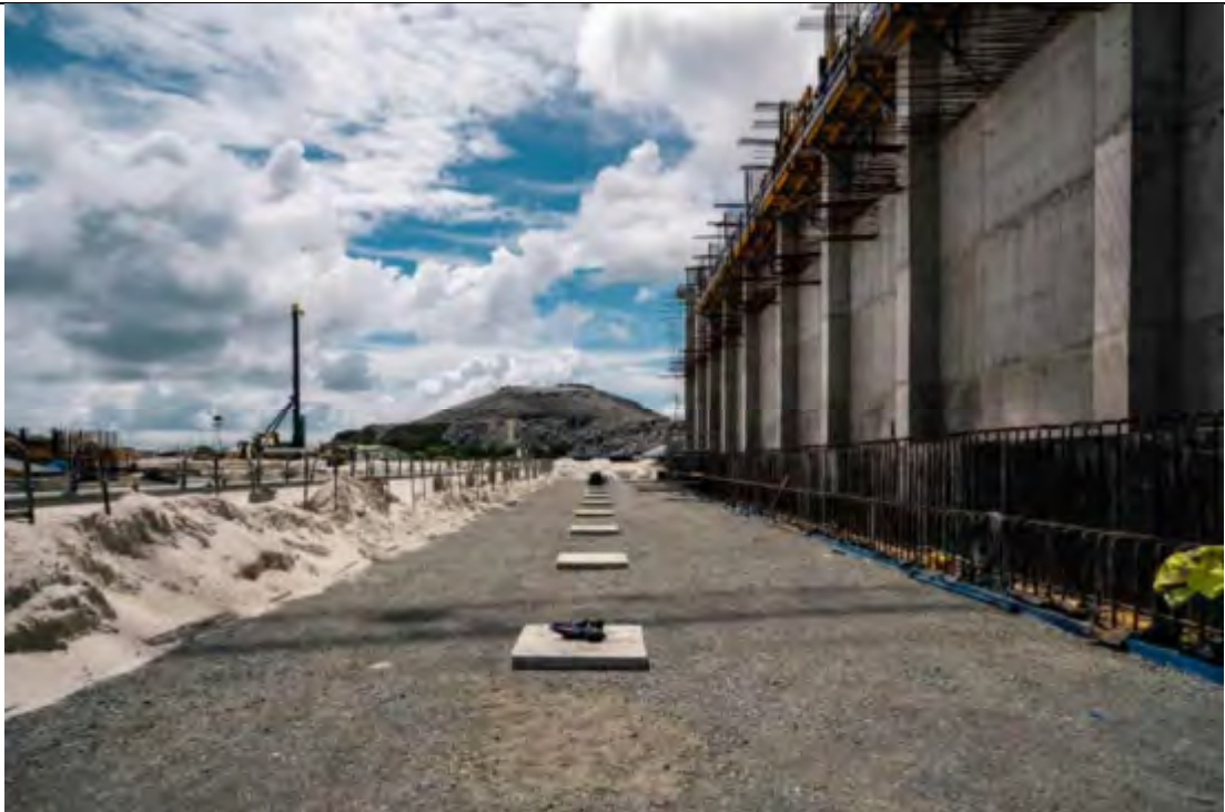
INCINERATOR AREA - STRUCTURAL BACKFILLING IN PROGRESS
