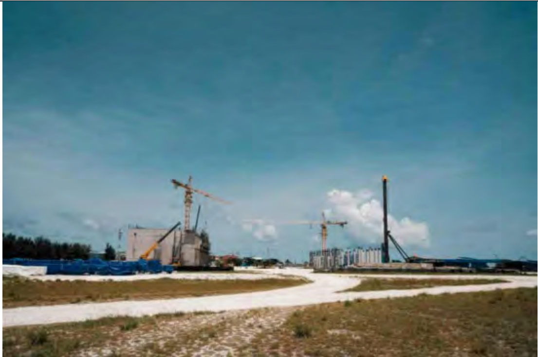
OVERALL VIEW FROM EAST SIDE
