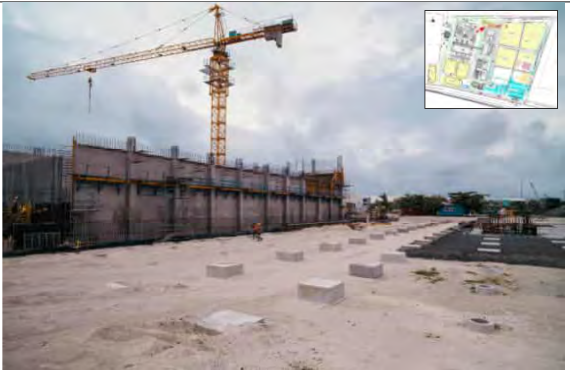
OVERALL - POINT THREE
