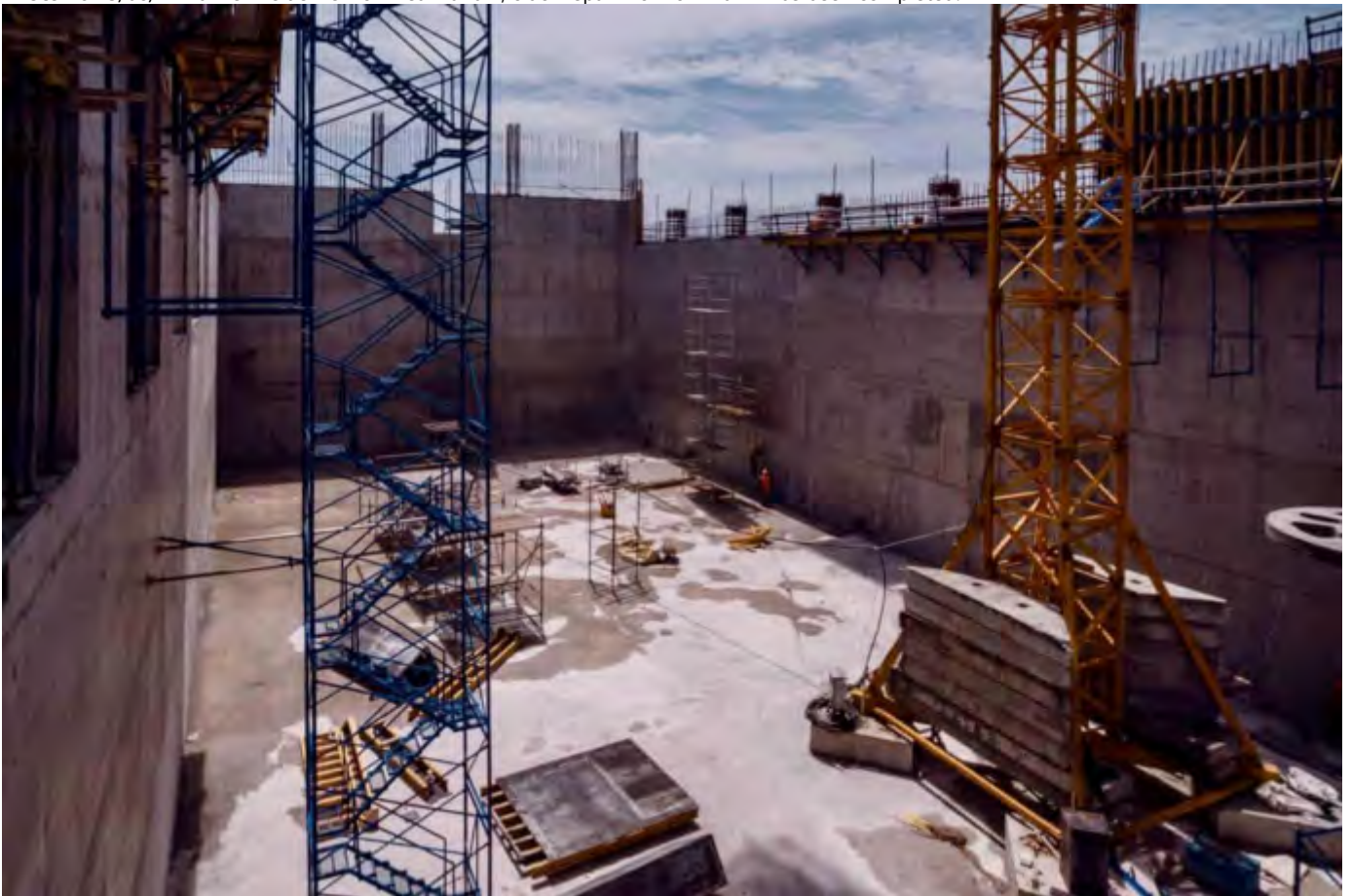
Photo 11 13/08/24 – Bunker inside view of Area 2 and 3.
