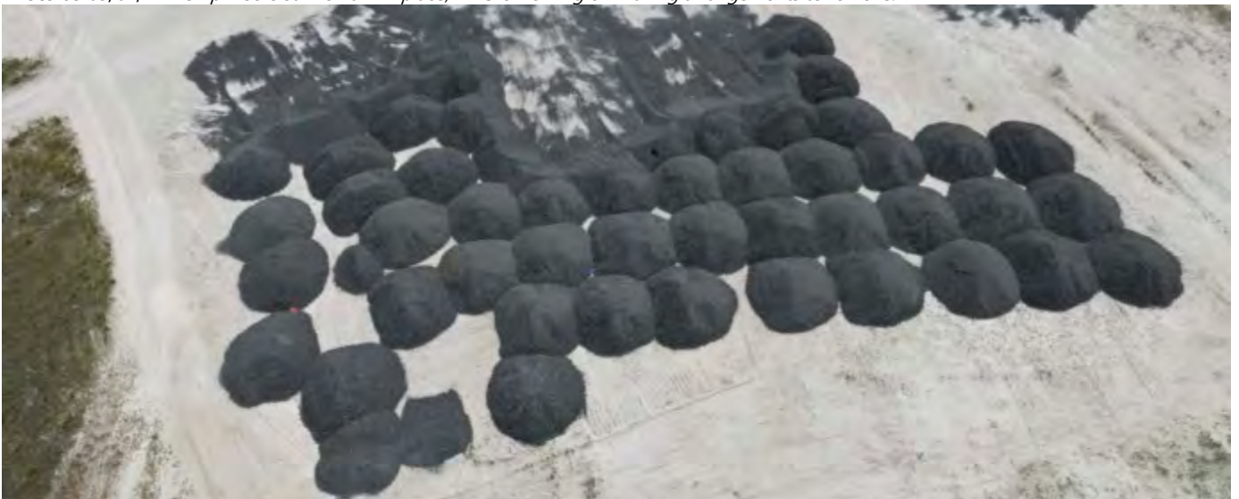
Photo 10 09/07/24– Backfilling material delivered to site and stockpiled in the laydown area.
