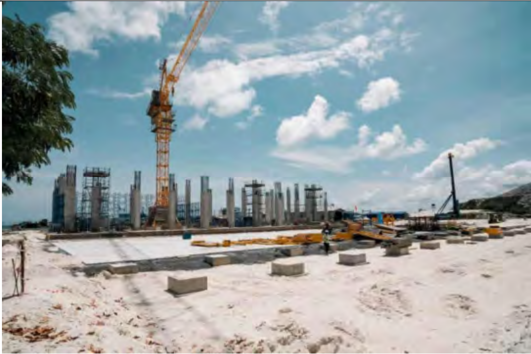
COLUMNS ADJACENT TO APC AREA IN PROGRESS.
