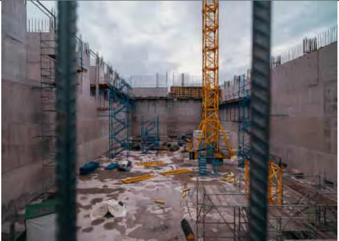
BUNKER (INSIDE) VIEW.
