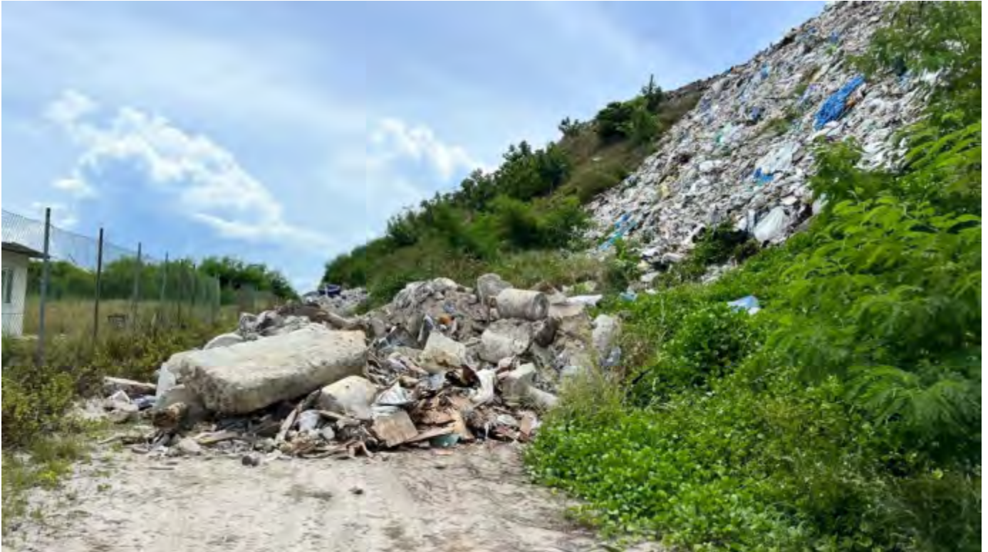
Photo 11 25/07/24 – C&D waste placed by WAMCO in the landfill area next to the site boundary fence.
