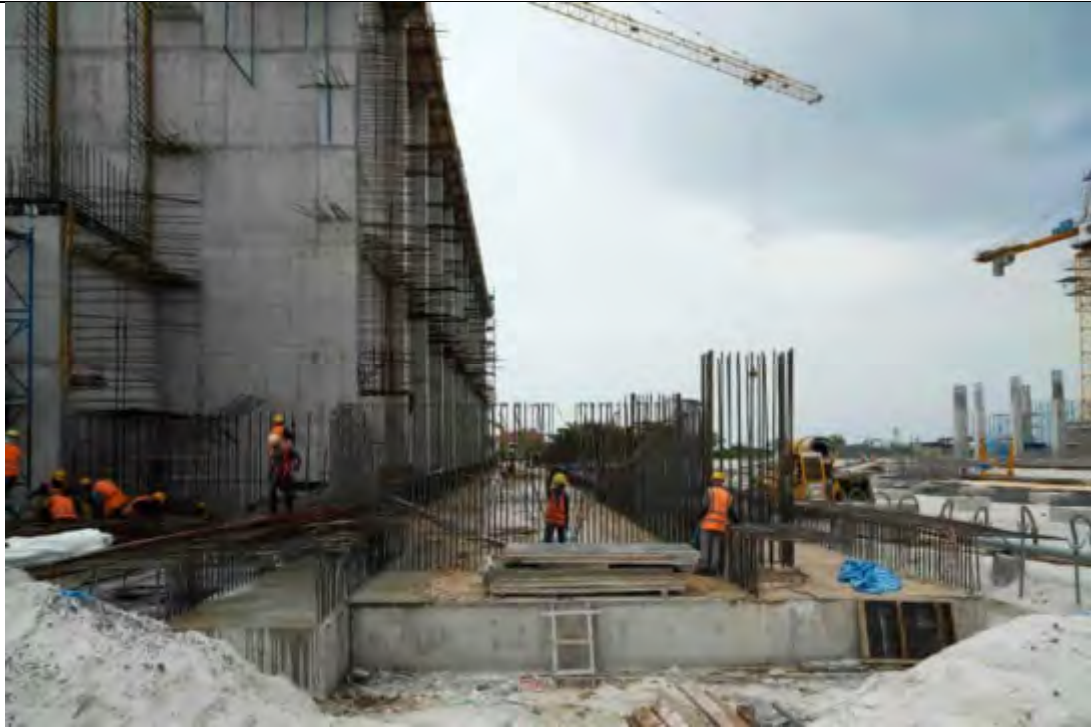
INCINERATOR AREA - AREA 12 FOUNDATION COMPLETED
