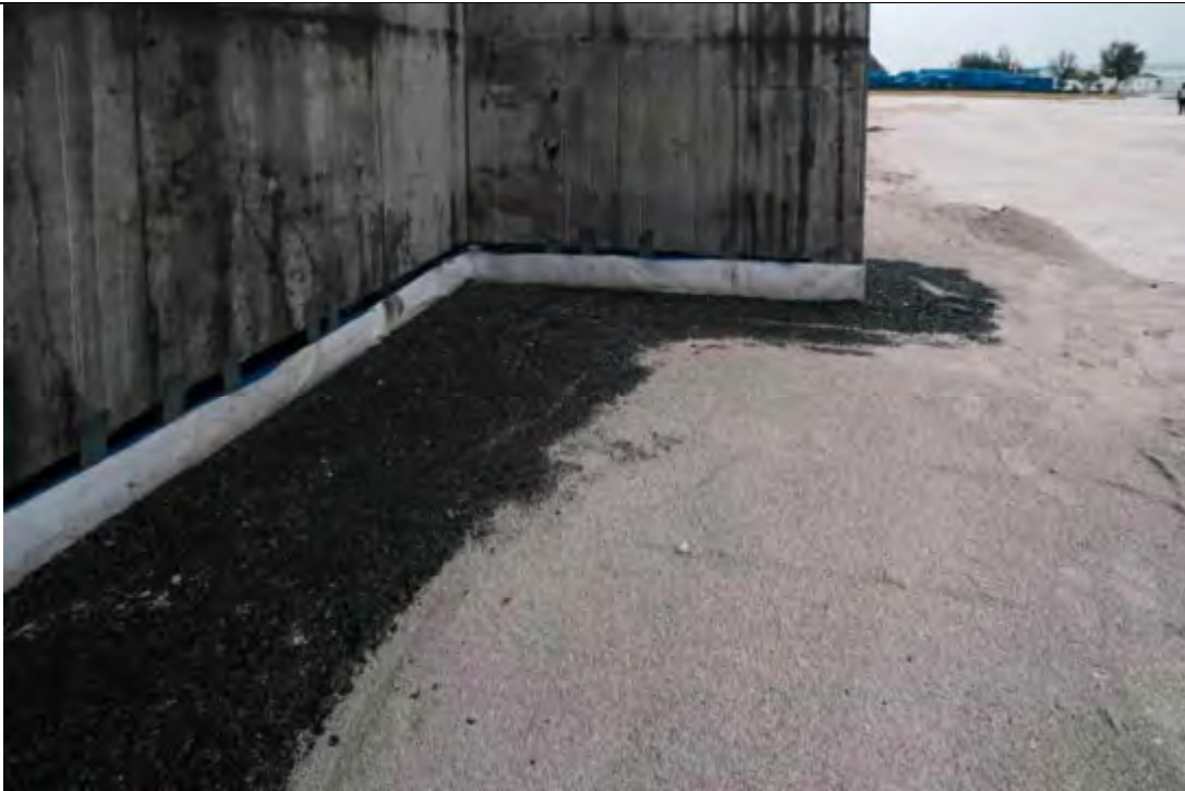
BUNKER SOUTH SIDE BACKFILLING REMEDIAL COMPLETED.
