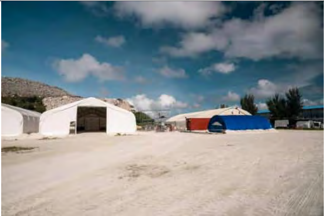
CONSTRUCTION OF DEDICATED HAZARDOUS STORAGE AREA.
