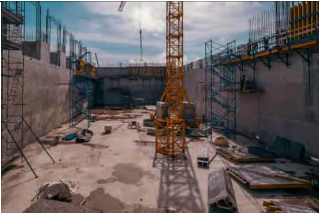
BUNKER - VIEW FROM INSIDE (EAST)
