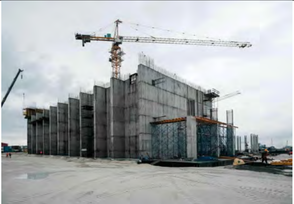
BUNKER AREA - OVERALL BUNKER WALL 7 th LAYER 90% COMPLETED.
