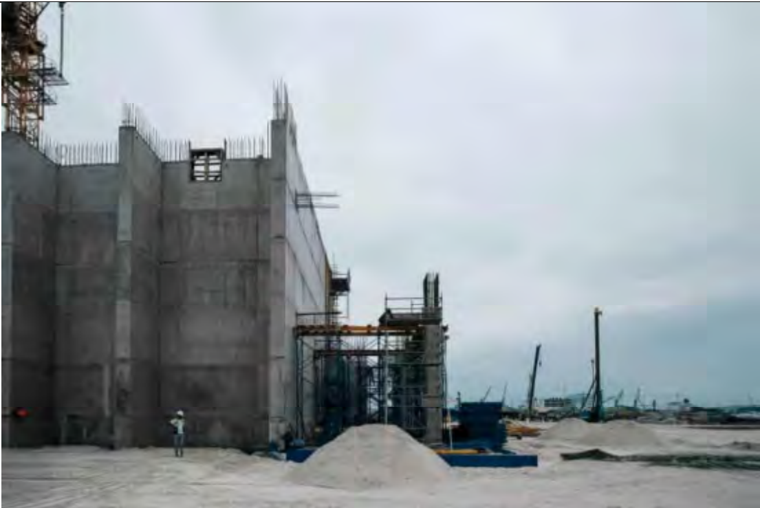
BUNKER EAST SIDE - ELEVATOR SHAFT AND COLUMN UP TO +7.8M
