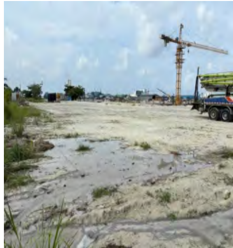
Discharge of Waste water from sedimentation tank in batching plant to adjacent land owned by third party observed during site visit in July month for inspection
