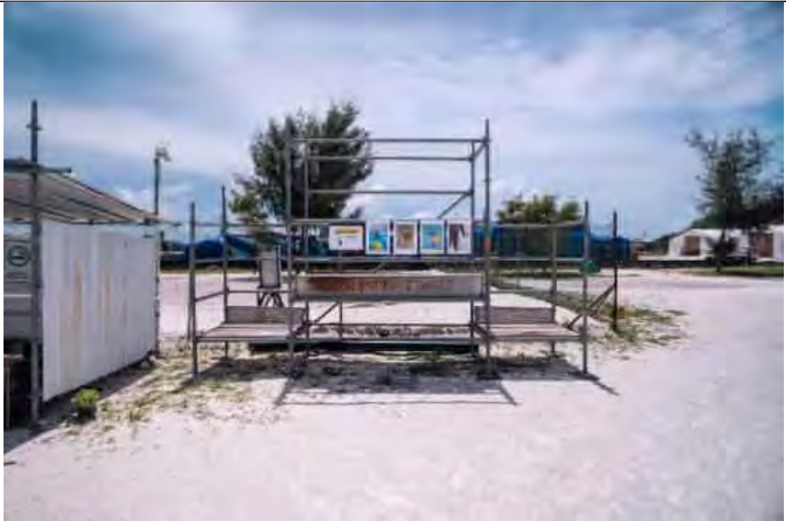
MOCK-UP WORKING PLATFORM INSTALLED AS REFERENCE AND FREQUENT TRAINING DURING TOOLBOX MEETING
