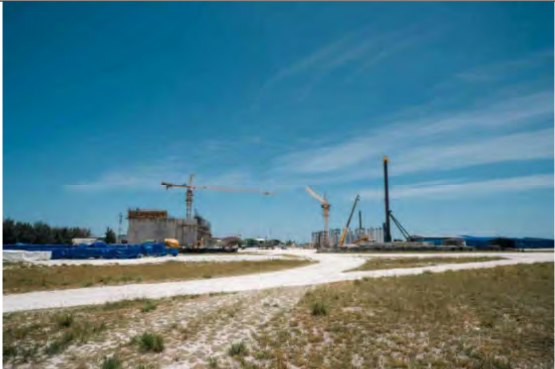
OVERALL VIEW FROM EAST SIDE
