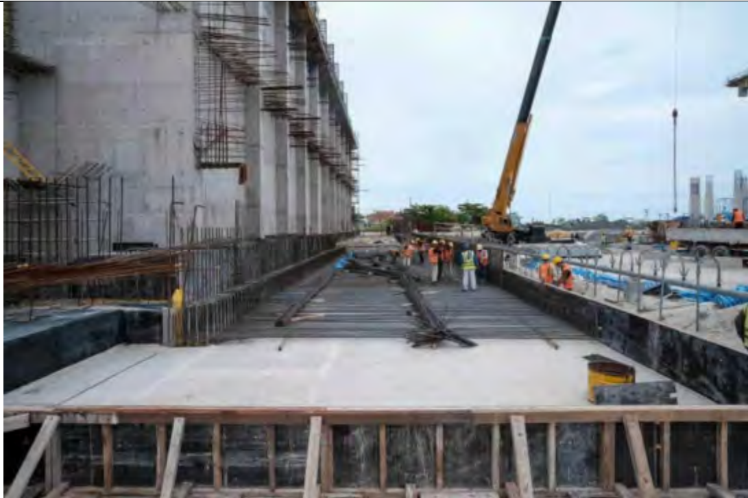
INCINERATOR AREA - AREA 12 REINFORCEMENT BAR AND FORMWORK IN PROGRESS
