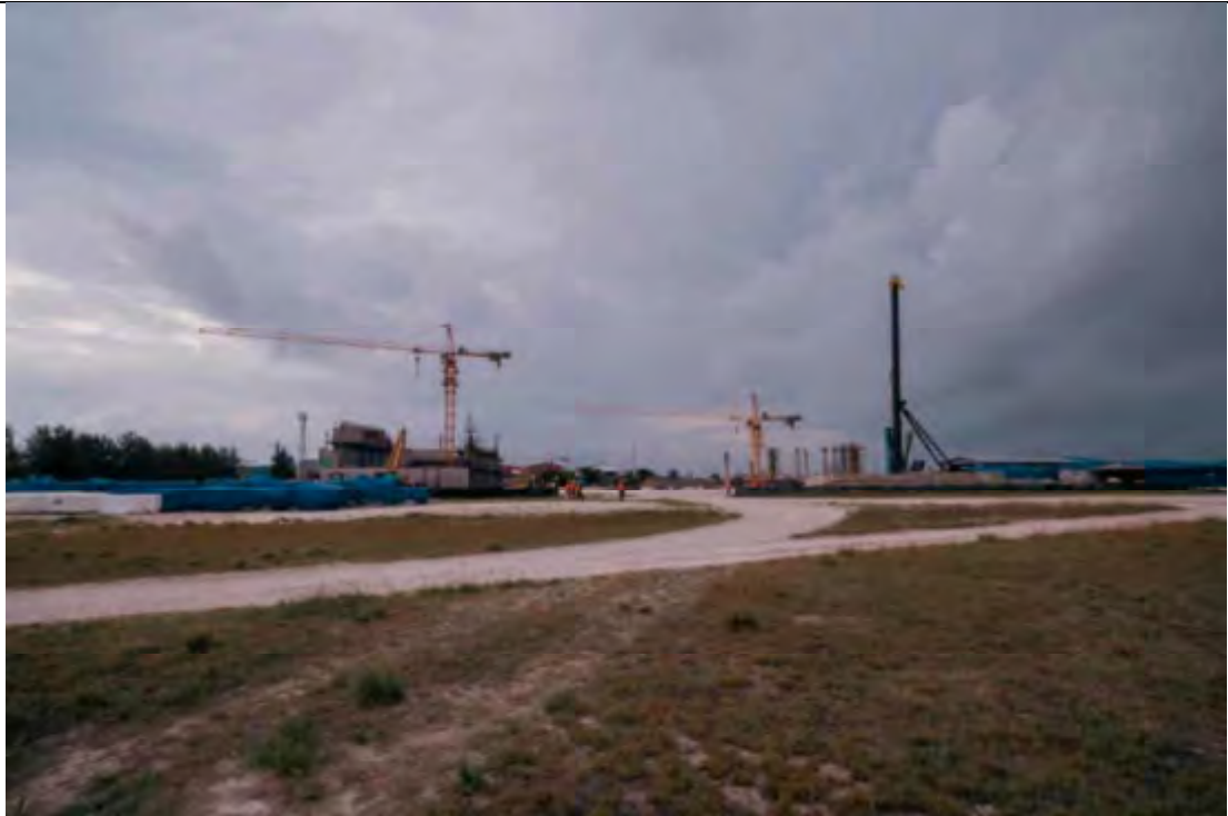
OVERALL VIEW FROM EAST SIDE
