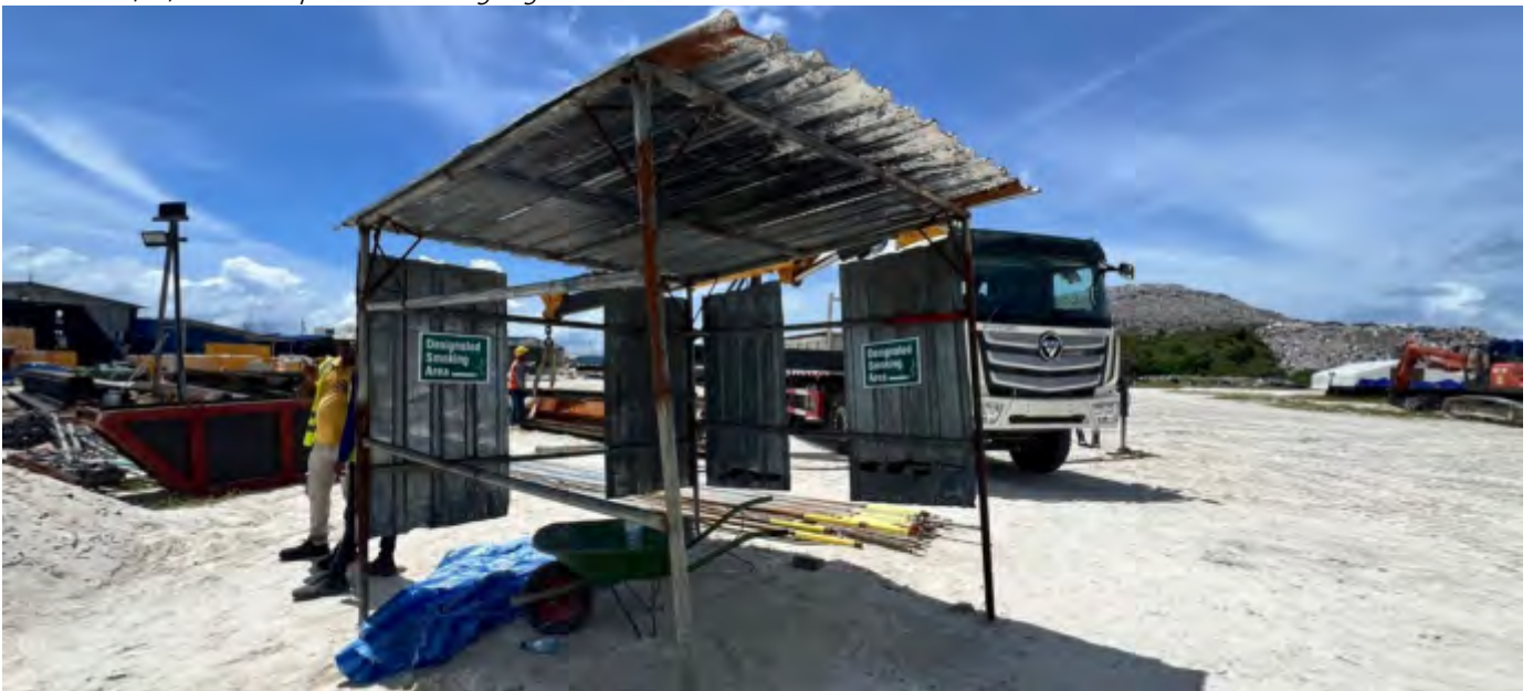
Photo 06 18/07/24 – Resting shack/smoking area has been setup close to the work area.
