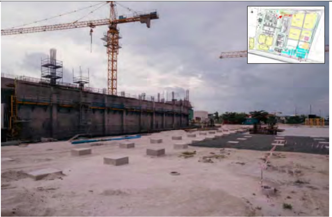
OVERALL - POINT THREE
