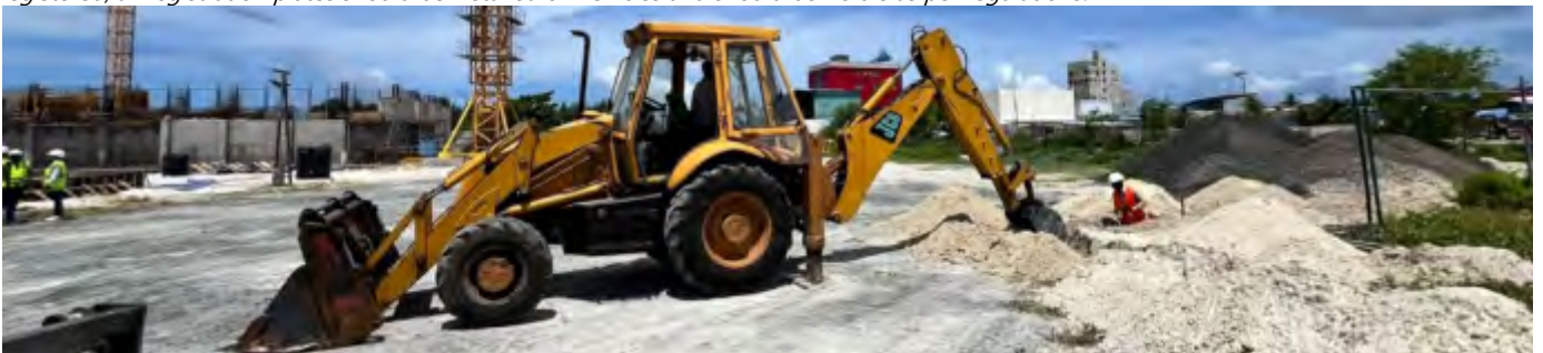
Photo 10 18/07/24– Excavation work is ongoing for temporary cable laying.
