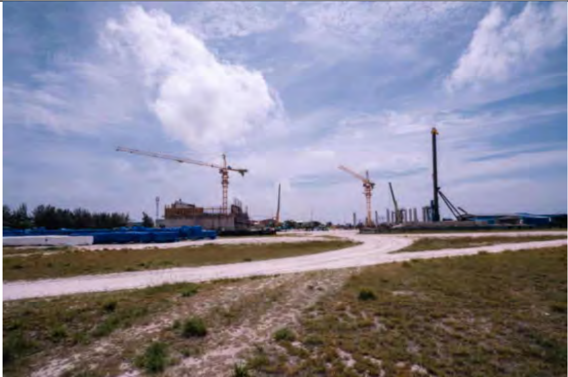
OVERALL VIEW FROM EAST SIDE
