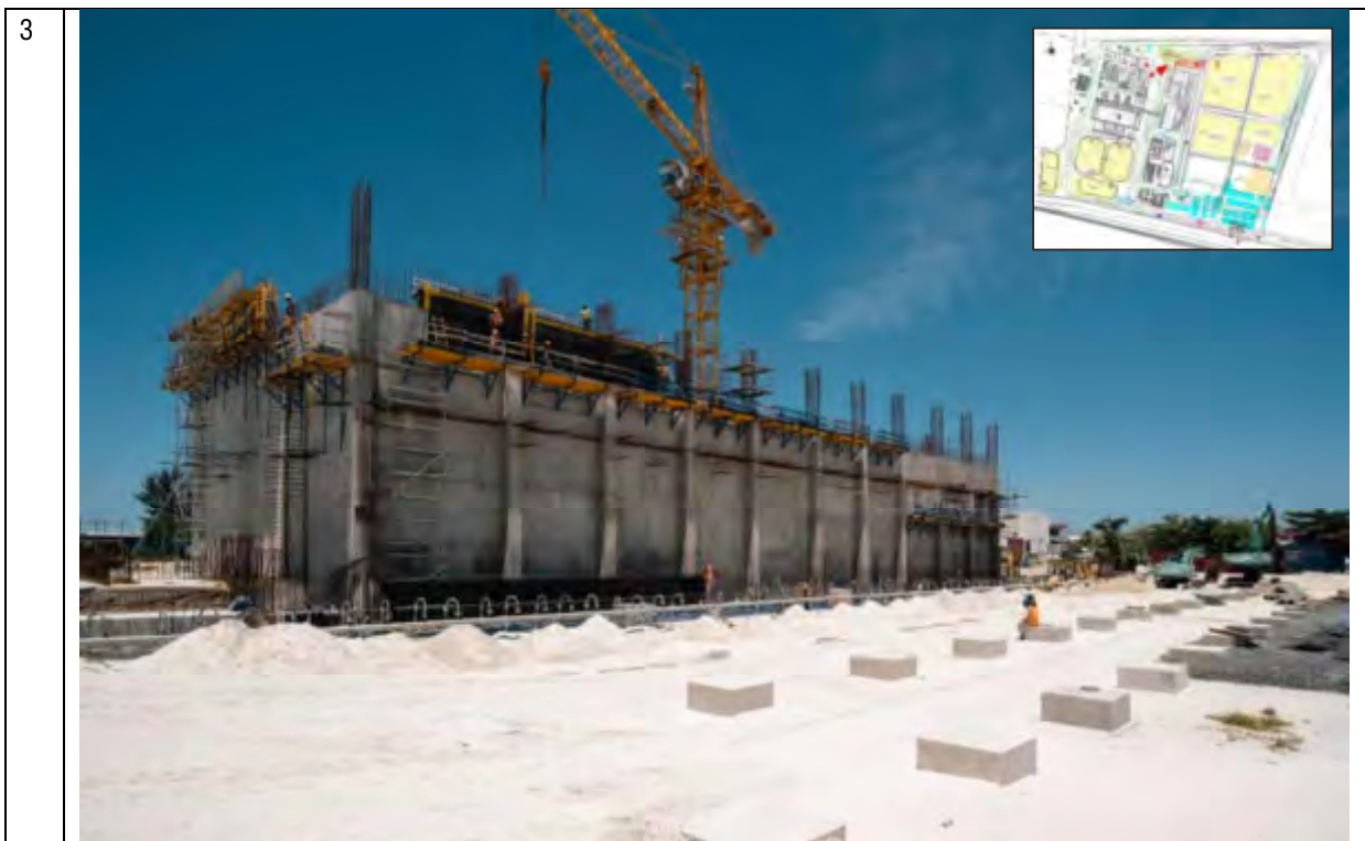
OVERALL - POINT THREE
