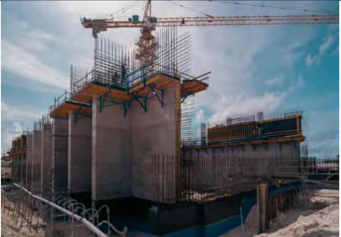
BUNKER AREA - OVERALL BUNKER WALL 4 th LAYER COMPLETED 55%
