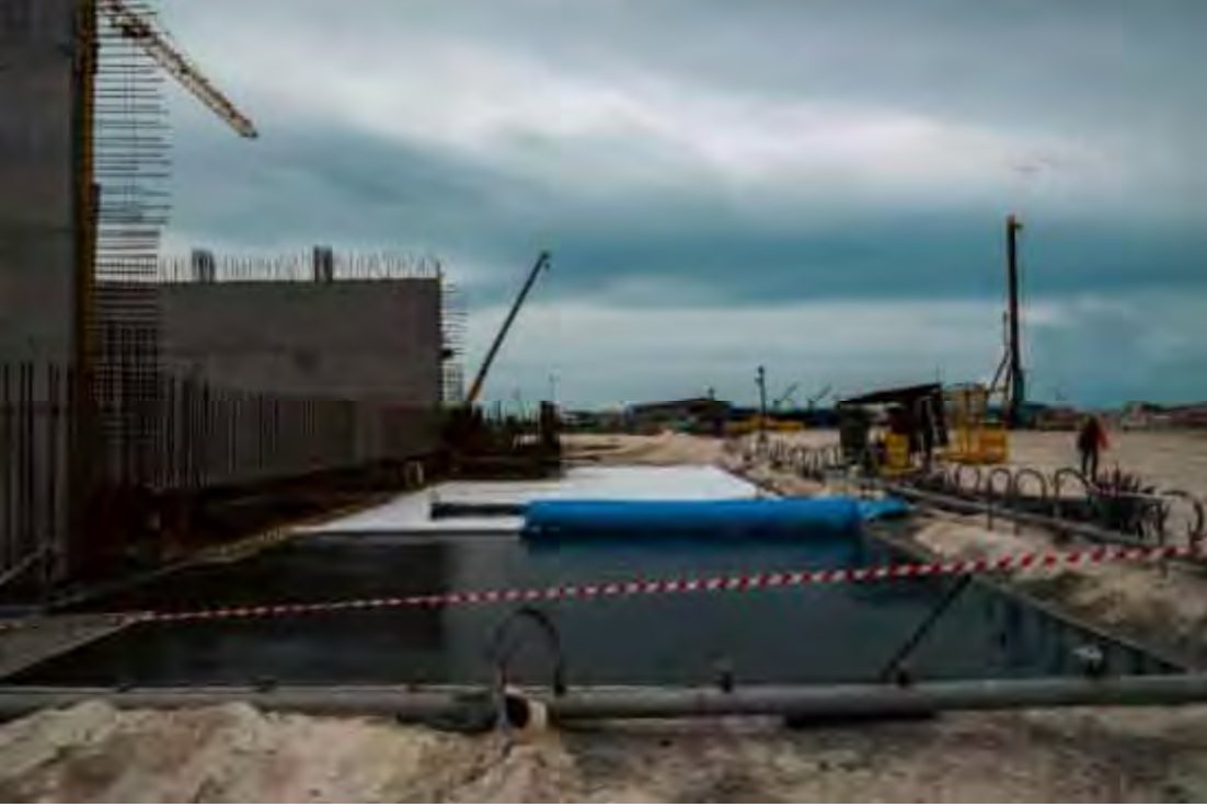
BUNKER EAST SIDE - WATERPROOFING IN PROGRESS.
