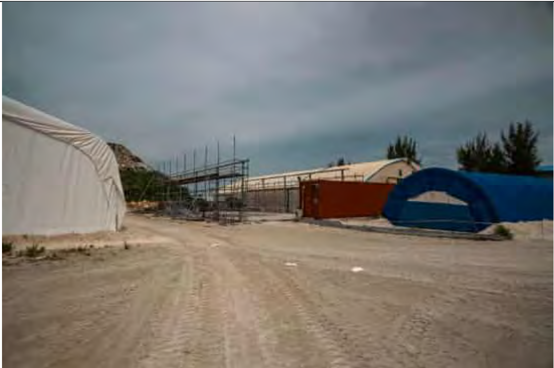
CONSTRUCTION OF DEDICATED HAZARDOUS STORAGE AREA.
