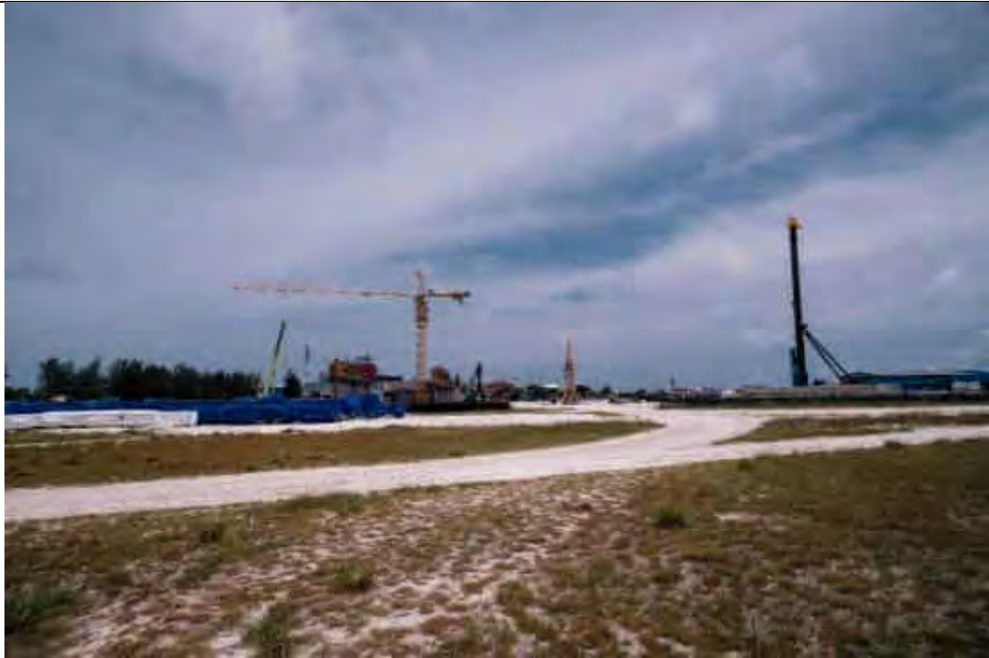
OVERALL VIEW FROM EAST SIDE
