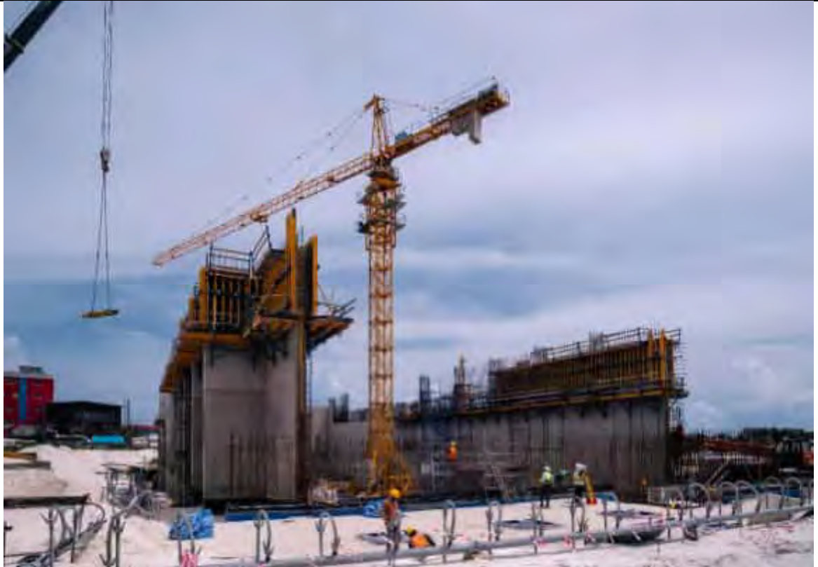
BUNKER AREA - OVERALL BUNKER WALL 4 th LAYER COMPLETED 65%
