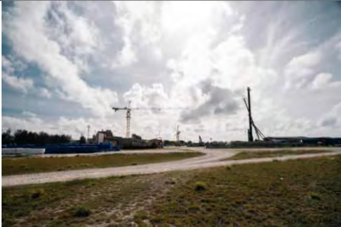
OVERALL VIEW FROM EAST SIDE
