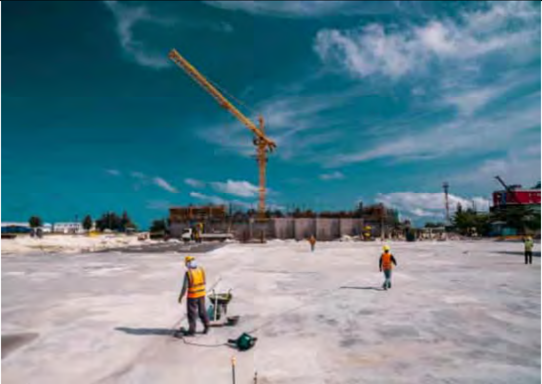
APC AREA - LEAN CONCRETE 100% COMPLETED.
