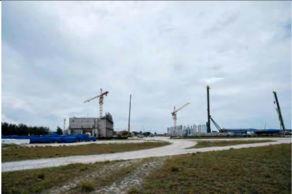
OVERALL VIEW FROM EAST SIDE
