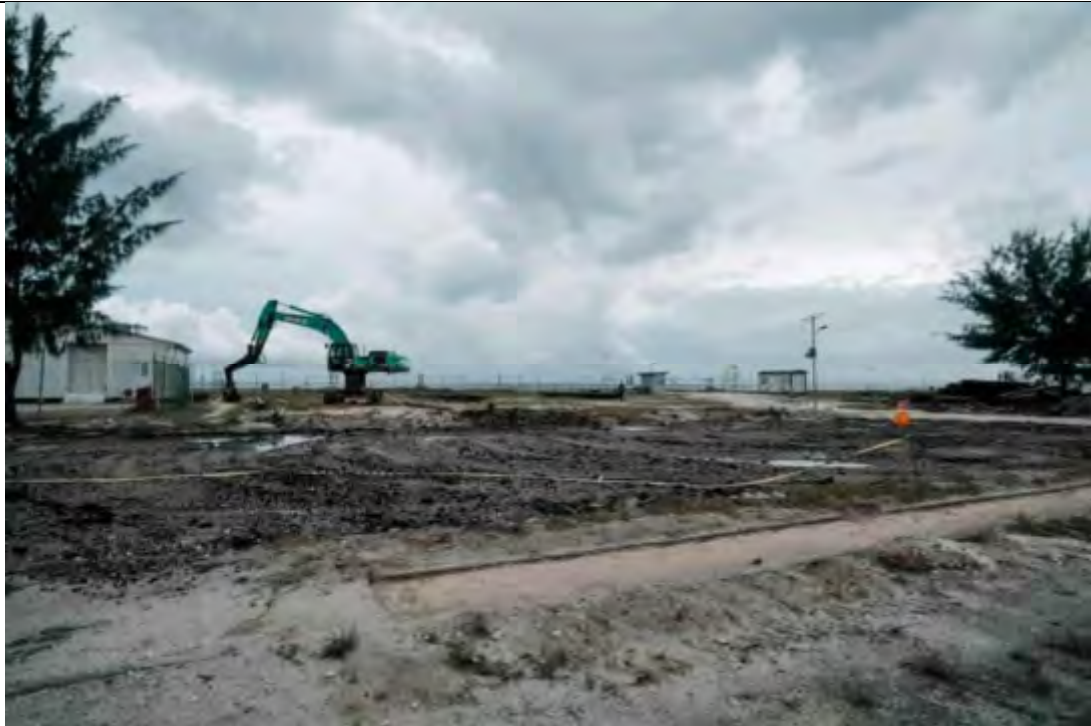
WATER INTAKE - SITE CLEARING IN PROGRESS.
