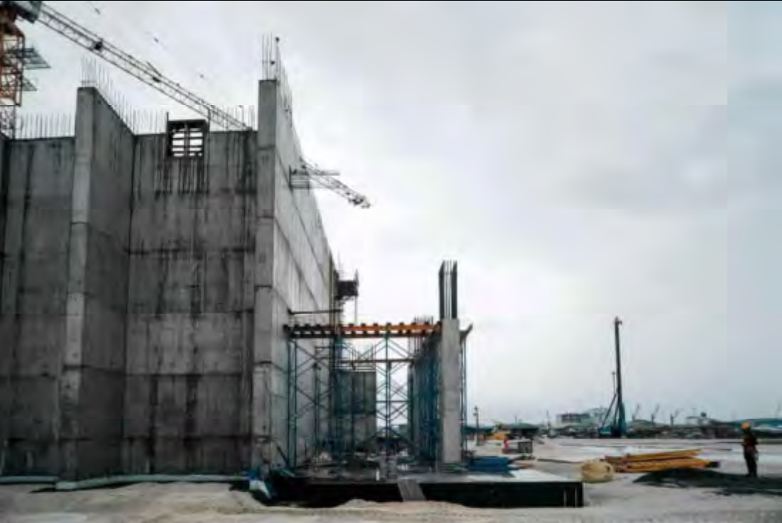
BUNKER EAST SIDE - ELEVATOR SHAFT AND COLUMN UP TO +5.0M
