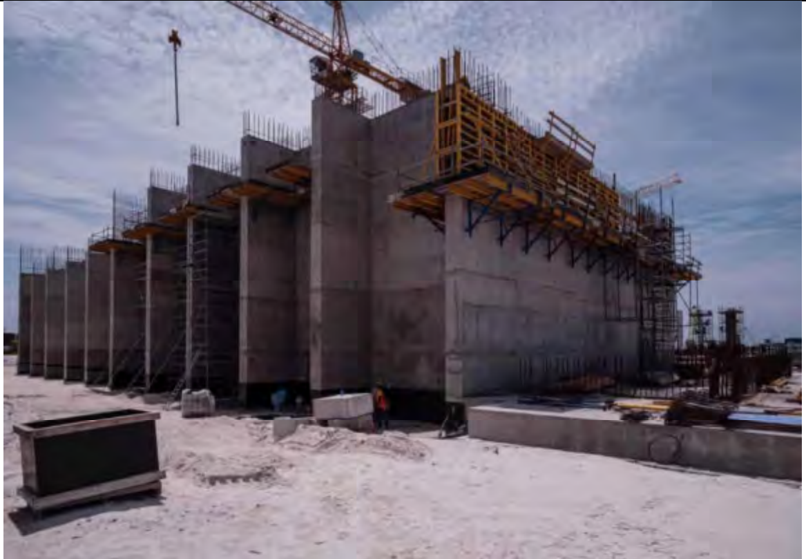
BUNKER AREA - OVERALL BUNKER WALL 4 th LAYER COMPLETED 100%
