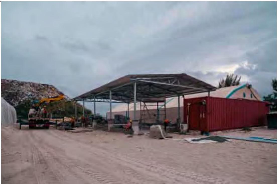
CONSTRUCTION OF DEDICATED HAZARDOUS STORAGE AREA.
