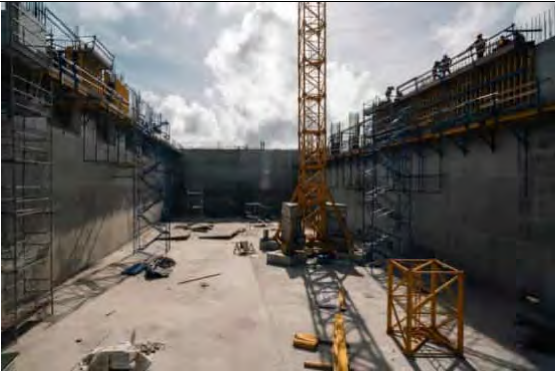
BUNKER - VIEW FROM INSIDE (EAST)
