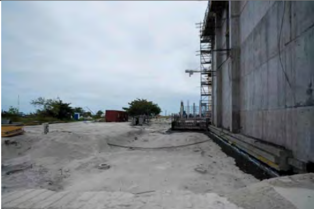
BUNKER WEST SIDE - SPUN PILE CUTTING COMPLETED.
