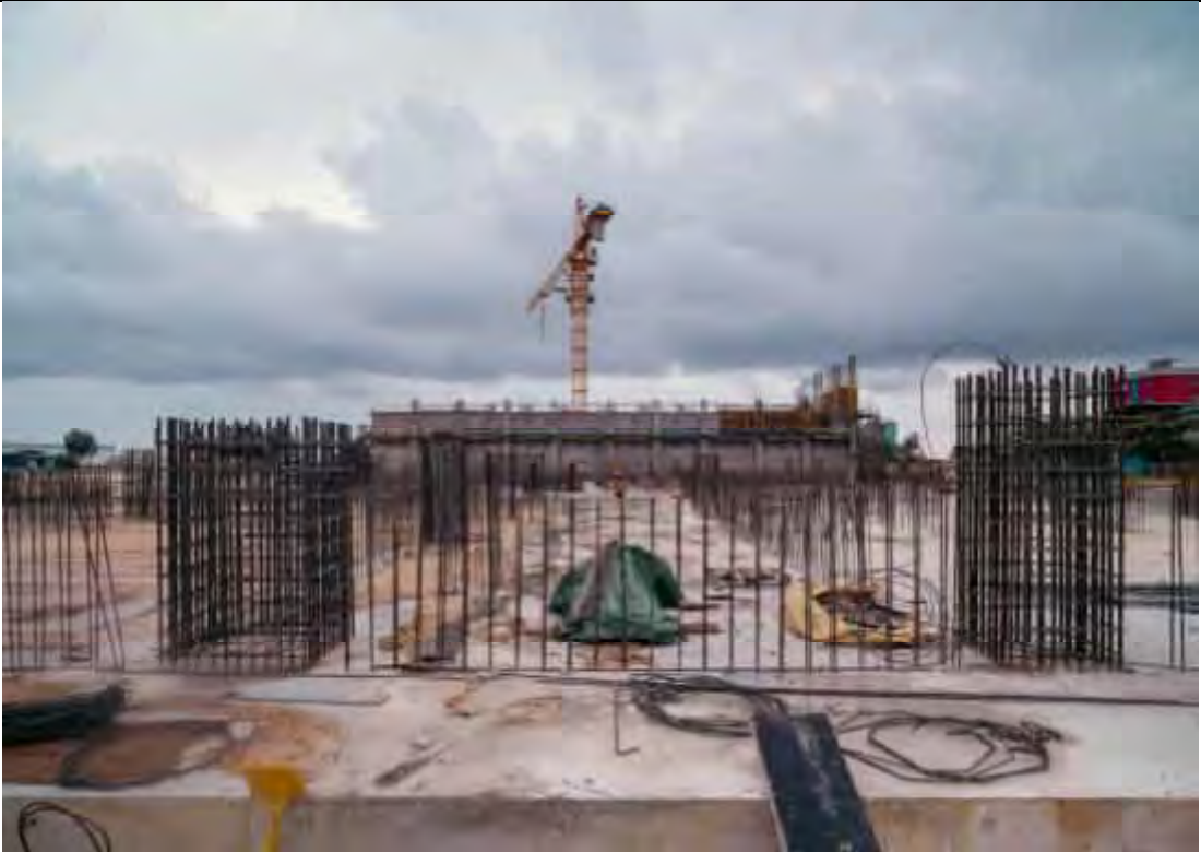
APC AREA - AREA 1, 2 & 3 CONCRETE CASTING FOR FOUNDATION COMPLETED. PROGRESSING TO COLUMN.
