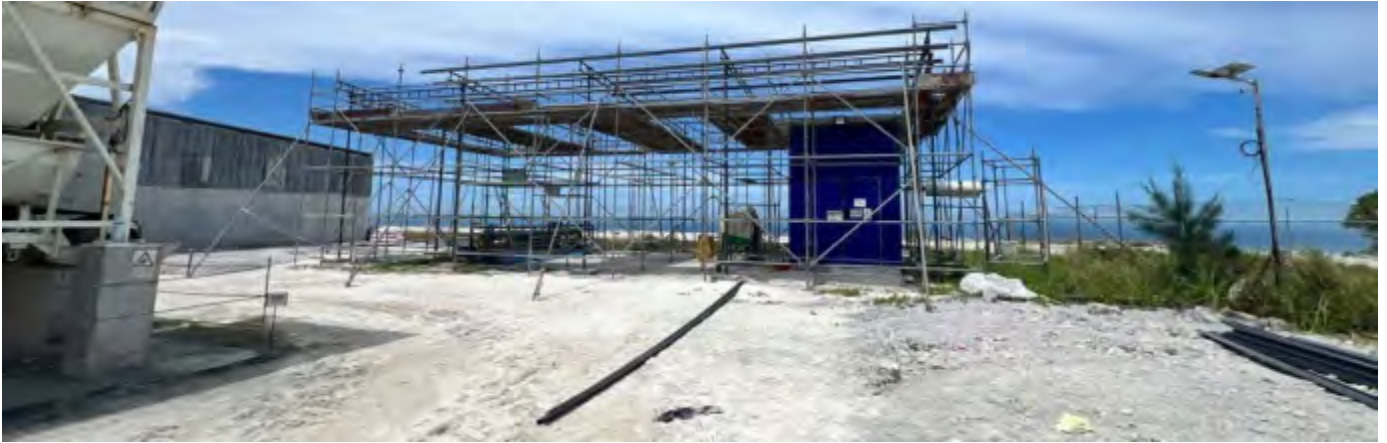
Photo 07 25/07/24 – Desalination plant building in the batching plant area is under construction.
