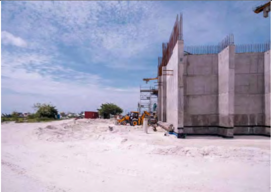
BUNKER WEST SIDE.
