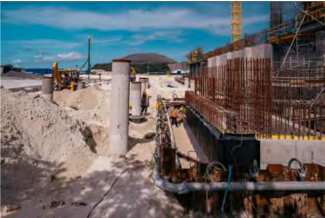
BACKFILLING ON GOING BEHIND BUNKER WALL
