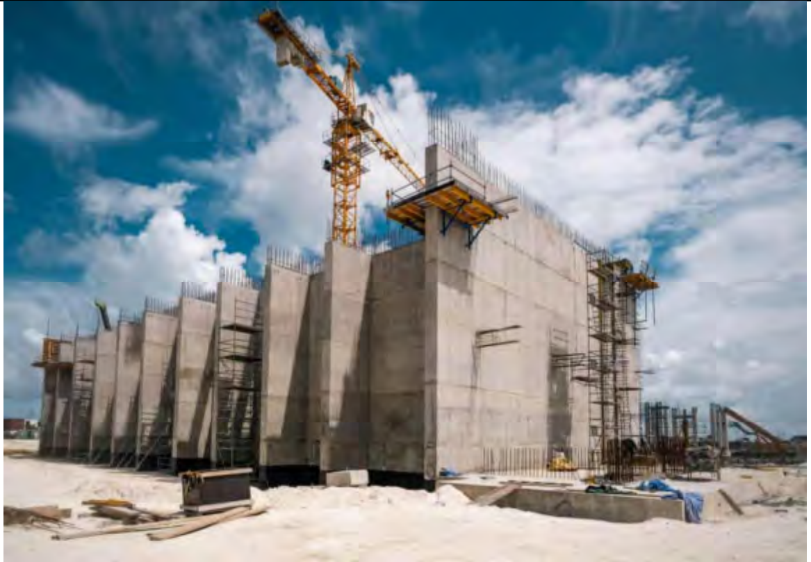
BUNKER AREA - OVERALL BUNKER WALL 6 th LAYER COMPLETED 45%
