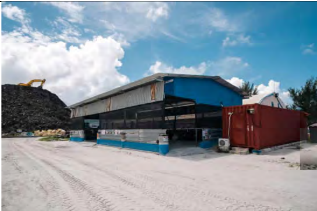
CHEMICAL STORAGE IN PROGRESS
