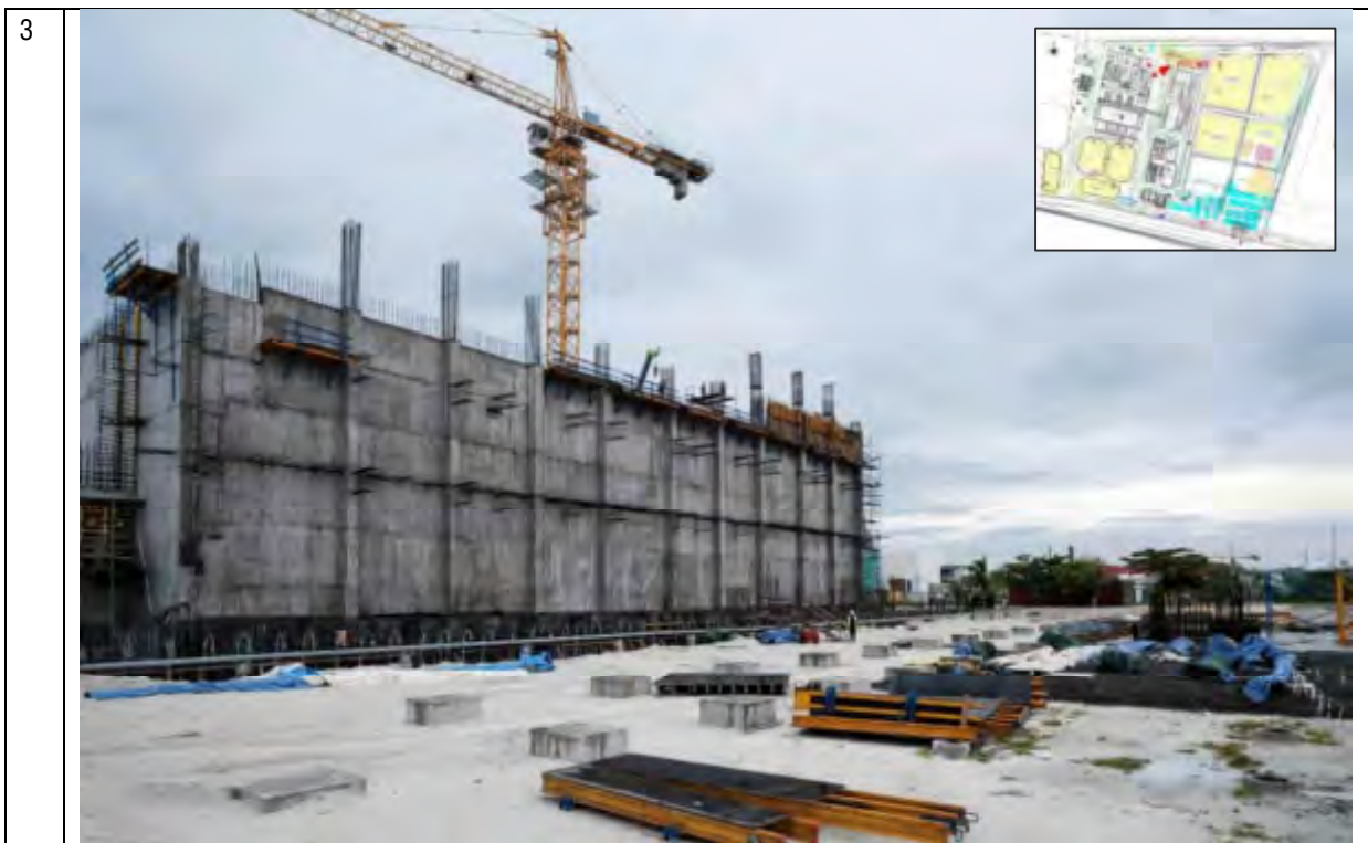
OVERALL - POINT THREE
