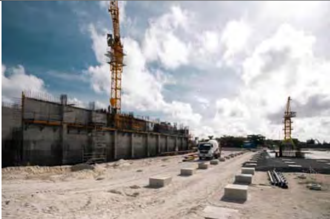
INCINERATOR AREA - PILECAPS IN PROGRESS.
