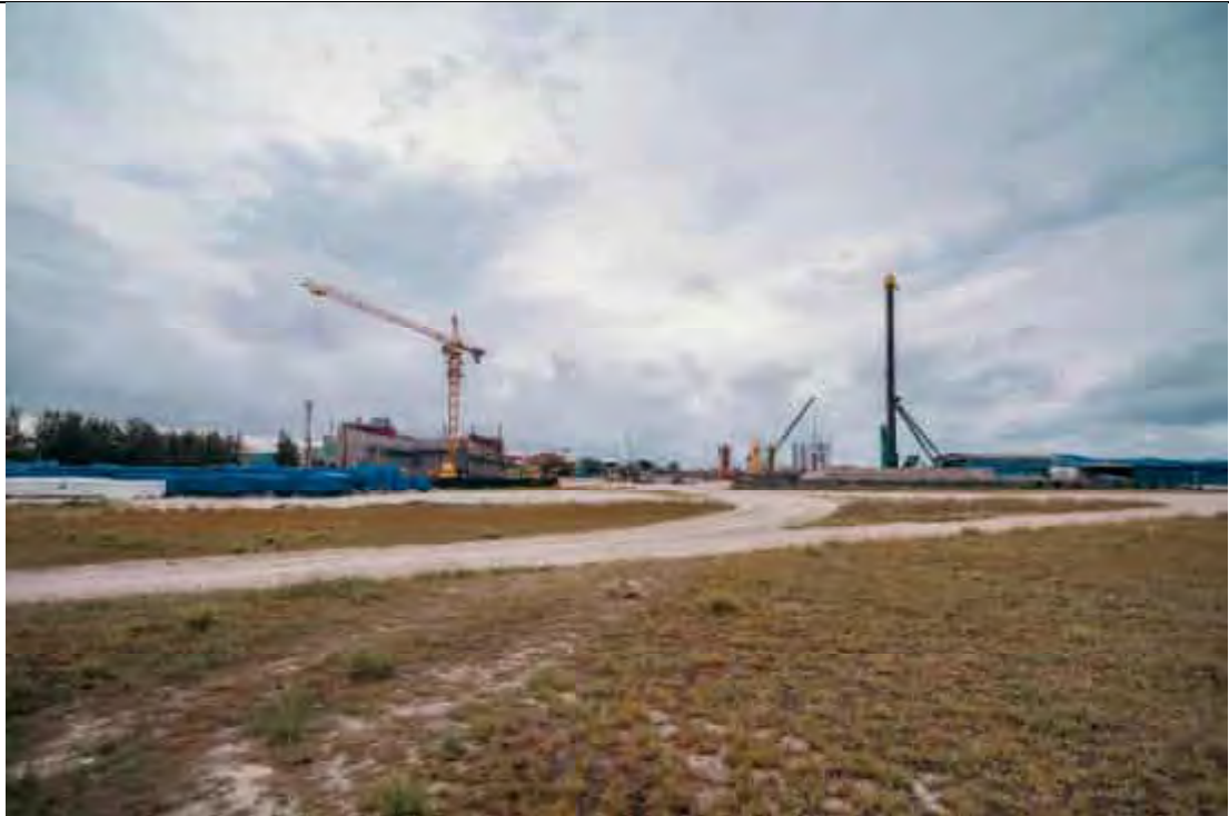
OVERALL VIEW FROM EAST SIDE
