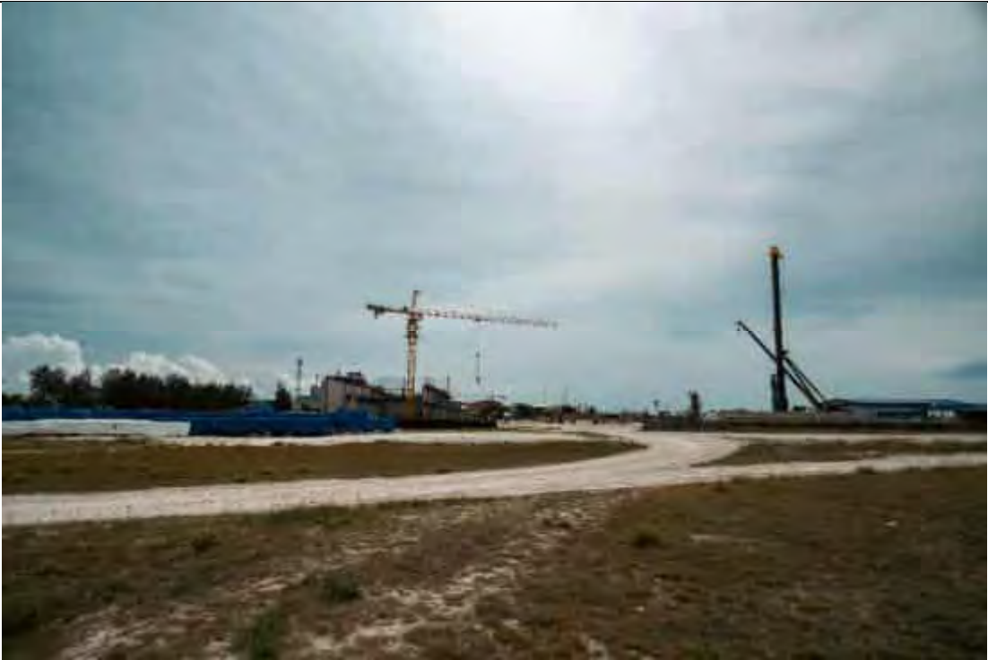
OVERALL VIEW FROM EAST SIDE
