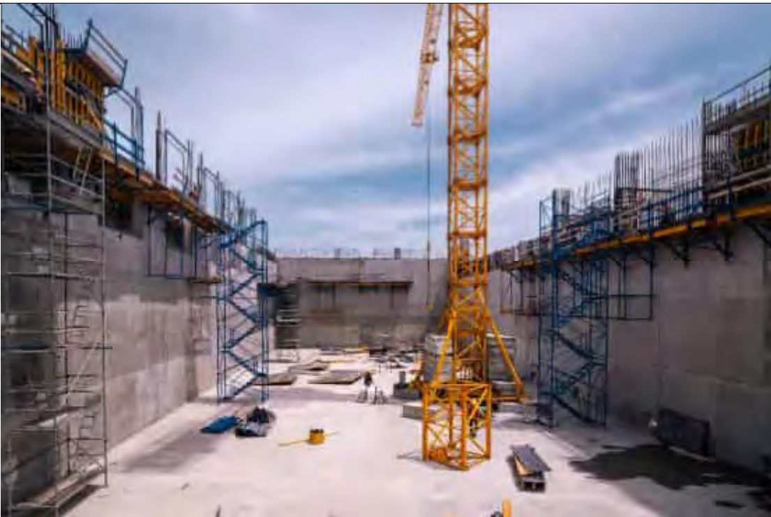
BUNKER - VIEW FROM INSIDE (EAST)
