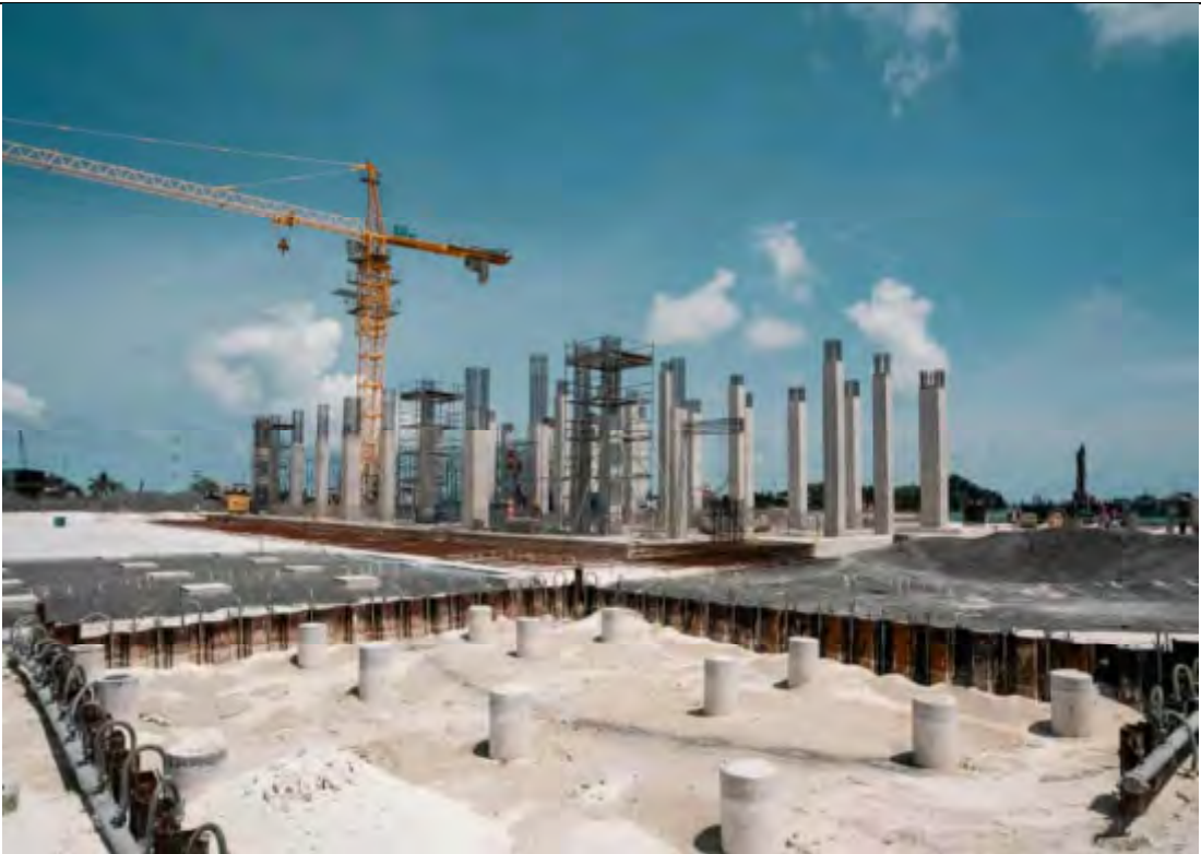
APC AREA - PREPARATION OF FALSEWORK FOR BEAMS IN PROGRES.
