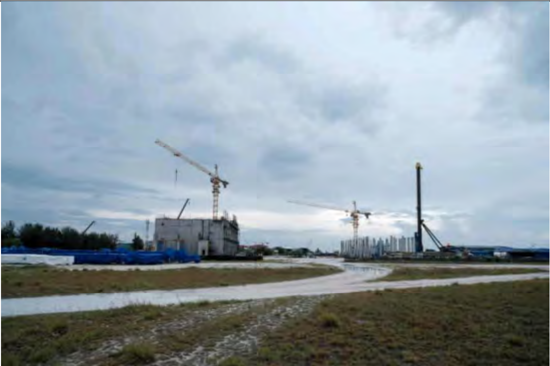
OVERALL VIEW FROM EAST SIDE
