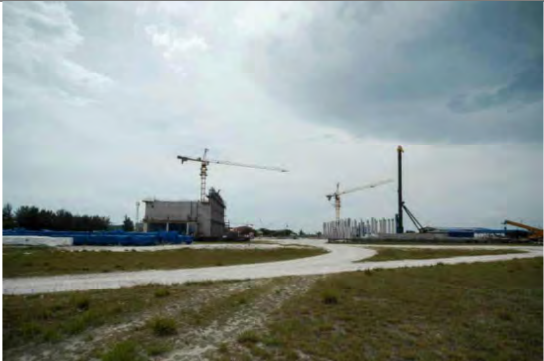
OVERALL VIEW FROM EAST SIDE
