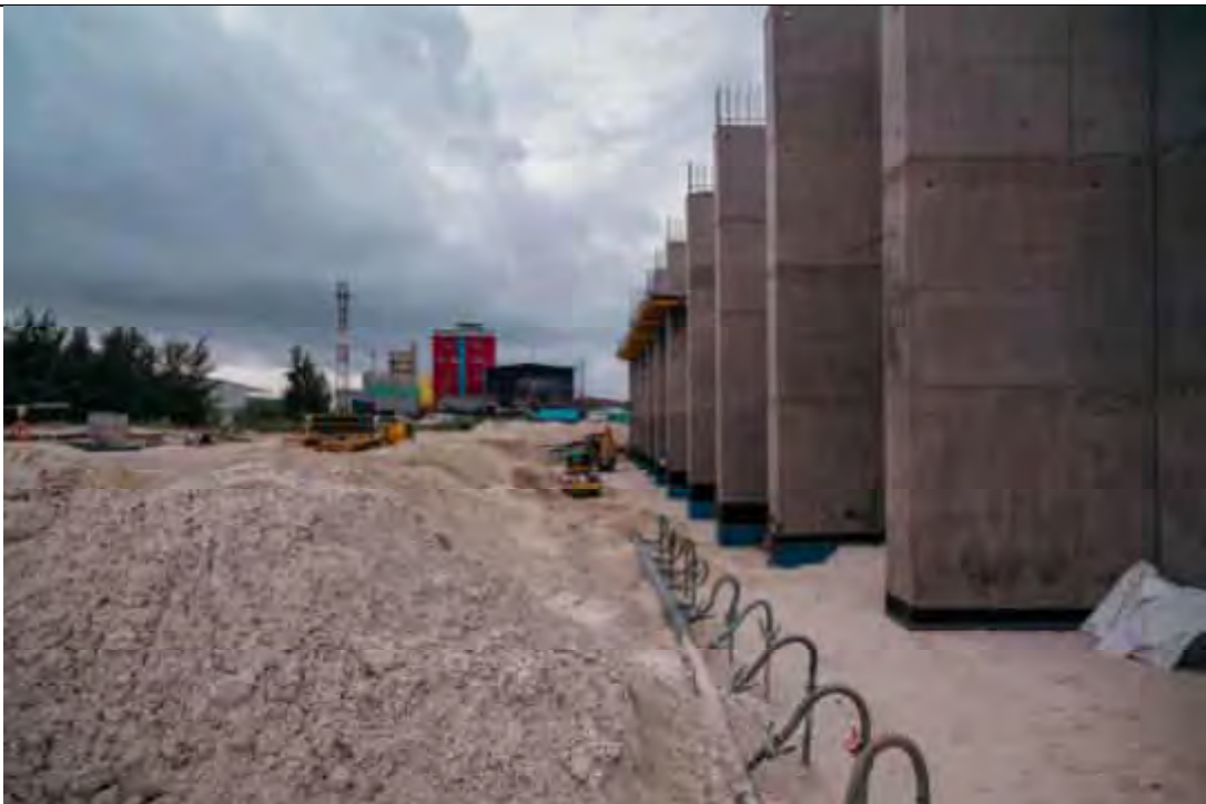
STRUCTURAL BACKFILLING BEHIND BUNKER WALL IN PROGRESS.
