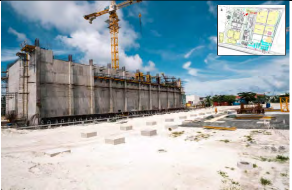
OVERALL - POINT THREE
