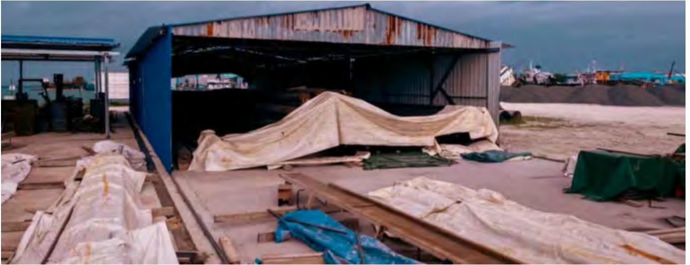
Photo 12 13/08/24– Reinforcement stock on site and workshop area.
