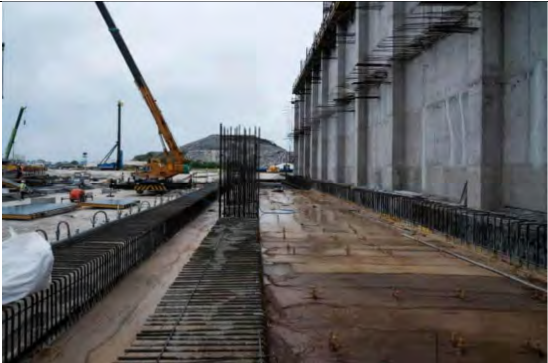
INCINERATOR AREA - AREA 11 FOUNDATION COMPLETED.
