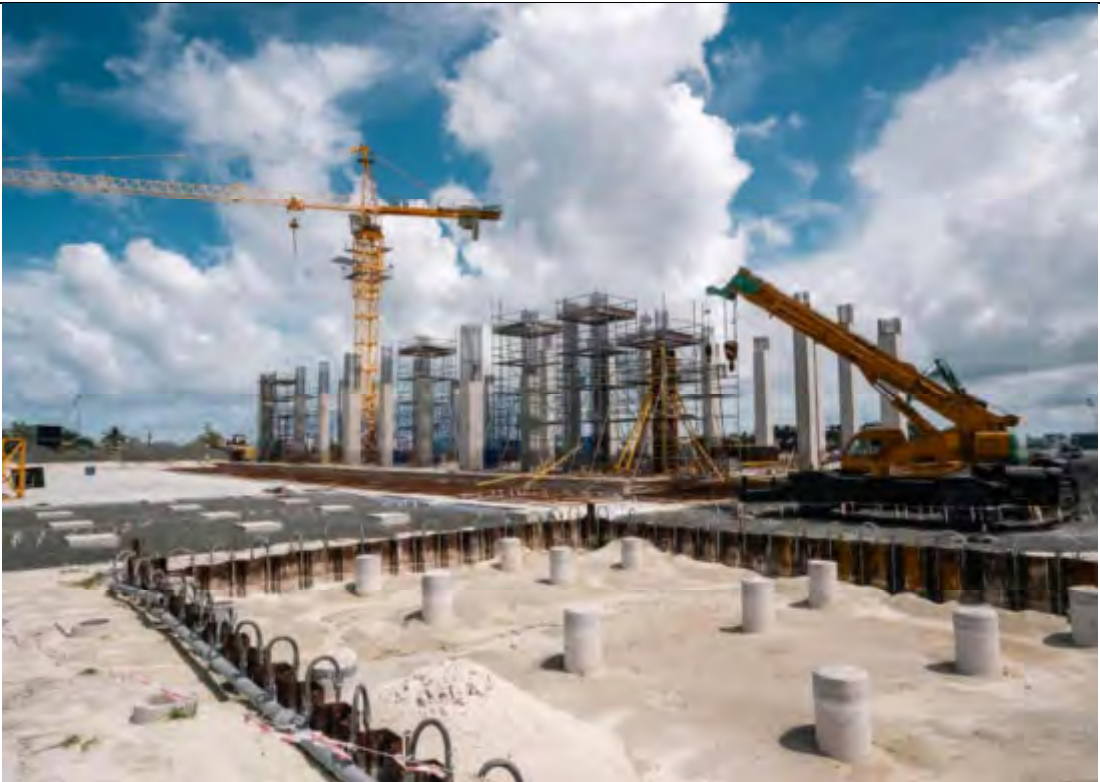
APC AREA - AREA 1, 2 & 3 CONCRETE CASTING FOR COLUMNS COMPLETED.
