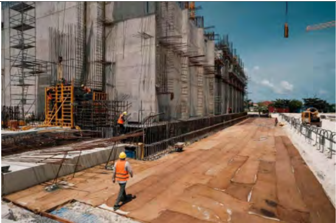
INCINERATOR AREA - LEAN CONCRETE COMPLETED.
