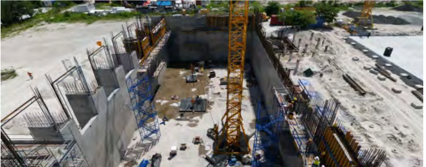
Photo 05 09/07/24 – Bunker wall construction is progressing as planned.
