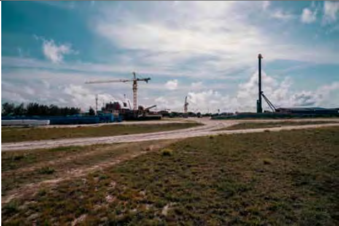
OVERALL VIEW FROM EAST SIDE
