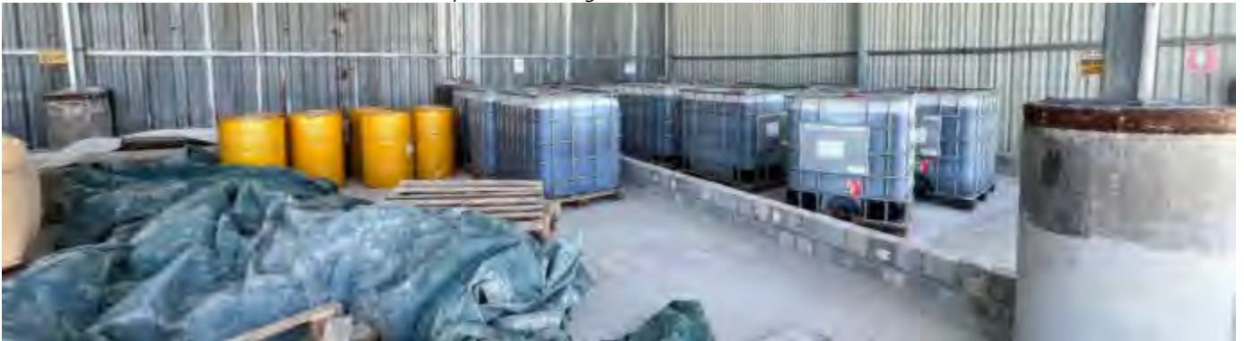
Photo 20 18/07/24– Chemical storage area, proper bund wall needs to be in place all around the storage area and all chemicals need to be moved to this dedicated areas as soon as possible.
