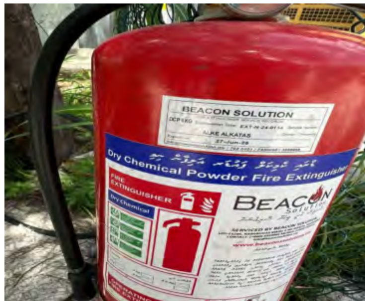
Figure 2: Fire extinguishers inspected by third party
