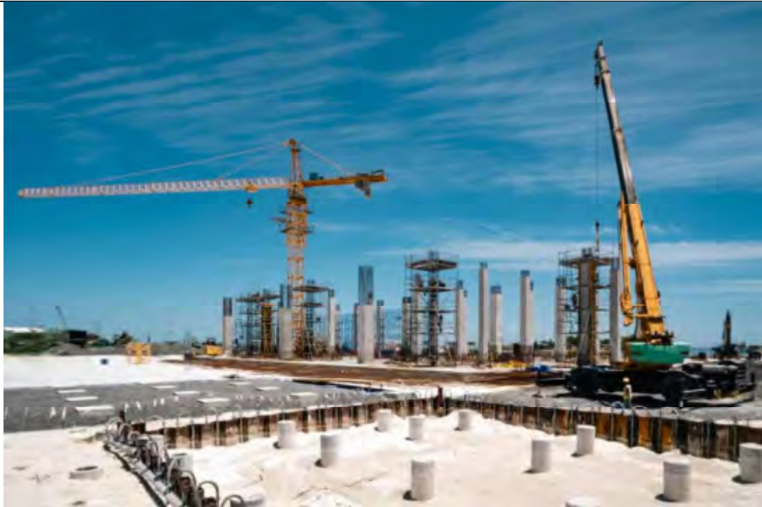
TOWER CRANE INSTALLATION COMPLETED AT APC AREA 1
