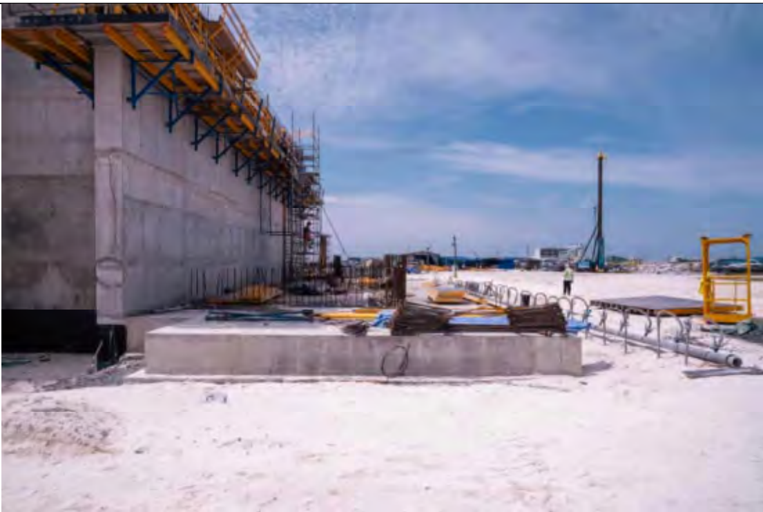
BUNKER EAST SIDE - CONCRETE CASTING FOR FOUNDATION SLAB COMPLETED.
