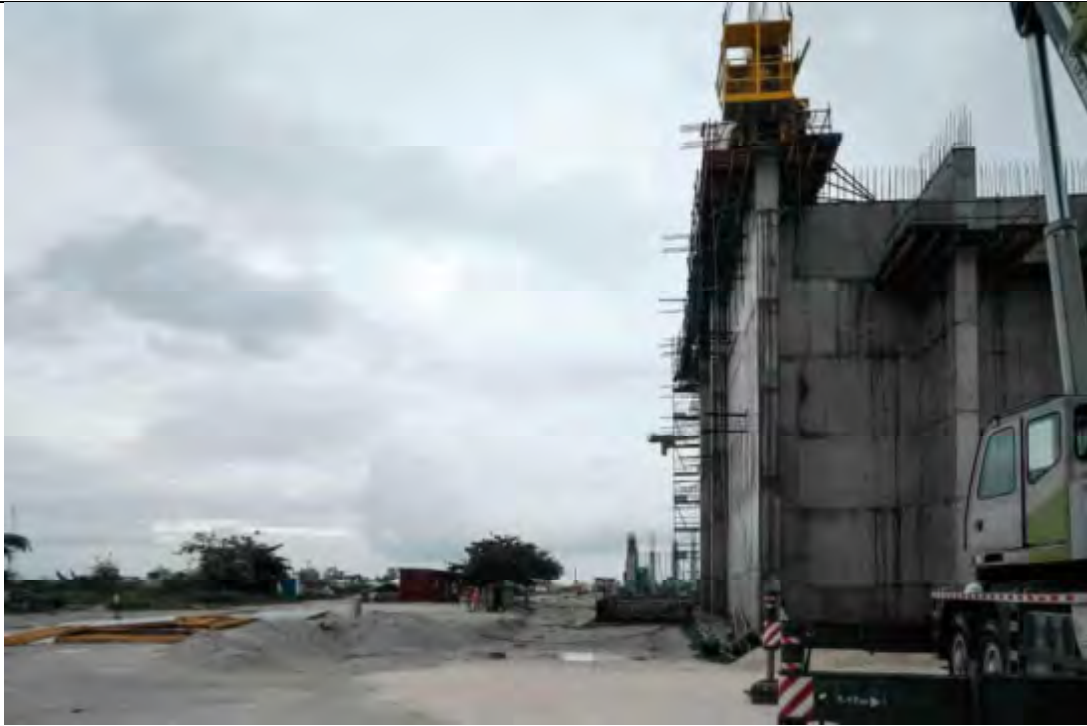
BUNKER WEST SIDE - SPUN PILE CUTTING COMPLETED.
