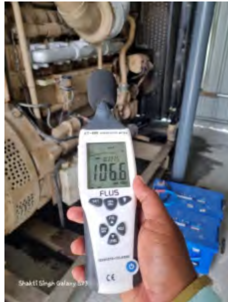
Batching Plant Generator
