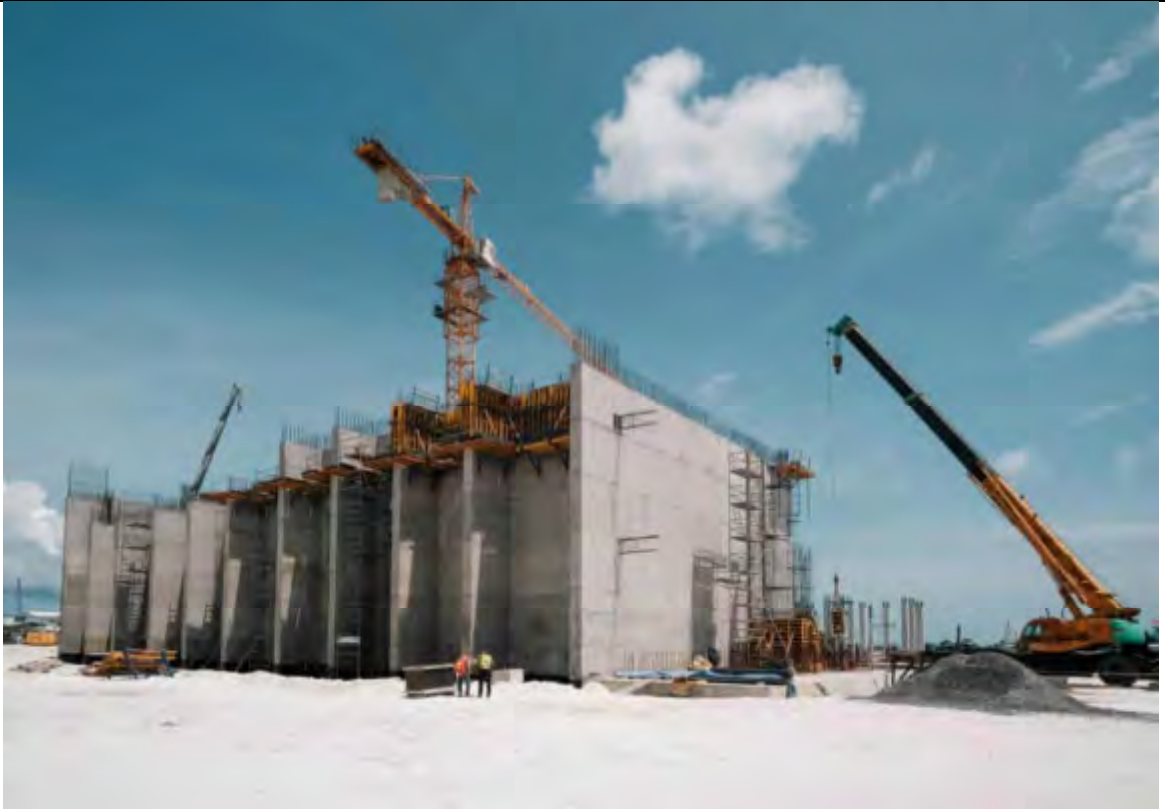
BUNKER AREA - OVERALL BUNKER WALL 1 ST TO 6 TH (+15.00) LAYER 100% COMPLETED.
