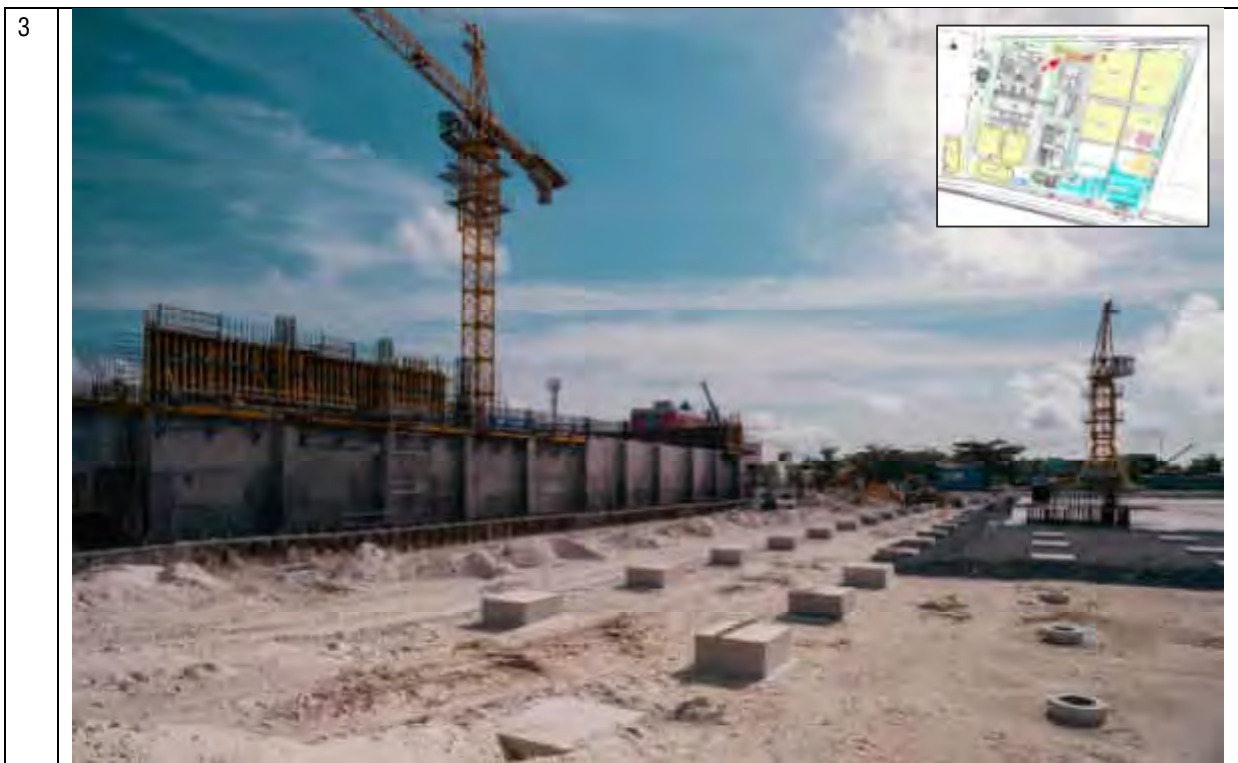
OVERALL - POINT THREE
