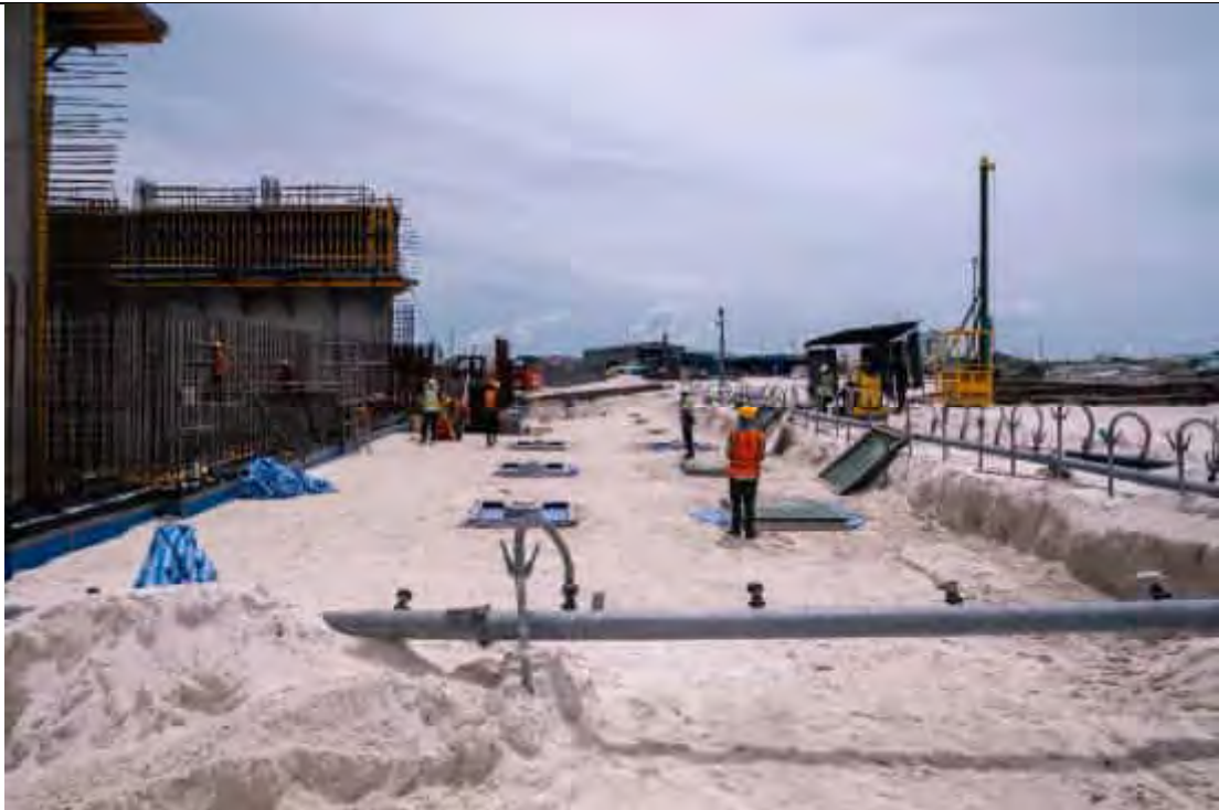
BUNKER EAST SIDE - EXCAVATION AND PILECAP IN PROGRESS.
