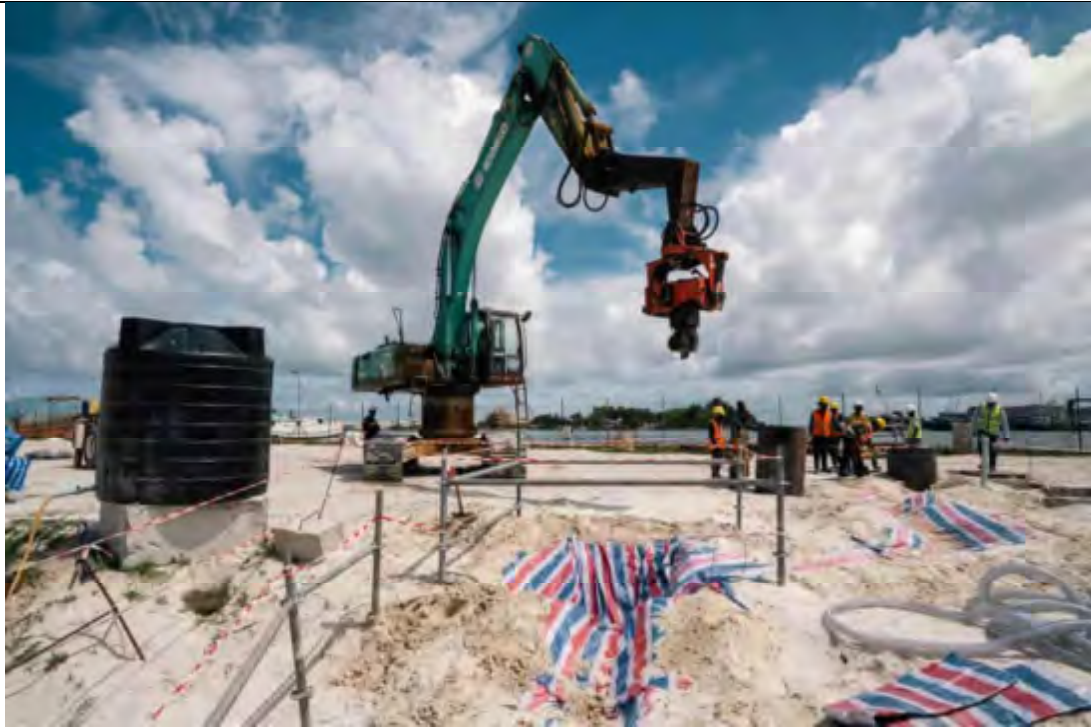
CHIMNEY AREA - TEST BORED PILE IN PROGRESS.
