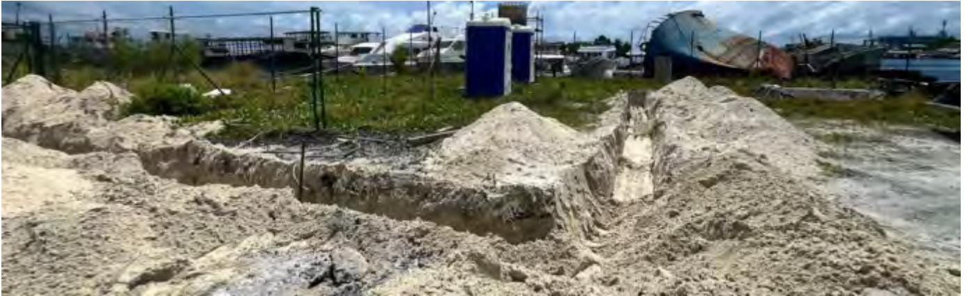
Photo 11 18/07/24 – Excavation work is ongoing for temporary cable laying.
