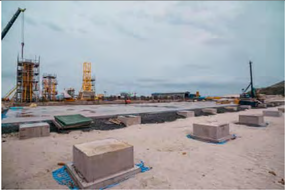
BOILER AREA - NO ACTIVIITY.
