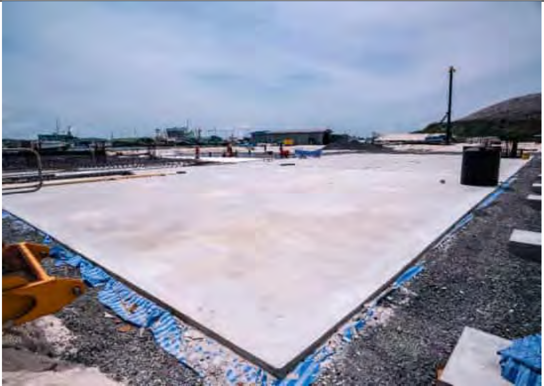
BOILER AREA - LEAN CONCRETE 100%, NO FURTHER ACTIVITIES.
