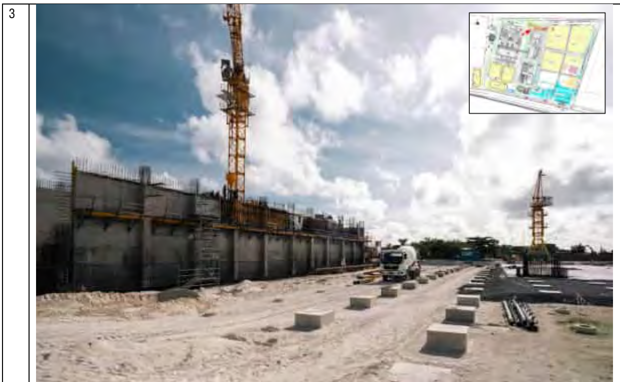
OVERALL - POINT THREE
