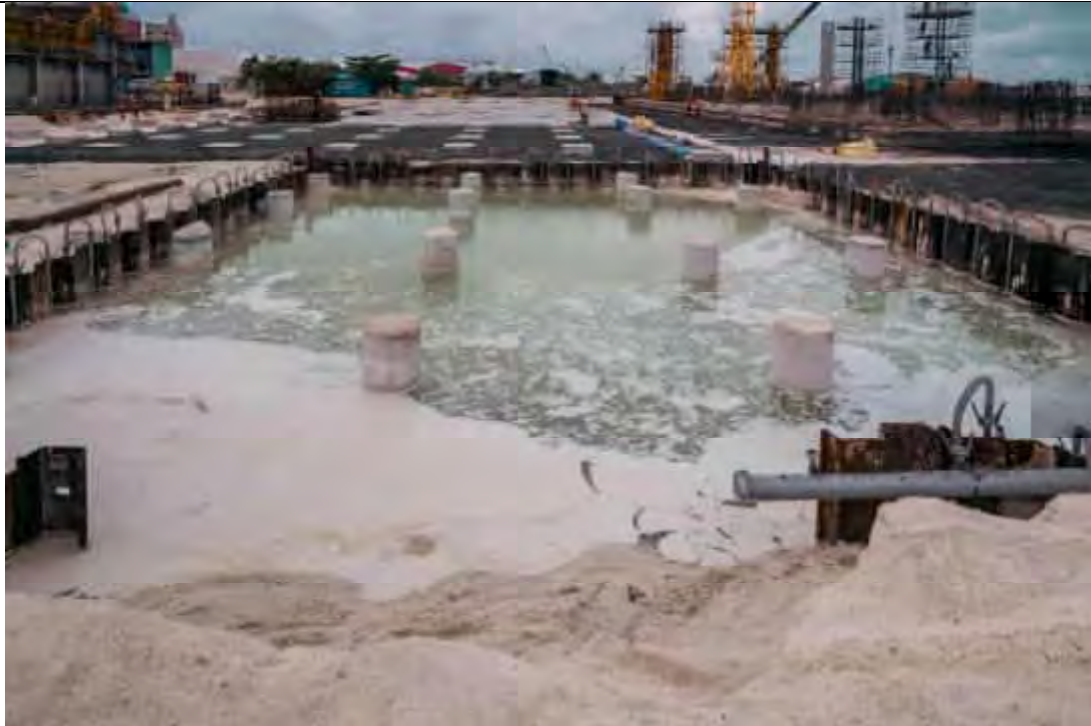
TURBINE AREA - SHEETPILE COMPLETED.
