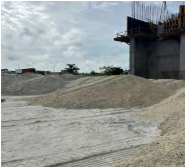
Storage of soil at construction site for backfilling.
