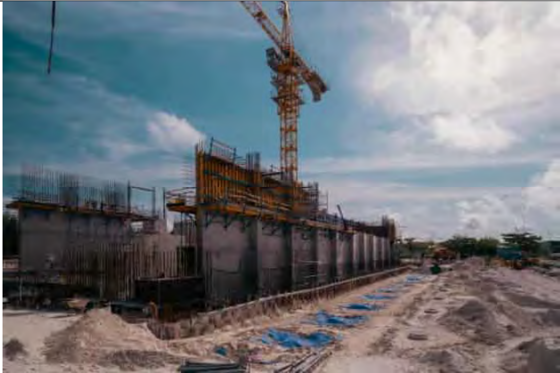
INCINERATOR -REMOVAL OF SHEETPILE ANCHORE WAS SUCCESS.
