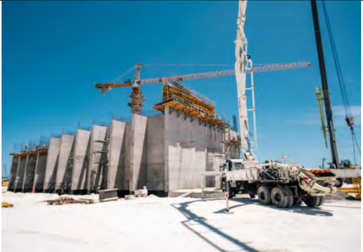
BUNKER AREA - OVERALL BUNKER WALL 5 th LAYER COMPLETED 95%
