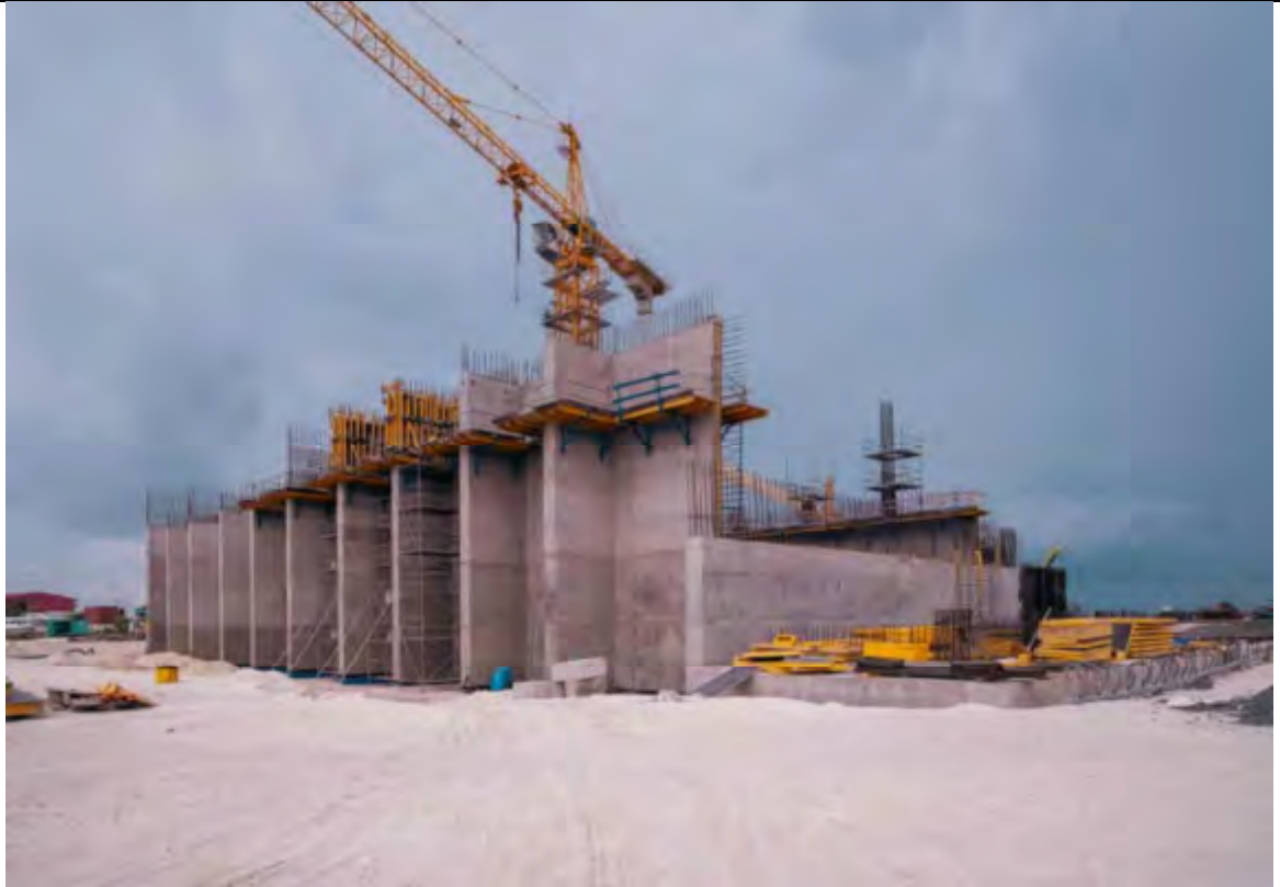
BUNKER AREA - OVERALL BUNKER WALL 4 th LAYER COMPLETED 85%
