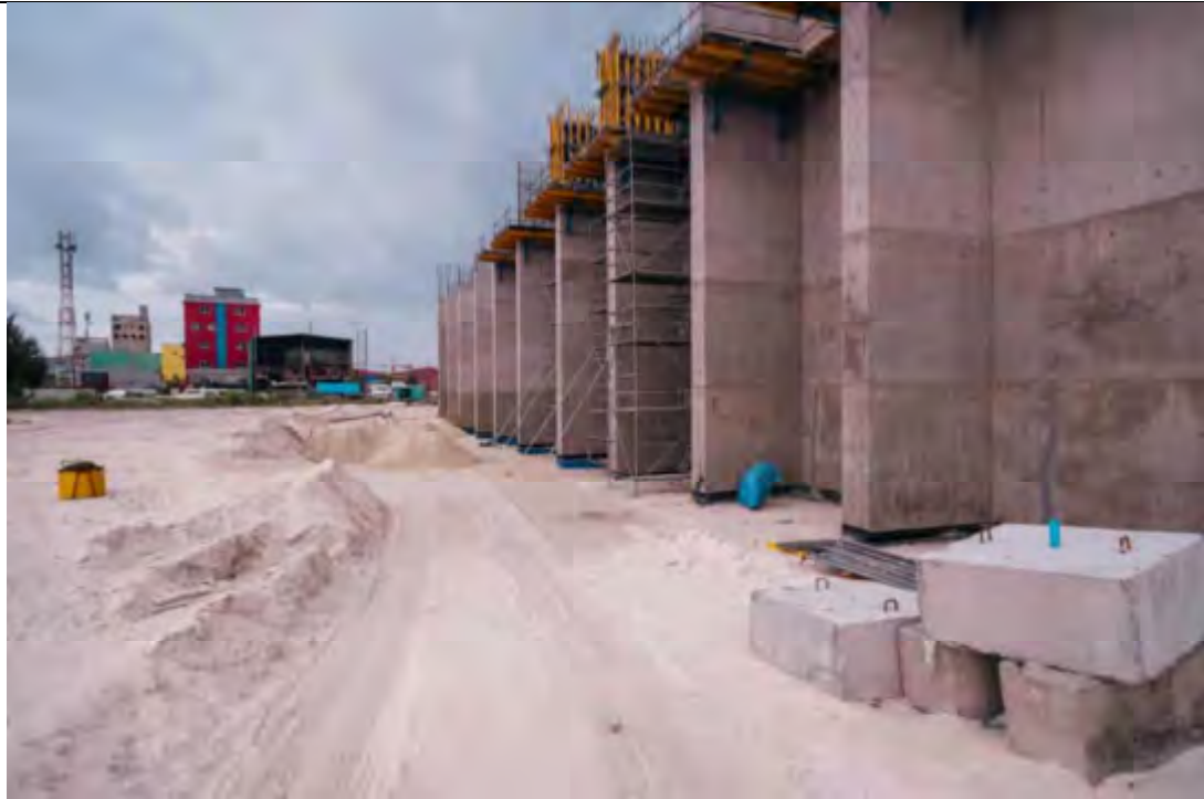
STRUCTURAL BACKFILLING WORK BEHIND BUNKER WALL IN PROGRESS
