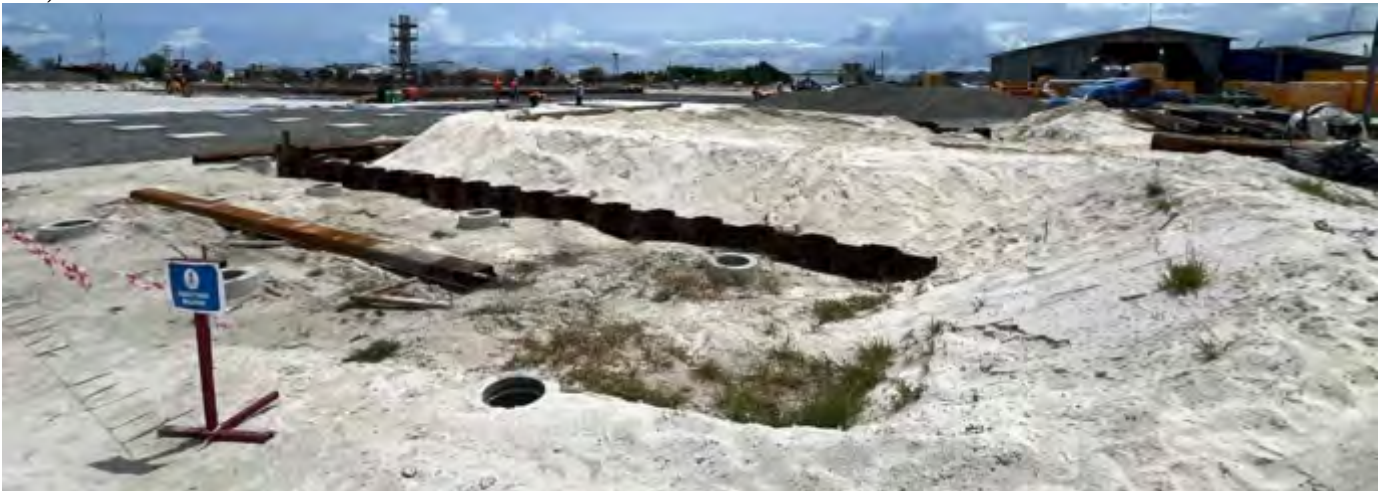
Photo 03 25/07/24 – Sheet piling work for the turbine foundation area is ongoing.
