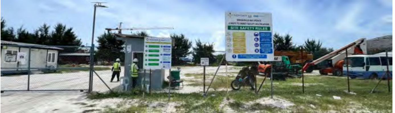
Photo 09 25/07/24– Safety signage placed at the main entrance to the site.
