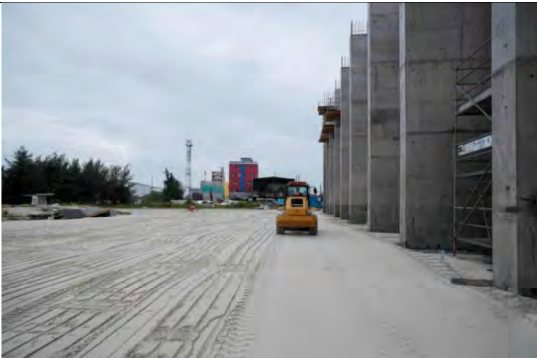
BUNKER SOUTH SIDE BACKFILLING IN PROGRESS.
