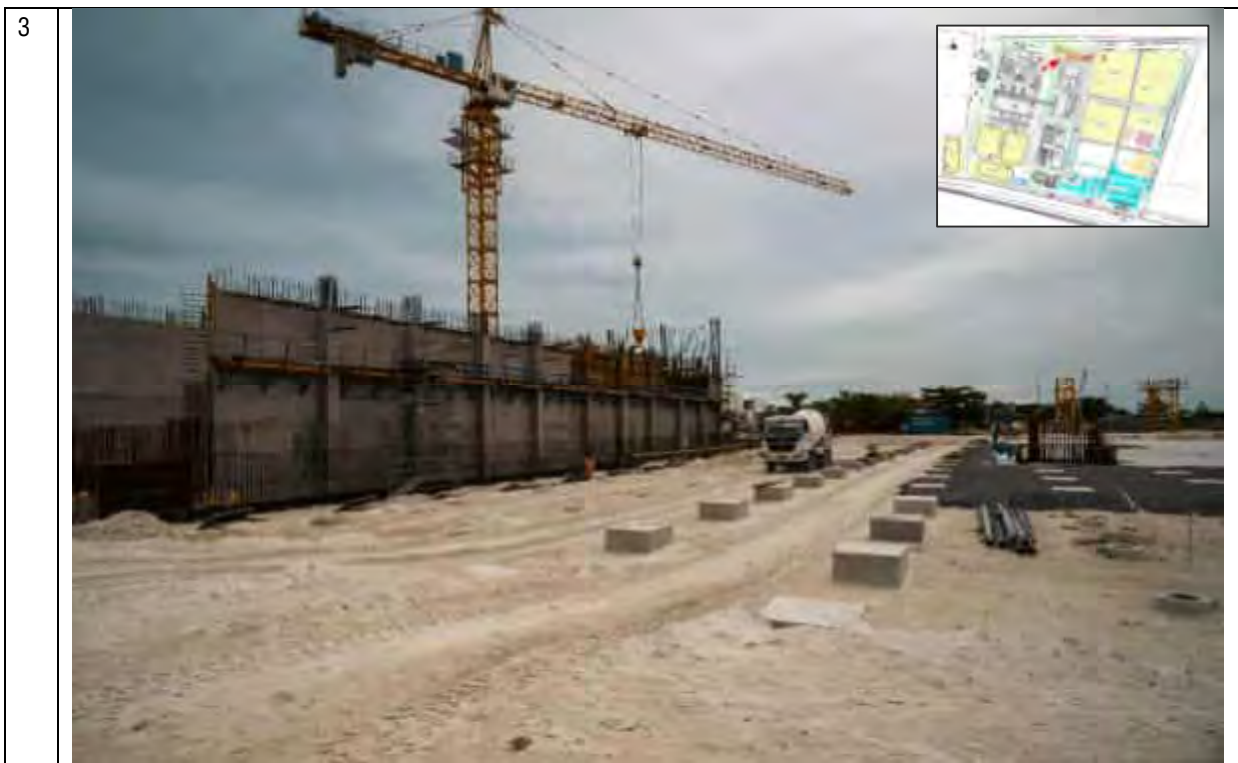
OVERALL - POINT THREE
