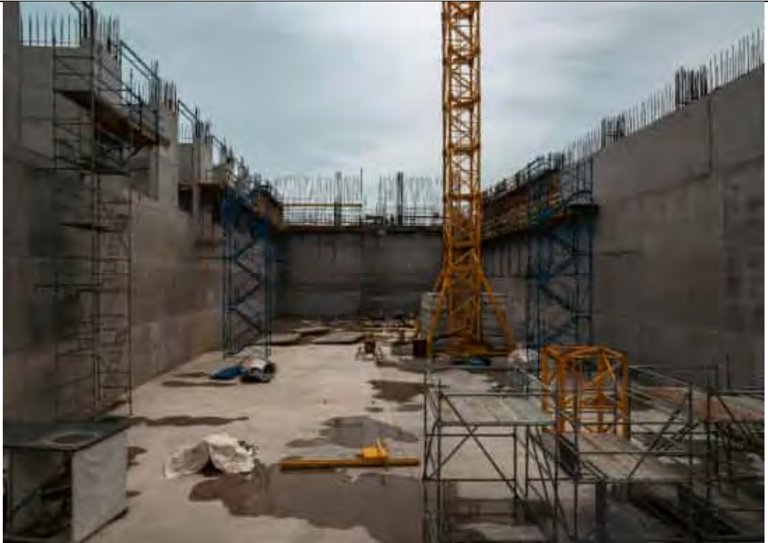
BUNKER (INSIDE) VIEW.
