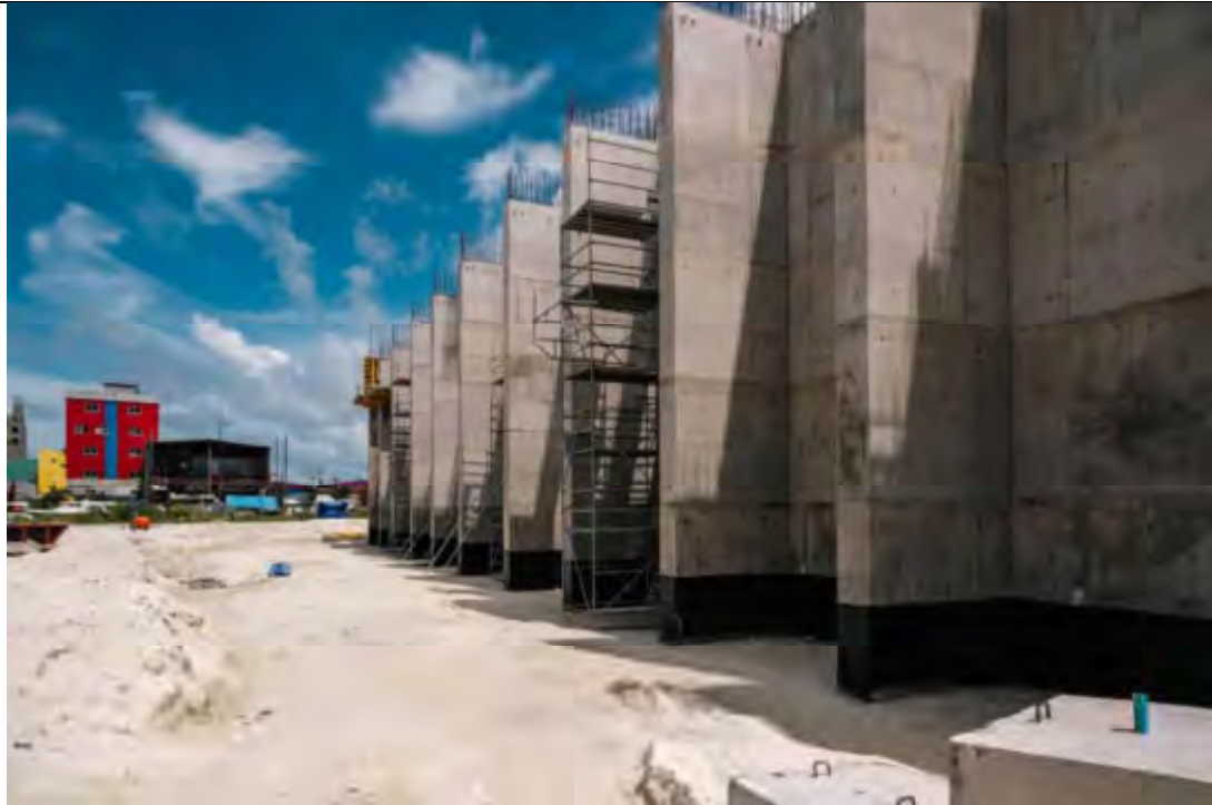
STRUCTURAL BACKFILLING WORK BEHIND BUNKER WALL RECTIFIED
