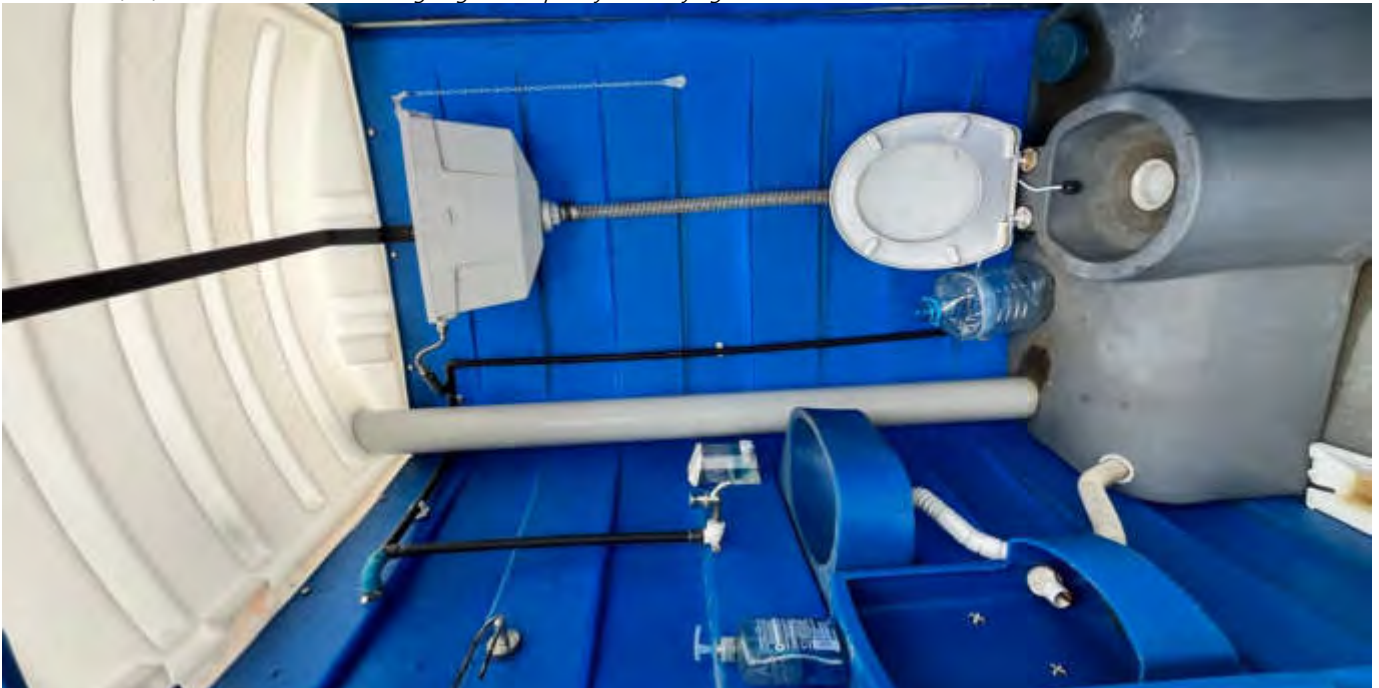
Photo 12 18/07/24– Portable toilets are kept cleaned and maintained.
