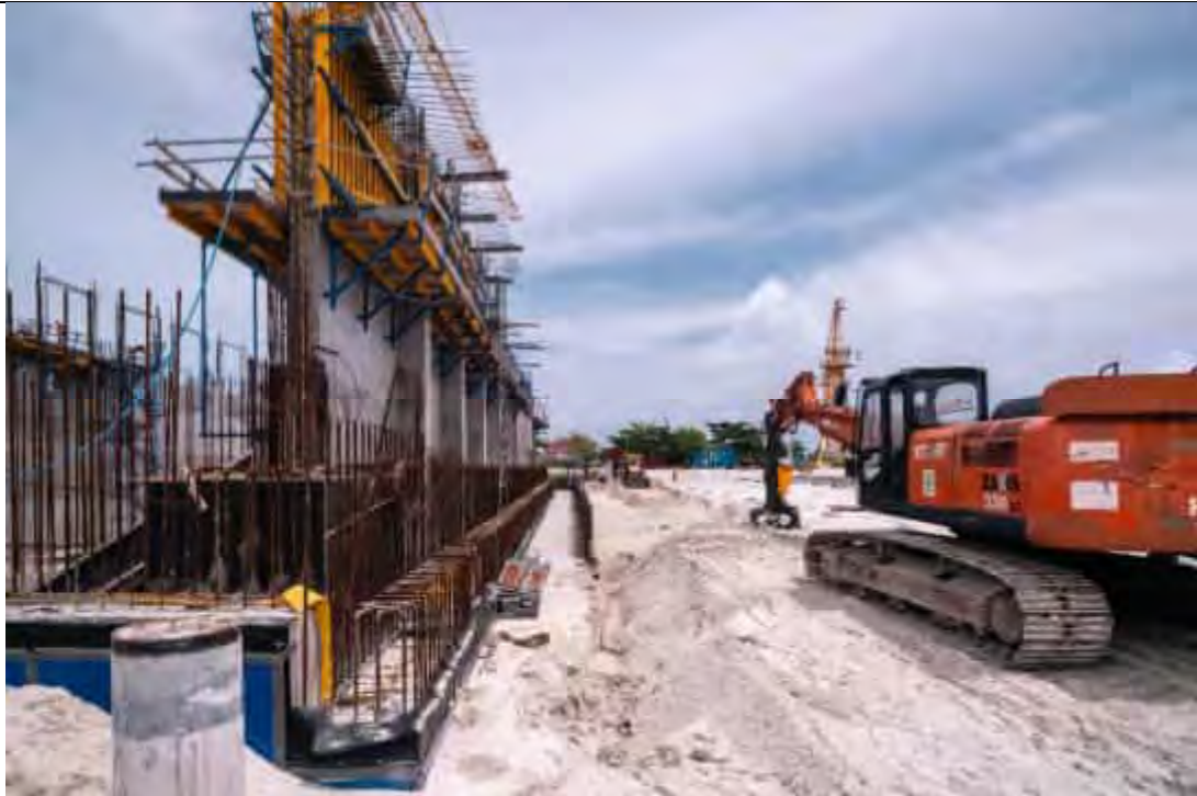
INCINERATOR AREA - EXCAVATION & SPUN PILE CUTTING IN PROGRESS.
