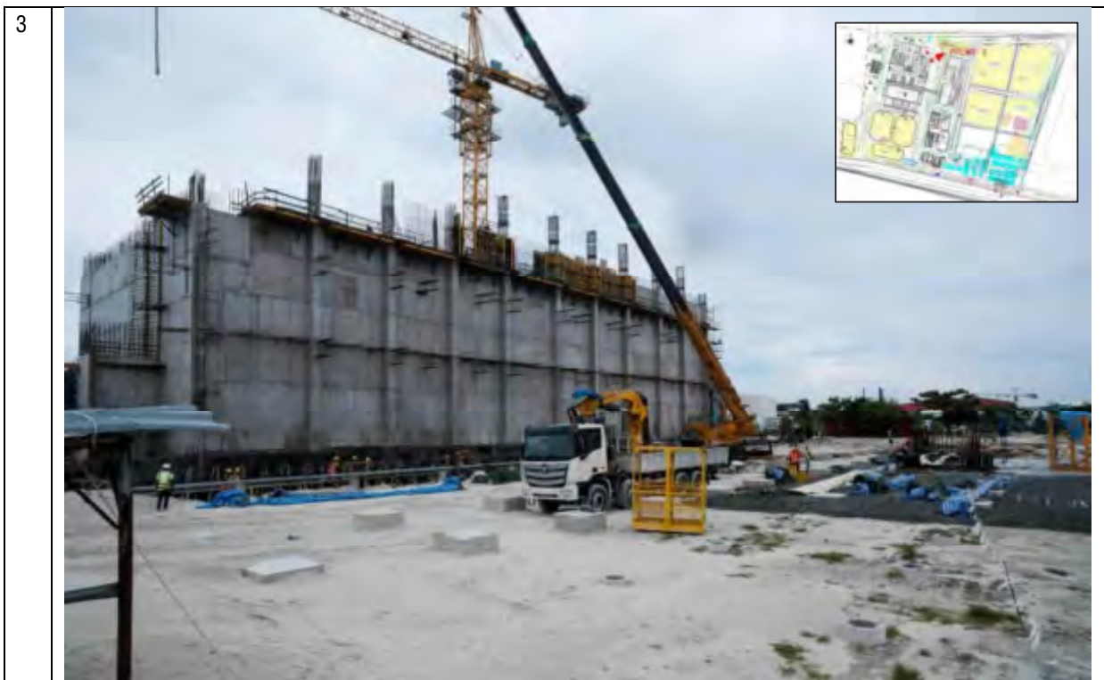
OVERALL - POINT THREE
