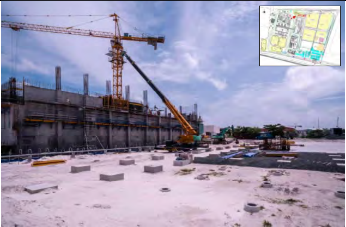
OVERALL - POINT THREE
