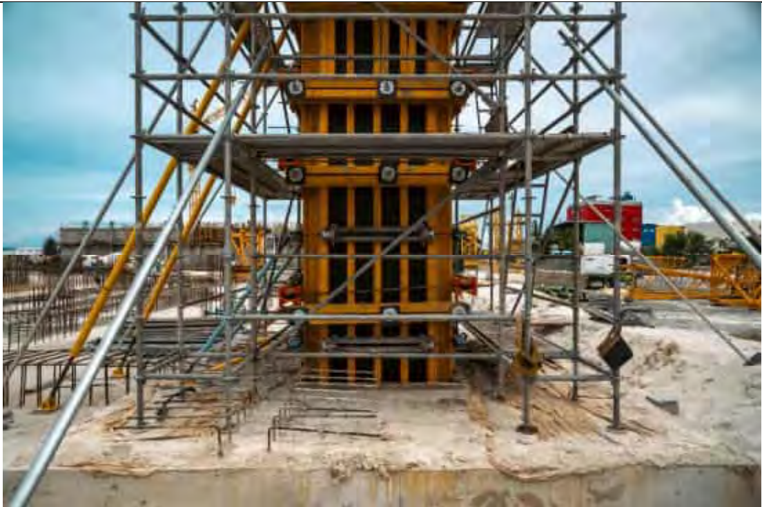
MOCKUP FOR COLUMN SUPPORT AND FORMWORK AT APC AREA.
