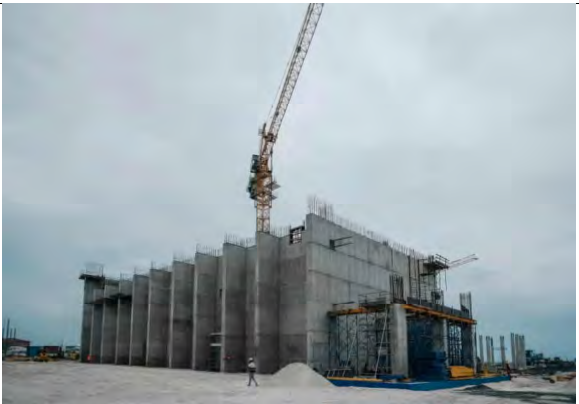
BUNKER AREA - OVERALL BUNKER WALL 7 th LAYER 100% COMPLETED.
