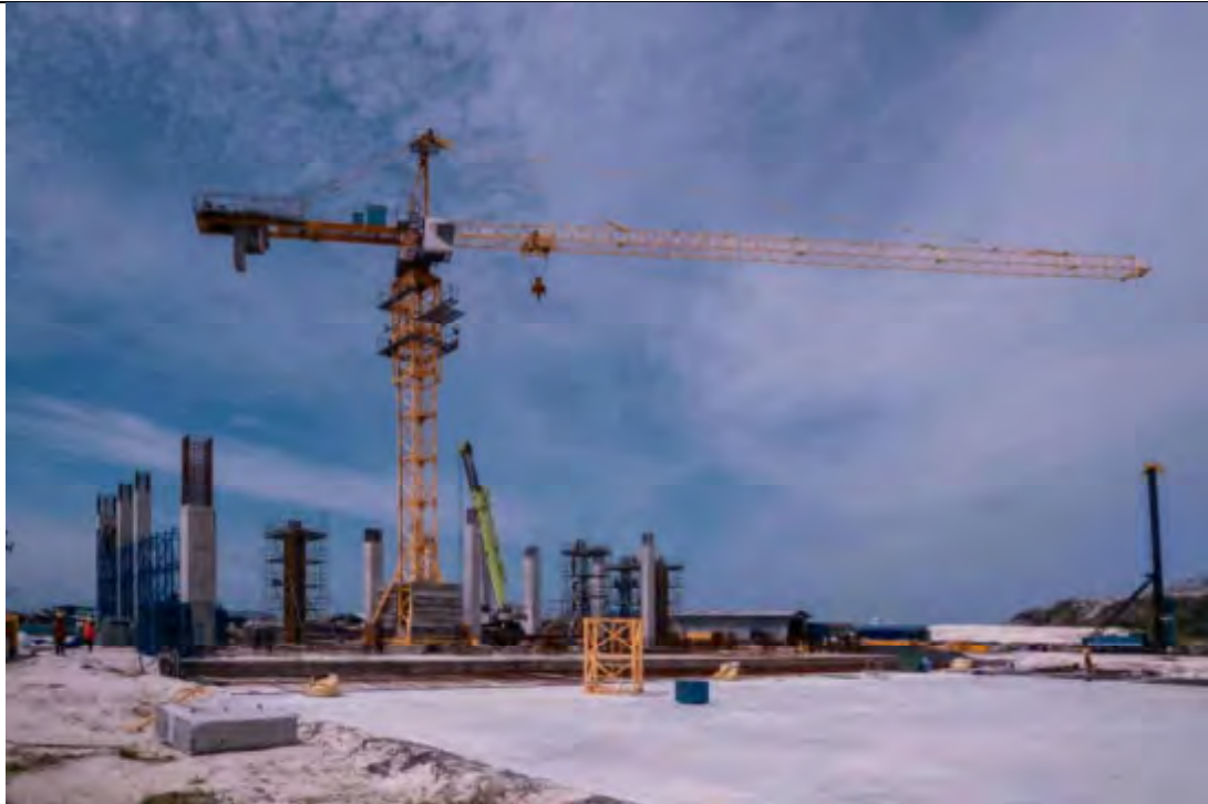
TOWER CRANE INSTALLATION COMPLETED AT APC AREA 1
