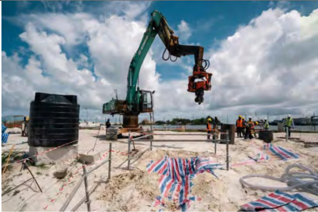
CHIMNEY AREA - TEST BORED PILE IN PROGRESS.
