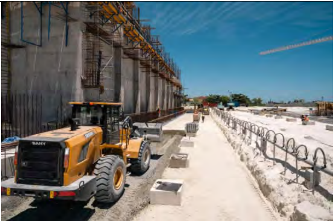
INCINERATOR AREA - STRUCTURAL BACKFILLING IN PROGRESS
