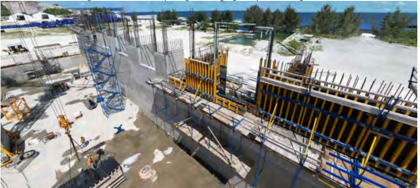
Photo 07 09/07/24 – The scaffolding at the bunker area is regularly inspected for safety.
