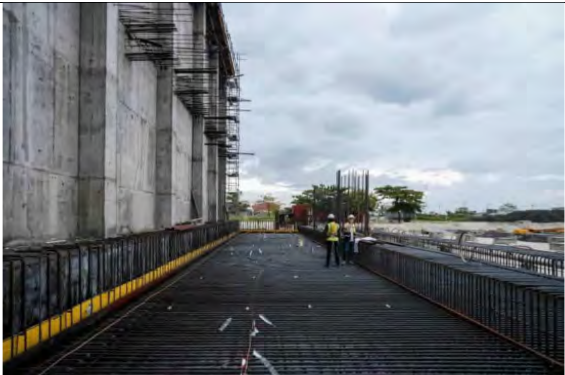
INCINERATOR AREA - AREA 11 REINFORCEMENT BAR AND FORMWORK IN PROGRESS.
