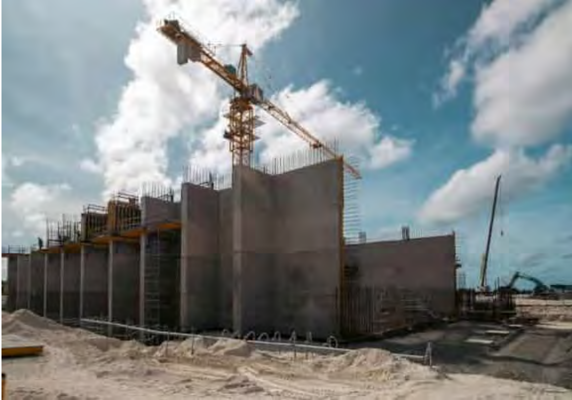
BUNKER AREA - OVERALL BUNKER WALL 4 th LAYER COMPLETED 75%
