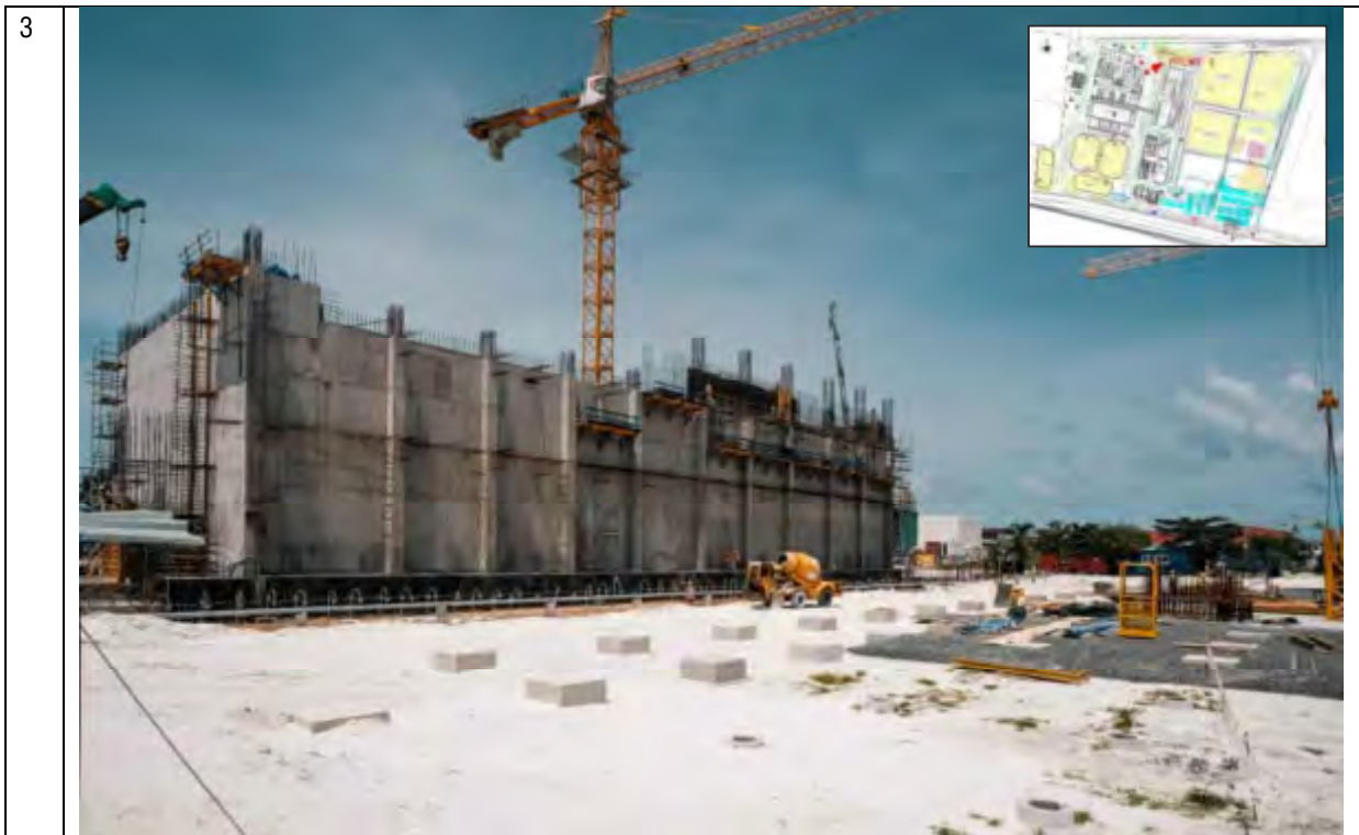
OVERALL - POINT THREE
