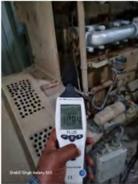
Batching Plant Generator
