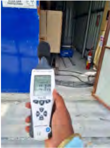
Batching Plant Generator
