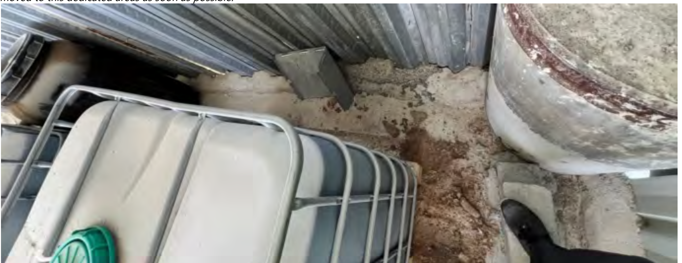
Photo 21 18/07/24– Chemical storage area, proper bund wall needs to be in place all around the storage area and all chemicals need to be moved to this dedicated areas as soon as possible.
