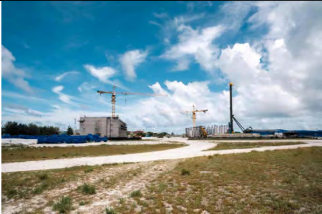
OVERALL VIEW FROM EAST SIDE
