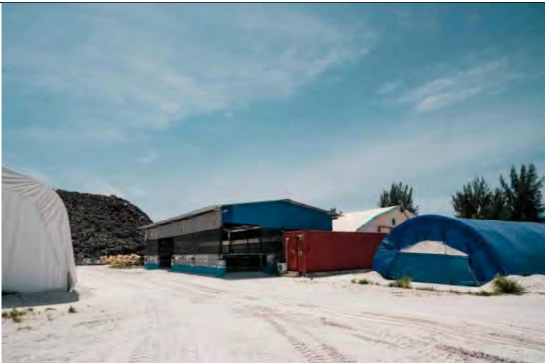
CHEMICAL STORAGE PREPARATION IN PROGRESS
