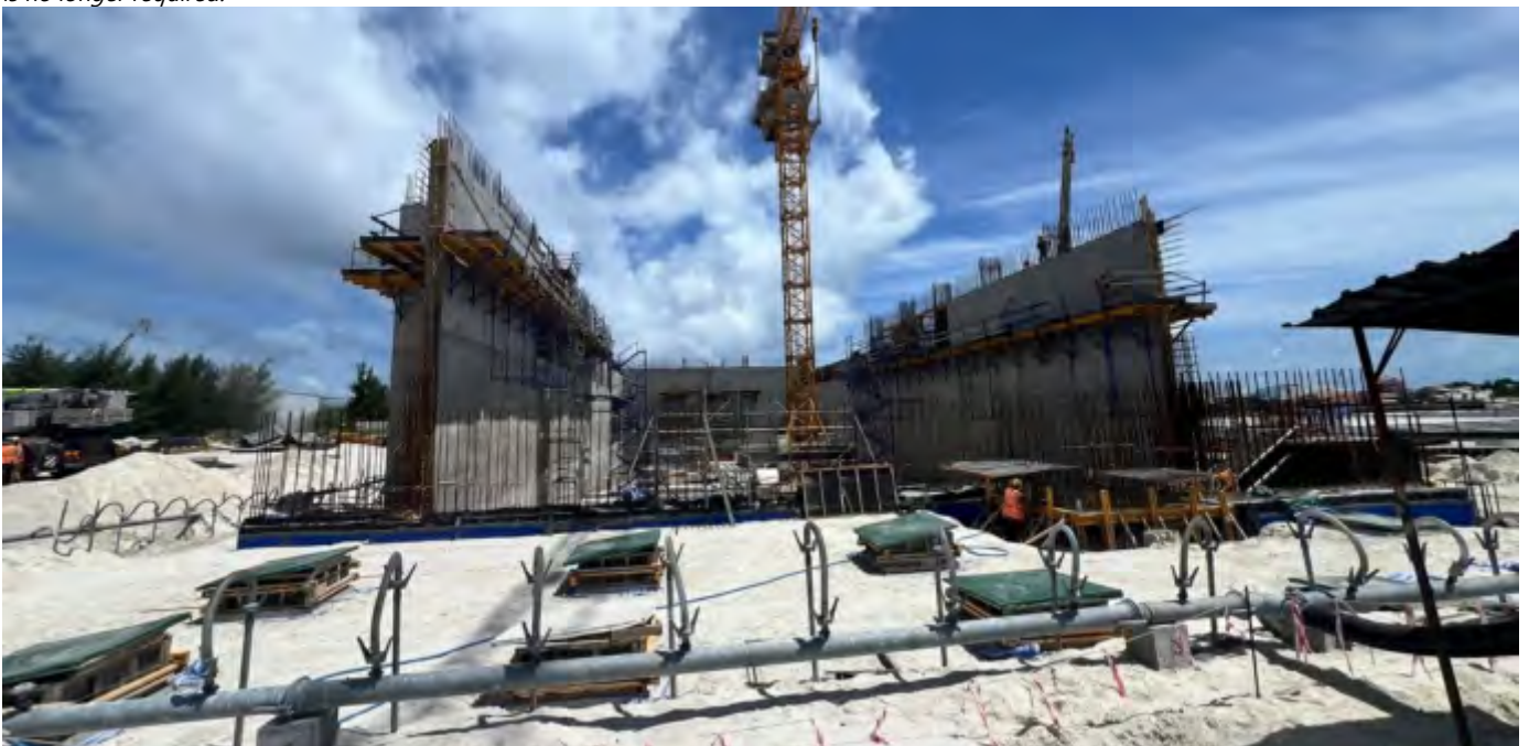
Photo 03 18/07/24 – Construction work on the bunker walls is ongoing as planned.
