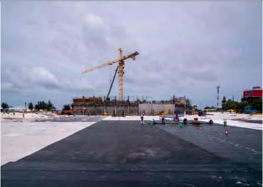
APC AREA - WATERPROOFING WORK 100% COMPLETED AT AREA 1.
