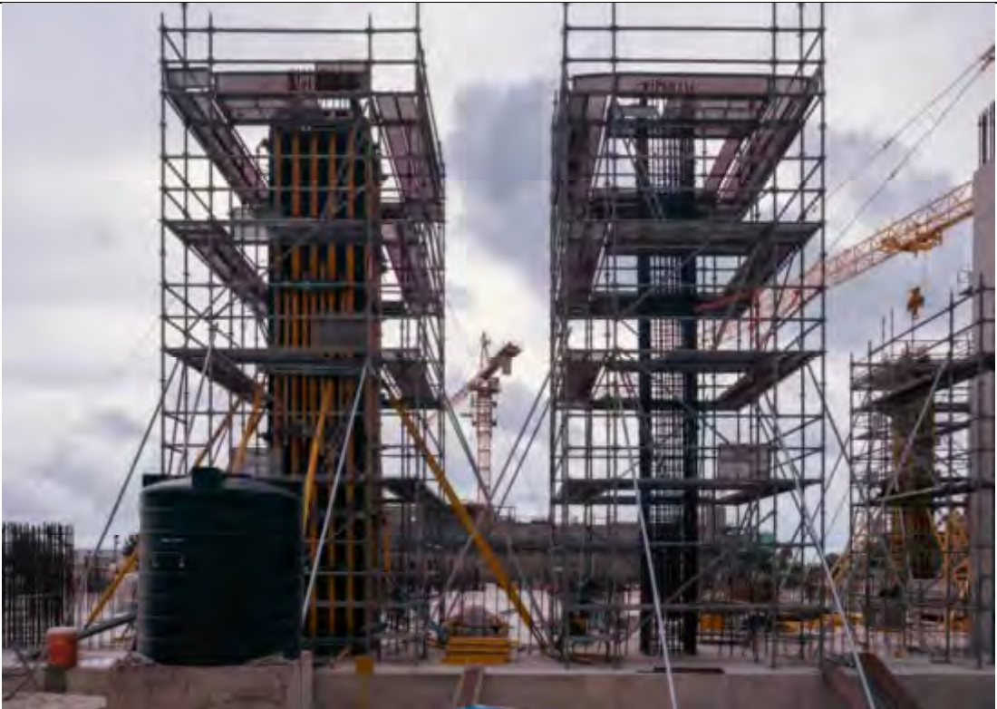
APC AREA - AREA 1, 2 & 3 CONCRETE CASTING FOR COLUMNS IN PROGRESS.
