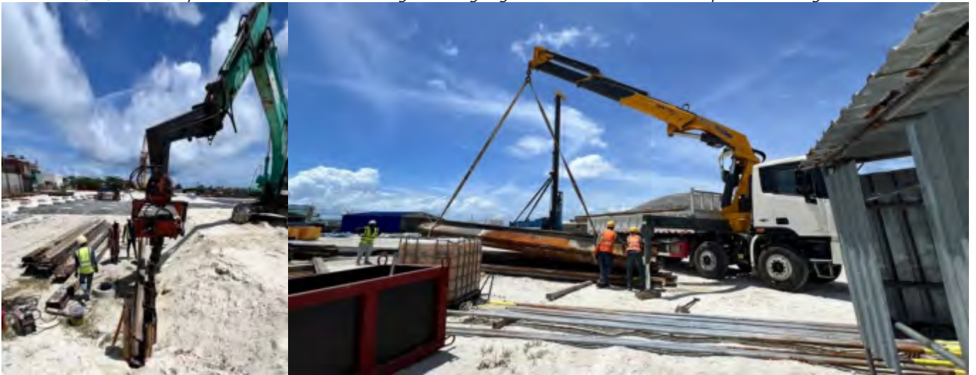
Photo 05 18/07/24 – Sheet pile works are ongoing for the turbine foundation area.
