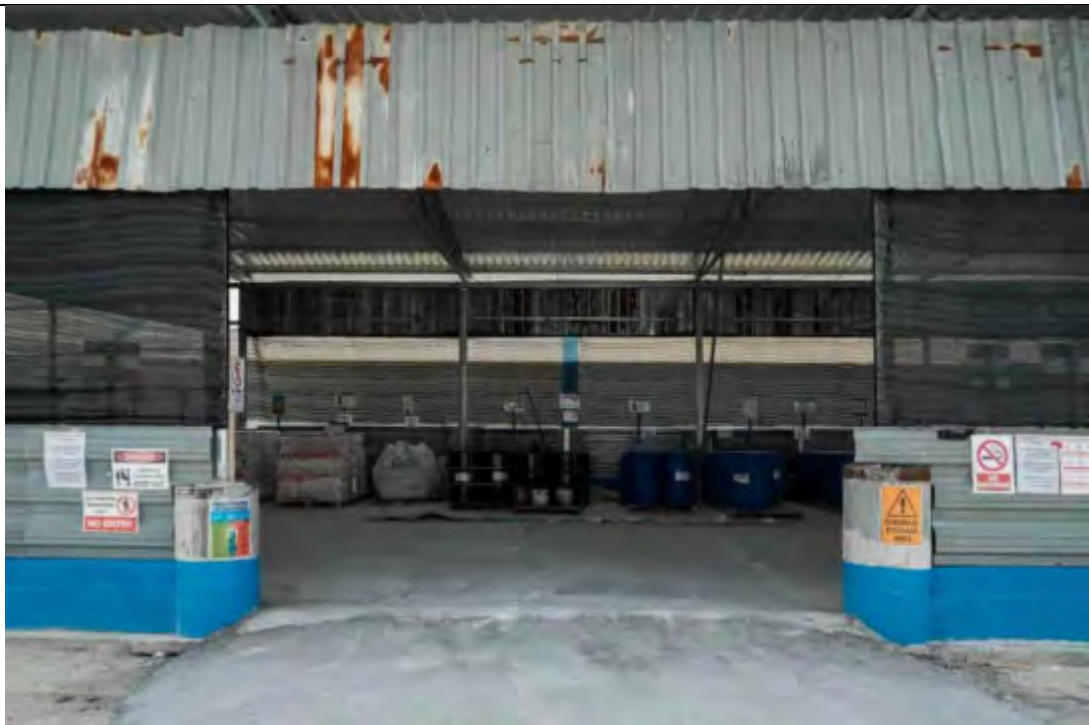
NEW CHEMICAL STORAGE COMPLETED. PENDING INSPECTION
