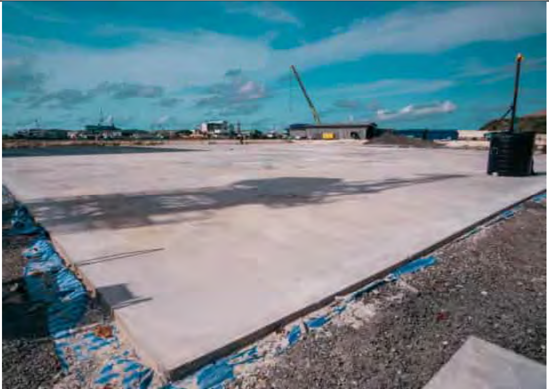
BOILER AREA - BACKFILLING 100% COMPLETED, LEAN CONCRETE 100%.
