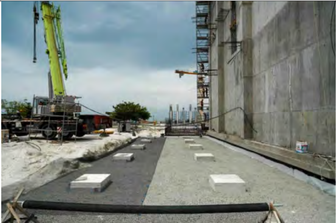
BUNKER WEST SIDE - PILECAPS COMPLETED. BACKFILLING WORK IN PROGRESS
