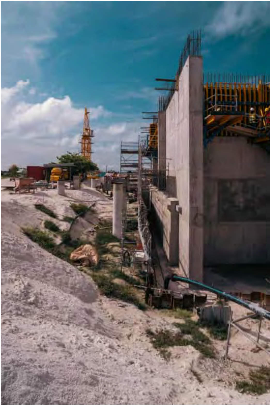
BUNKER WEST SIDE
