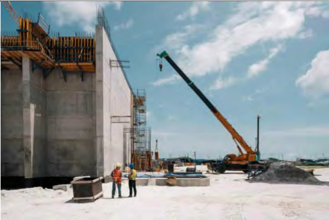
BUNKER EAST SIDE - REINFORCEMENT BAR FOR LIFT SHAFT IN PROGRESS.
