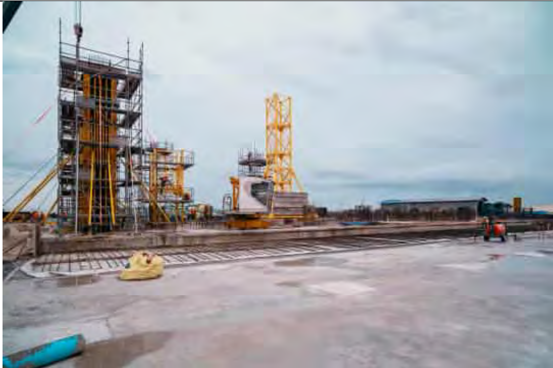
TOWER CRANE INSTALLATION IN PROGRESS AT APC AREA 1.
