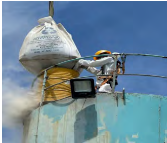
Figure 12: Status of PPEs during transferring cement and fly ash from bags to hoppers of batching plant
