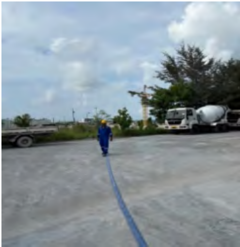
Discharge of Waste water from sedimentation tank in batching plant to adjacent land owned by third party observed during site visit in July month for inspection
