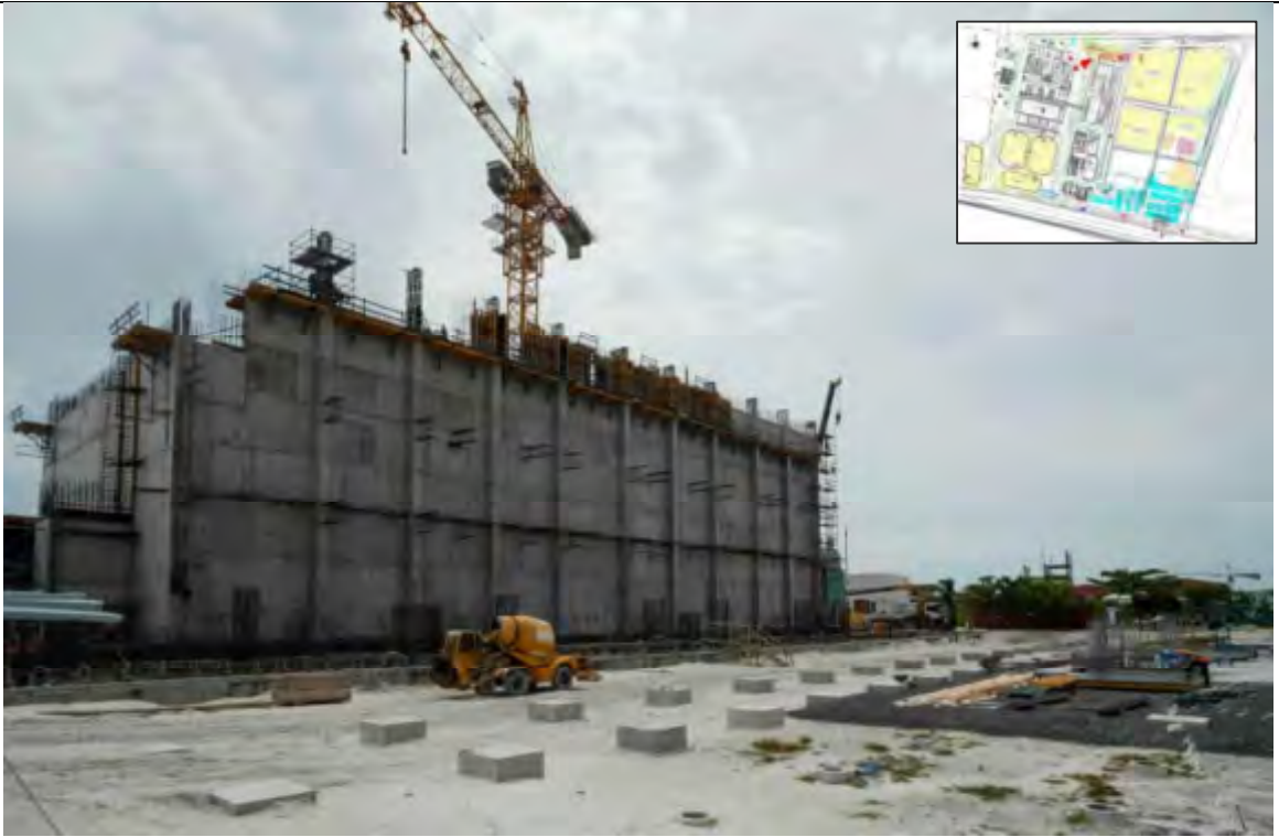
OVERALL - POINT THREE
