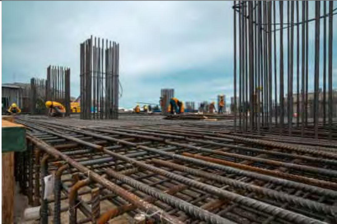
APC AREA - REINFORCEMENT BAR AND FORMWORK AREA 2 IN PROGRESS.
