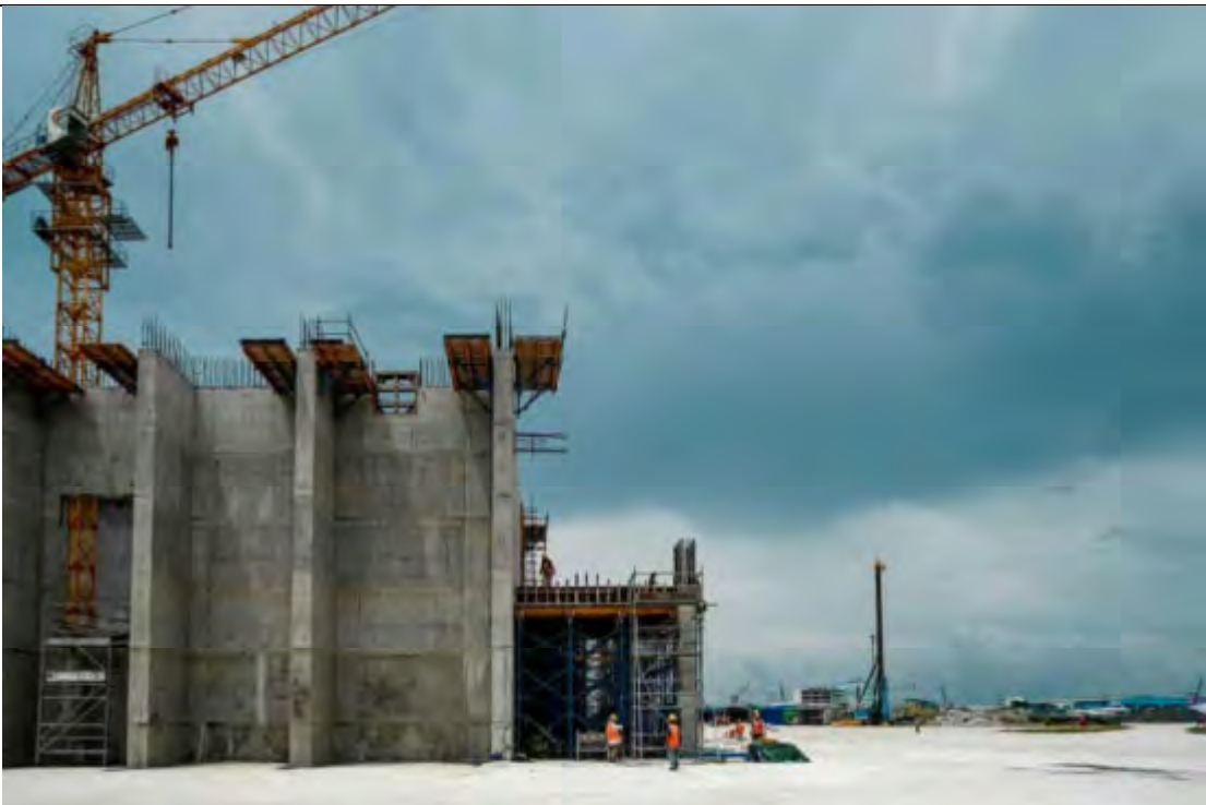
BUNKER EAST SIDE - BEAMS PREPARATION IN PROGRESS
