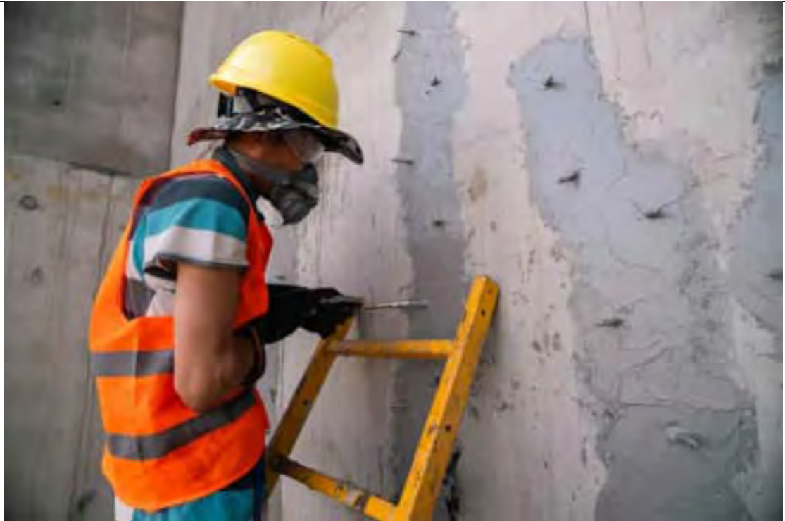
CRACK REMEDIAL WORK FOR EXTERNAL BUNKER WALL.
