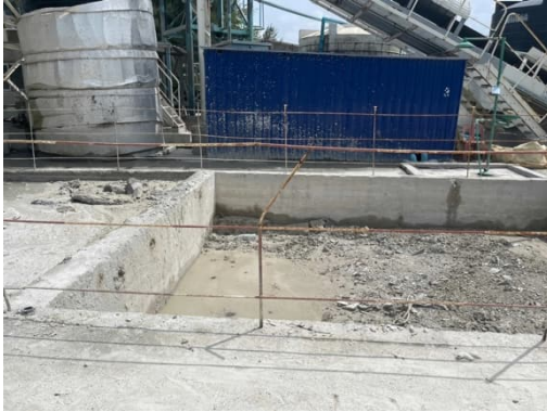
Figure 7: Waste concrete wash pits on two different visits
